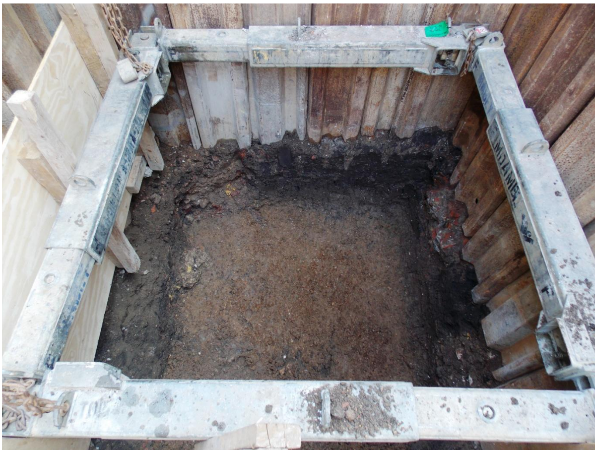
Plate 1: Trench overview at the level of the natural gravel [3], facing east.
