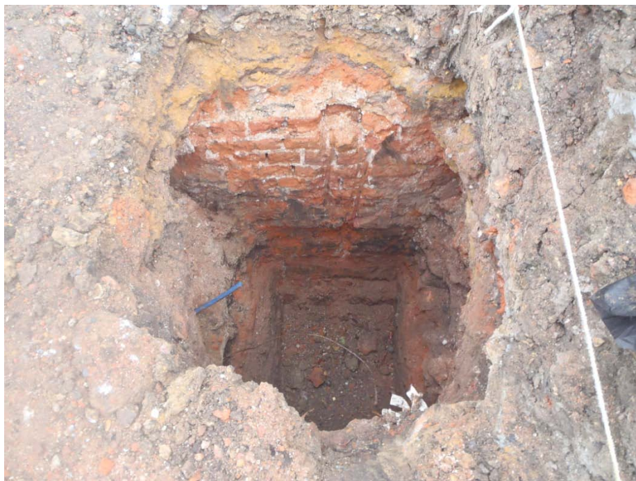
Plate 4: Pad Hole 18, Chalk Footing With Wall On Top, View - West
