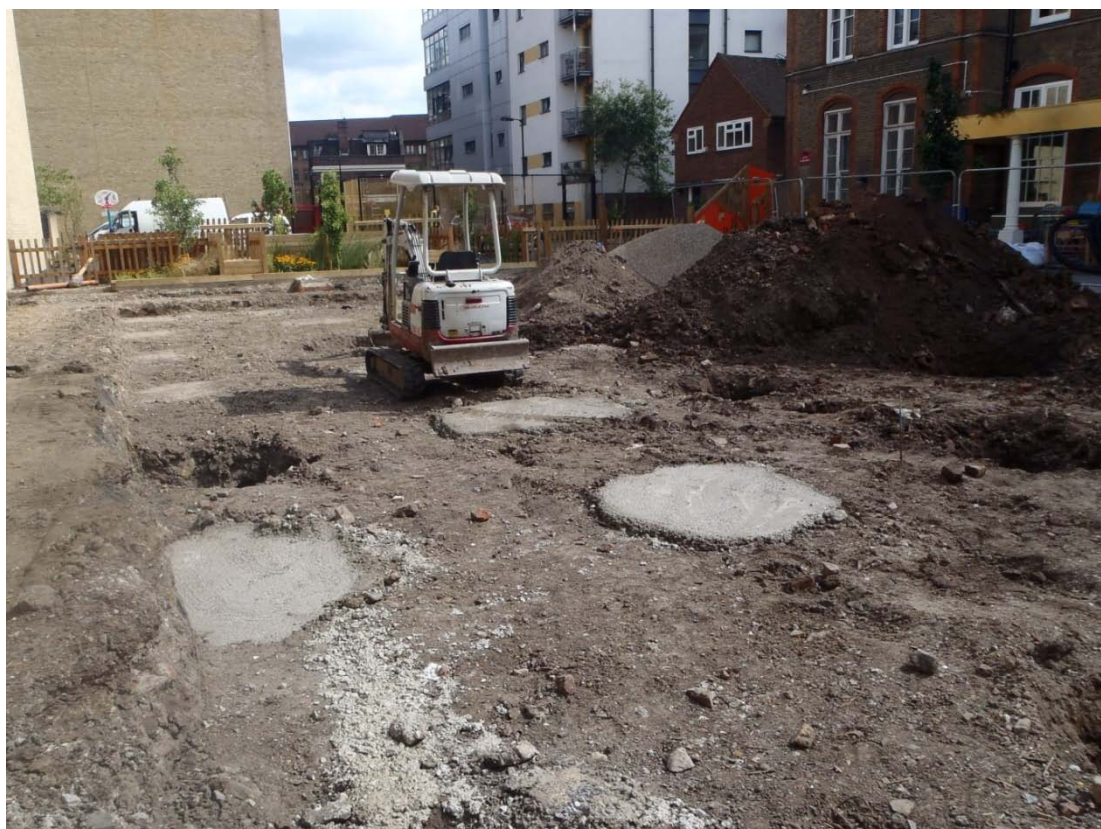
Plate 5: General Site View, Post Excavation, View - East
