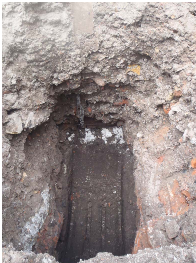
Plate 4: Pad Hole 18, Chalk Footing With Wall On Top, View - West
