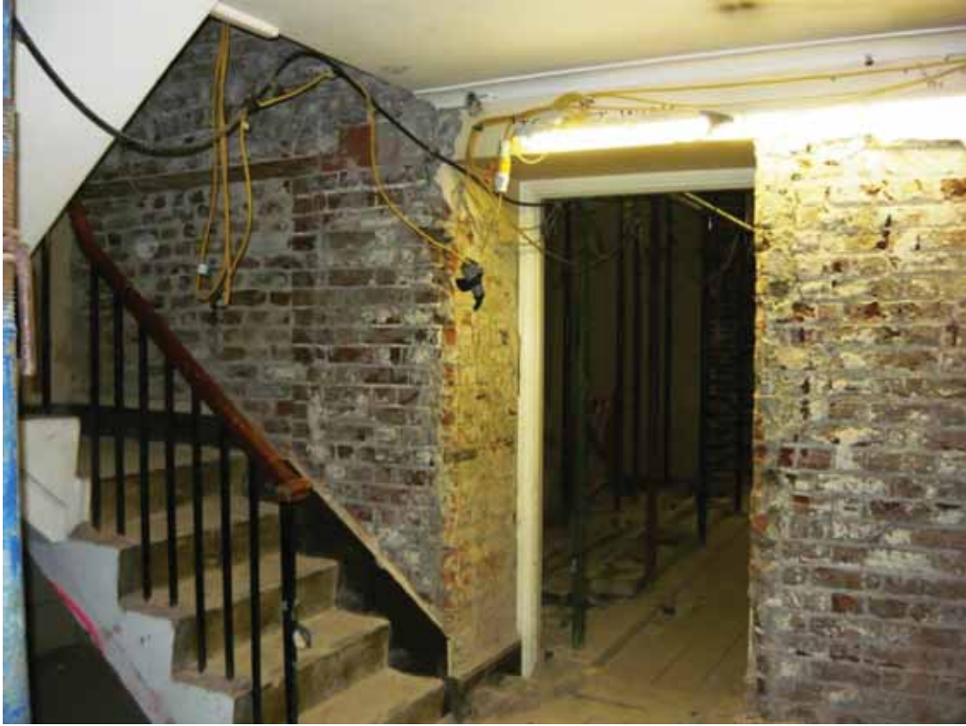
Plate 253: North wall of Corridor 06LG looking north (EAF10 BHD7 (16))
