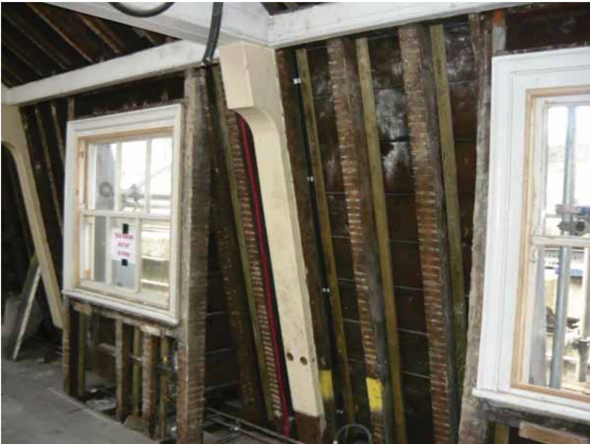
Plate 689: West wall of Room T08, looking south-west (EAF10 BHD10 (76))
