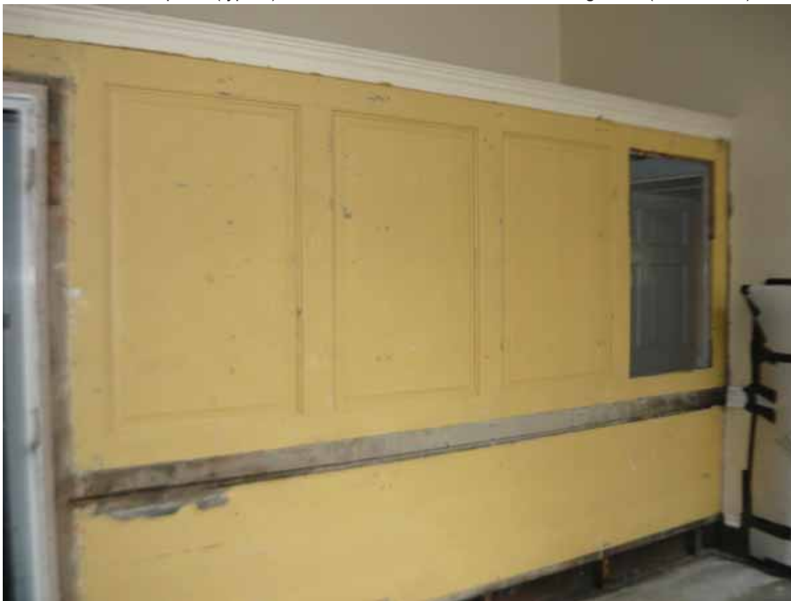
Plate 547: West partition wall in Room F27, looking north-west (EAF10 BHD3 (21))
