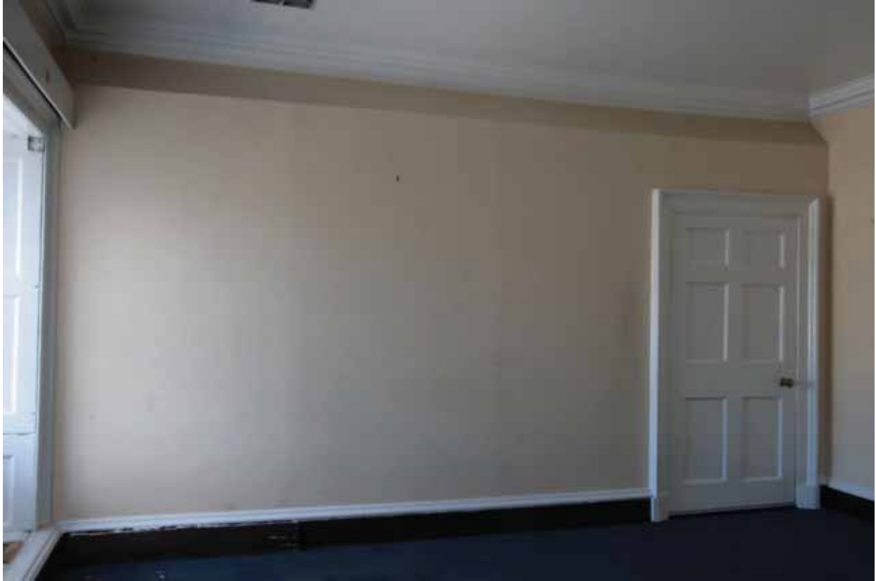
Plate 563: North partition wall in Room S02, looking north (EAF10 150)
