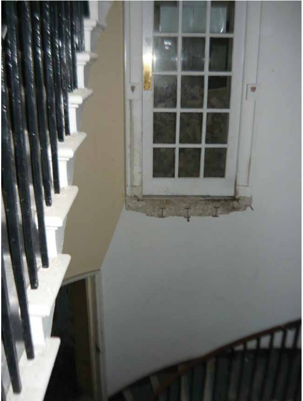
Plate 237: Removed link bridge in Stairs 02LG looking north (EAF10 BHD3 (44))
