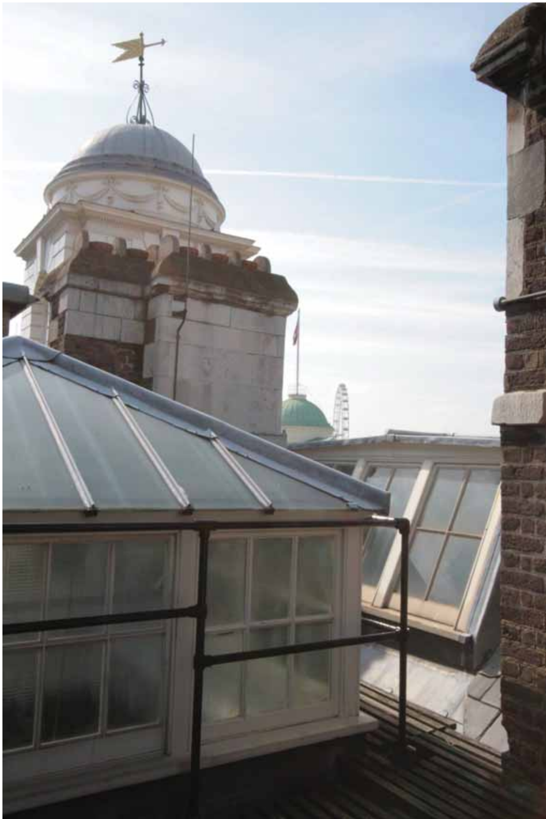
Plate 799: Lantern skylight over the Corridor 03T, looking south-west (EAF10 24)
