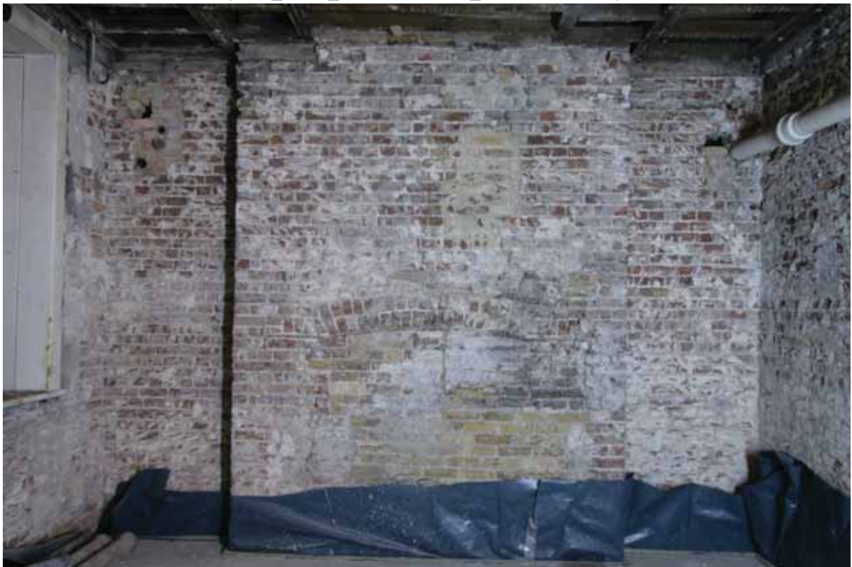
Plate 12: North wall of Room B44, looking north (EAF10 A100 036)
