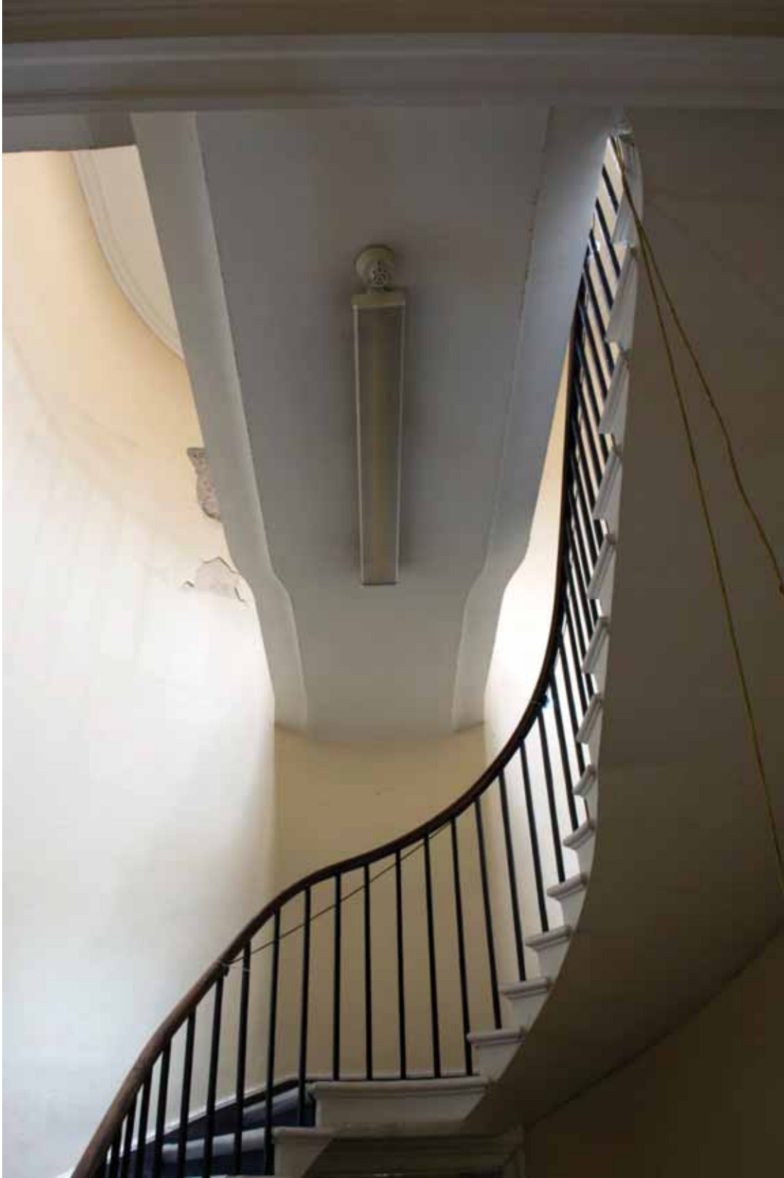
Plate 598: Underside of link bridge in Stairs 02S looking north (EAF10 B100 0957)
