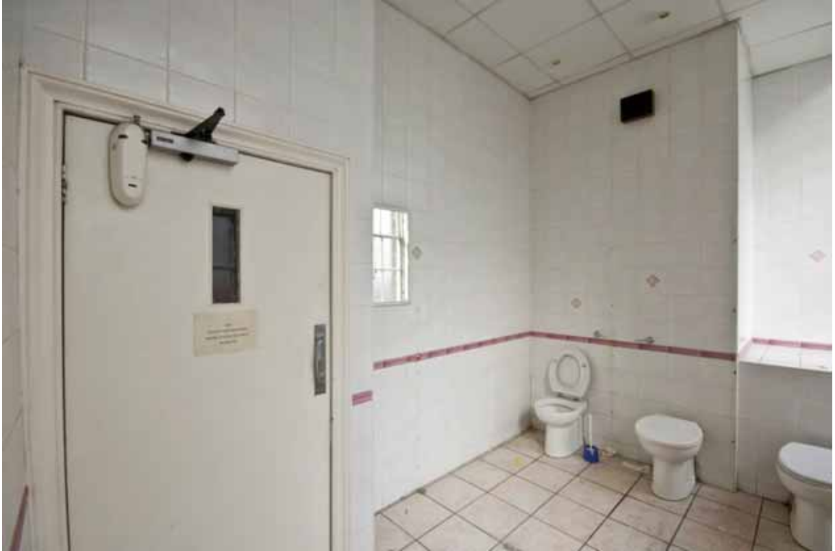
Plate 422: West (left) and north (right) partition walls in Room G20, looking north-west (EAF10 B100 0887)
