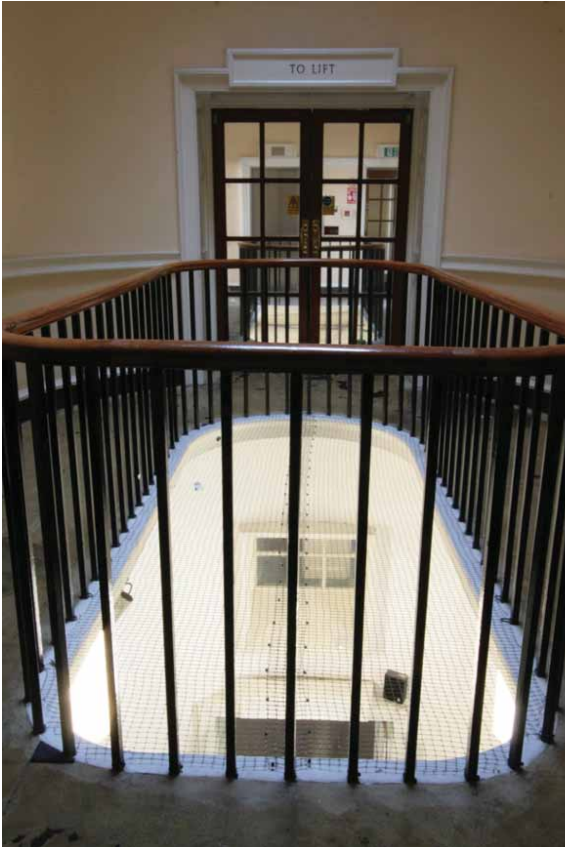
Plate 495: Lightwell in Corridor 02F looking south (EAF10 159a)
