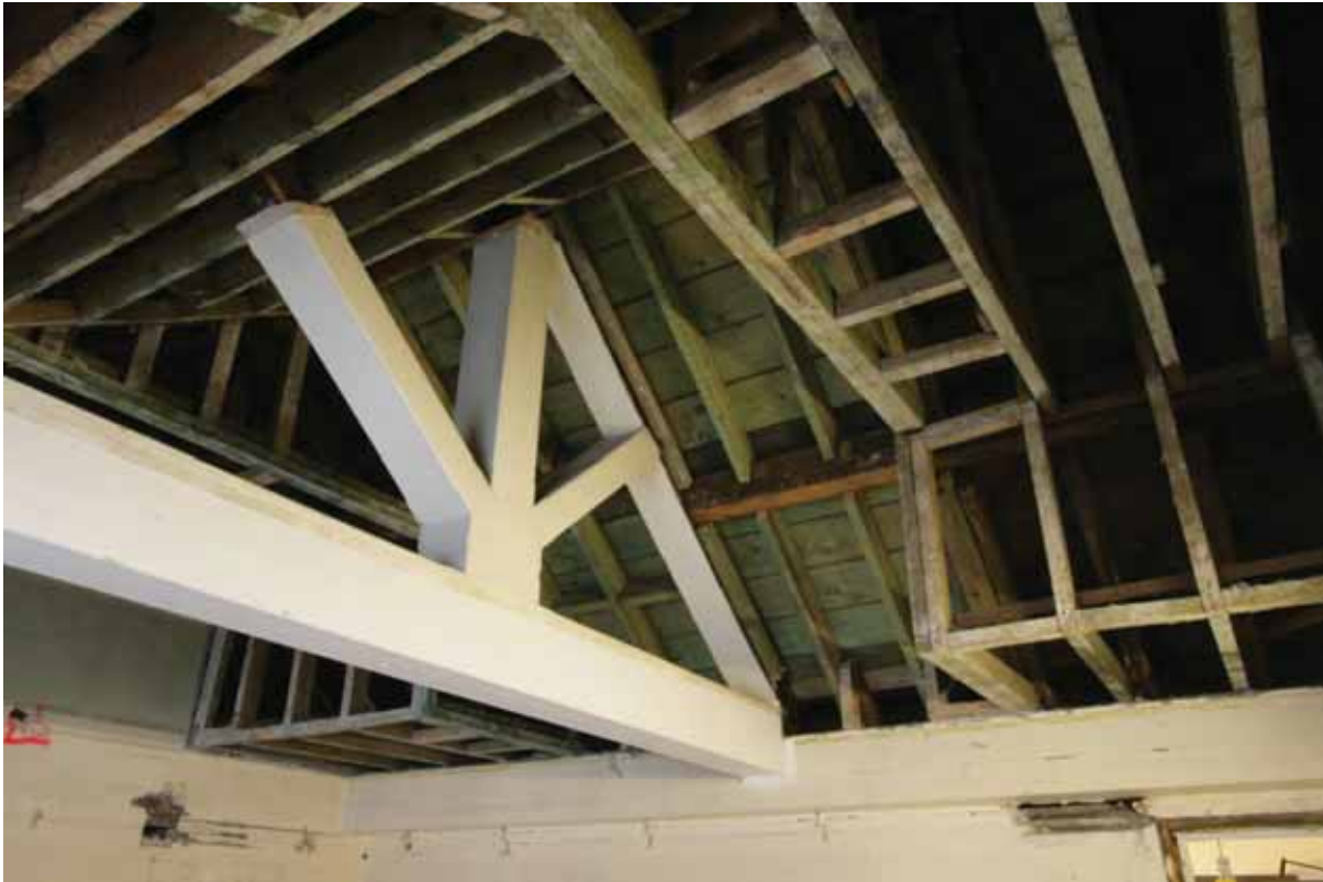
Plate 729: East-west roof truss in Room T115, looking south-west (EAF10 A100 009)
