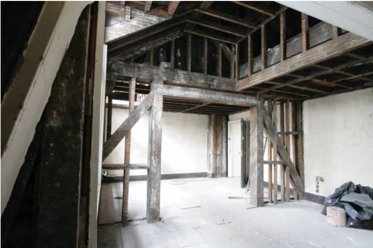
Plate 676: North partition (foreground) wall in Room T03, looking north-east (EAF10 A100 007)
