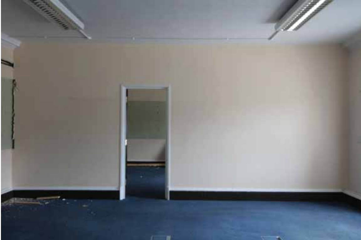
Plate 551: South partition wall in Room S96, looking south (EAF10 159)
