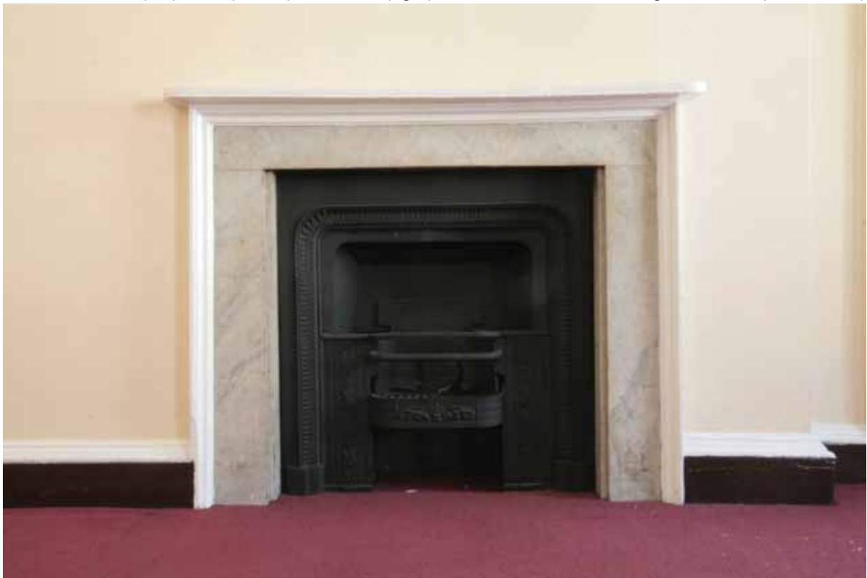
Plate 625: Fireplace (type 3) in the north wall of Room S17, looking north (EAF10 0137)
