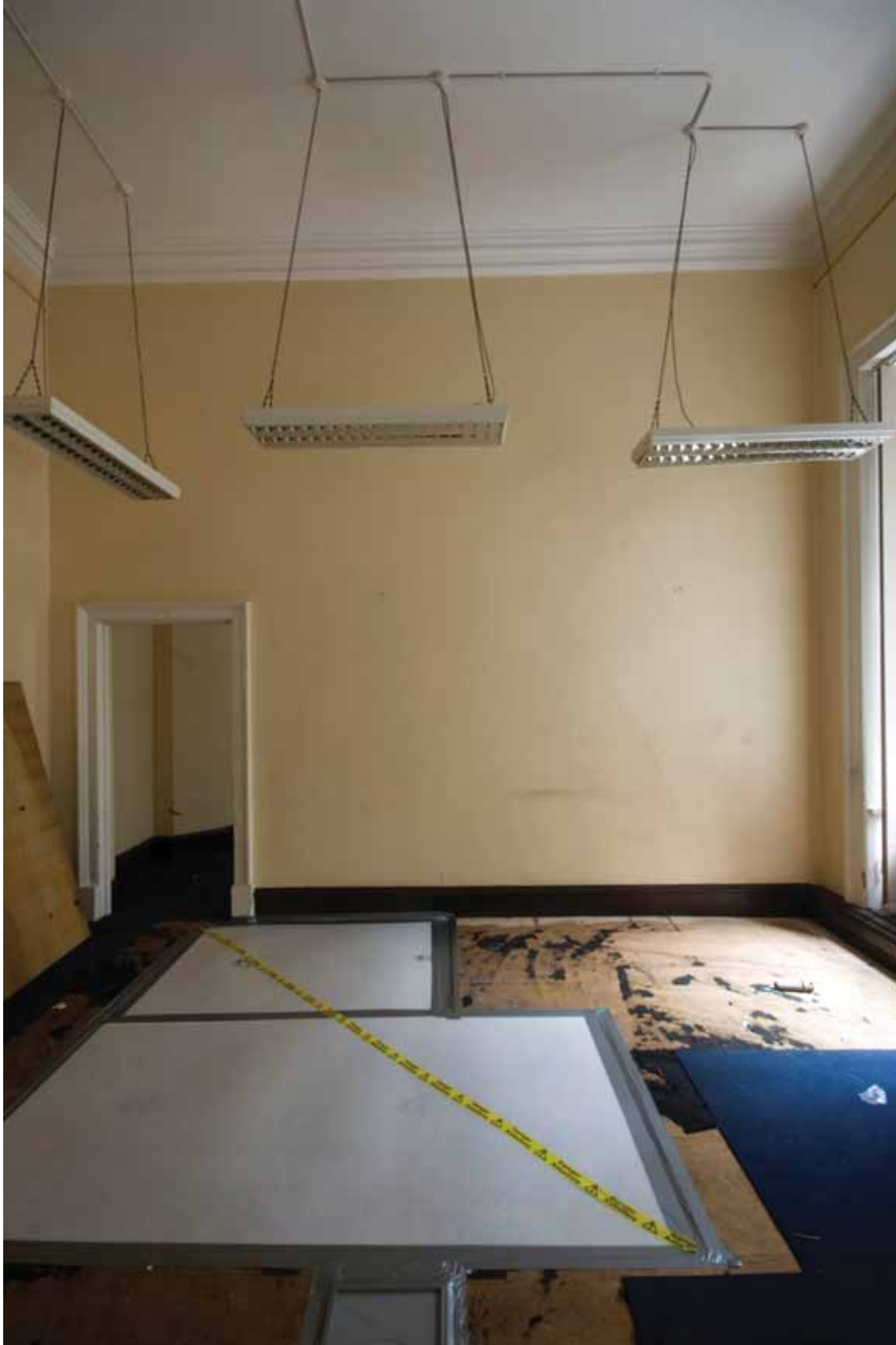
Plate 273: North (partition) wall in Room M21, looking north (EAF10 LG100 1082)
