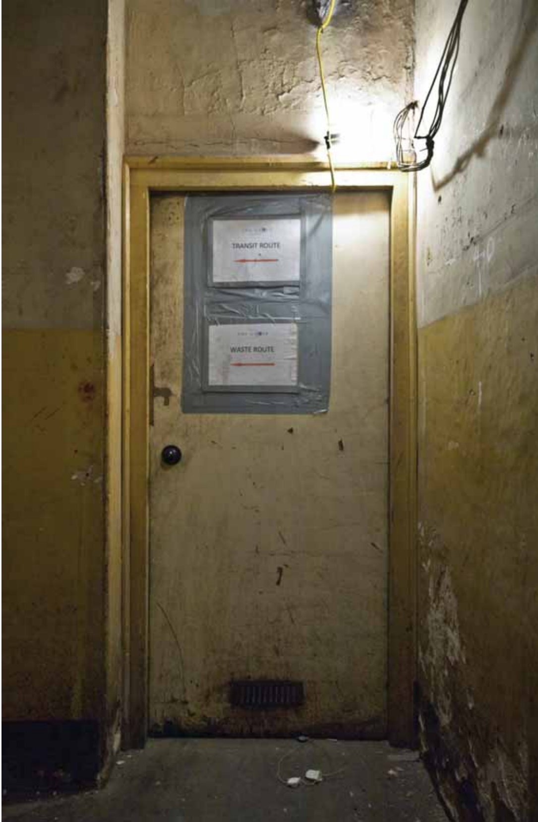
Plate 149: Doorway in the south wall of Room B53, looking south (DSC_1496 _sitecode EAF10_© PCA Ltd 2010 _1)
