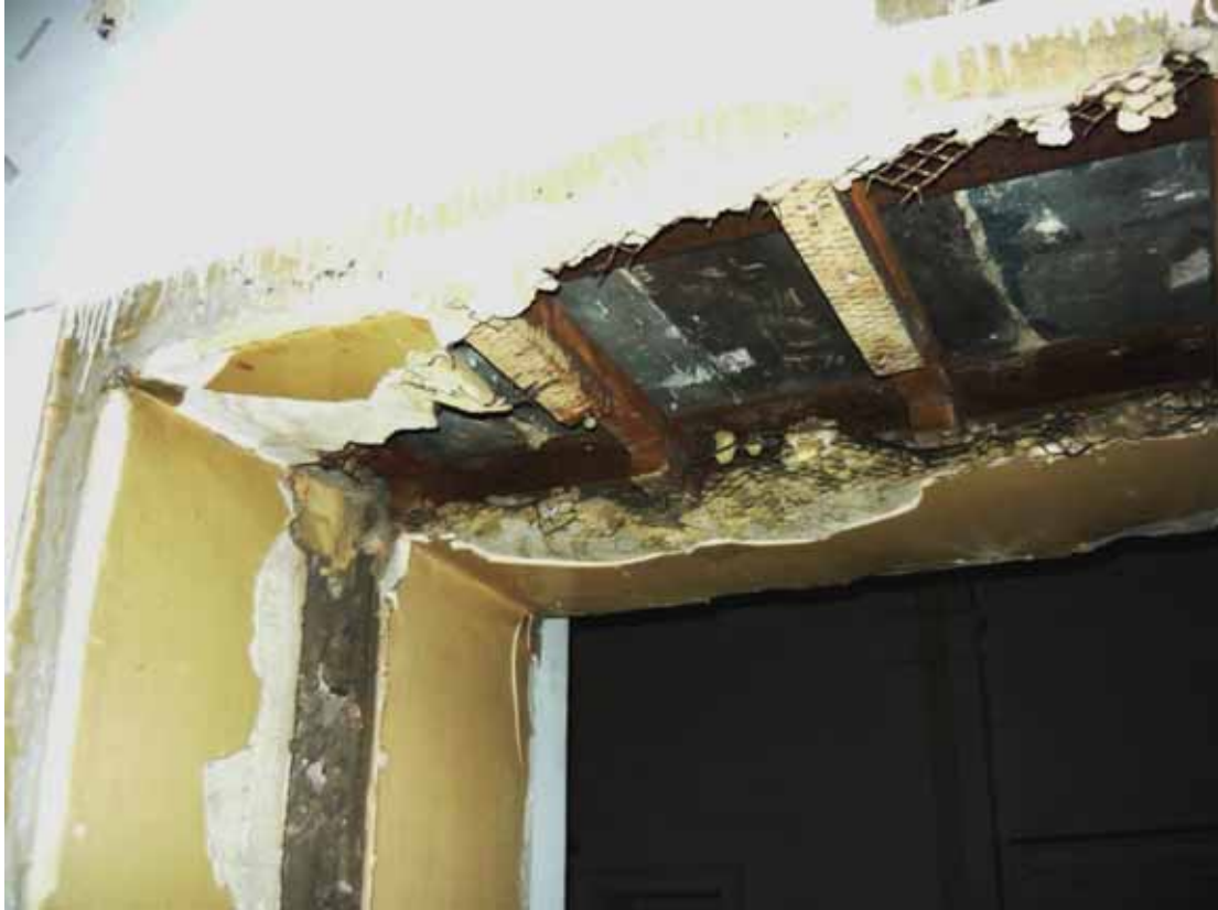
Plate 400: Doorway in the south wall of Corridor 09G looking south-east (EAF10 BHD8 (127))
