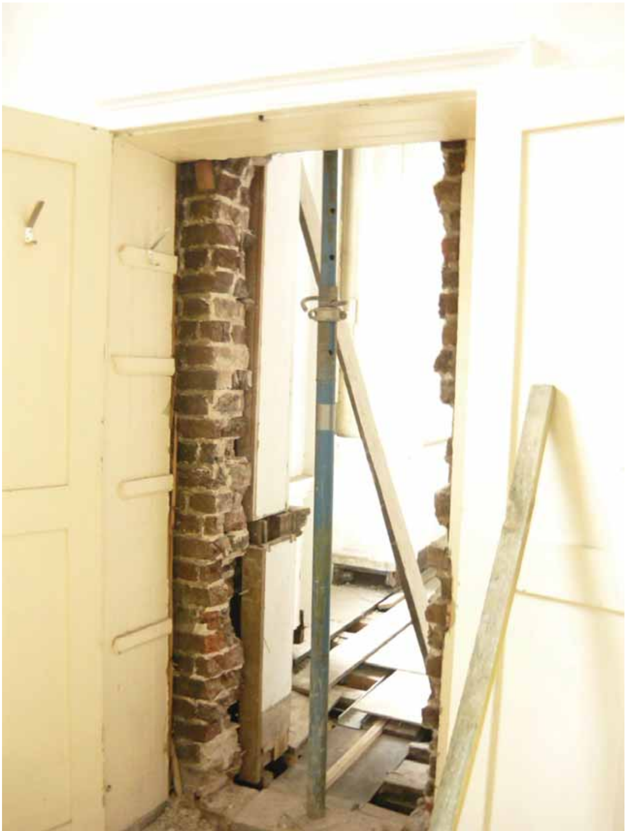
Plate 336: Removed brickwork at the back of a cupboard at the west end of the north wall in Room G42, looking north-west (EAF10 BHD8 (124))
