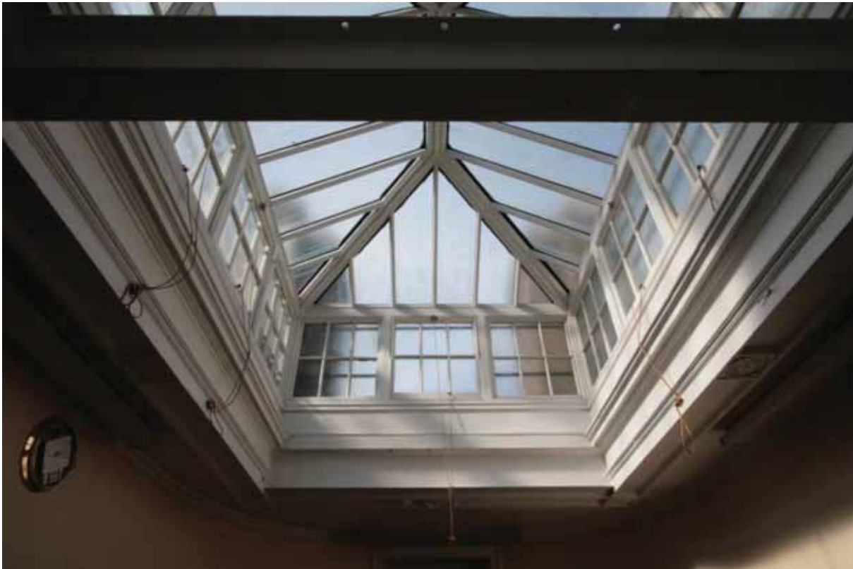
Plate 714: Skylight over Corridor 03T, looking north (EAF10 35)
