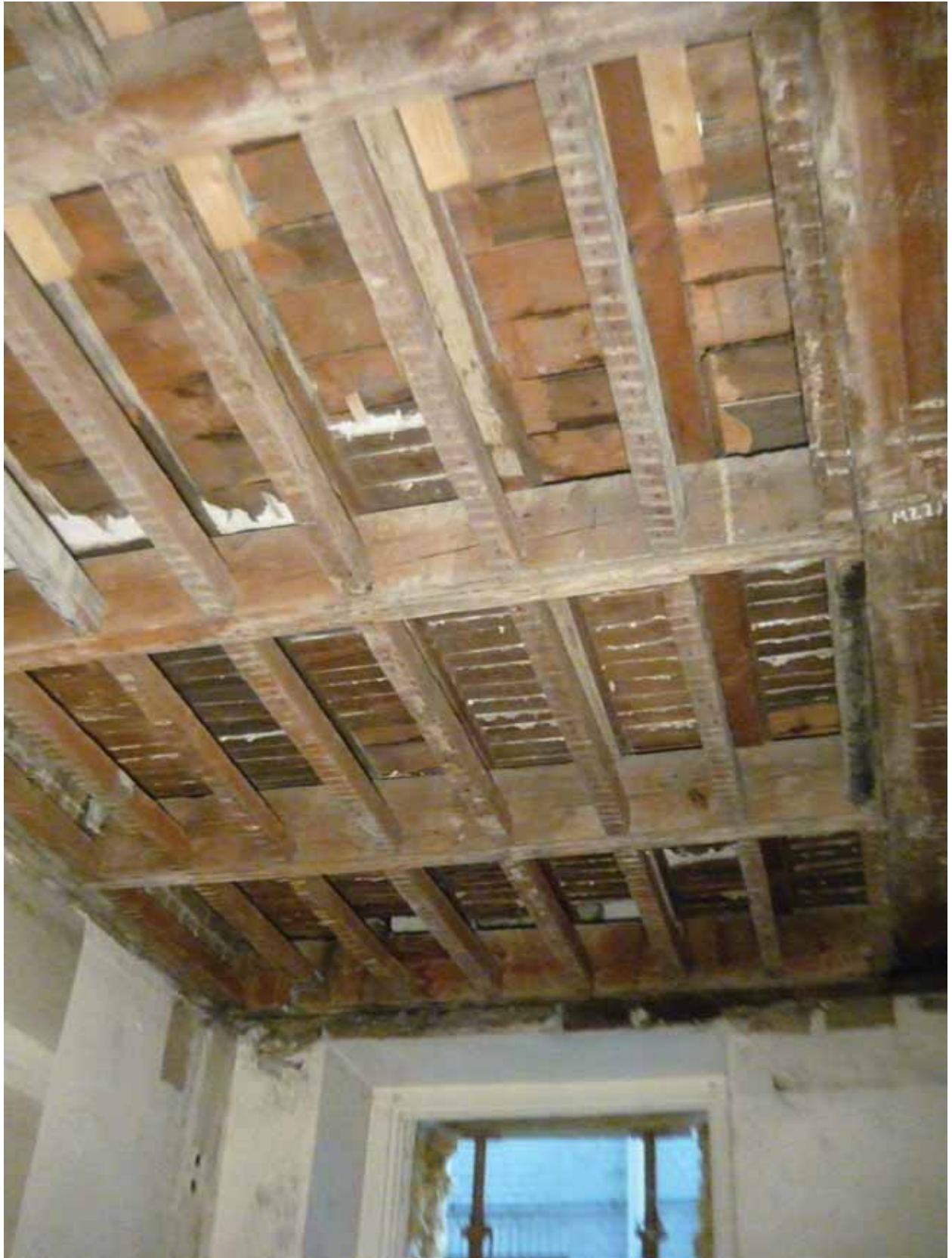
Plate 154: North-east corner of Room B53, looking east (EAF10 BHD5 (176))
