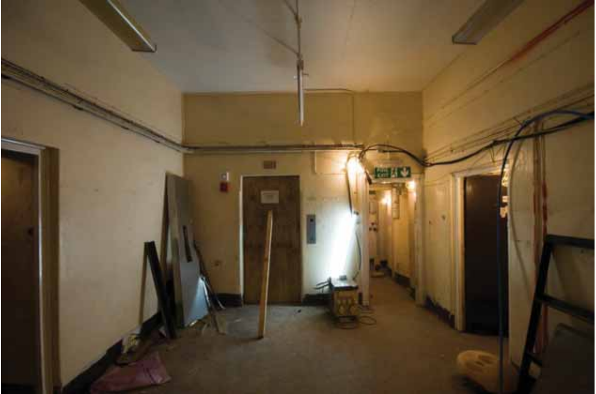
Plate 94: Corridor 3, looking south (DSC_1475 _sitecode EAF10_© PCA Ltd 2010)
