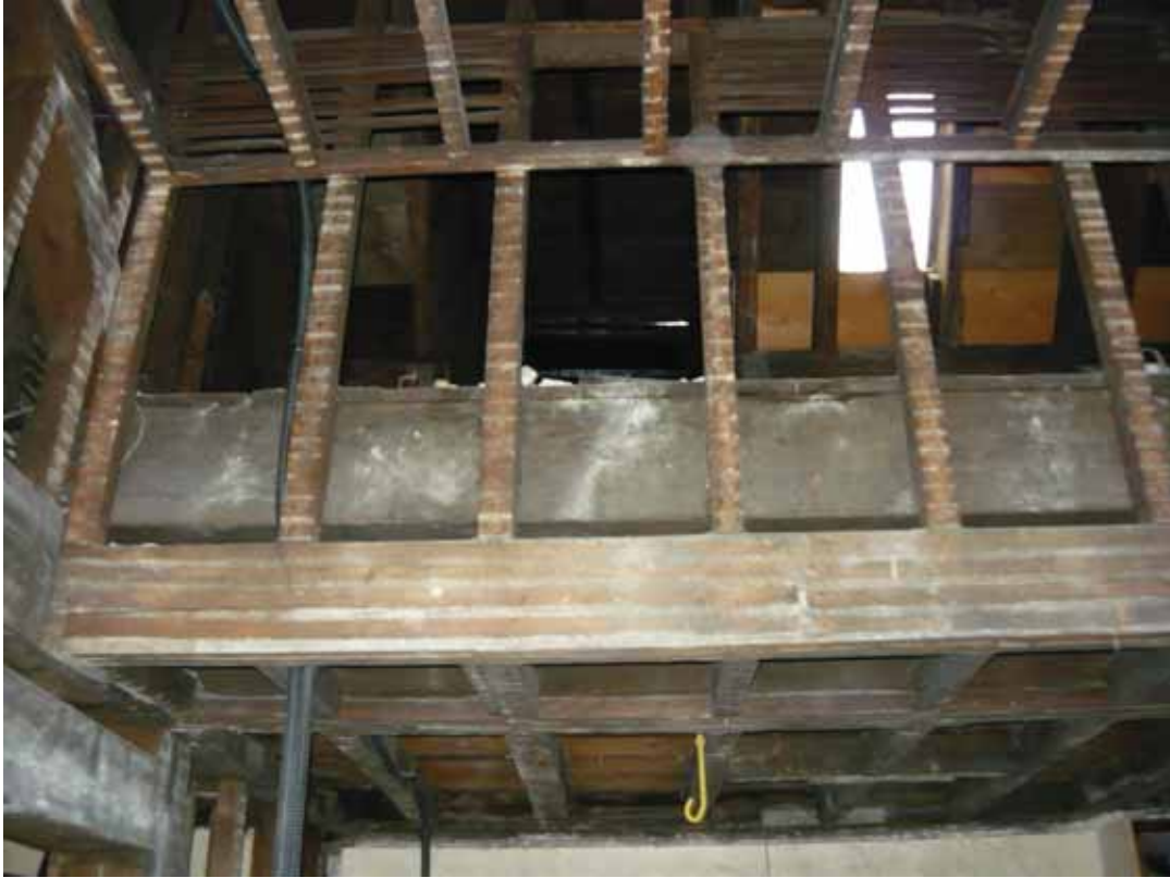
Plate 677: Exposed roof structure above Room T03, looking east (EAF10 BHD10 (63))
