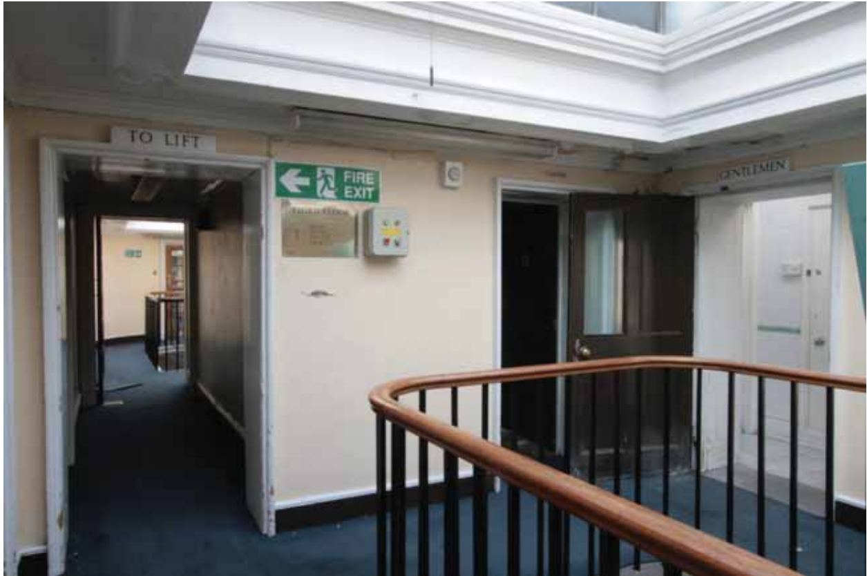
Plate 718: North wall of Corridor 05T, looking north (EAF10 37)
