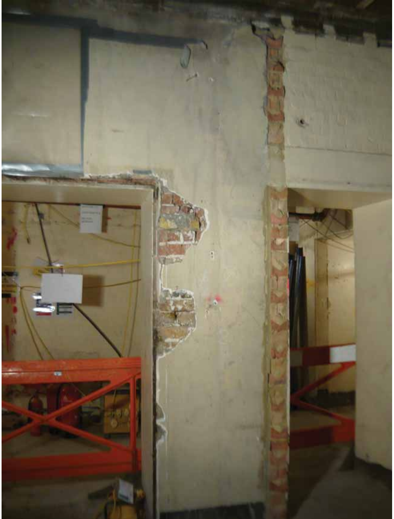
Plate 139: West wall of Room B51, looking west (EAF10 BHD5 (158))
