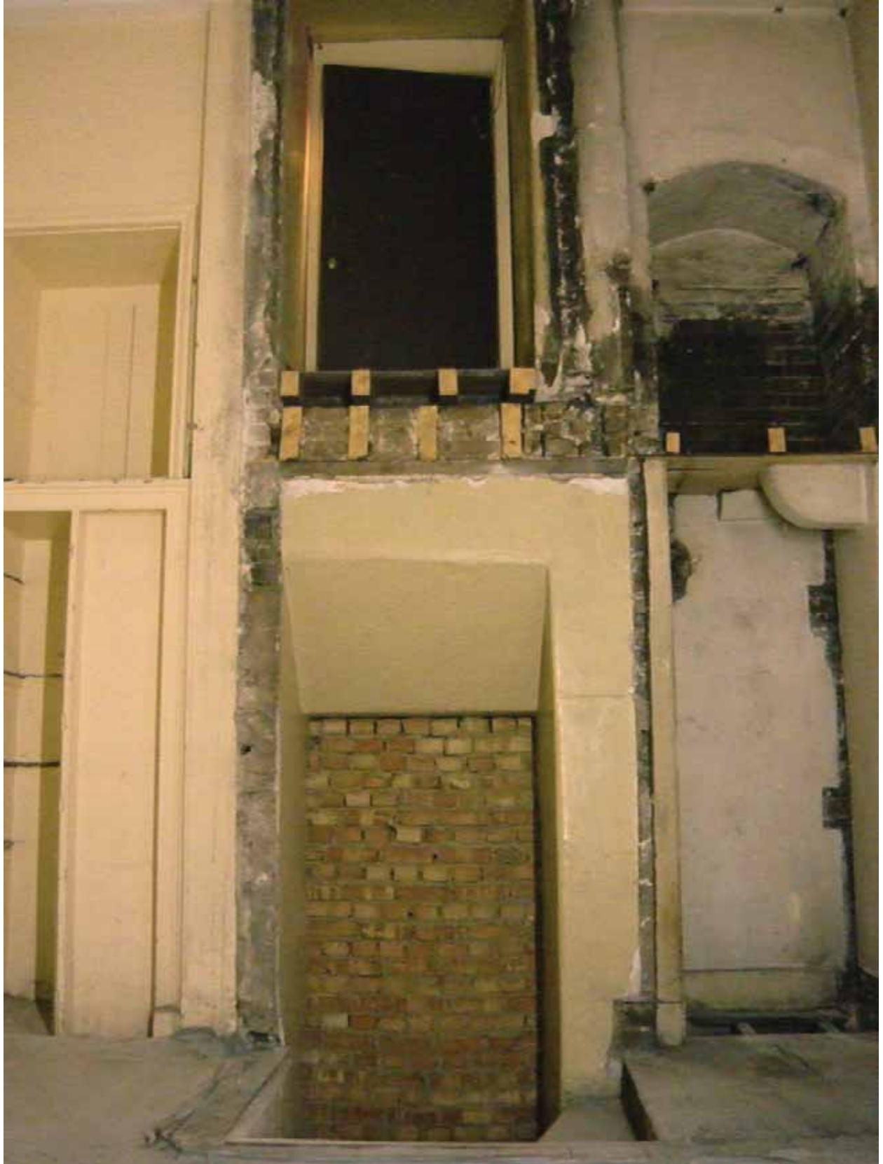
Plate 223: South wall of Room M18, looking south (EAF10 BHD6 (39))
