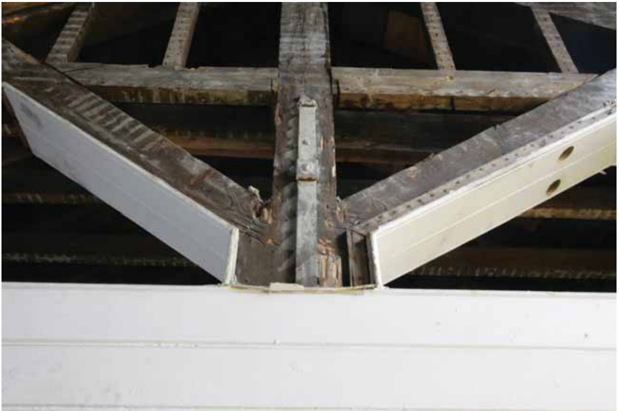
Plate 774: Detail of southern truss in Room T24, looking south (EAF10 A100 006)
