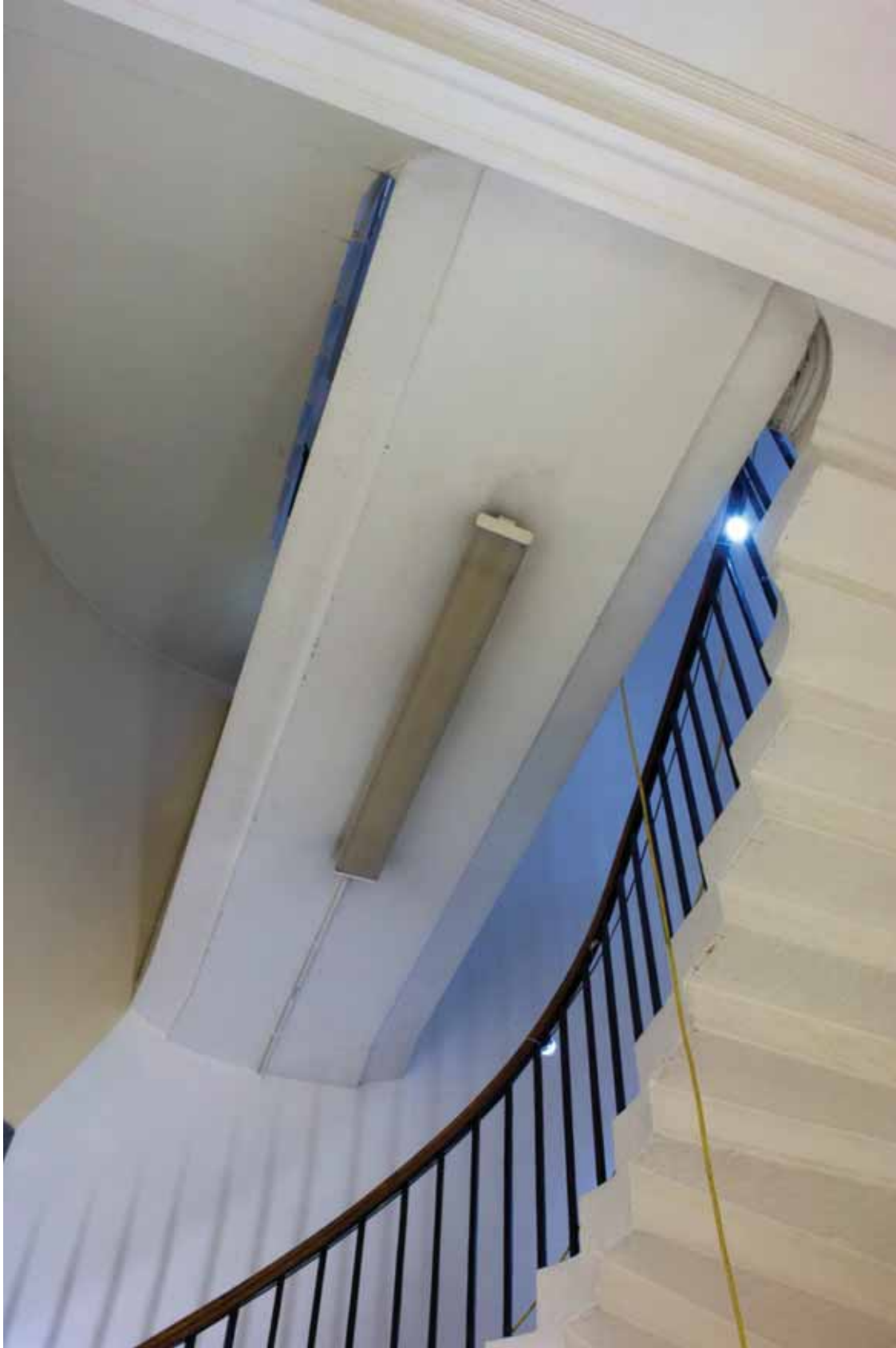
Plate 236: Underside of link bridge in Stairs 02LG looking north (EAF10 LG100 1058)
