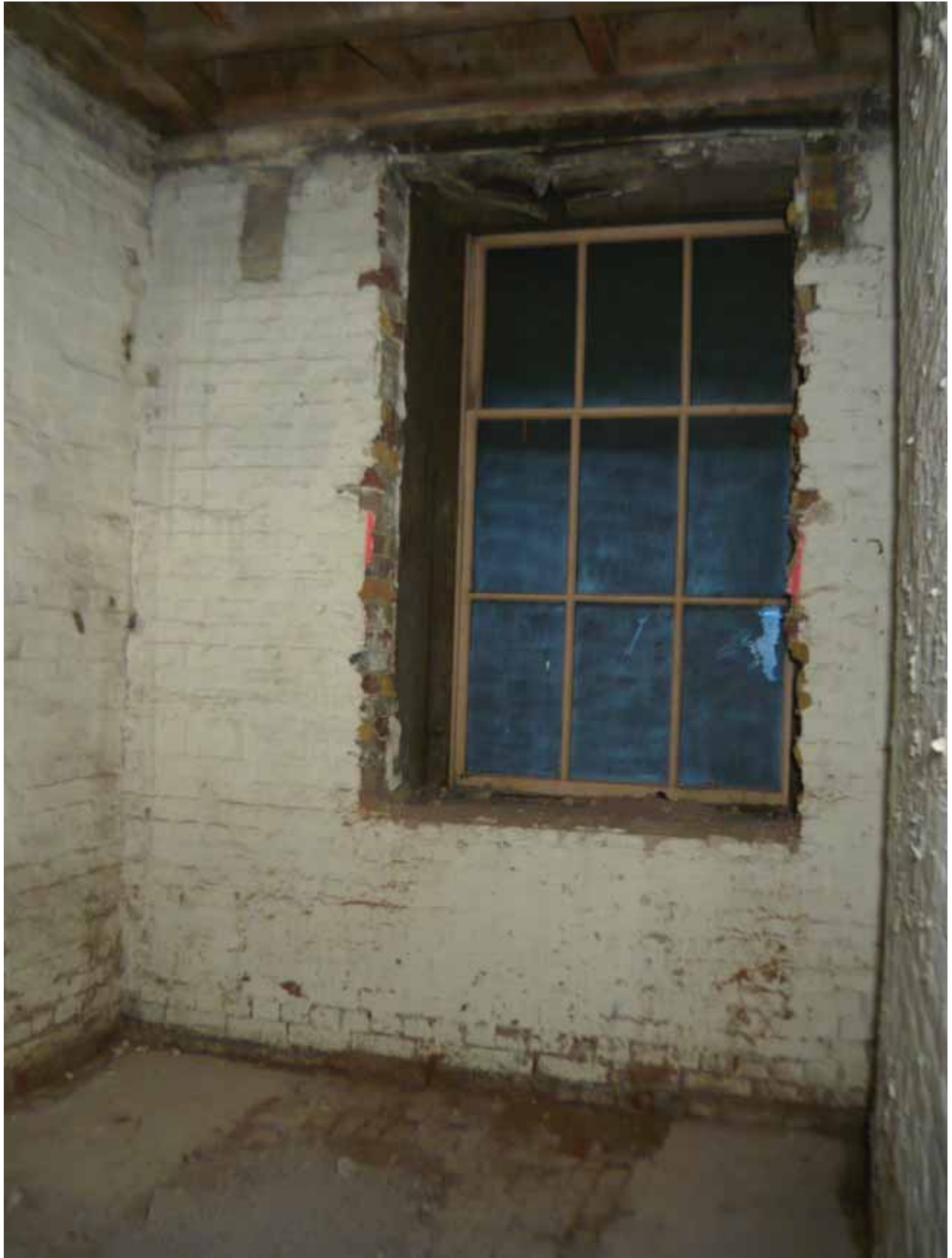
Plate 114: East wall of Room B49B, looking east (EAF10 BHD5 (134))
