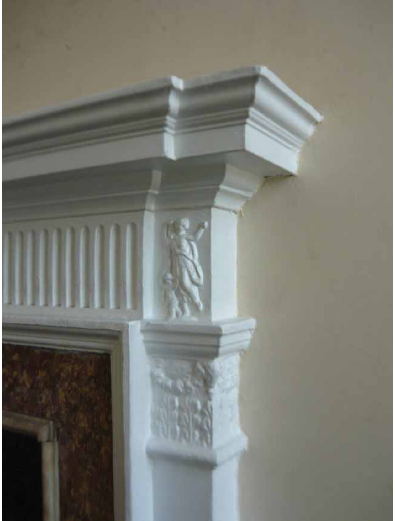
Plate 463: West end of fireplace in the south wall of Room F02, looking south-east (EAF10 BHD1 (85))
