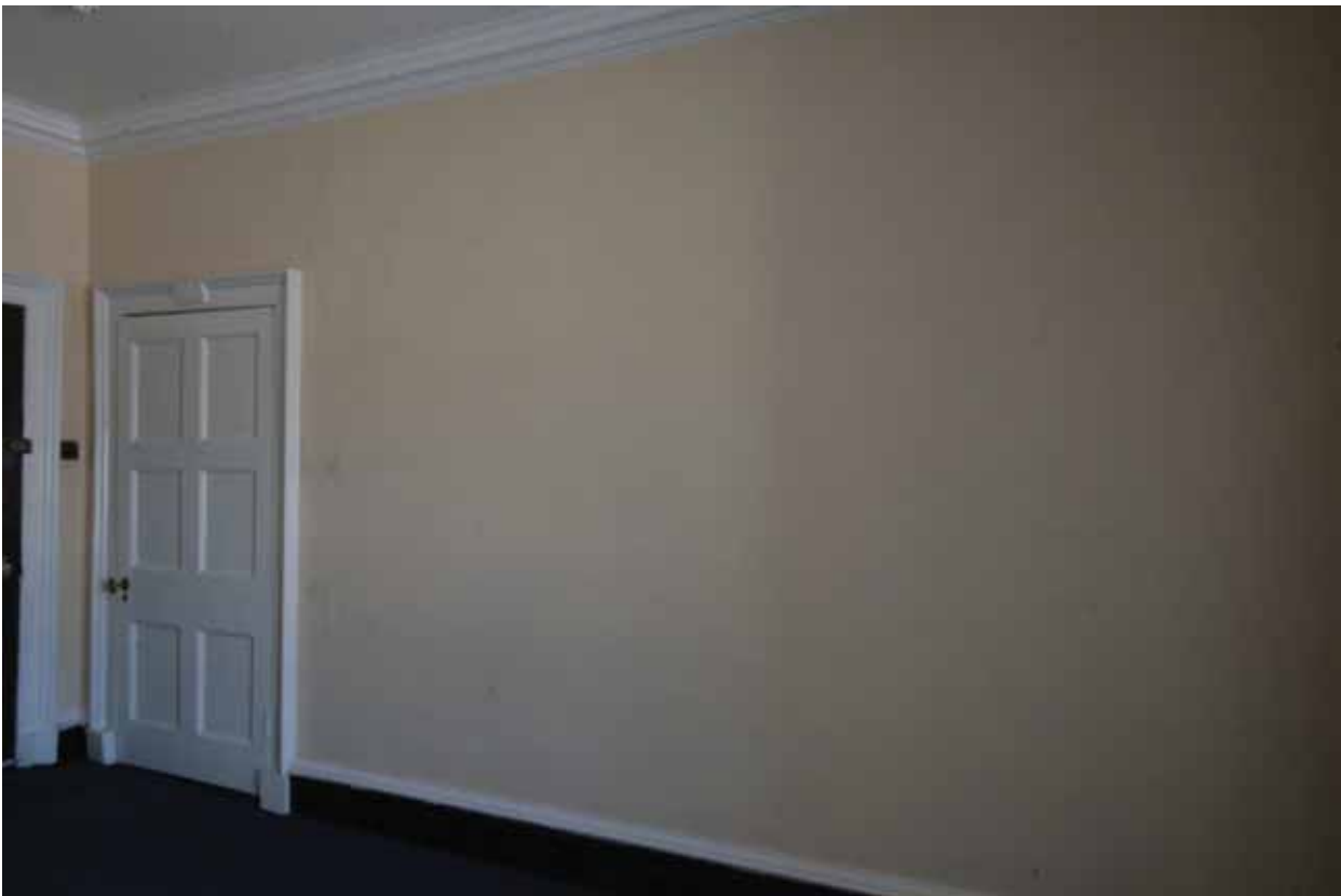
Plate 564: South partition wall in Room S02, looking south-east (EAF10 151)
