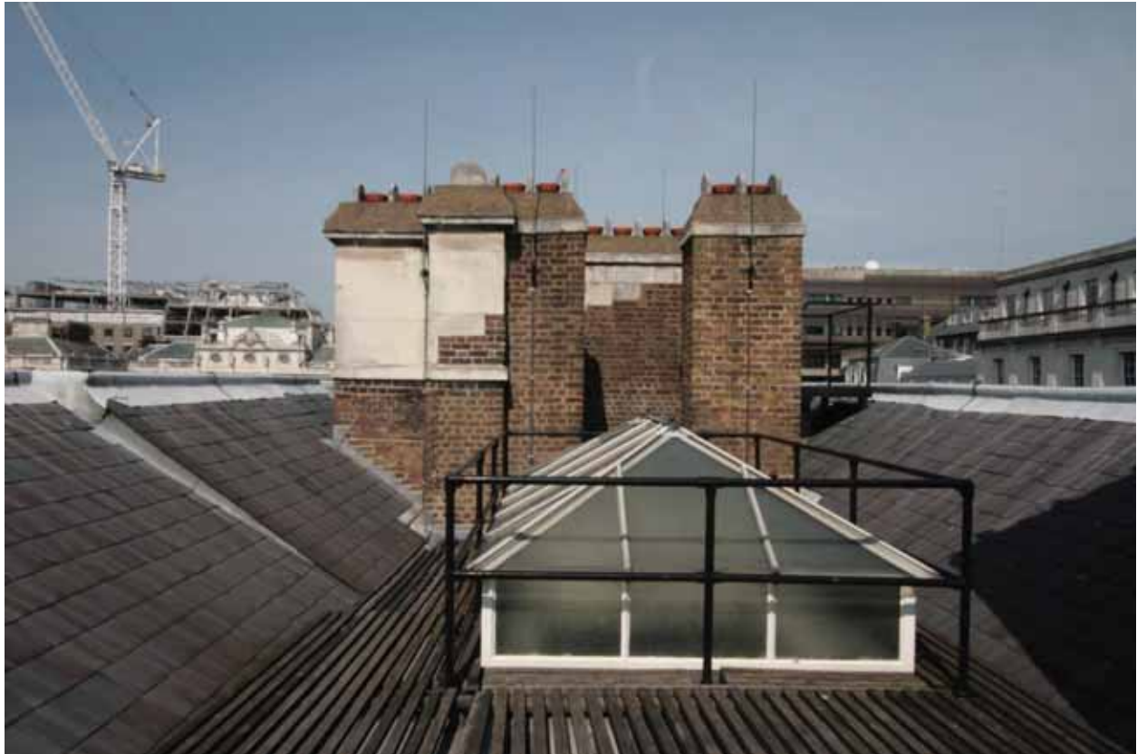
Plate 792: Lantern skylight over Corridor 09T, looking north (EAF10 29)
