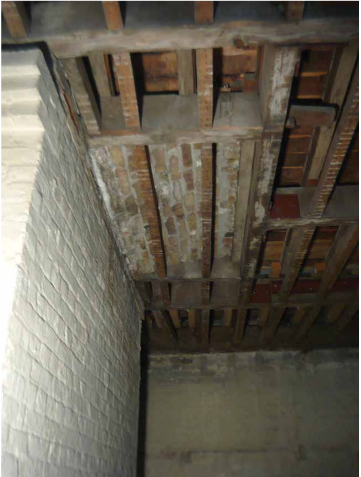
Plate 146: South wall in Room B52, looking west (EAF10 BHD5 (168))
