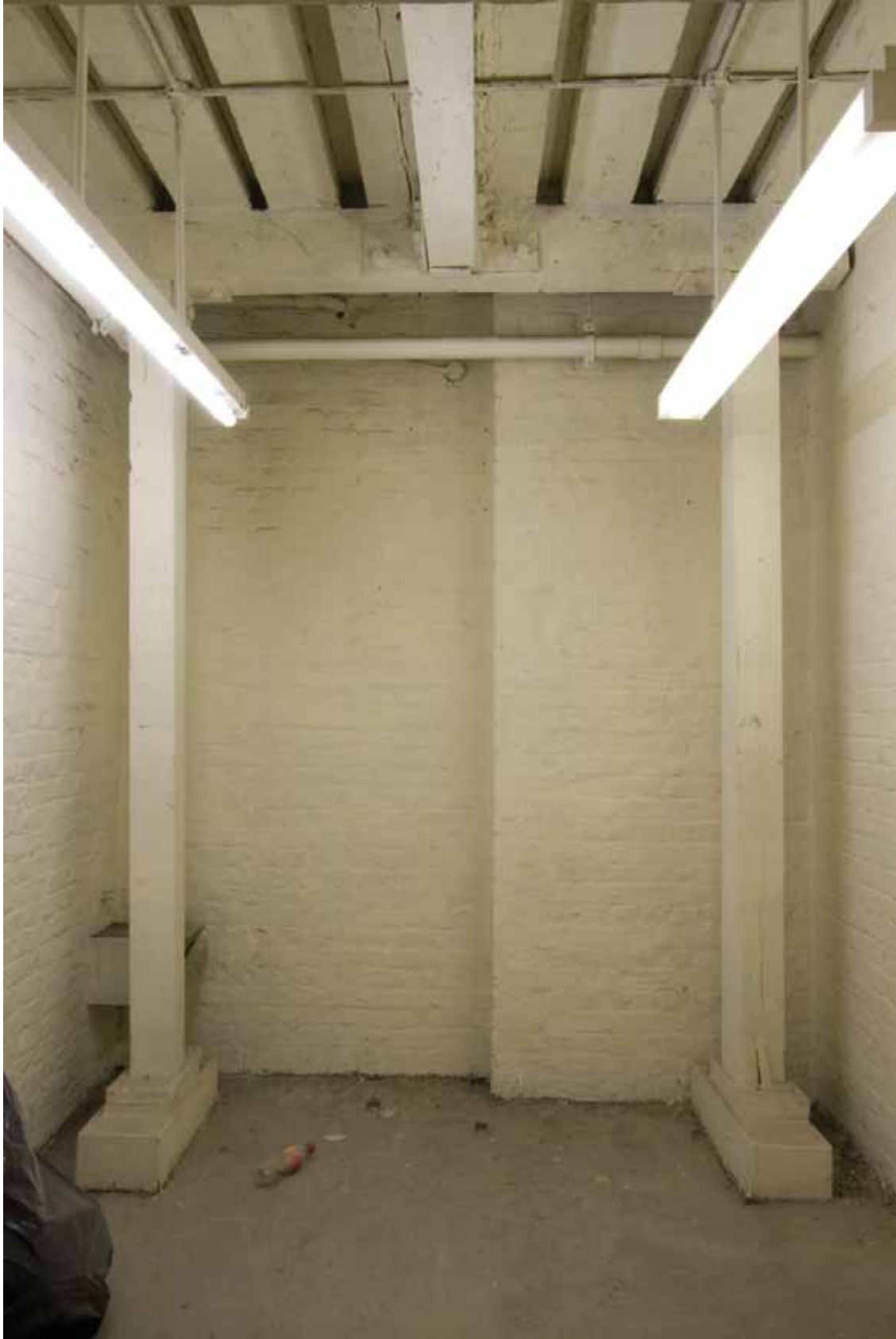
Plate 34: South wall of Rooms B47B, looking south (EAF10 D100 031a)
