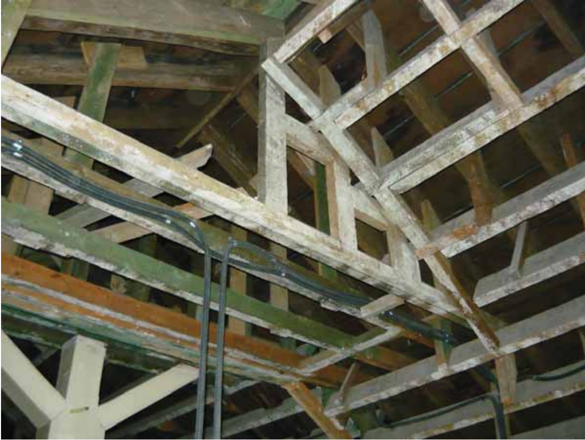
Plate 657: Roof structure above Room T120, looking south-west (EAF10 BHD10 (50))
