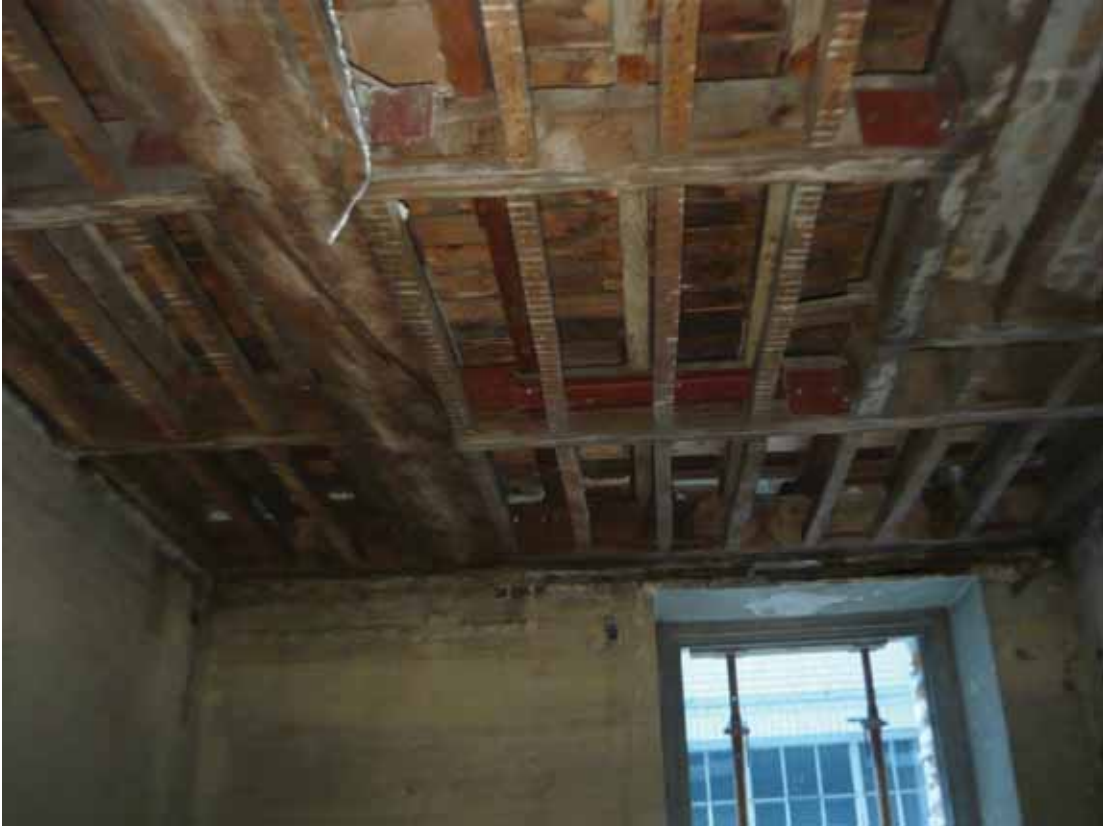
Plate 144: Ceiling in Room B52, looking east (EAF10 BHD5 (170))
