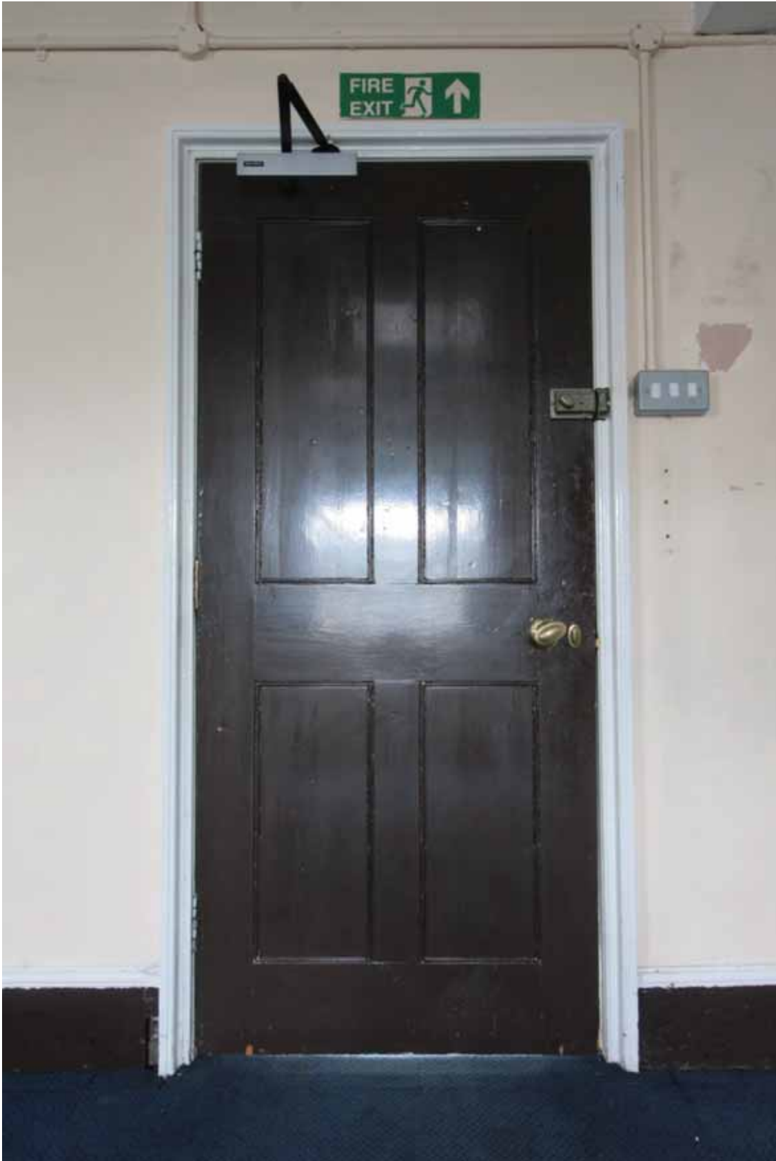
Plate 649: Doorway in the east wall of Room T120, looking east (EAF10 52)
