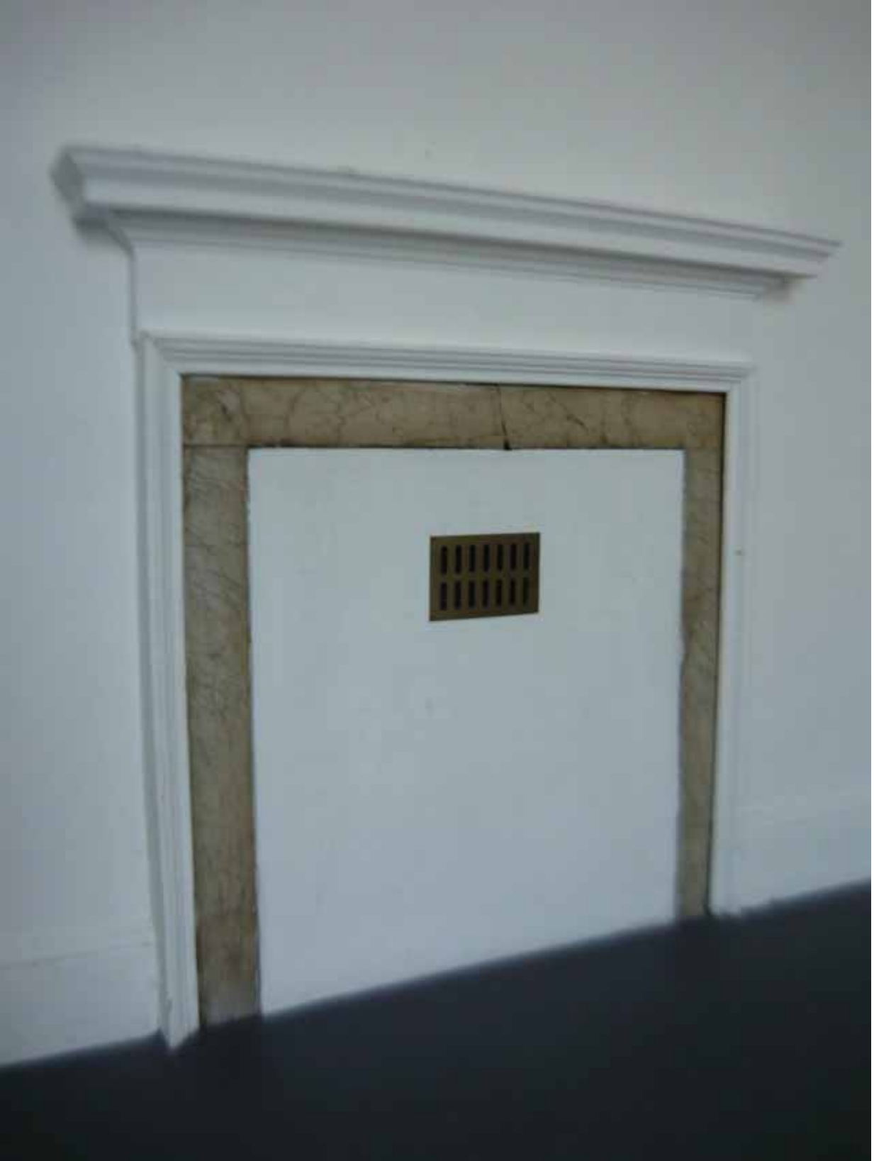
Plate 337: Fireplace (type 2) in the east wall in Room G42, looking south-east (EAF10 BHD1 (60))
