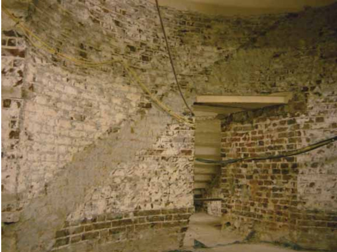
Plate 103: South wall of Corridor 6, looking south-east (EAF10 BHD13 (19))
