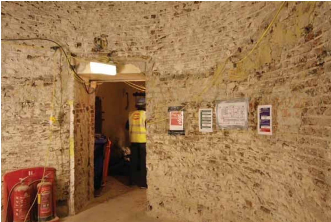
Plate 90: South wall of Corridor 2, looking south-east (EAF10 A100 044)
