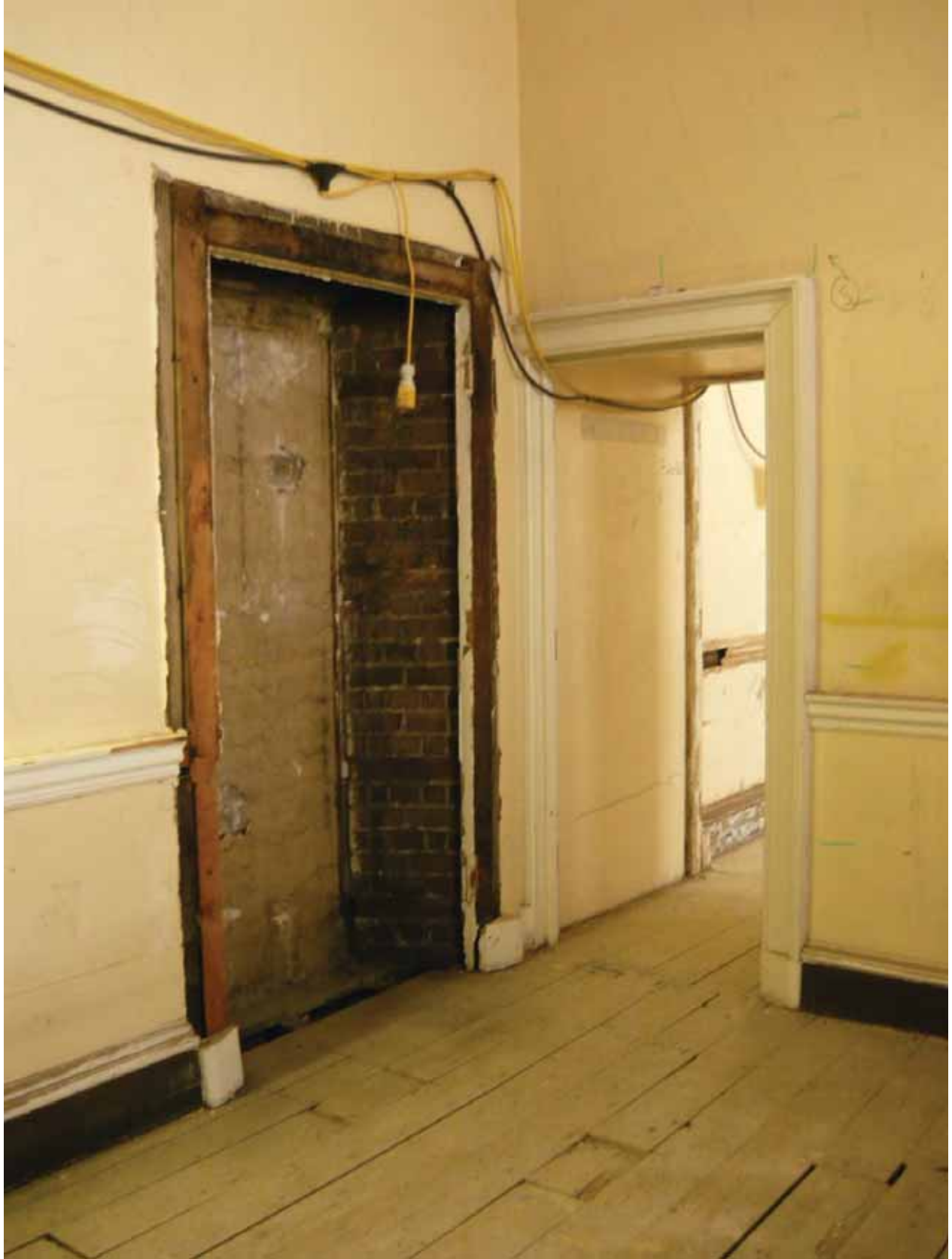
Plate 472: South-east corner of Room F03, looking south-east (EAF10 BHD8 (22))
