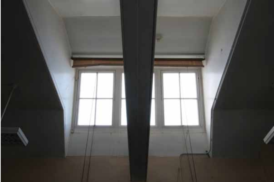
Plate 663: Inserted dormer window above the east wall of Room T01, looking east (EAF10 170)
