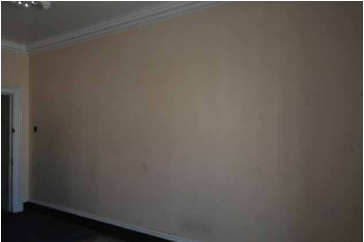
Plate 570: South partition wall in Room S09, looking south-east (EAF10 0113)
