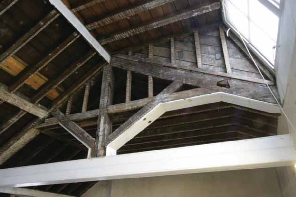
Plate 773: Southern truss in Room T24, looking south (EAF10 A100 005)
