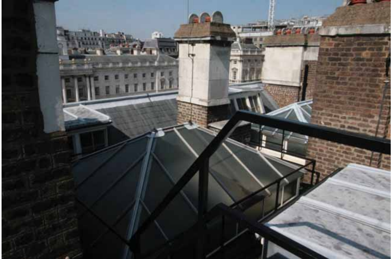
Plate 795: Lantern skylight over Corridor 08T, looking north-west (EAF10 26)
