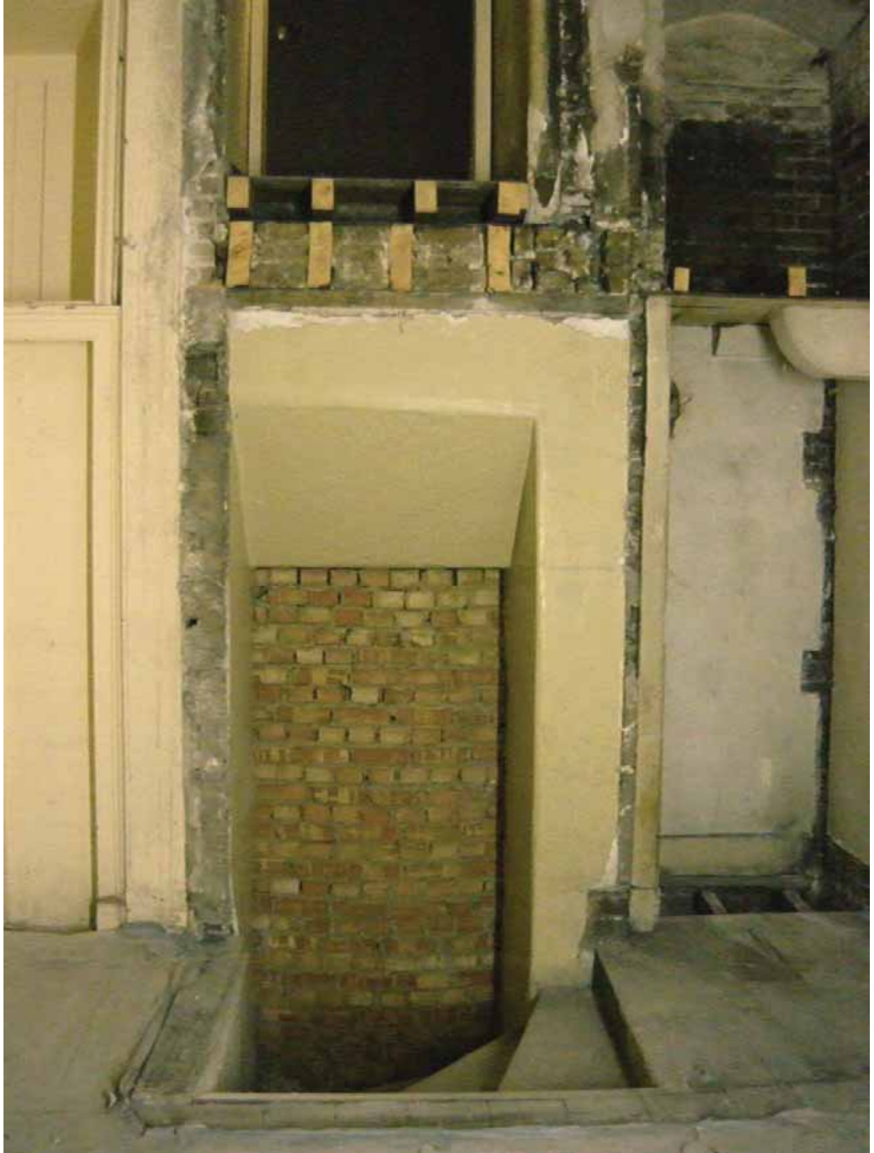
Plate 224: South wall of Room M18, looking south (EAF10 BHD6 (43))
