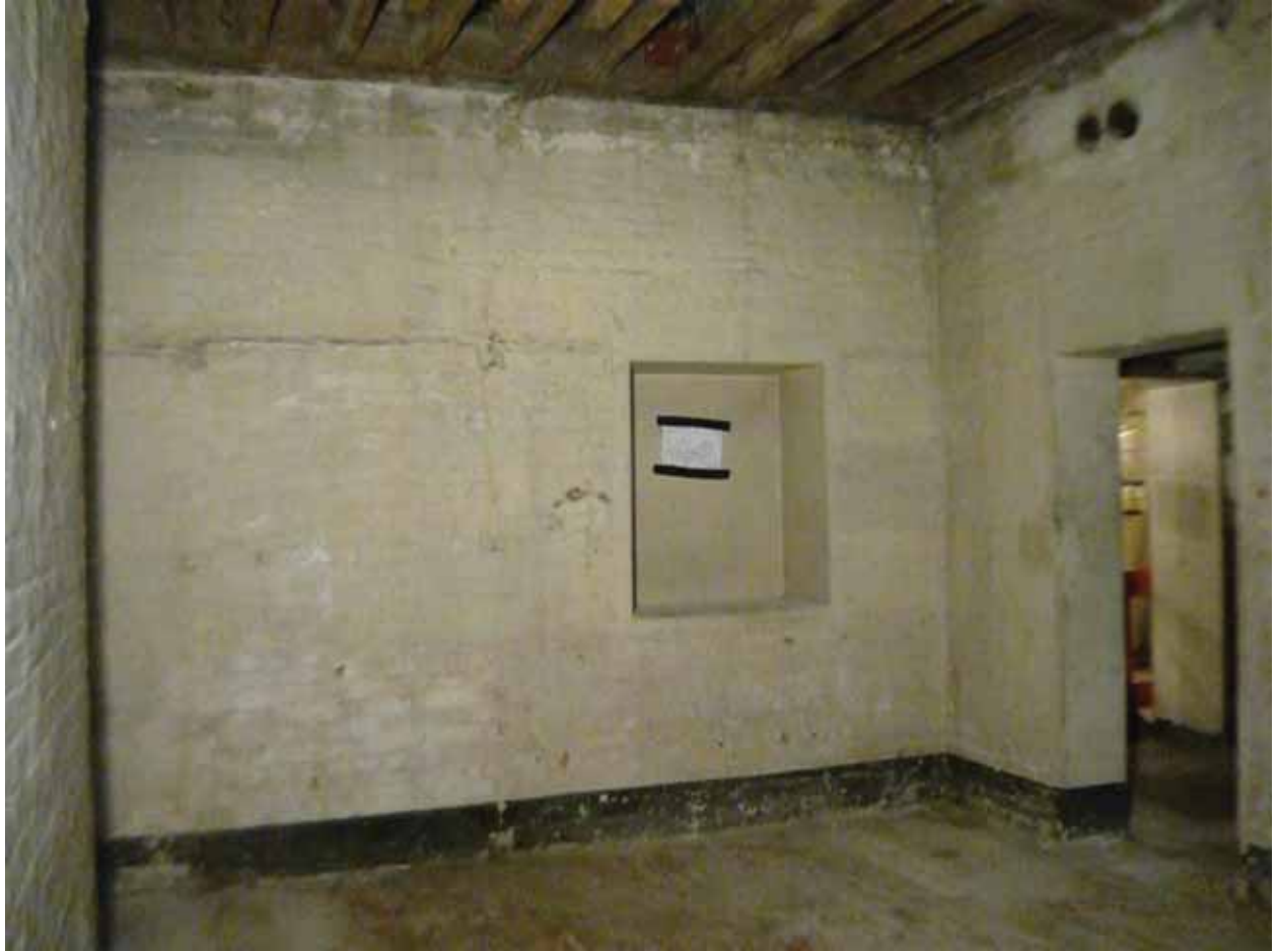
Plate 138: West wall of Room B52, looking west (EAF10 BHD5 (165))
