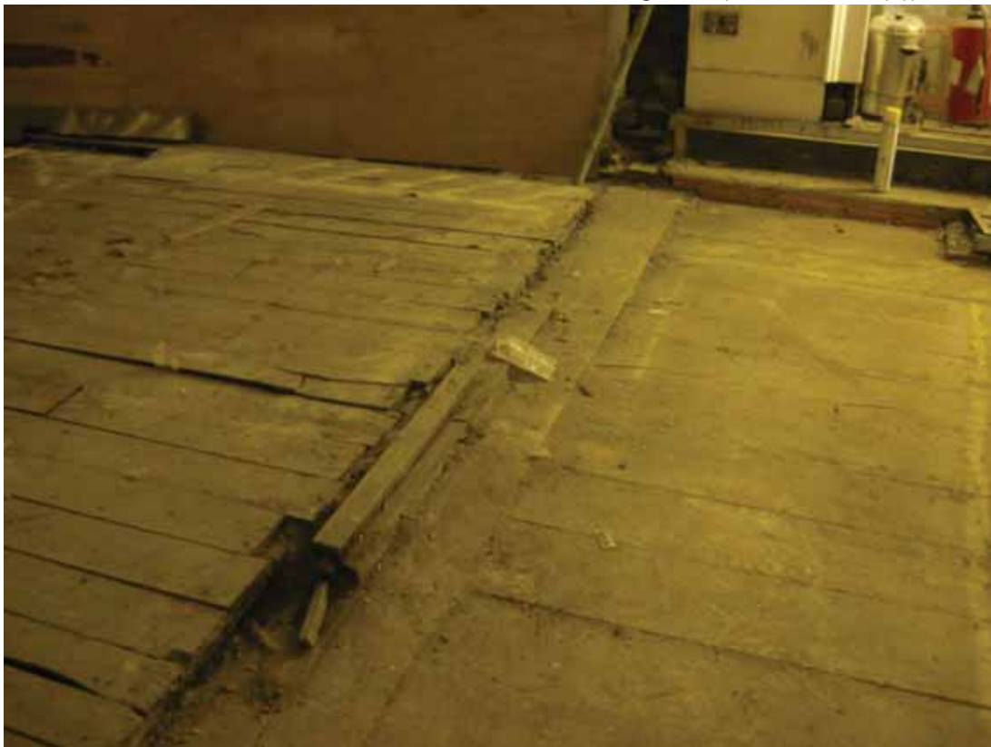
Plate 434: Raised floor in Room G24 (left), looking -east (EAF10 BHD8 (116))
