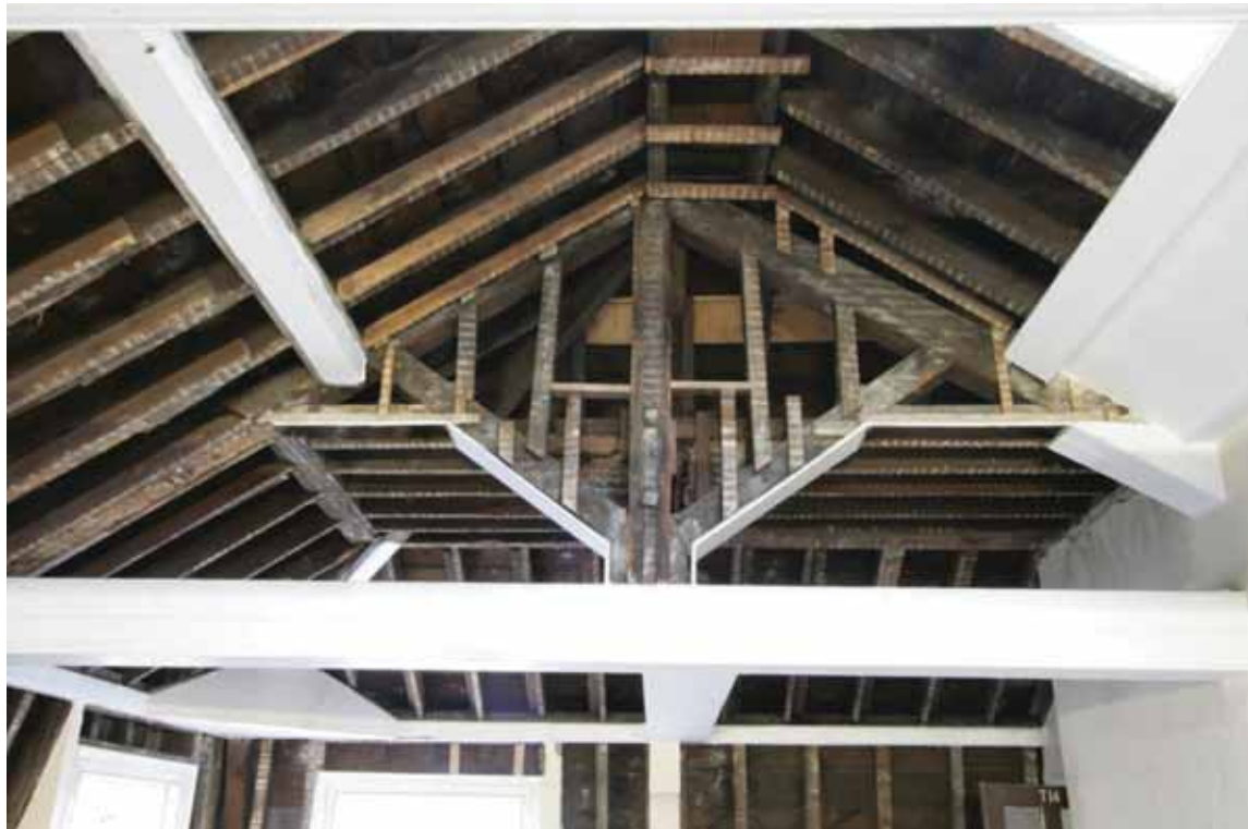
Plate 697: Northernmost truss in Room T09, looking north (EAF10 A100 004)
