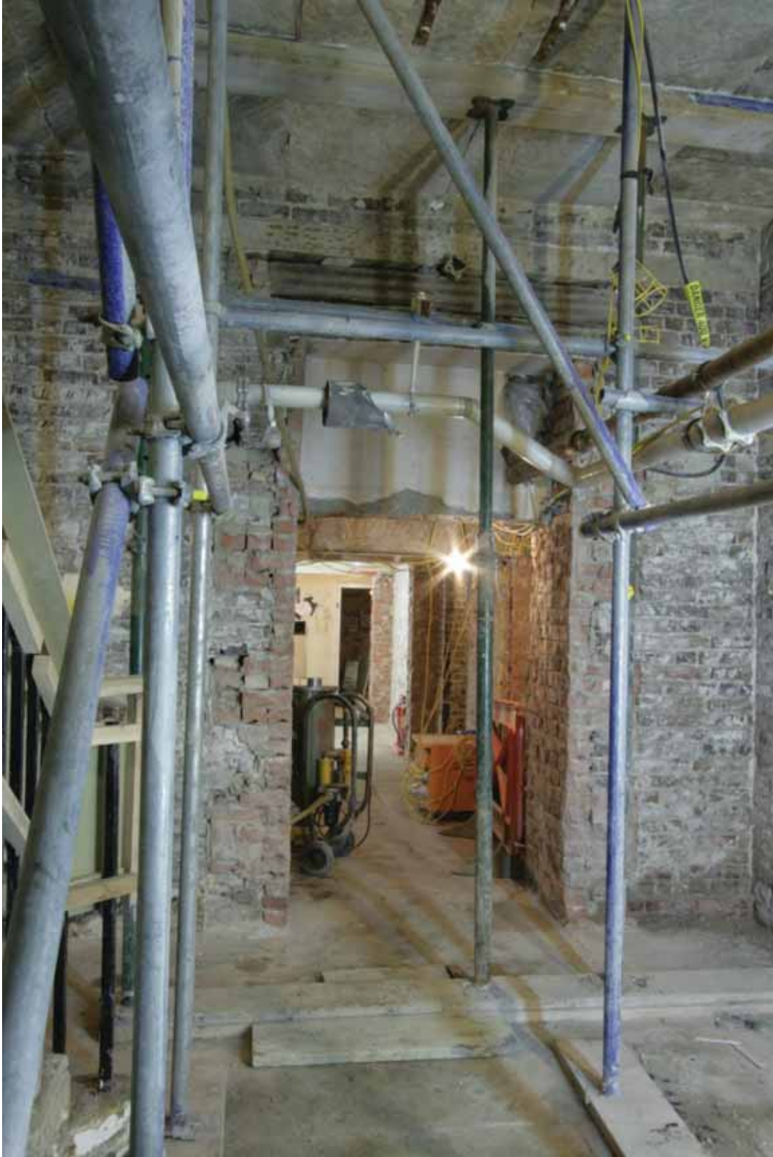
Plate 74: South doorway in Stairs 01, looking south (EAF10 A100 040)
