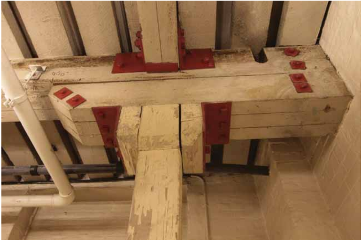
Plate 55: North-west corner of Room B48A, looking west (EAF10 D100 034a)
