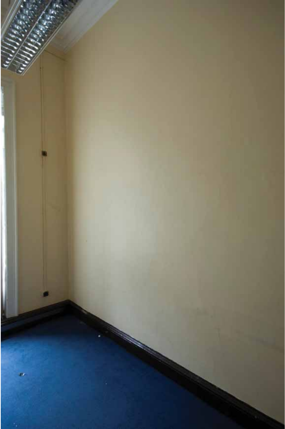
Plate 272: South (partition) wall in Room M32, looking south-east (EAF10 LG100 1087)
