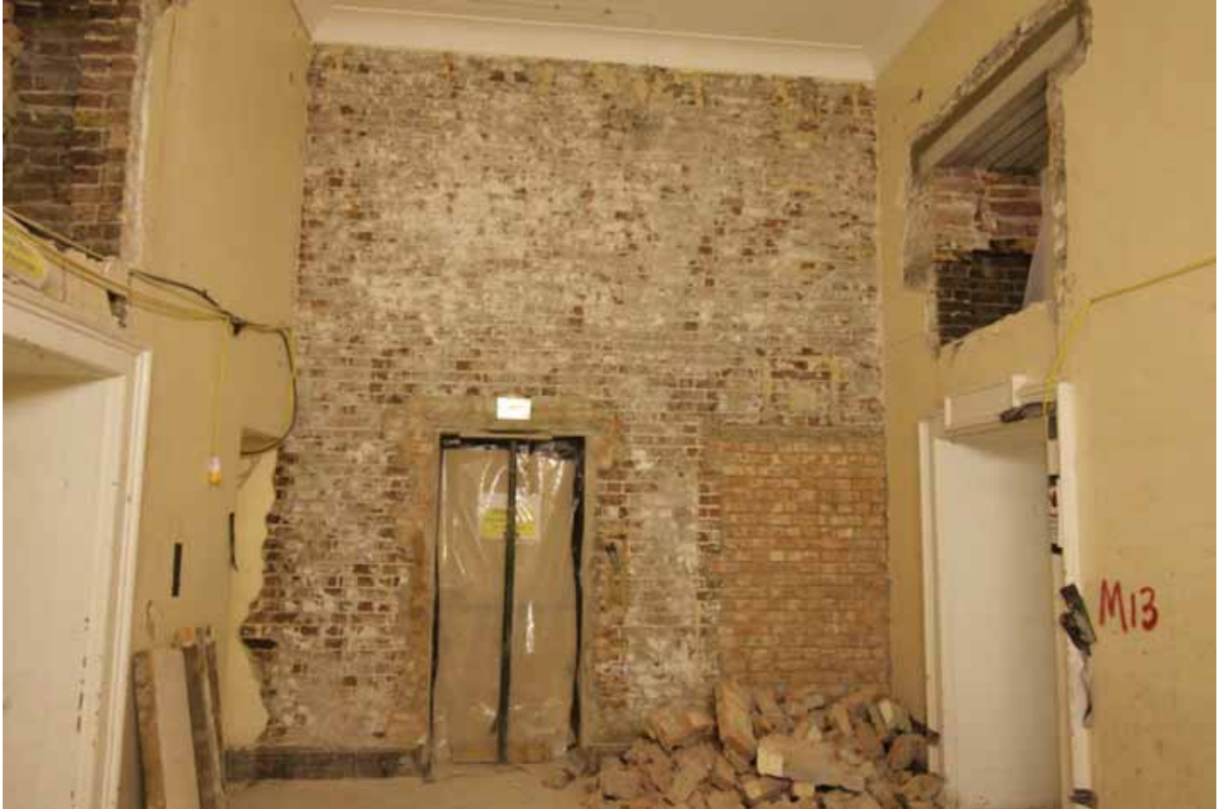
Plate 229: Plaster removed from the south wall of Corridor 03LG, looking south (EAF10 A100 028)
