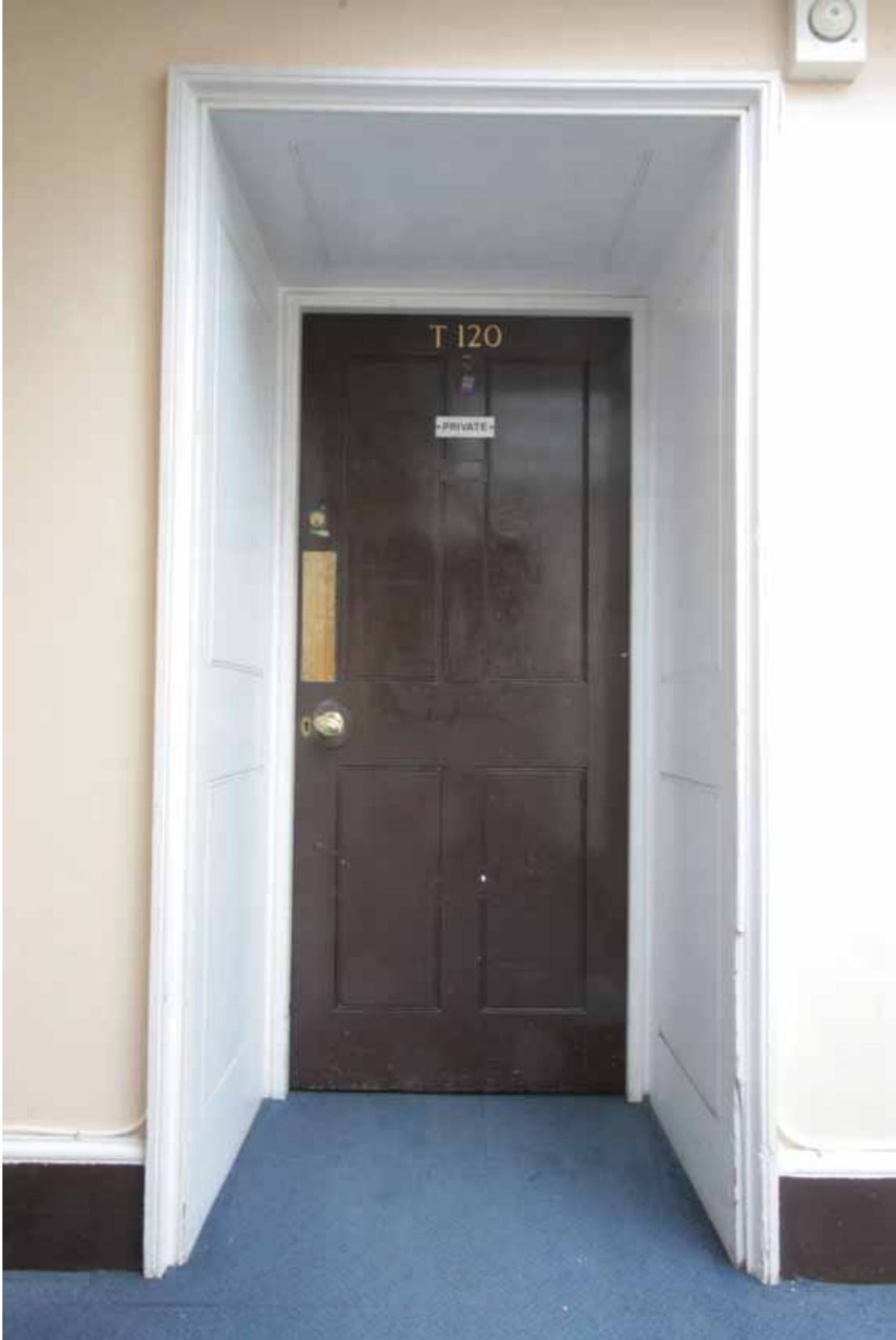
Plate 722: Doorway in the west wall of Corridor 09T, looking west (EAF10 51)
