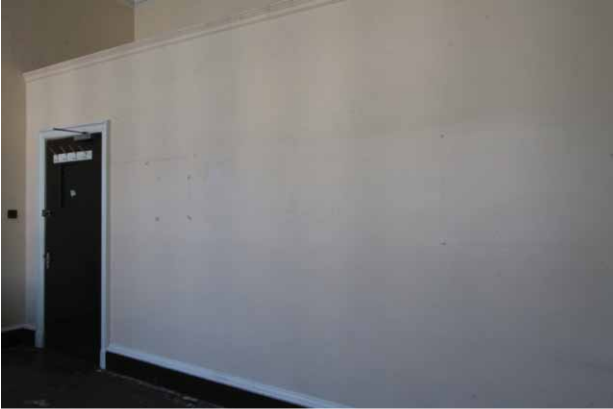
Plate 548: West partition wall in Room F28, looking south-west (EAF10 152)
