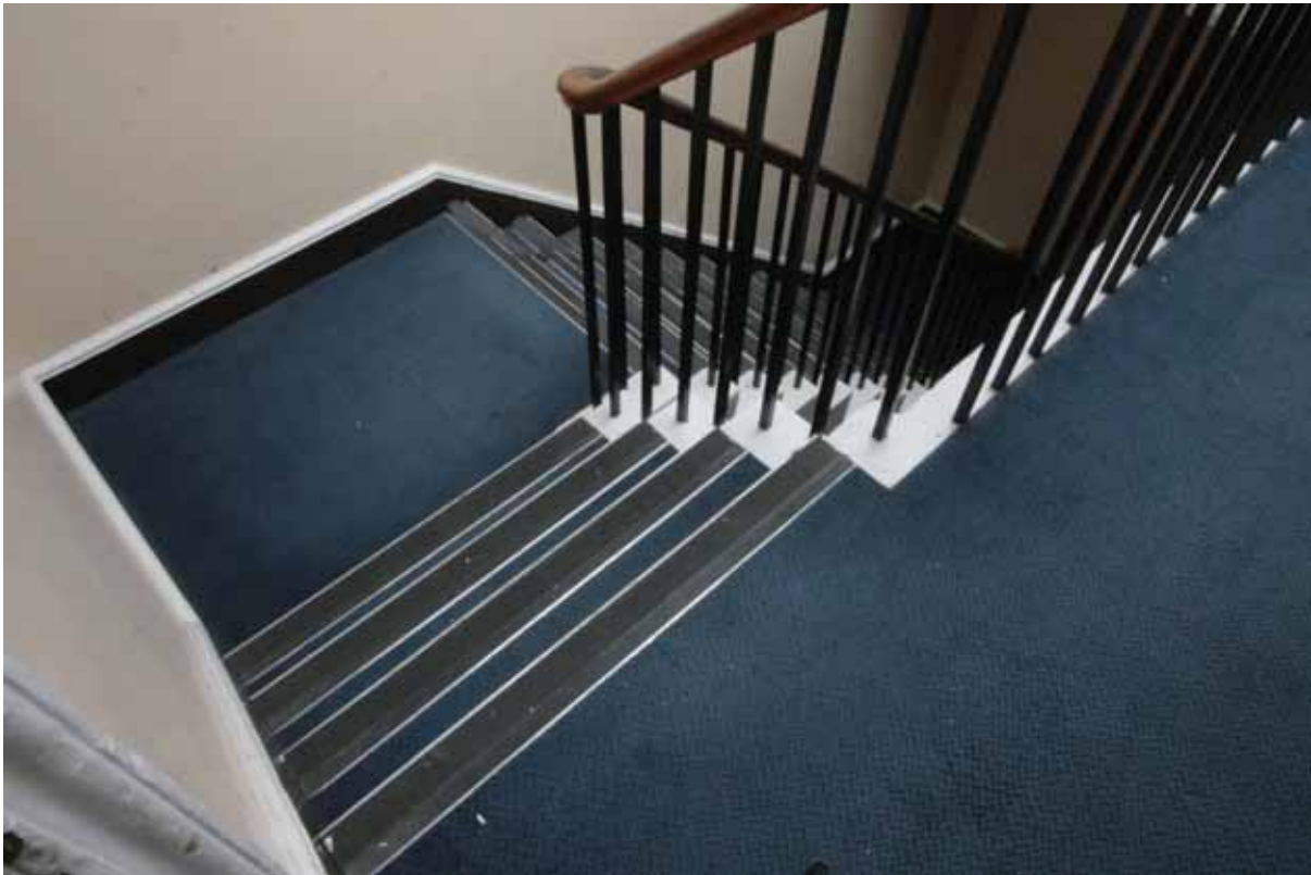
Plate 721: Staircase leading down west then north in Corridor 07T, looking north-west (EAF10 48)
