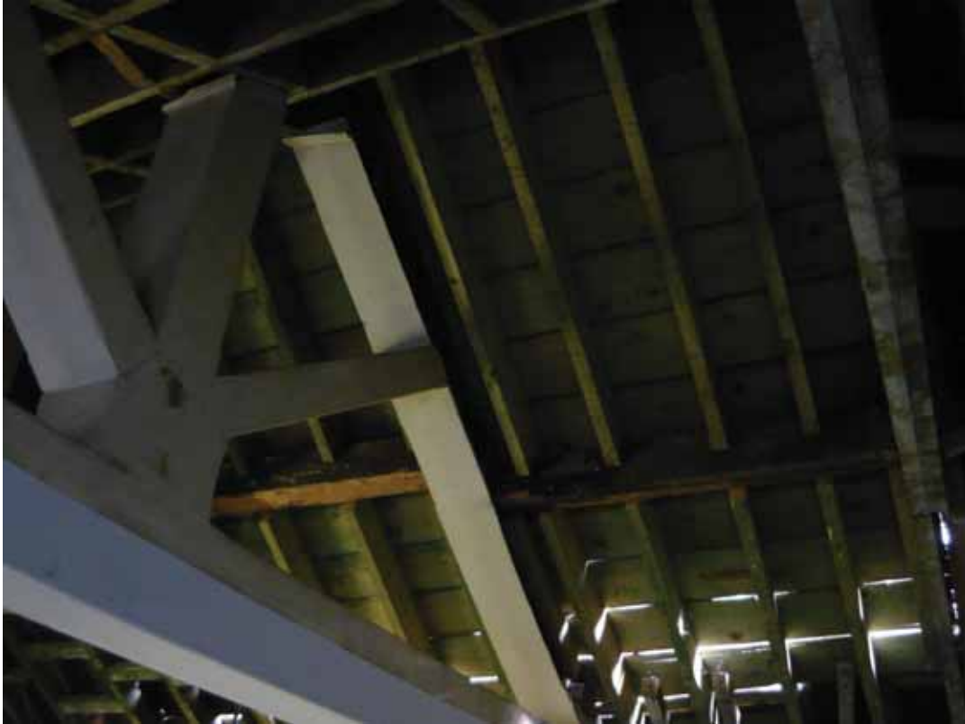
Plate 653: Roof structure above Room T120, looking north-east (EAF10 BHD10 (45))
