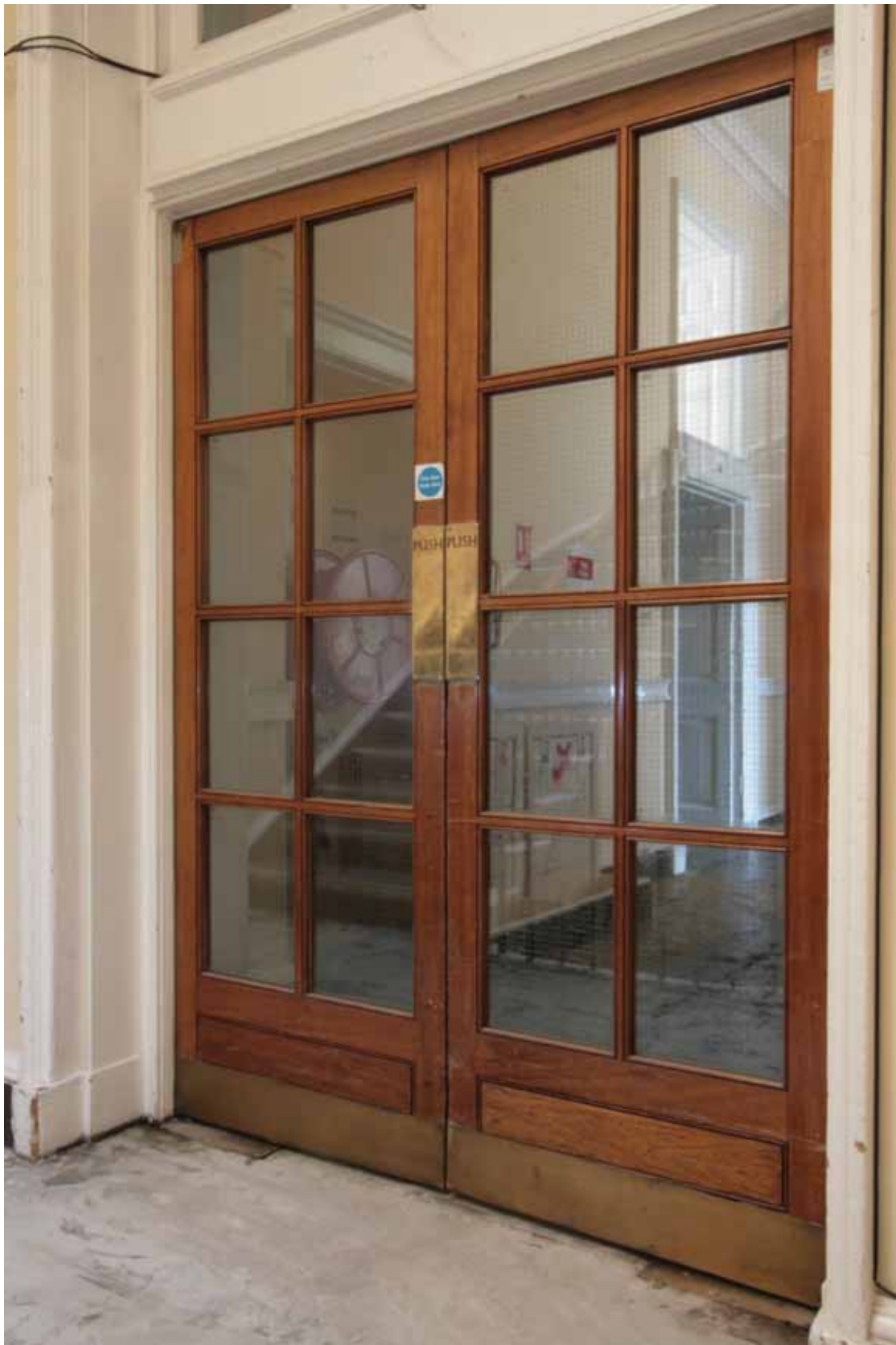
Plate 494: Doorway in the south wall of Stairs 01F, looking south-east (EAF10 156)
