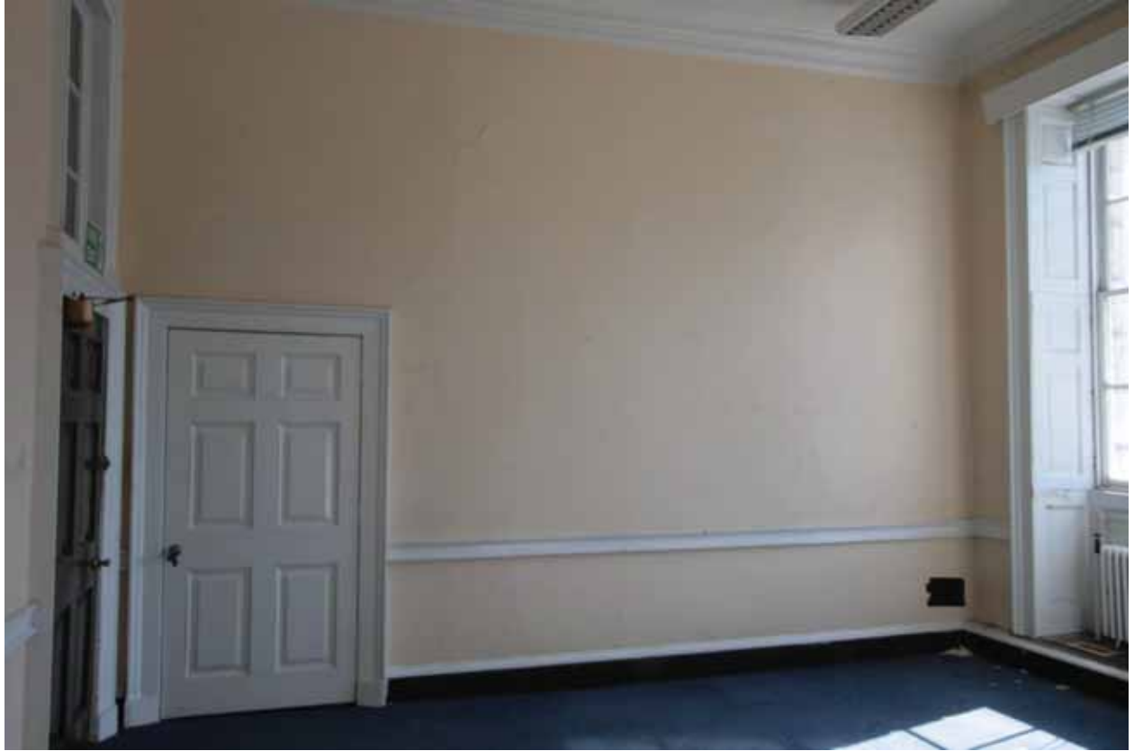
Plate 481: South partition wall in Room F08, looking south (EAF10 158)
