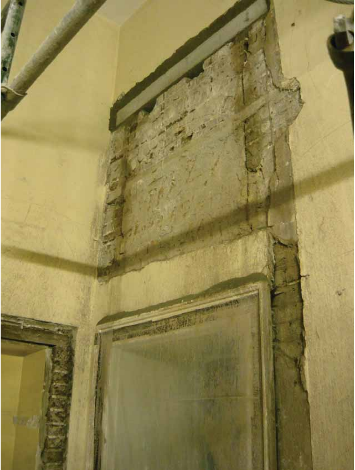
Plate 305: Infilled fanlight above the west doorway in Room M26/M27, looking south-west (EAF10 BHD6 (85))
