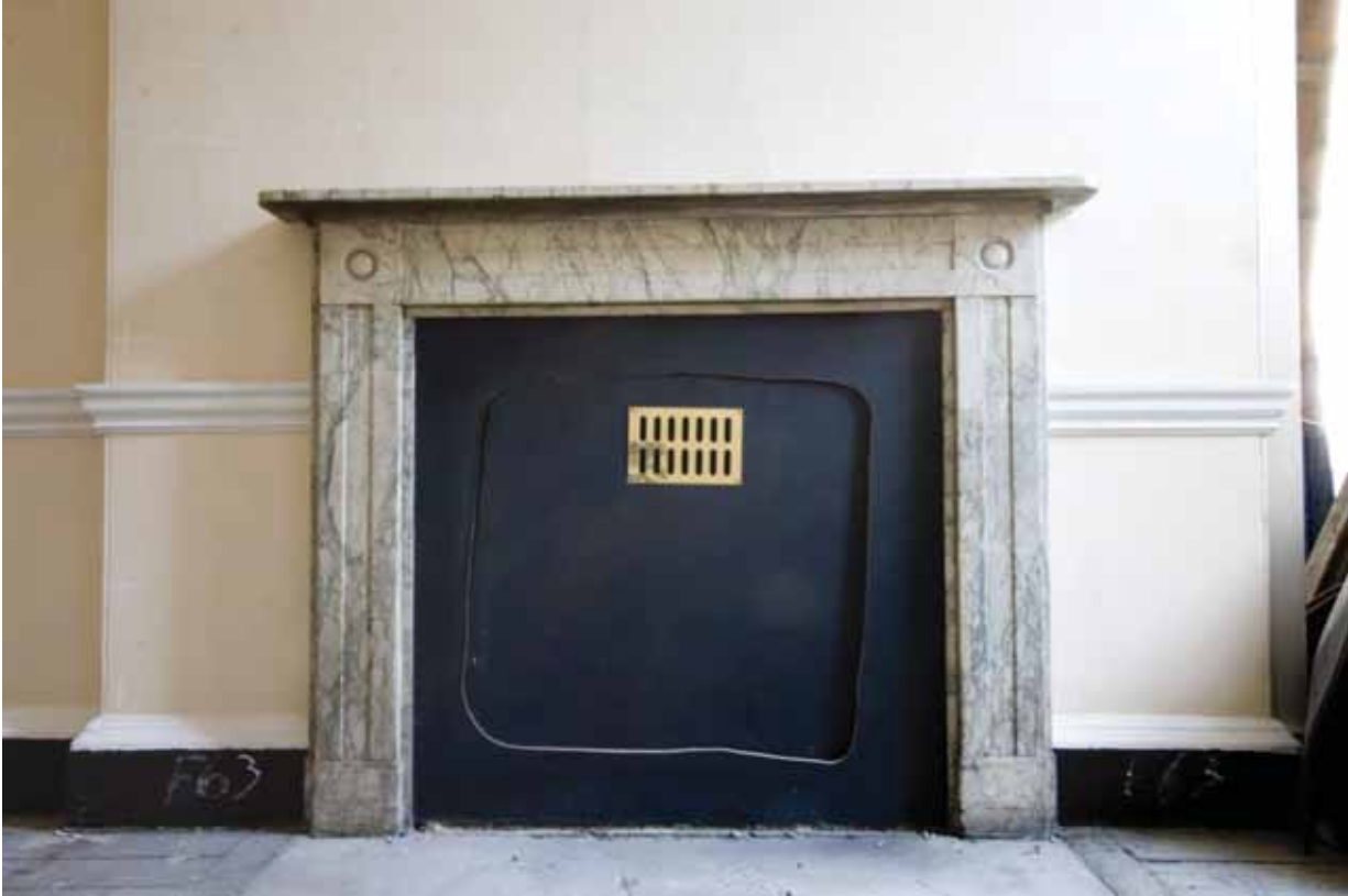
Plate 514: Fireplace (type 16) in the north wall of Room F63, looking north (EAF10 165a)
