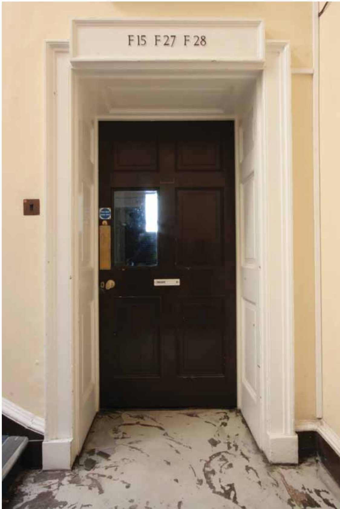
Plate 493: Doorway in the east wall of Stairs 01F, looking east (EAF10 149)
