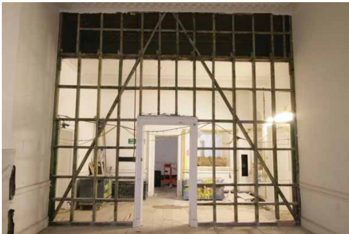
Plate 408: Studwork partition in Room G16, looking west (EAF10 A100 023a)
