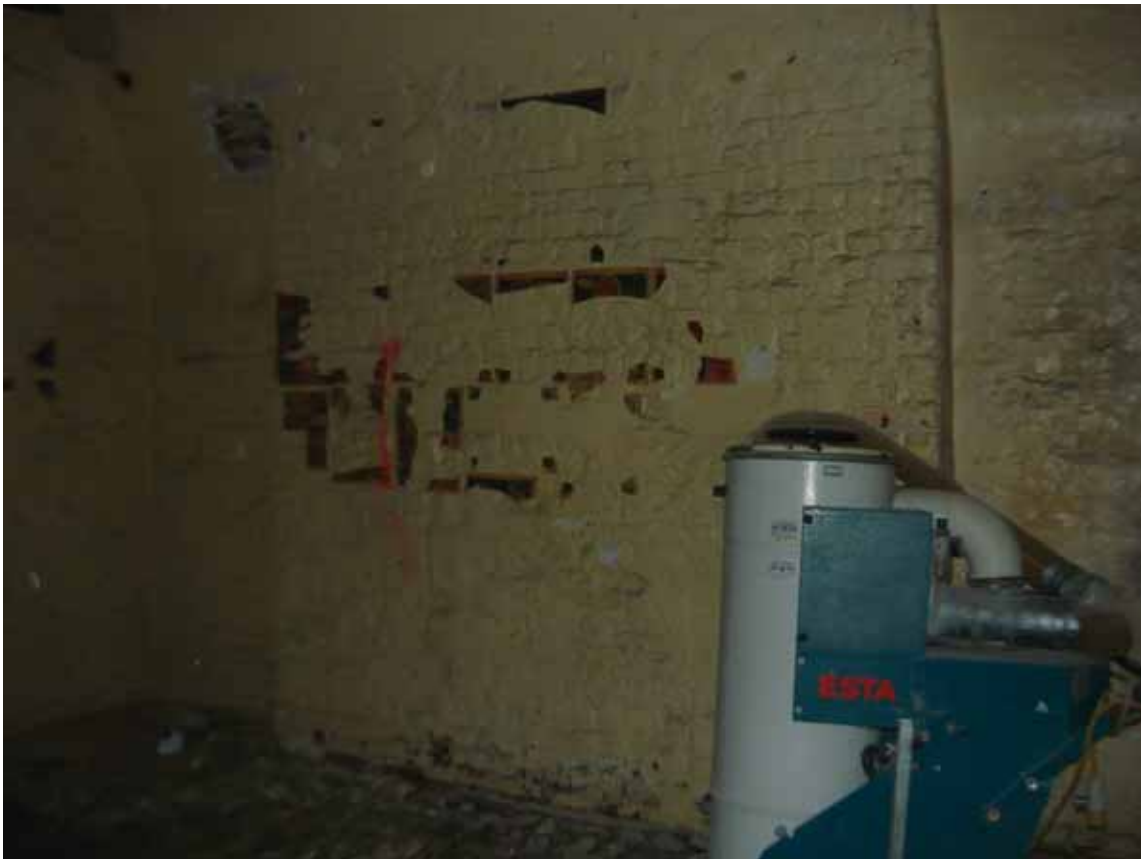
Plate 7: North wall of Room B42, looking north-west (EAF10 BHD5 (206))
