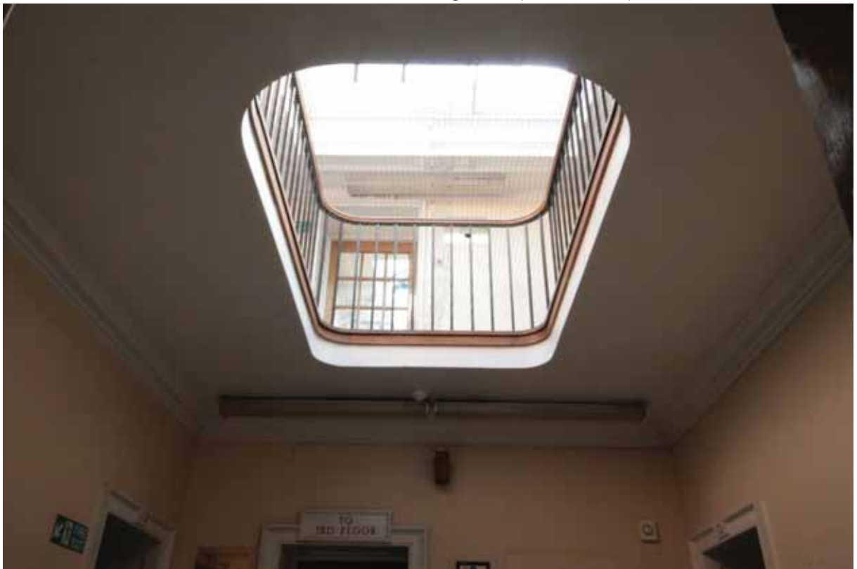
Plate 602: Ceiling in Stairs 02S looking south (EAF10 0130)
