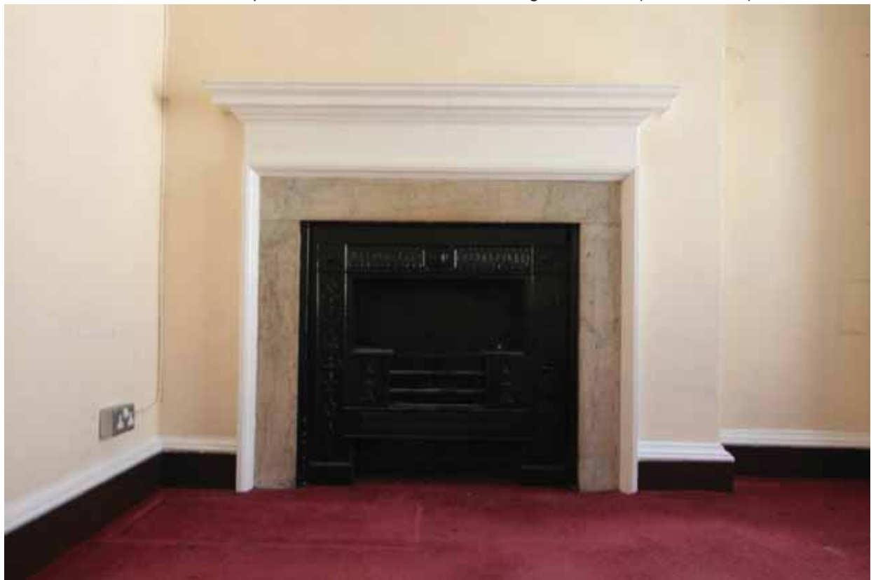
Plate 642: Fireplace (type 2) in the north wall of Room S27, looking north (EAF10 0108)
