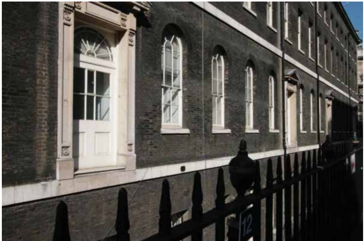
Plate 2: Ground floor level of the east (rear) elevation of Somerset House East Wing, viewed from the south-east
