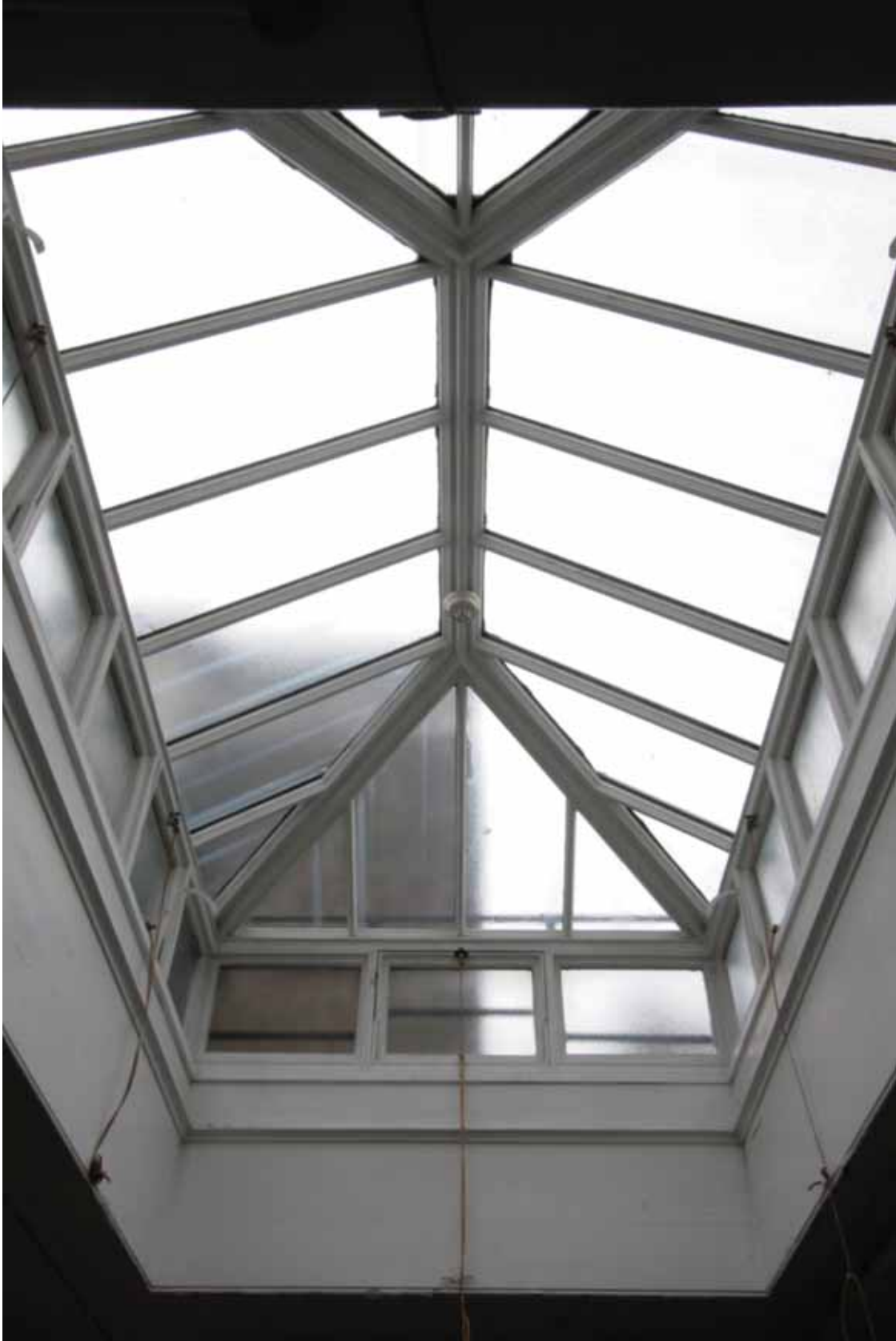
Plate 746: Skylight over the west end of Room T15, looking north (EAF10 50)
