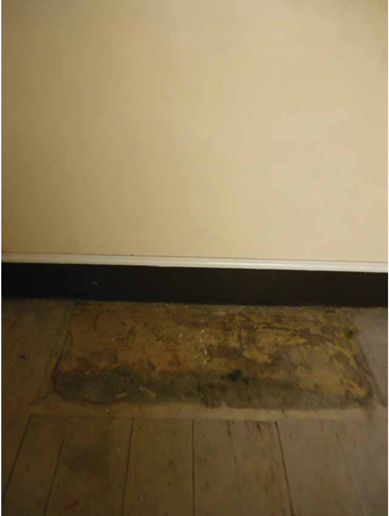
Plate 703: Stone hearth and infilled fireplace in the south wall of Room T14, looking south (EAF10 BHD2 (85))
