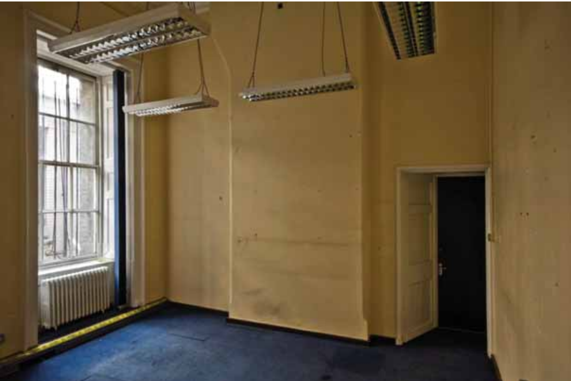
Plate 290: South wall in Room M24, looking south (EAF10 LG100 1012)
