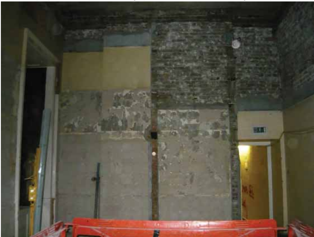
Plate 284: South wall of Room M116, looking south (EAF10 BHD8 (80))
