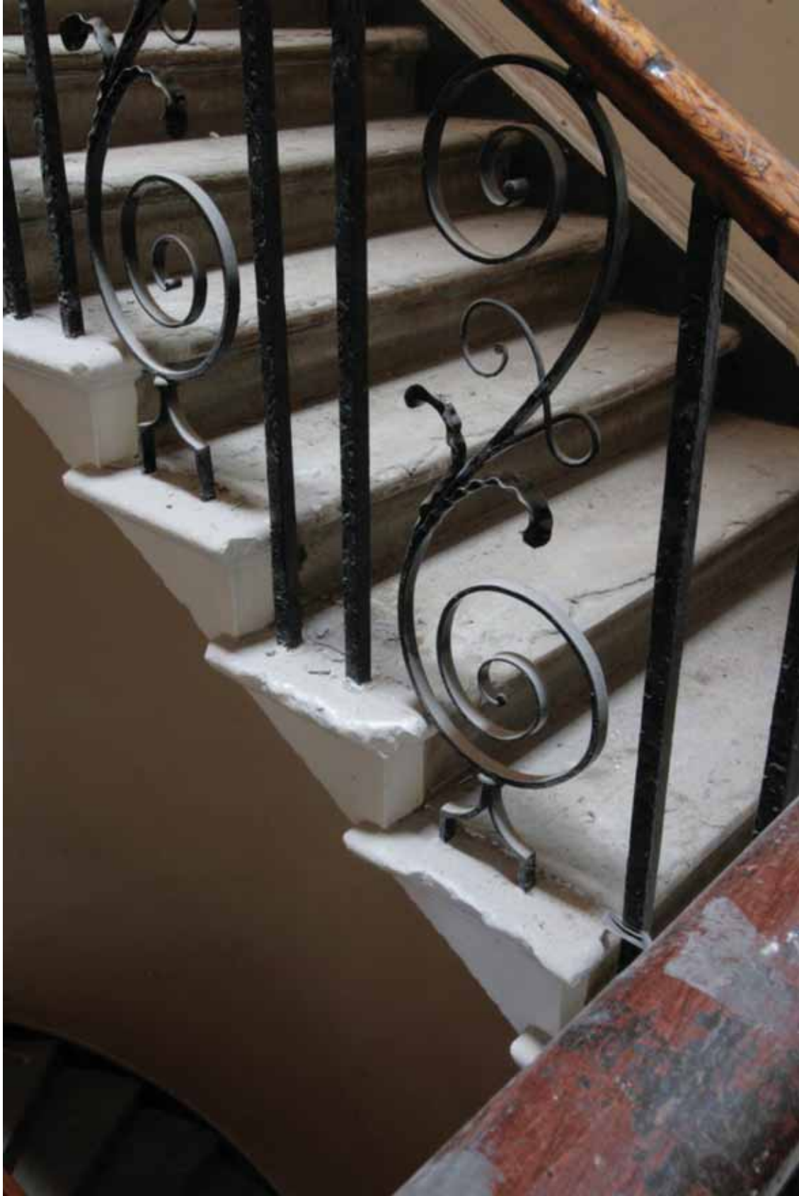
Plate 380: Stairs 01G, looking north (EAF10 263)
