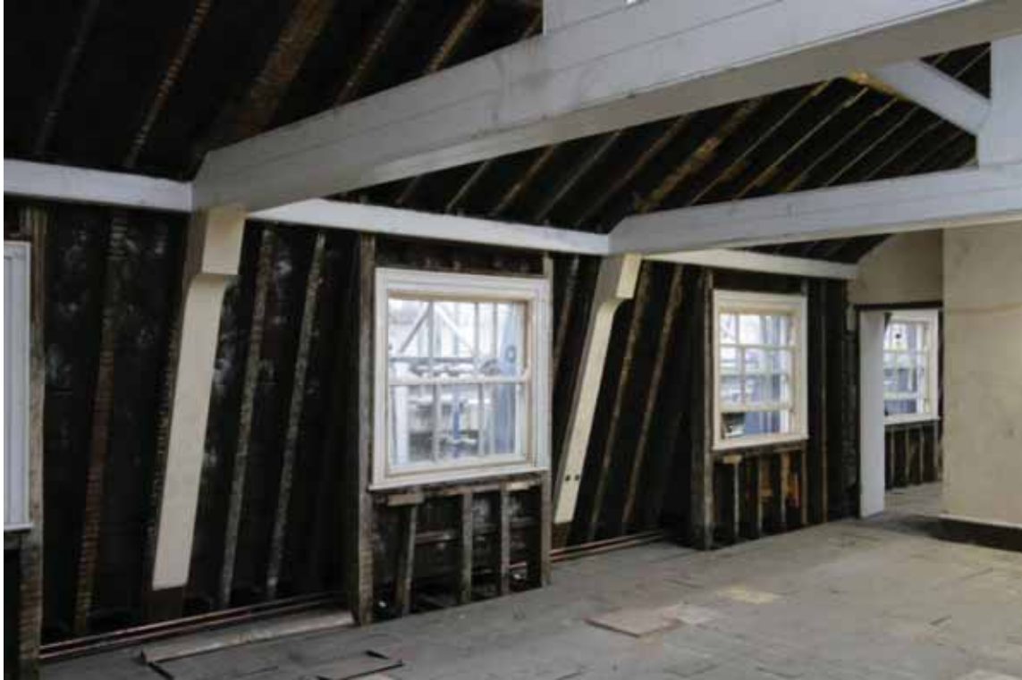
Plate 688: West wall of Room T08, looking north-west (EAF10 A100 014)
