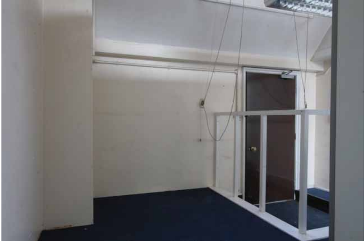
Plate 681: East wall of Room T05, looking east (EAF10 38)
