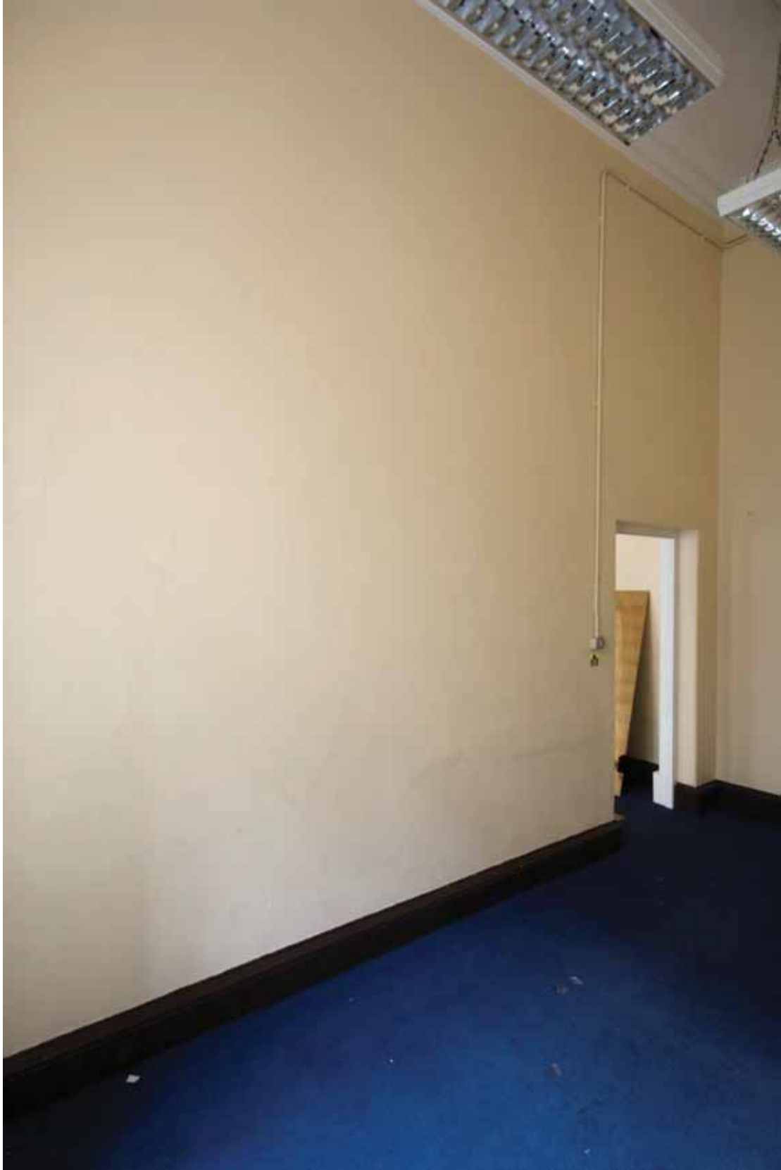
Plate 271: South (partition) wall in Room M32, looking south-west (EAF10 LG100 1086)
