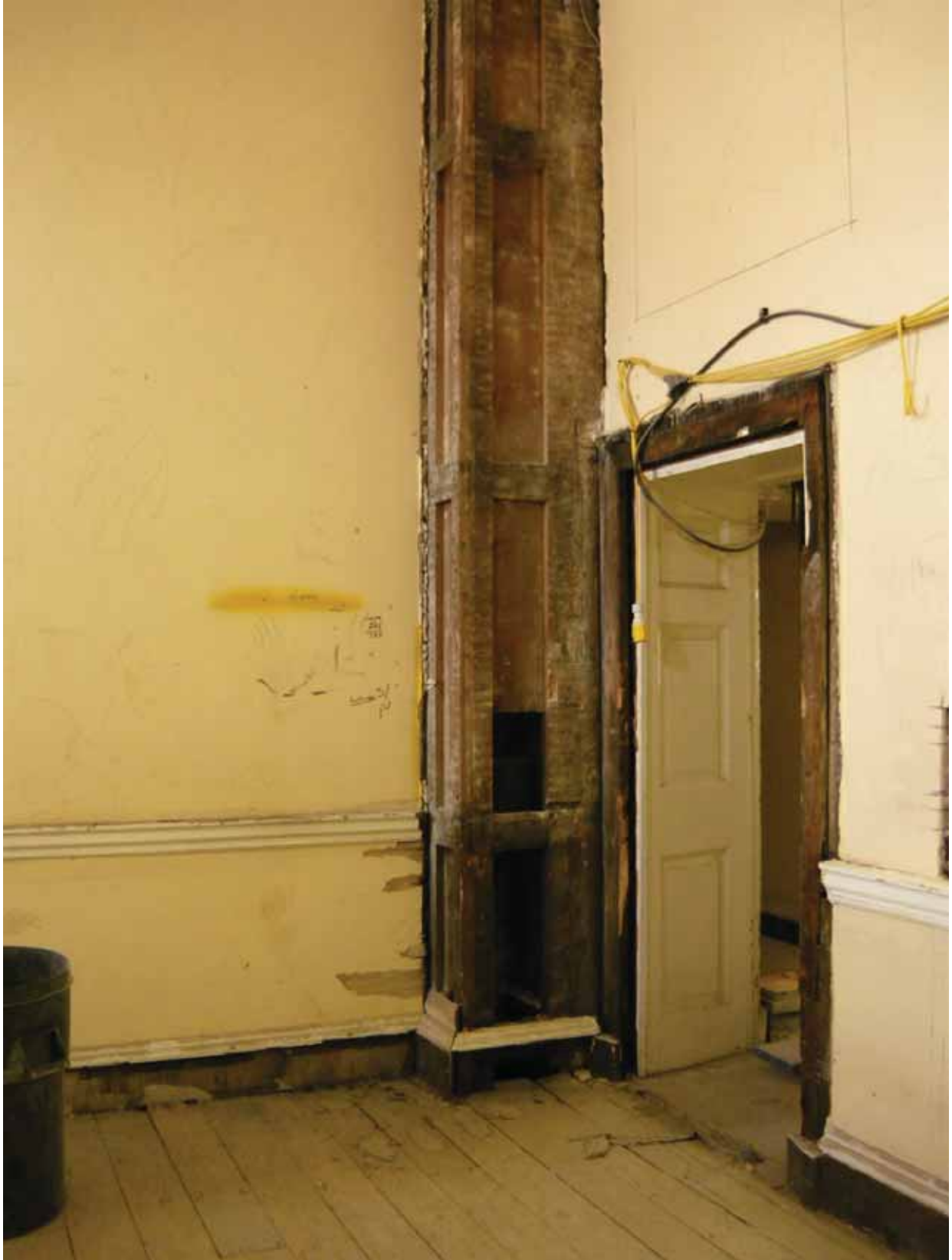
Plate 474: Boxed in weight for the clock in the north-east corner of Room F03, looking north (EAF10 BHD8 (17))
