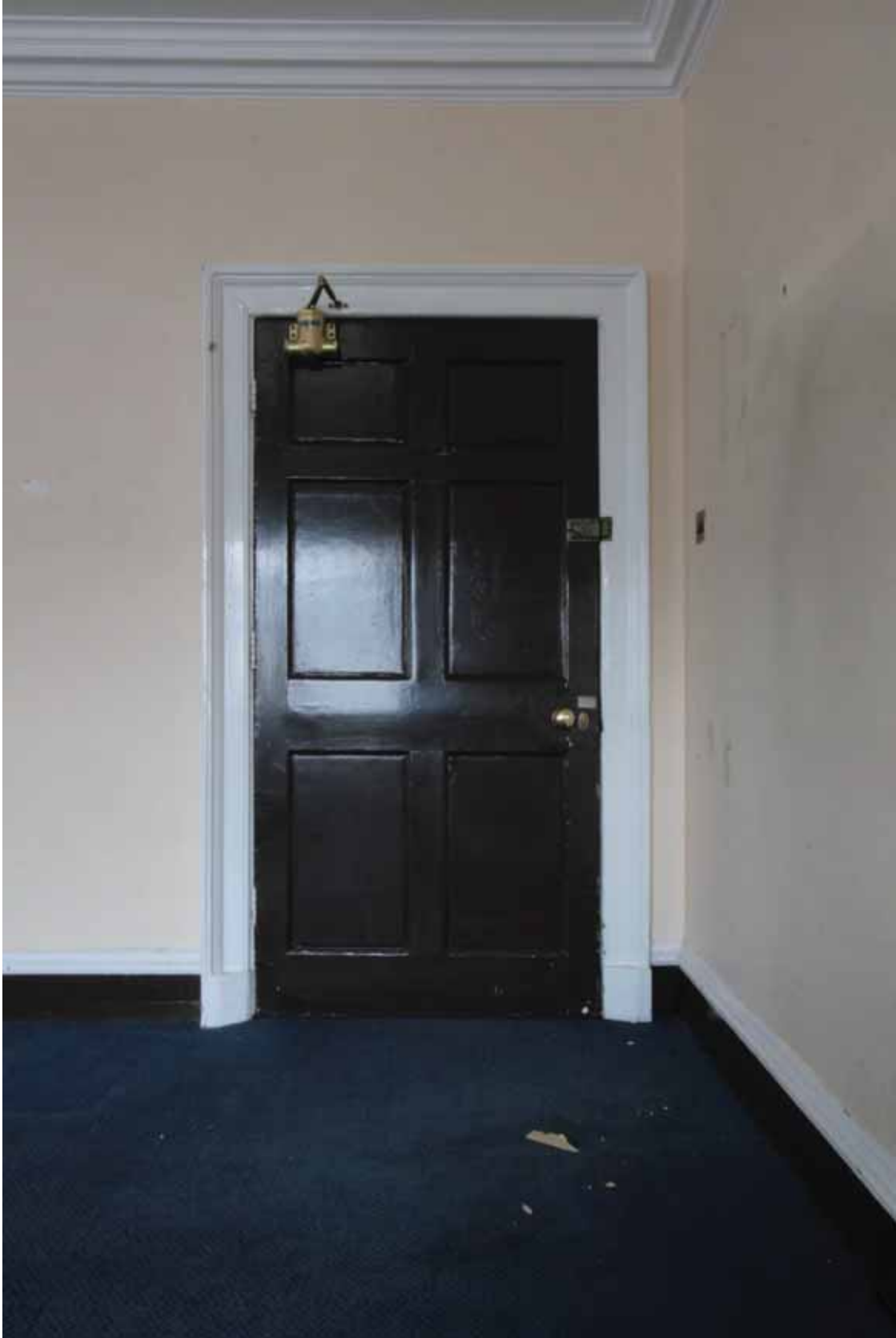
Plate 582: Doorway at the south end of the east wall in Room S10, looking east (EAF10 0096)
