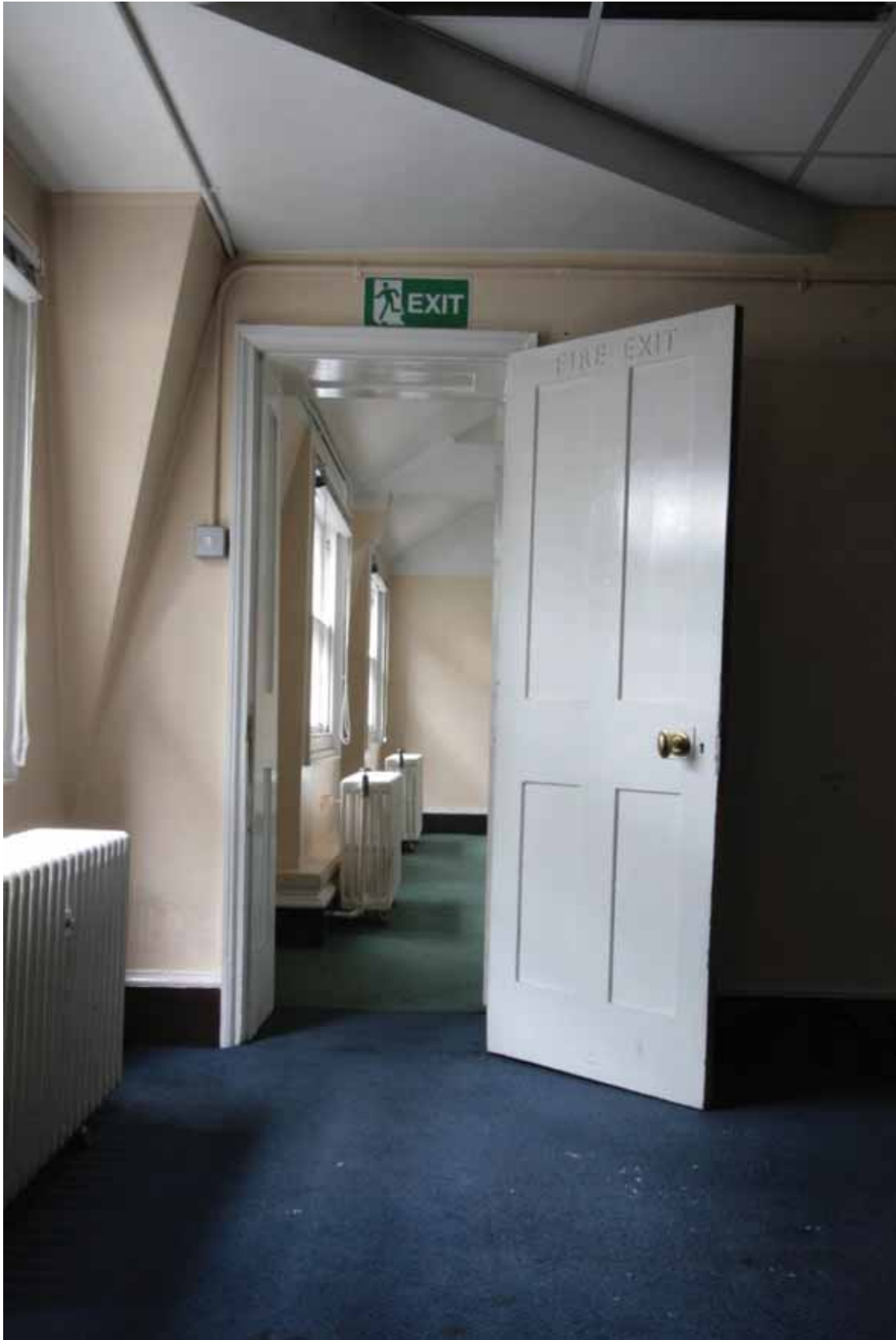
Plate 650: Doorway in the north wall of Room T120, looking north (EAF10 54)
