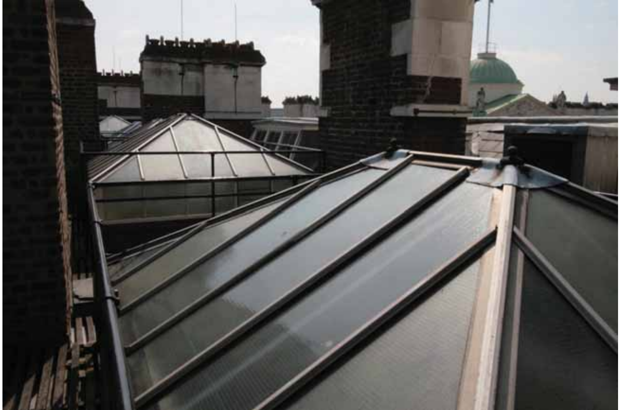
Plate 797: Lantern skylight over the Corridor 05T, looking south-west (EAF10 30)
