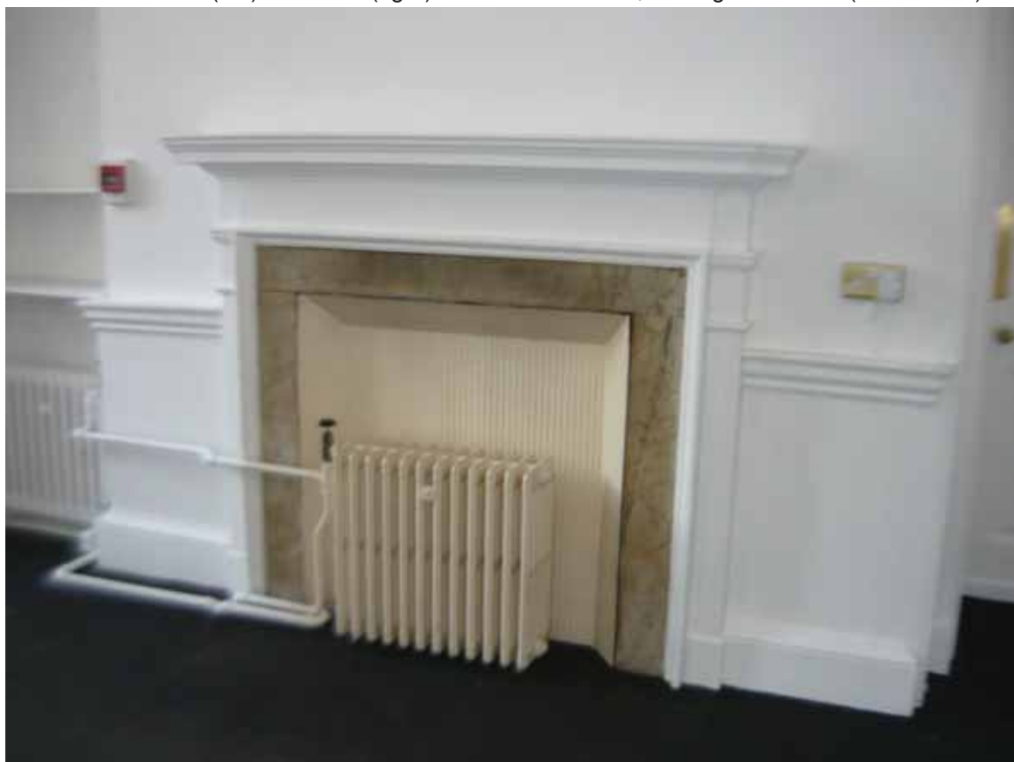
Plate 343: Fireplace (type 6) in the north wall of Room G01, looking north-west (EAF10 BHD1 (58))
