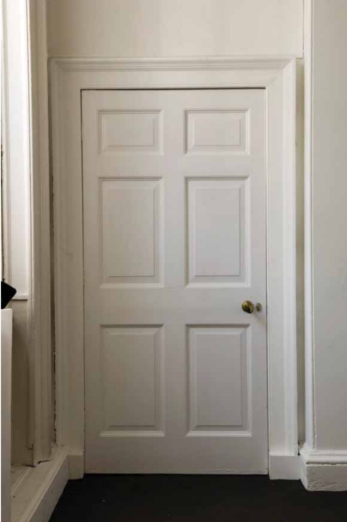
Plate 443: Doorway at the east end of the south wall in Room G26, looking south (EAF10 B100 0917)
