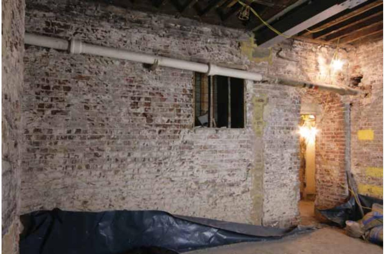
Plate 16: East wall of Room B43/B44, looking east (EAF10 A100 038)
