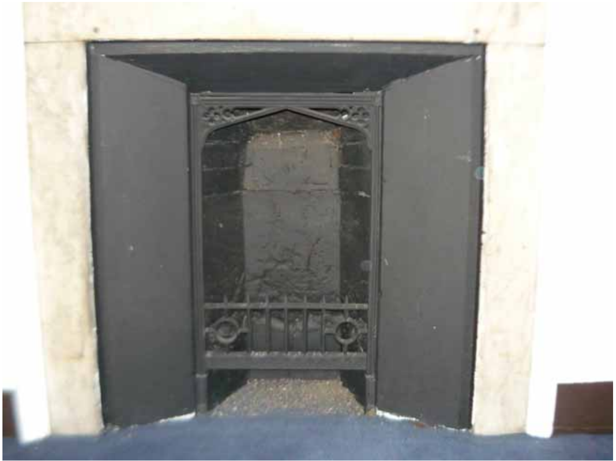
Plate 588: Fireplace (type 2) in the south wall of Room S15, looking south (EAF10 BHD1 (97))
