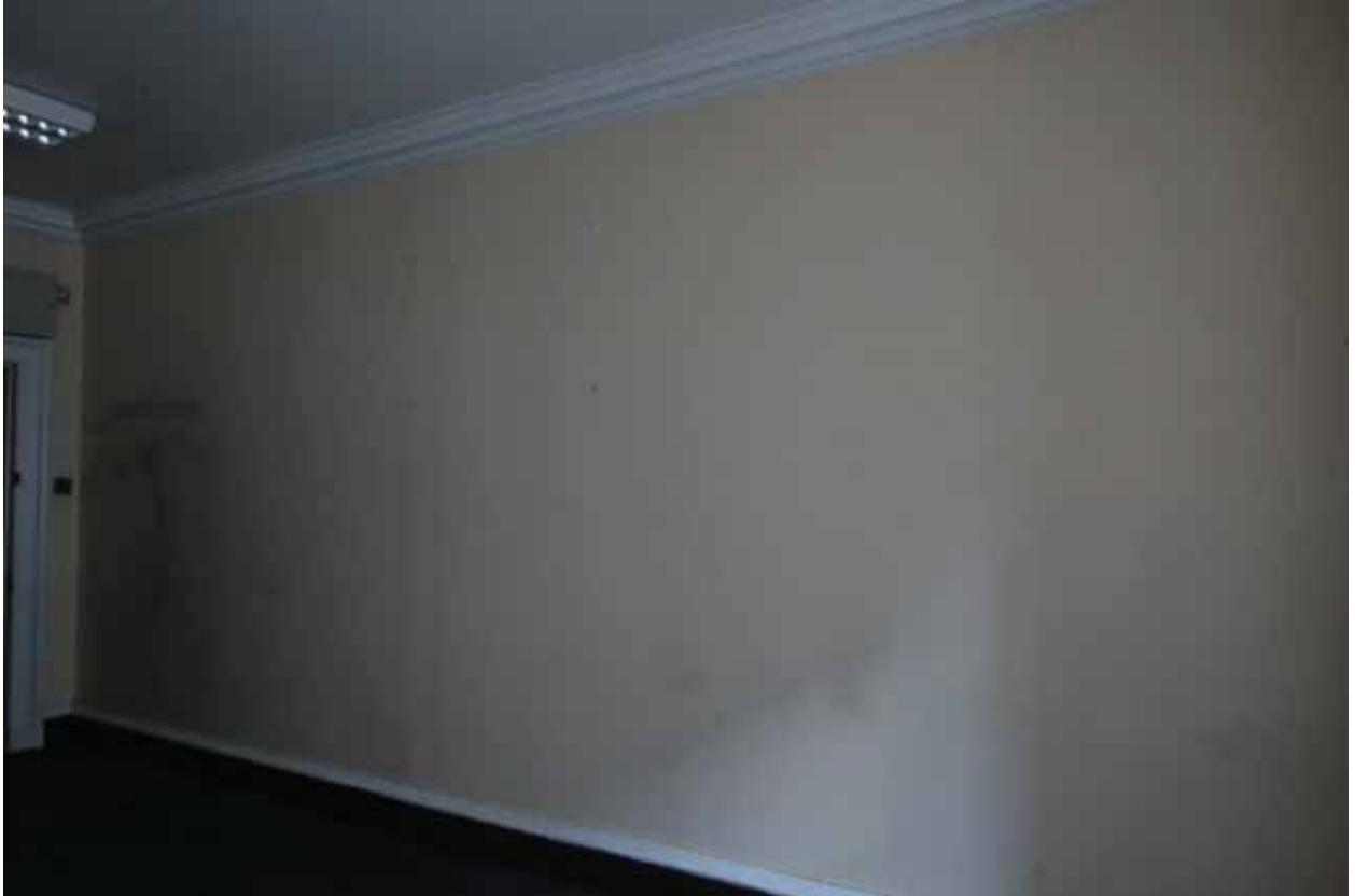
Plate 639: North partition wall in Room S25, looking north-west (EAF10 0117)
