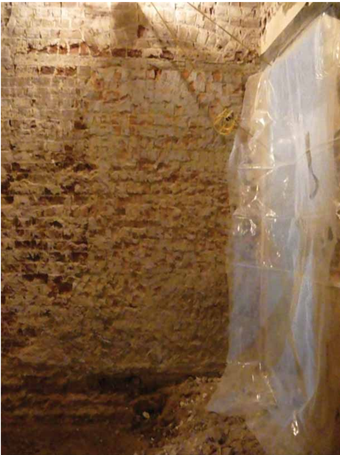
Plate 60: Blocked doorway at the south end of the east wall in Room B48D, looking east (EAF10 BHD6 (56))
