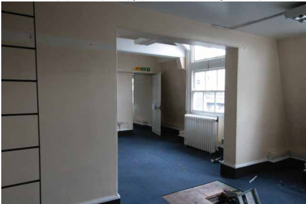
Plate 674: South partition (foreground) wall in Room T04, looking south-west (EAF10 47)
