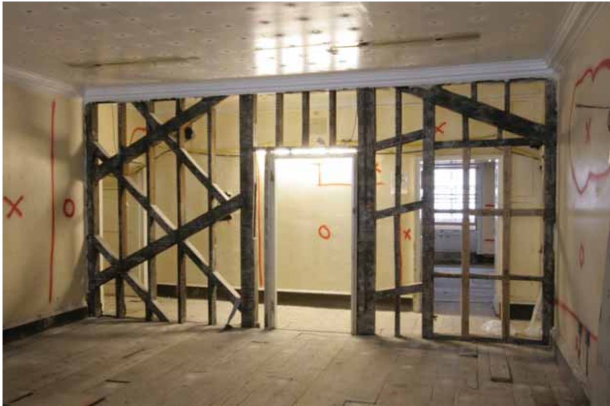
Plate 616: West partition wall in Room S16, looking west (EAF10 A100 015)
