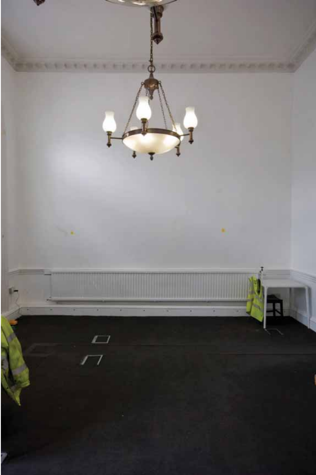
Plate 373: North wall of Room G09, looking north (EAF10 B100 0937)
