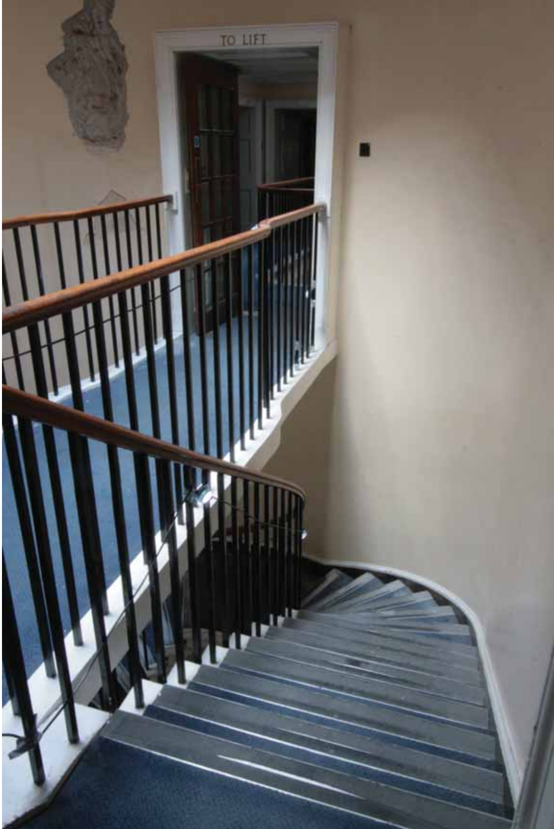
Plate 600: Link bridge in Stairs 02S looking north (EAF10 0131)
