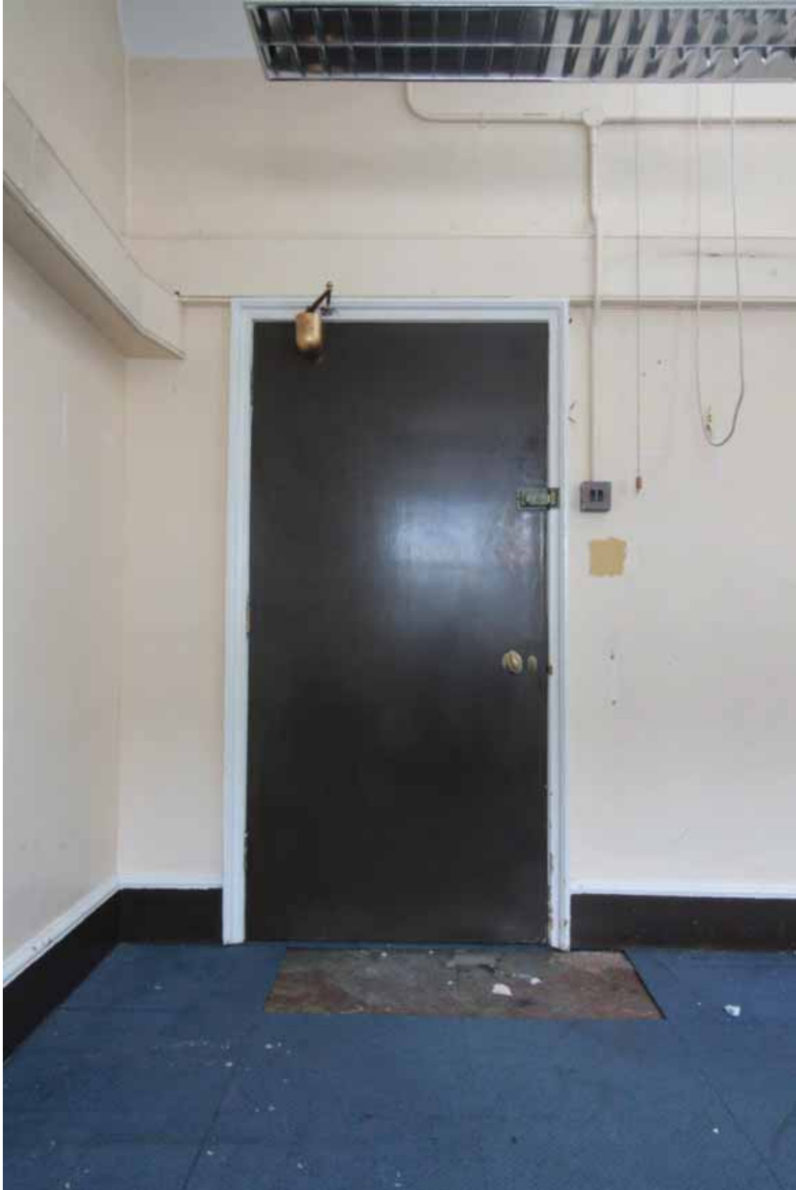
Plate 781: Doorway in the east wall of Room T25, looking east (EAF10 12)
