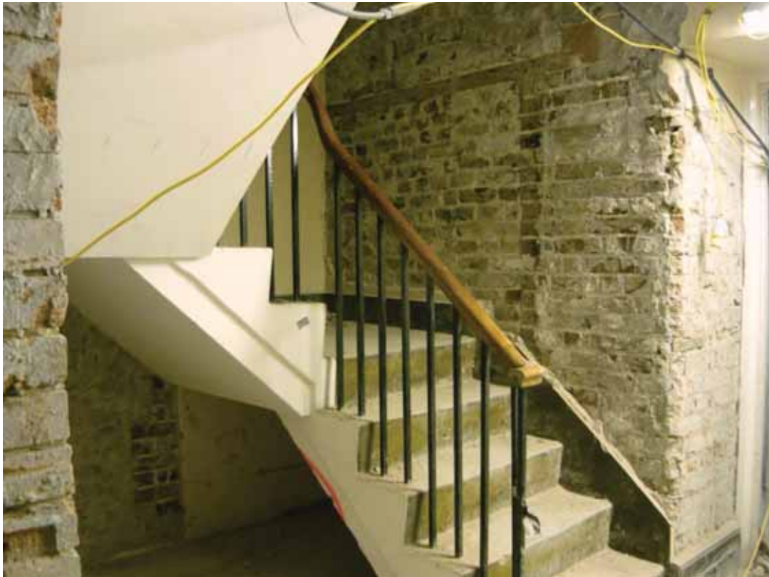
Plate 246: West (left) and north (right) walls of Corridor 06LG looking north-west (EAF10 BHD6 (90))
