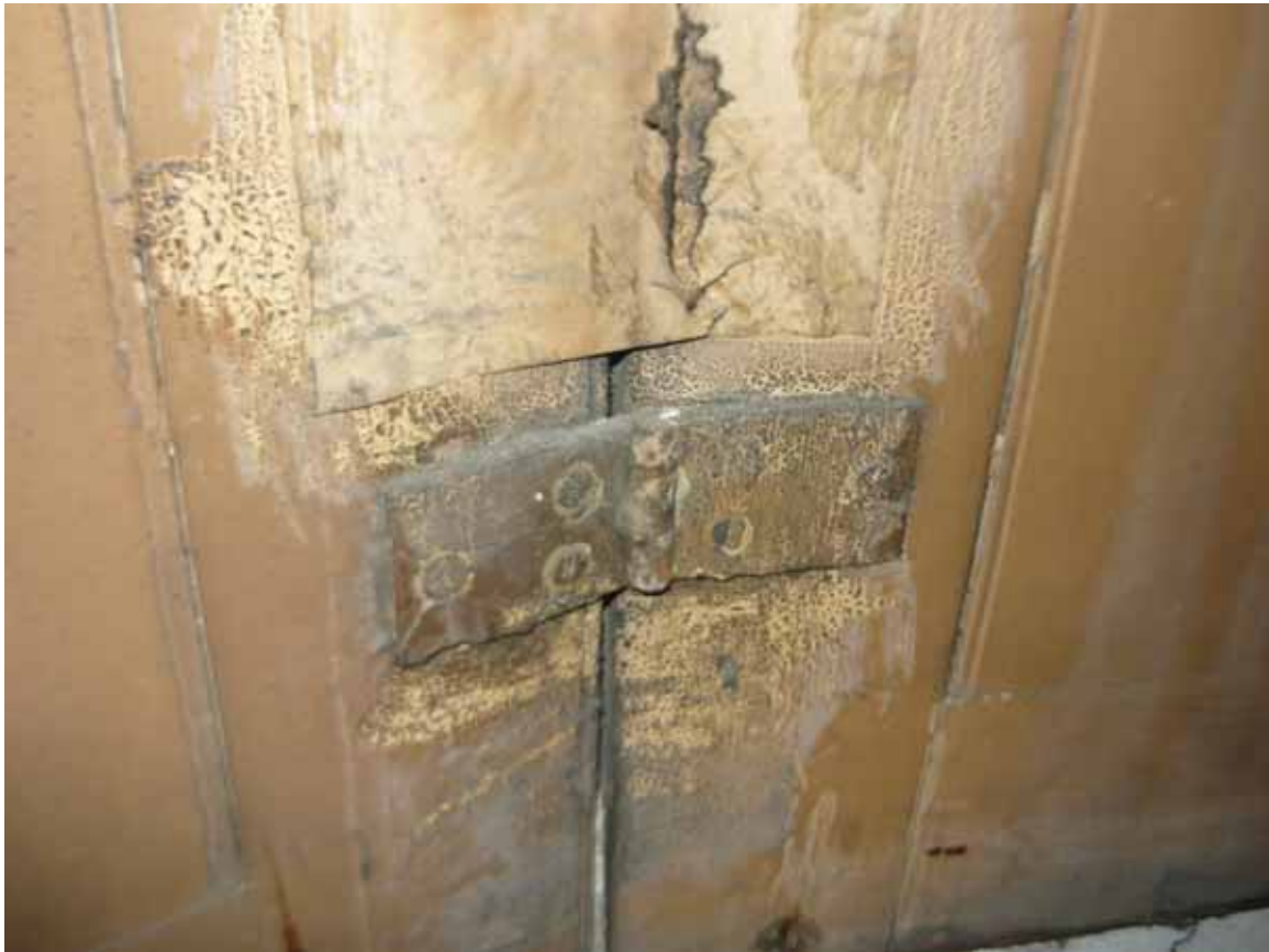
Plate 204: Hinge on window shutter in Room M16, looking west (EAF10 BHD3 (77))
