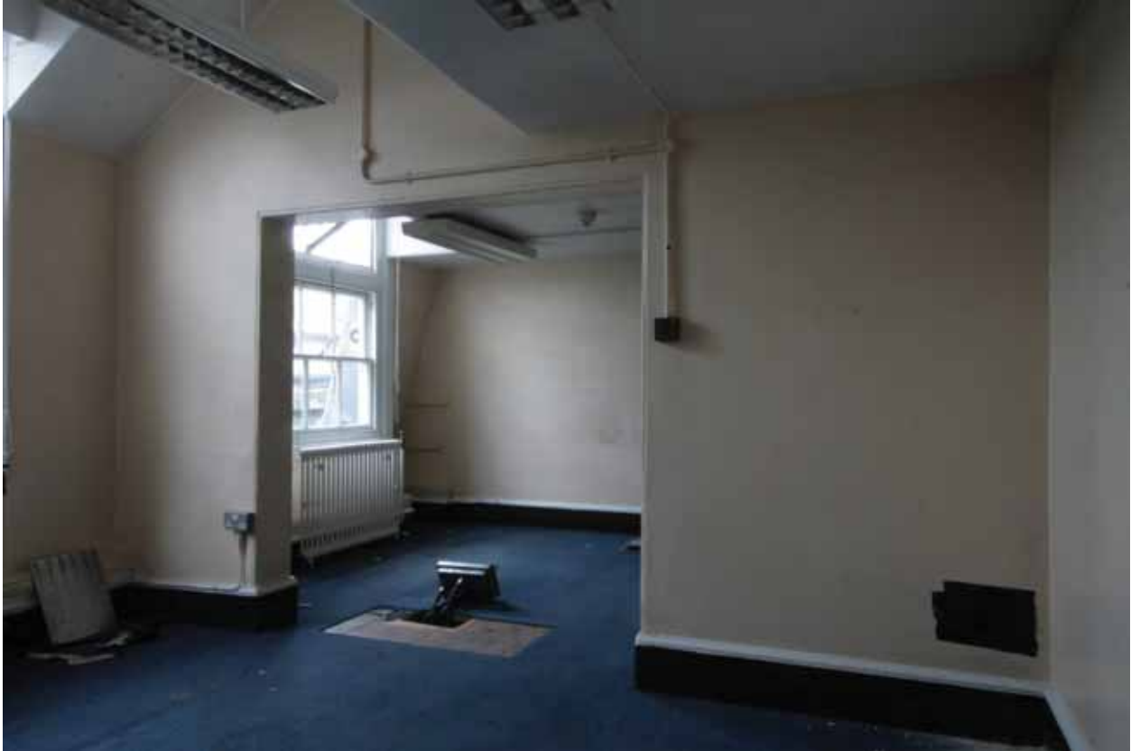
Plate 675: North partition (foreground) wall in Room T03, looking north-west (EAF10 47)
