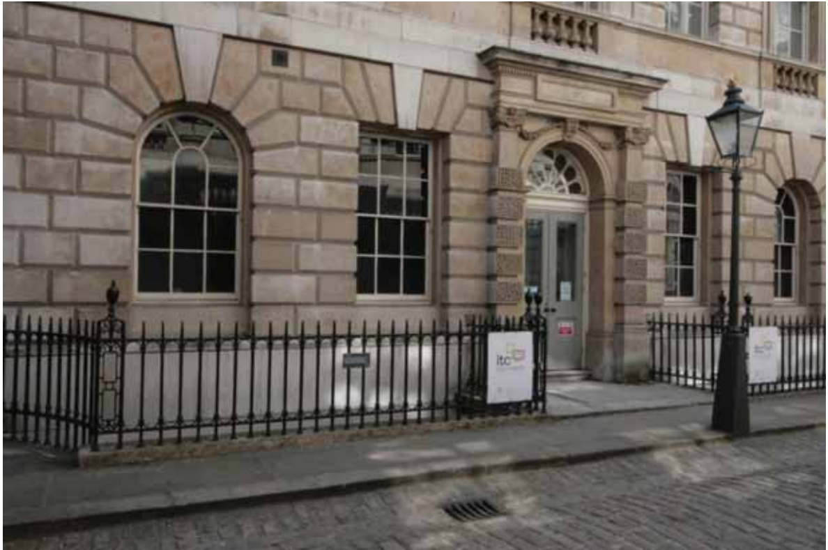
Plate 1c: Main ground floor entrance in the north (end) elevation of Somerset House East Wing, viewed from the north
