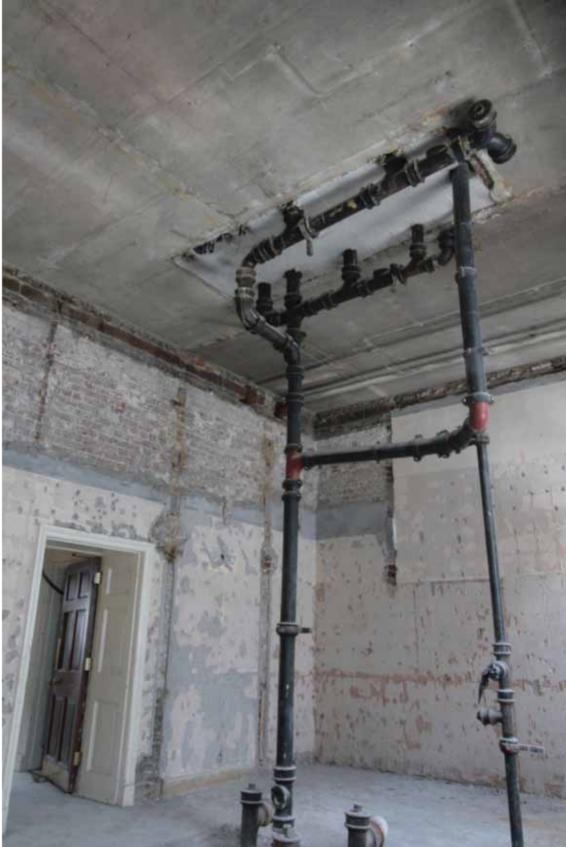
Plate 534: West (left) and north (right) walls in Room F20, looking north-west (EAF10 260)
