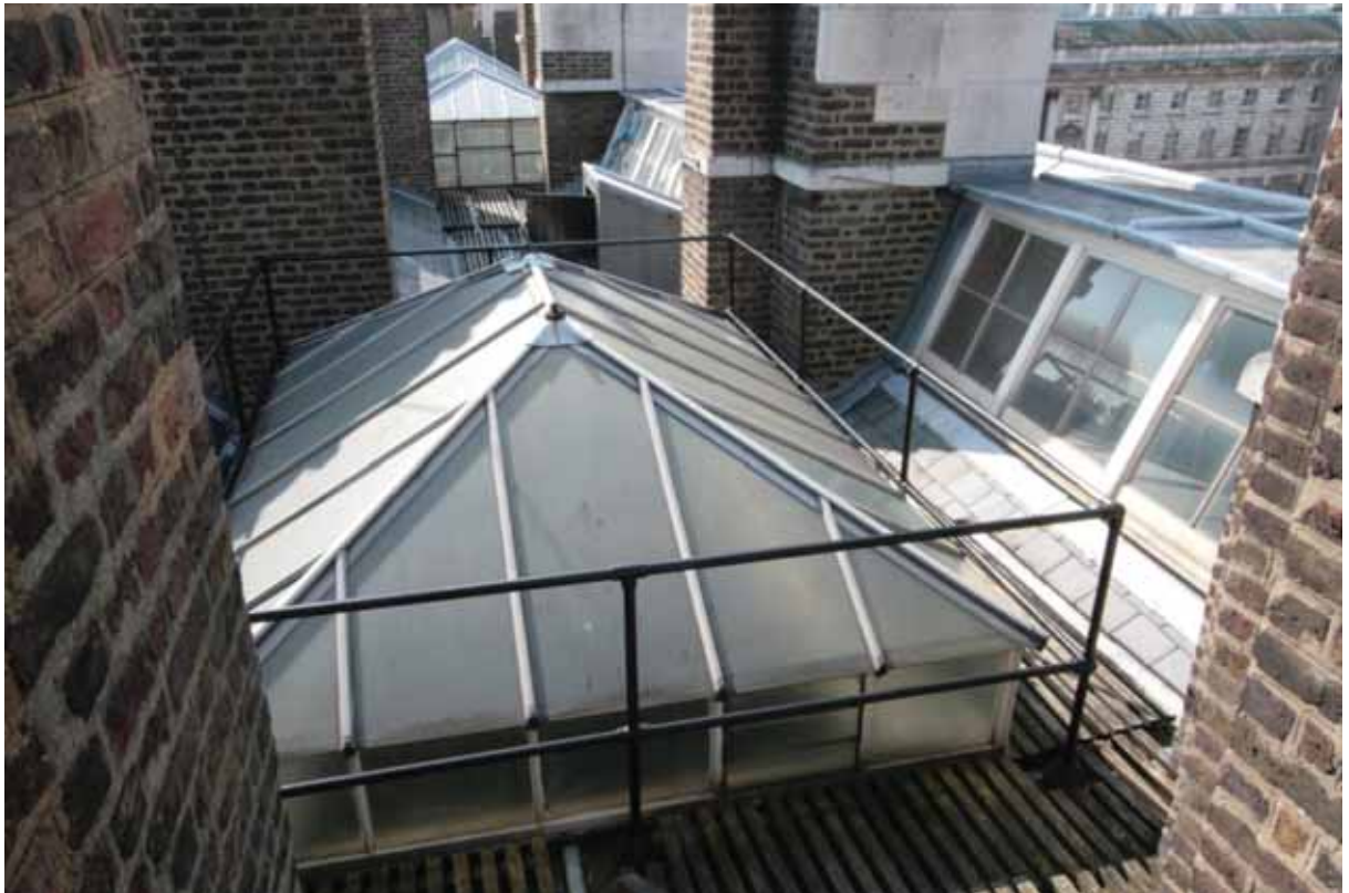
Plate 798: Lantern skylight over the Stairs 01T, looking south-west (EAF10 21a)
