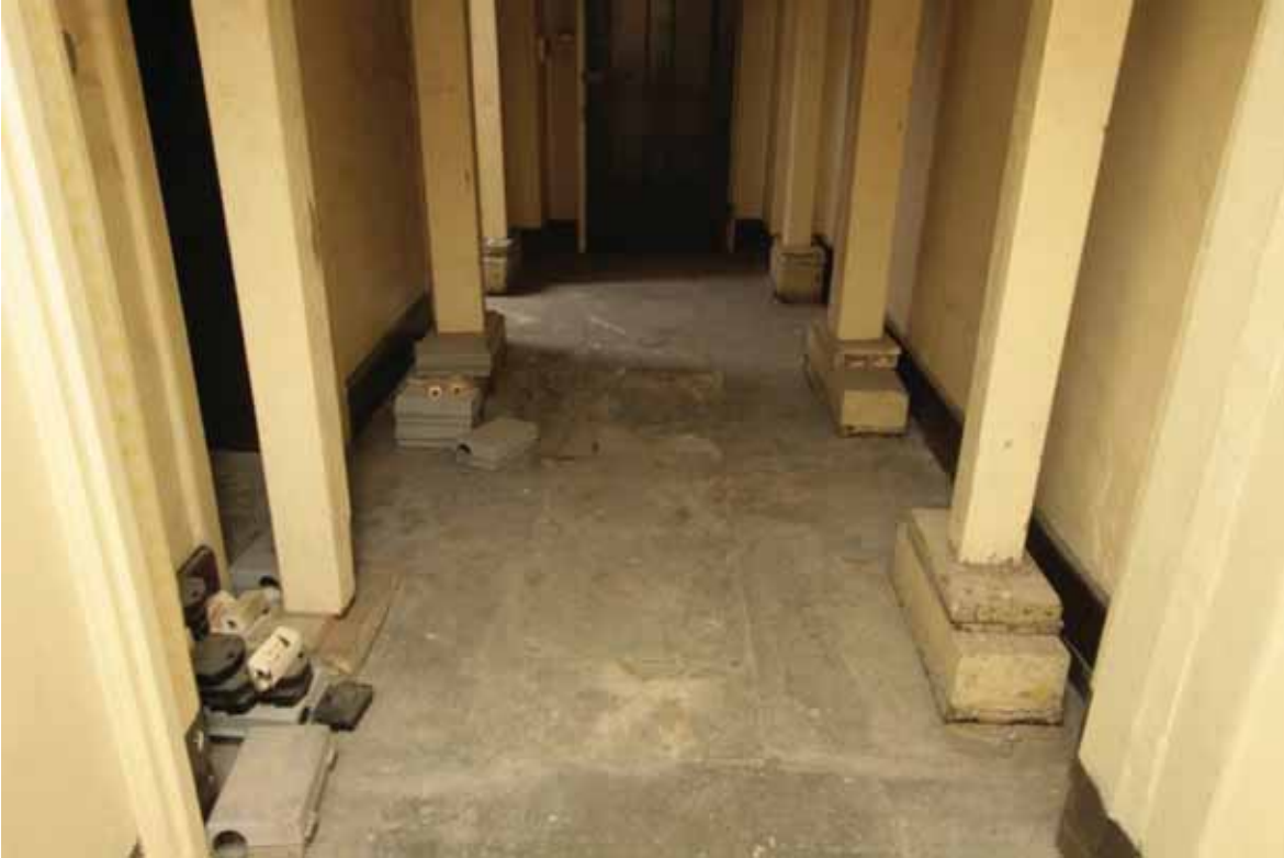
Plate 25: Corridor next to Rooms B45 and B46, looking west (EAF10 D100 026a)
