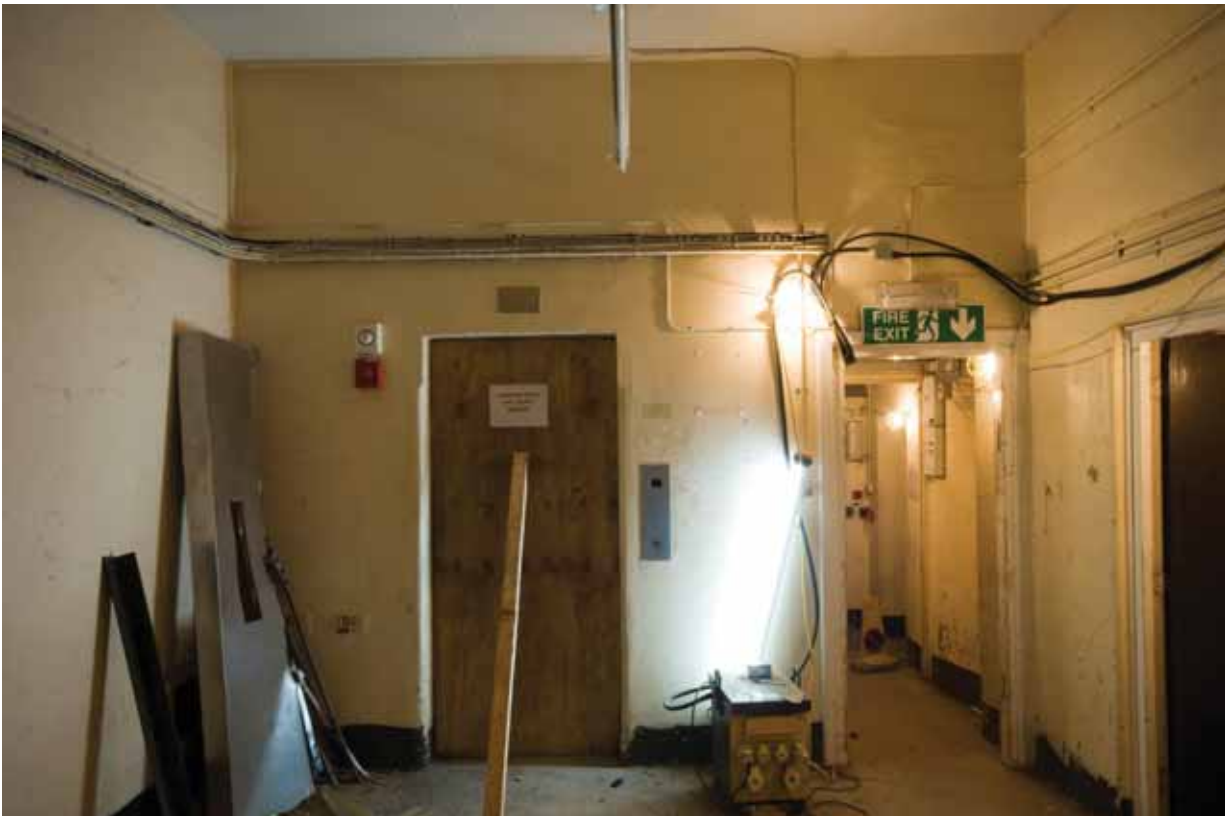
Plate 95: Corridor 3, looking south (DSC_1478 _sitecode EAF10_© PCA Ltd 2010)
