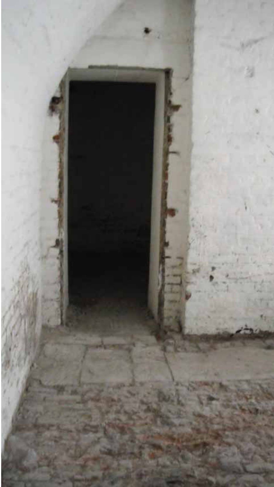
Plate 124: Doorway at the west end of the north wall in Room B50, looking north (EAF10 BHD4 (15))
