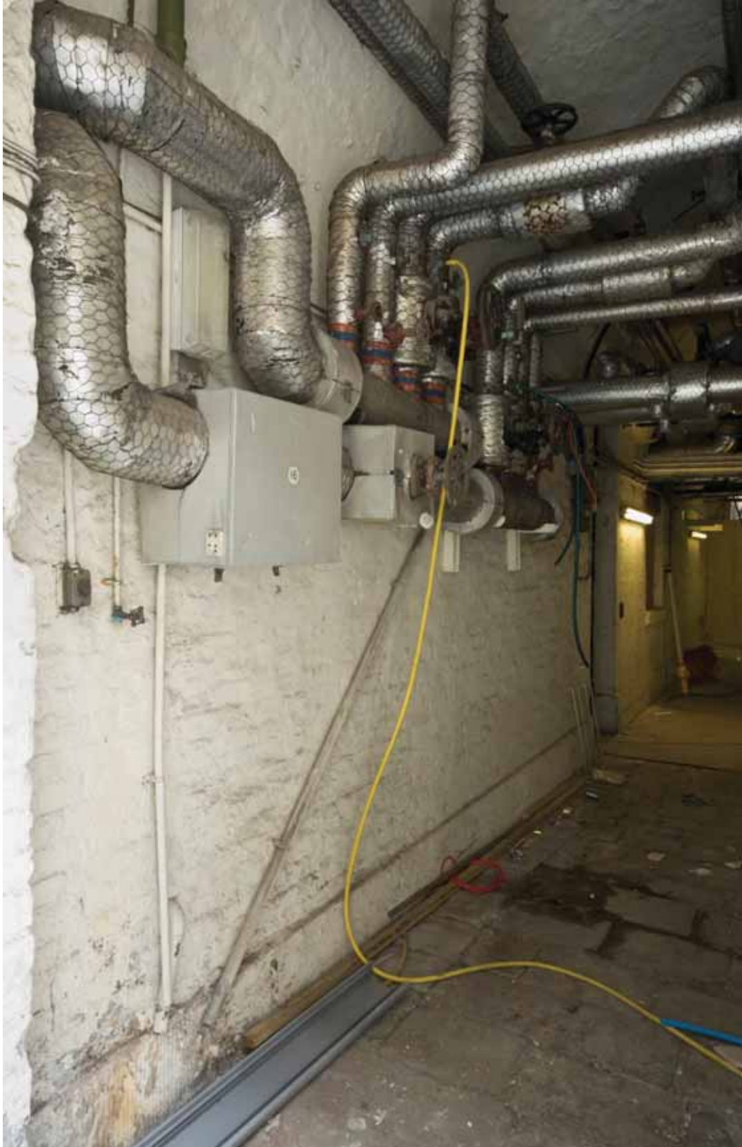
Plate 101: South wall of Corridor 5, looking south-west (DSC_1385_sitecode EAF10_© PCA Ltd 2010)
