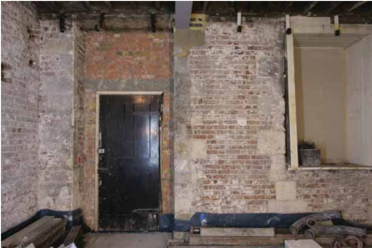
Plate 14: West wall of Room B43/B44, looking west (EAF10 A100 037)
