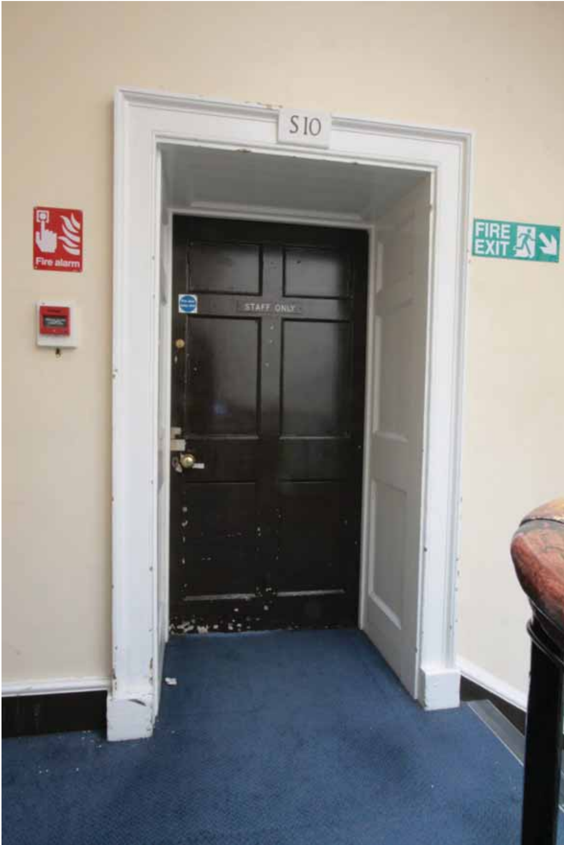
Plate 590: Doorway in the west wall of Stairs 01S, looking west (EAF10 0095)
