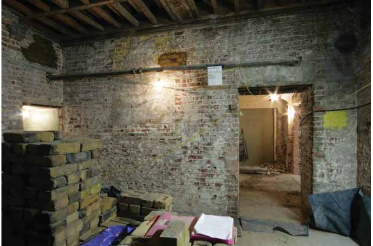
Plate 148: West wall in Room B53, looking west (EAF10 A100 041)
