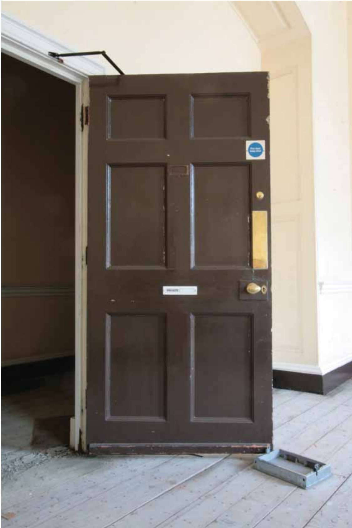
Plate 458: Doorway in the east wall of Room F01, looking south-east (EAF10 175)
