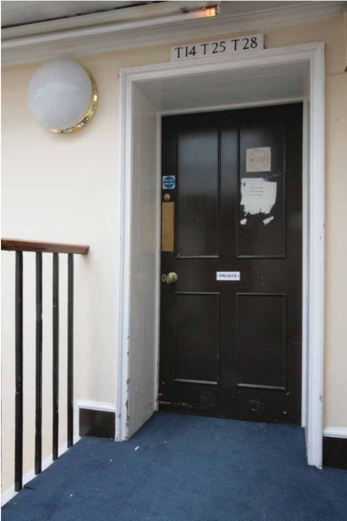
Plate 708: Doorway in the east wall of Stairs 01T, looking east (EAF10 13)
