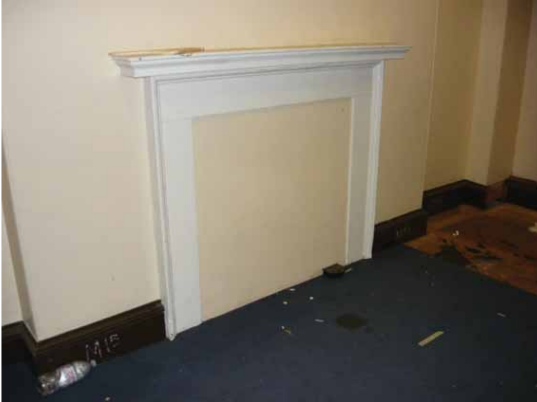
Plate 207: Fireplace in the south wall of Room M15, looking south-west (EAF10 BHD1 (21))
