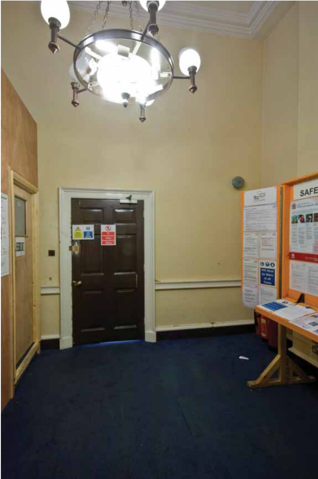
Plate 377: East wall in Room G15, looking east (EAF10 B100 0938)
