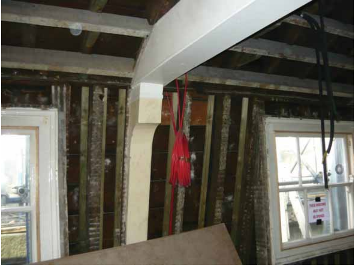
Plate 659: West wall in Room T119, looking north-west (EAF10 BHD10 (53))
