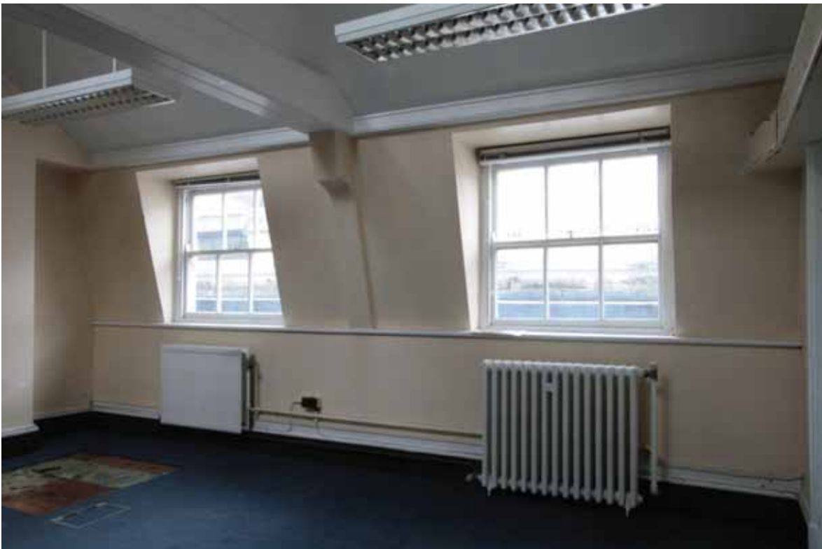
Plate 776: East wall of Room T25, looking east (EAF10 8)
