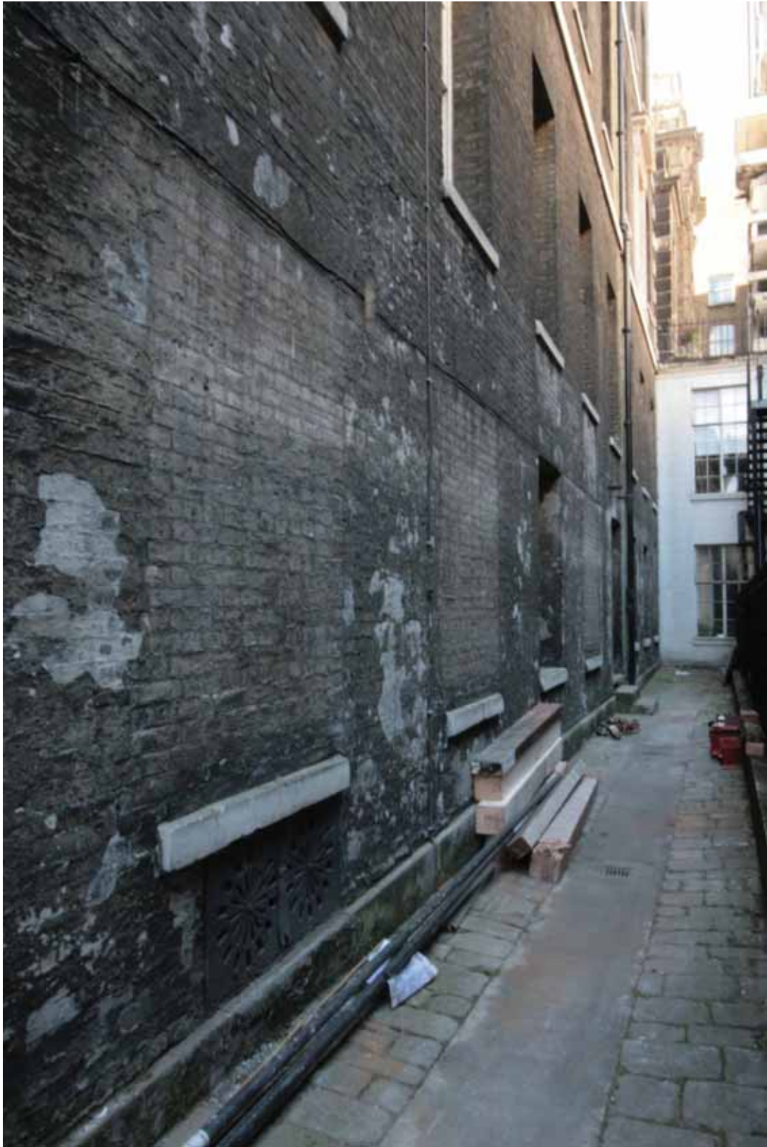
Plate 3: Bricked up basement window openings in the east (rear) elevation of Somerset House East Wing, viewed from the south-east
