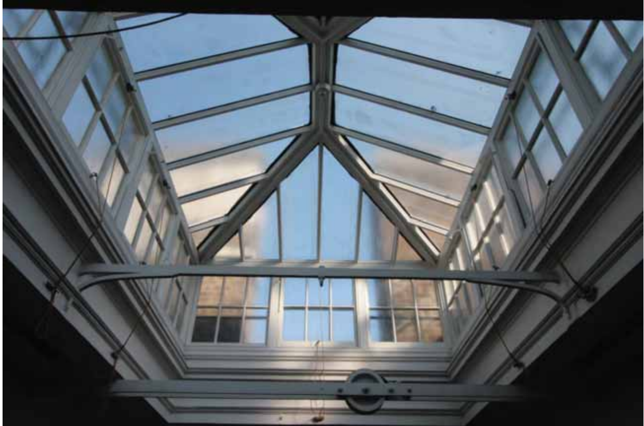
Plate 710: Skylight over Corridor 02T, looking north (EAF10 20)
