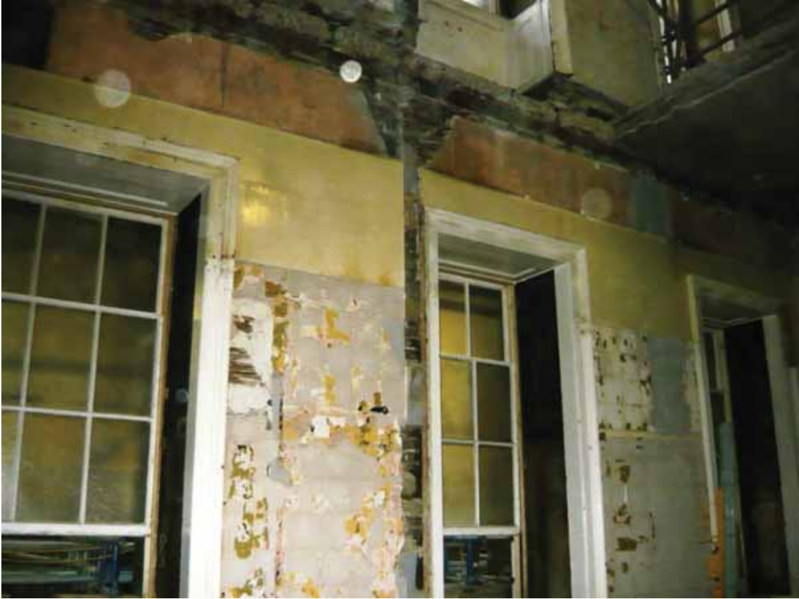
Plate 289: East wall in Room M116, looking east (EAF10 BHD8 (77))
