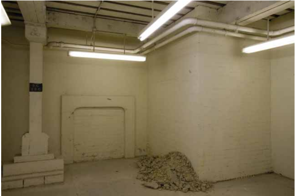
Plate 36: North wall of Room B47A, looking north (EAF10 D100 032)
