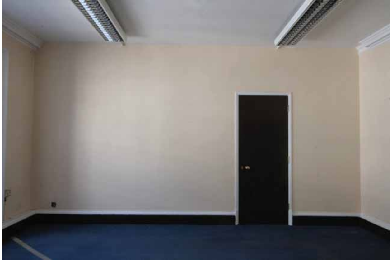
Plate 611: South partition wall in Room S93, looking south (EAF10 0163)
