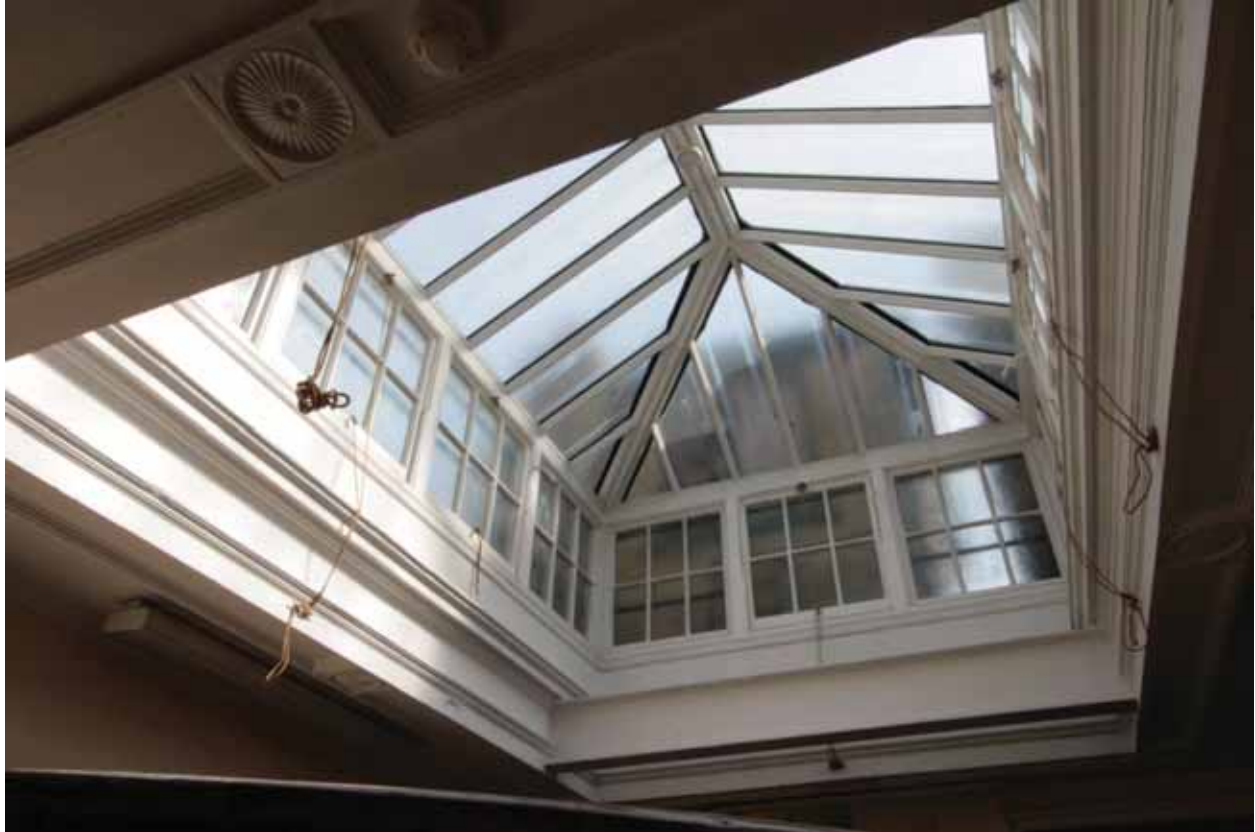
Plate 713: Skylight over Corridor 03T, looking south-east (EAF10 34)
