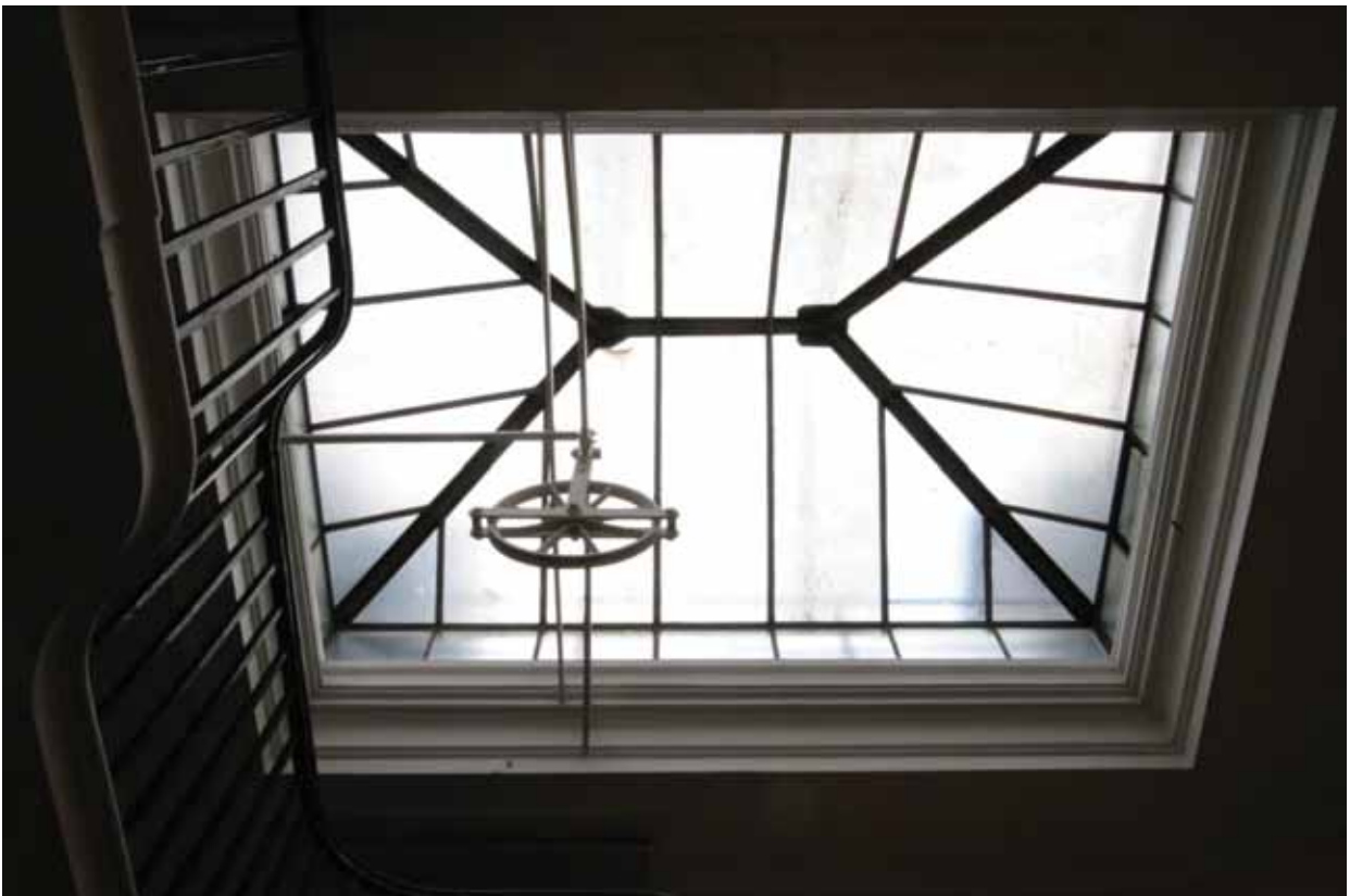
Plate 707: Skylight over Stairs 01T, looking west (EAF10 14)
