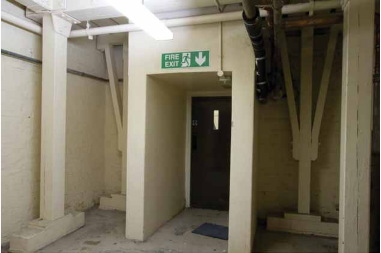
Plate 65: South door in Room B63, looking south (EAF10 D100 001a)
