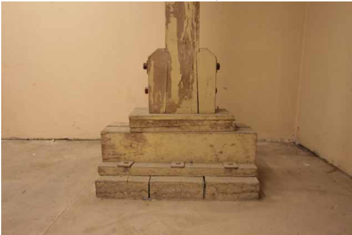
Plate 56: North-east corner of Room B48A, looking north (EAF10 D100 036)
