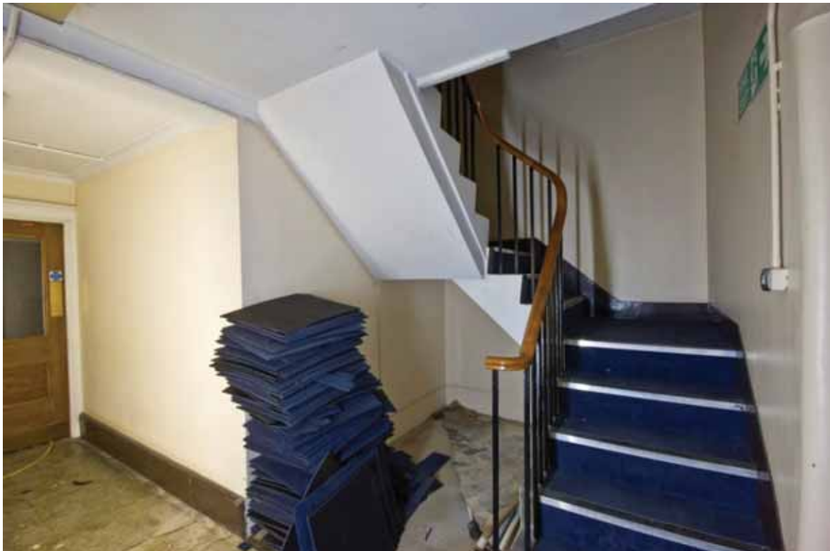
Plate 240: Corridor 06LG looking south-west towards dumb waiter (EAF10 LG100 1004)
