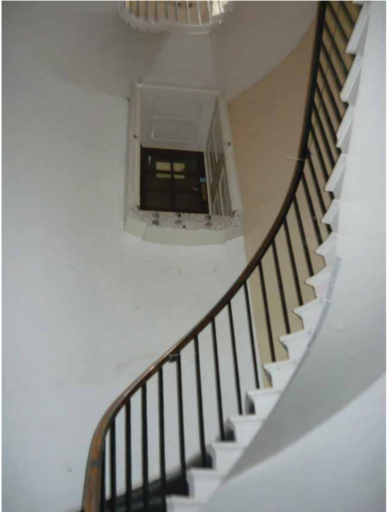
Plate 503: Removed link bridge in Stairs 02F looking north (EAF10 BHD3 (43))
