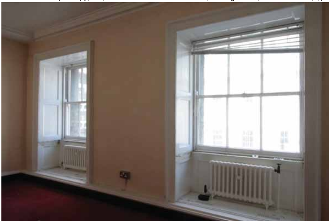
Plate 644: East wall in Room S27, looking north-east (EAF10 0104)
