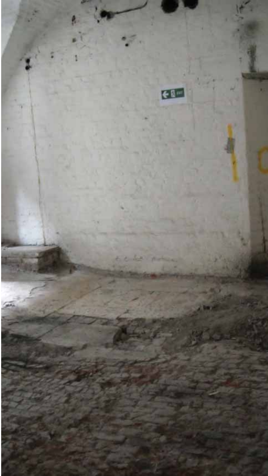
Plate 127: South wall in Room B50, looking south (EAF10 BHD4 (10))
