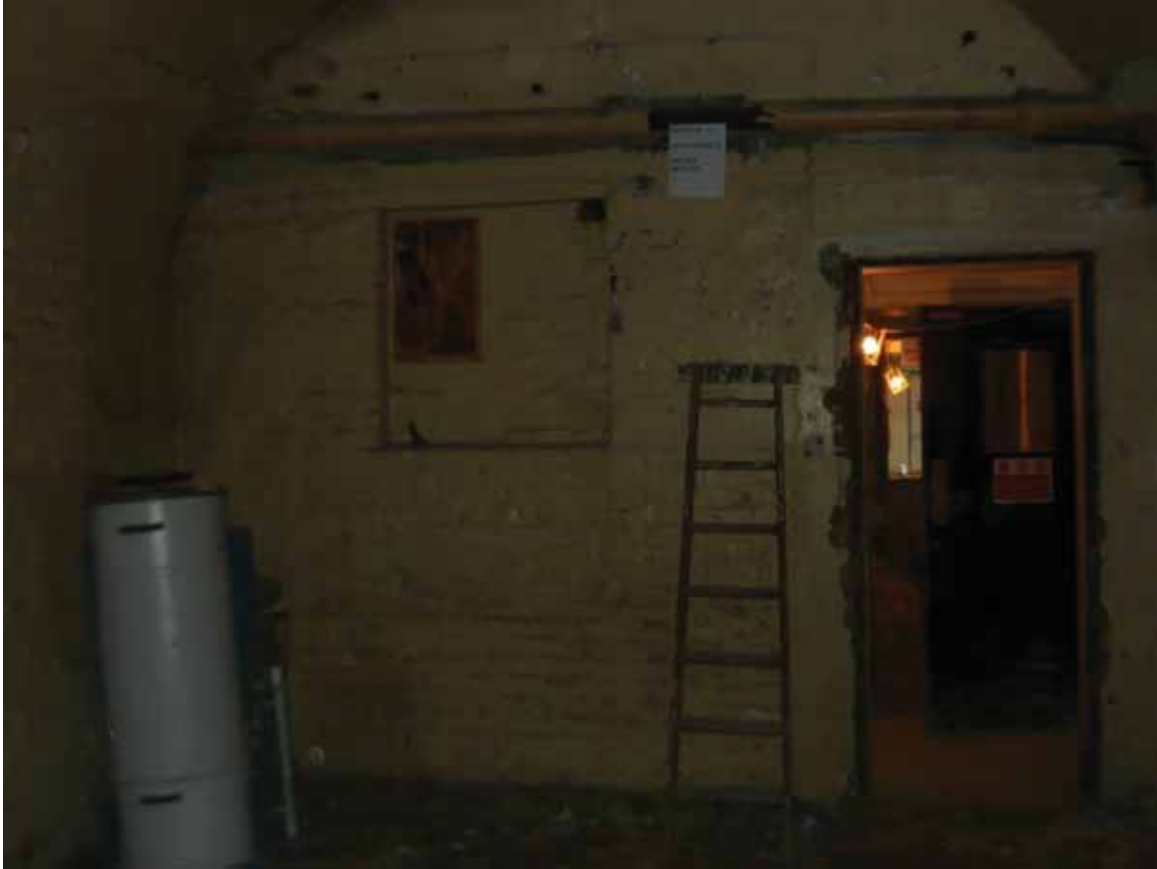
Plate 9: East wall of Room B42, looking east (EAF10 BHD5 (205))
