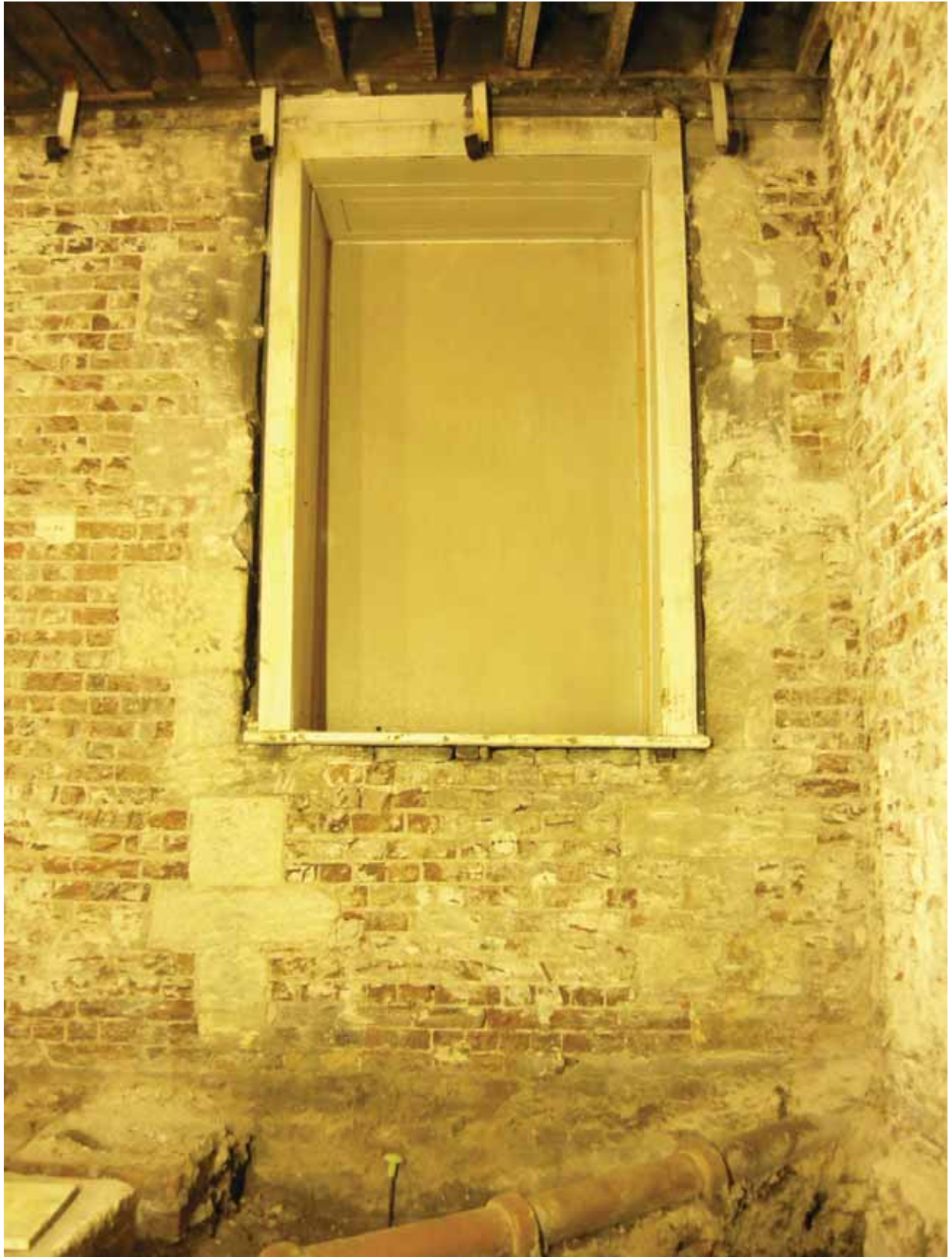
Plate 15: West wall of Room B43/B44, looking west (EAF10 BHD6 (131))
