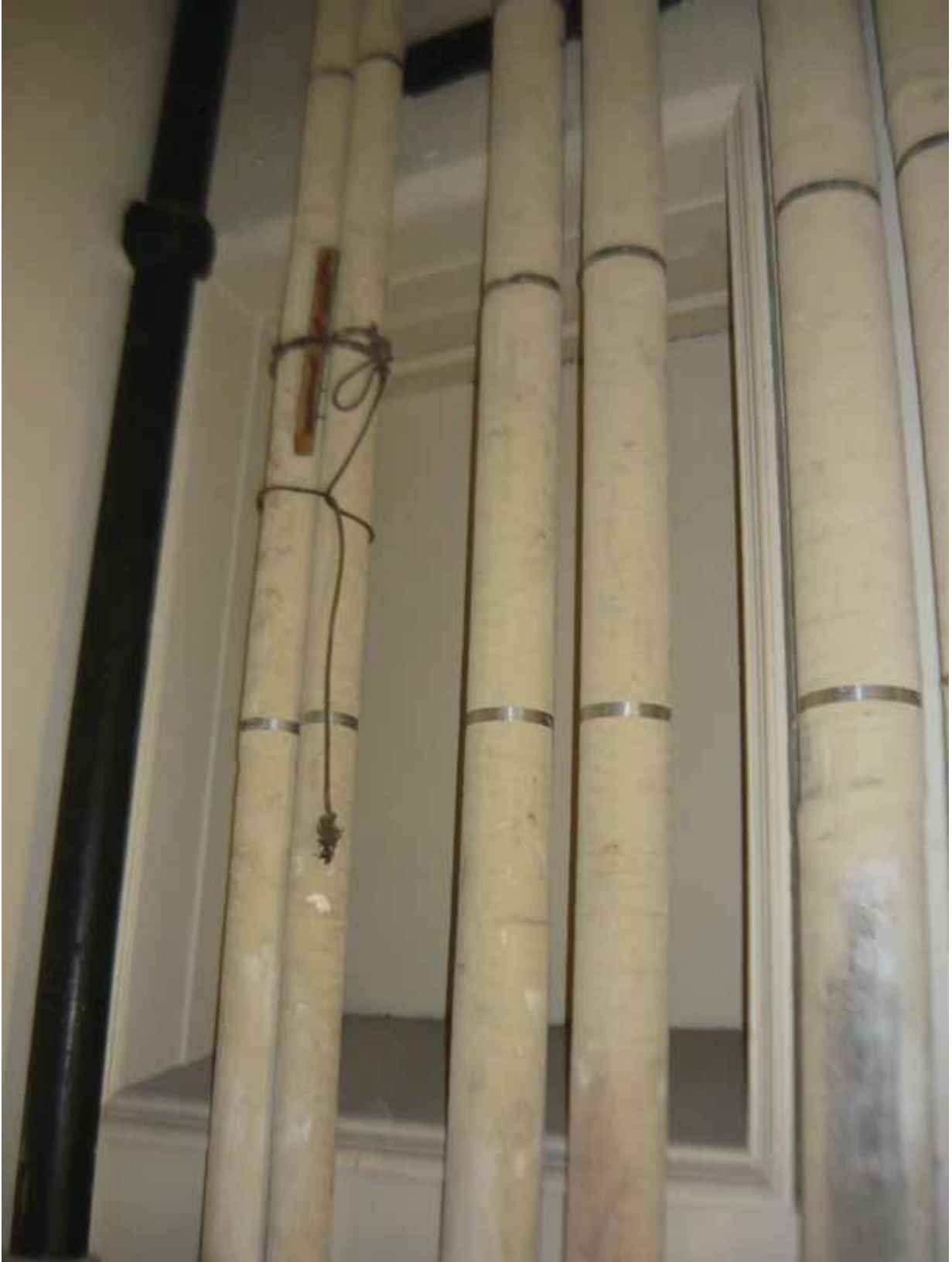
Plate 230: Recess marking the position of a former internal window at the north end of the east wall in Cupboard 01LG, looking north-east (EAF10 BHD3 (106))
