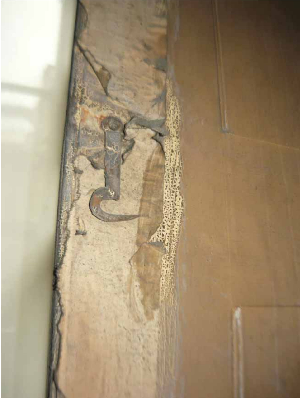
Plate 205: Hook on window shutter in Room M16, looking west (EAF10 BHD3 (78))
