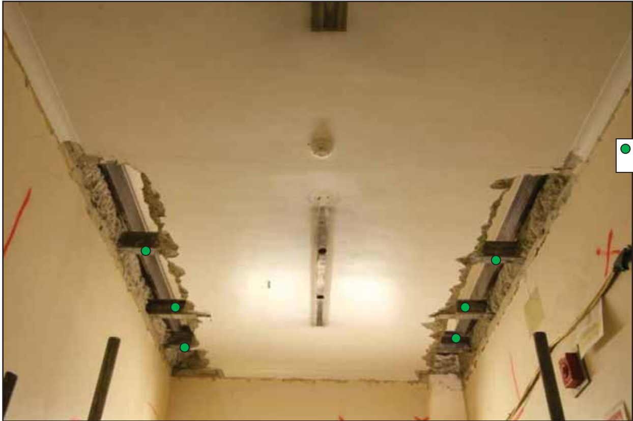
Plate 607: Ceiling of Corridor 09S looking south (EAF10 A100 018)
