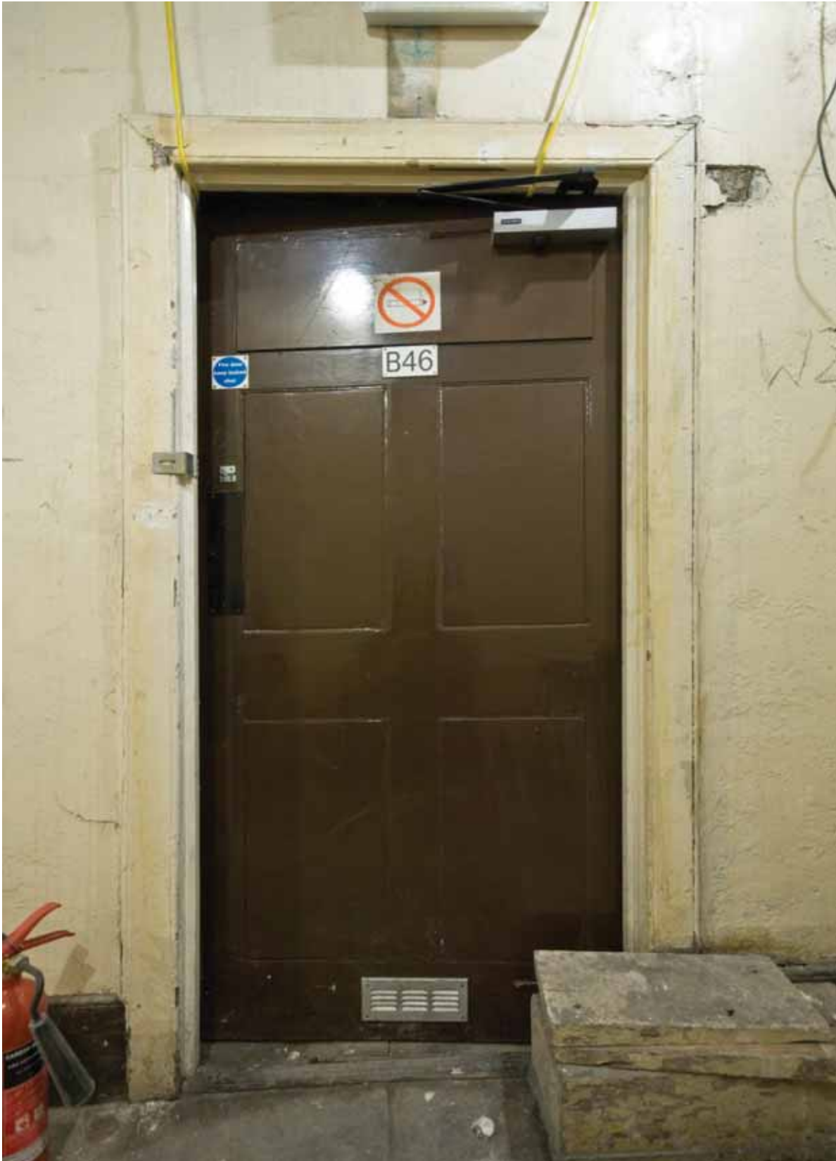
Plate 18: Door into Room B46 from Corridor, looking south (DSC_1469 _sitecode EAF10_© PCA Ltd 2010)
