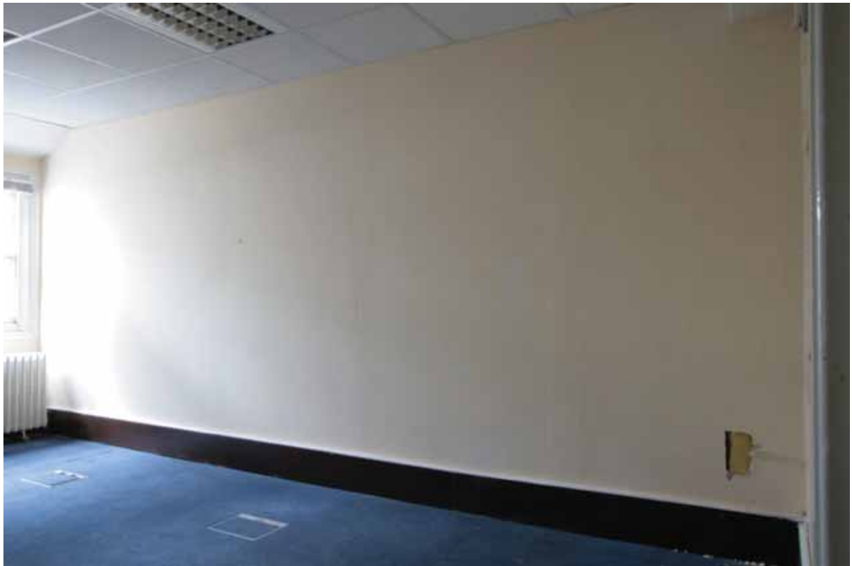
Plate 648: North partition wall in Room T120A, looking north-west (EAF10 58)
