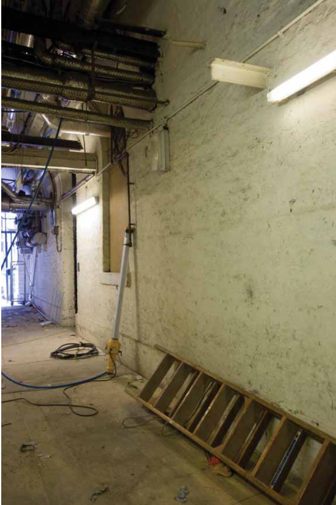
Plate 100: South wall of Corridor 5, looking south-east (DSC_1382_sitecode EAF10_© PCA Ltd 2010)
