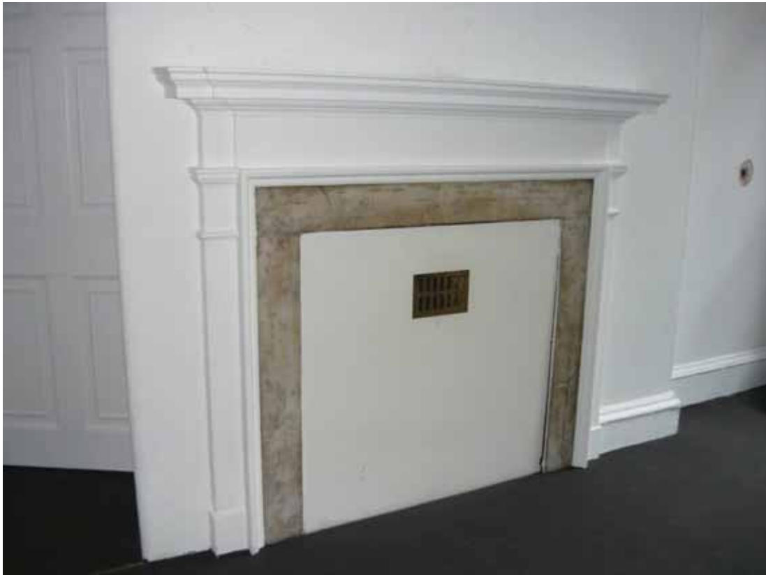
Plate 442: Fireplace (type 6) in the north wall of Room G26, looking north (EAF10 BHD1 (40))
