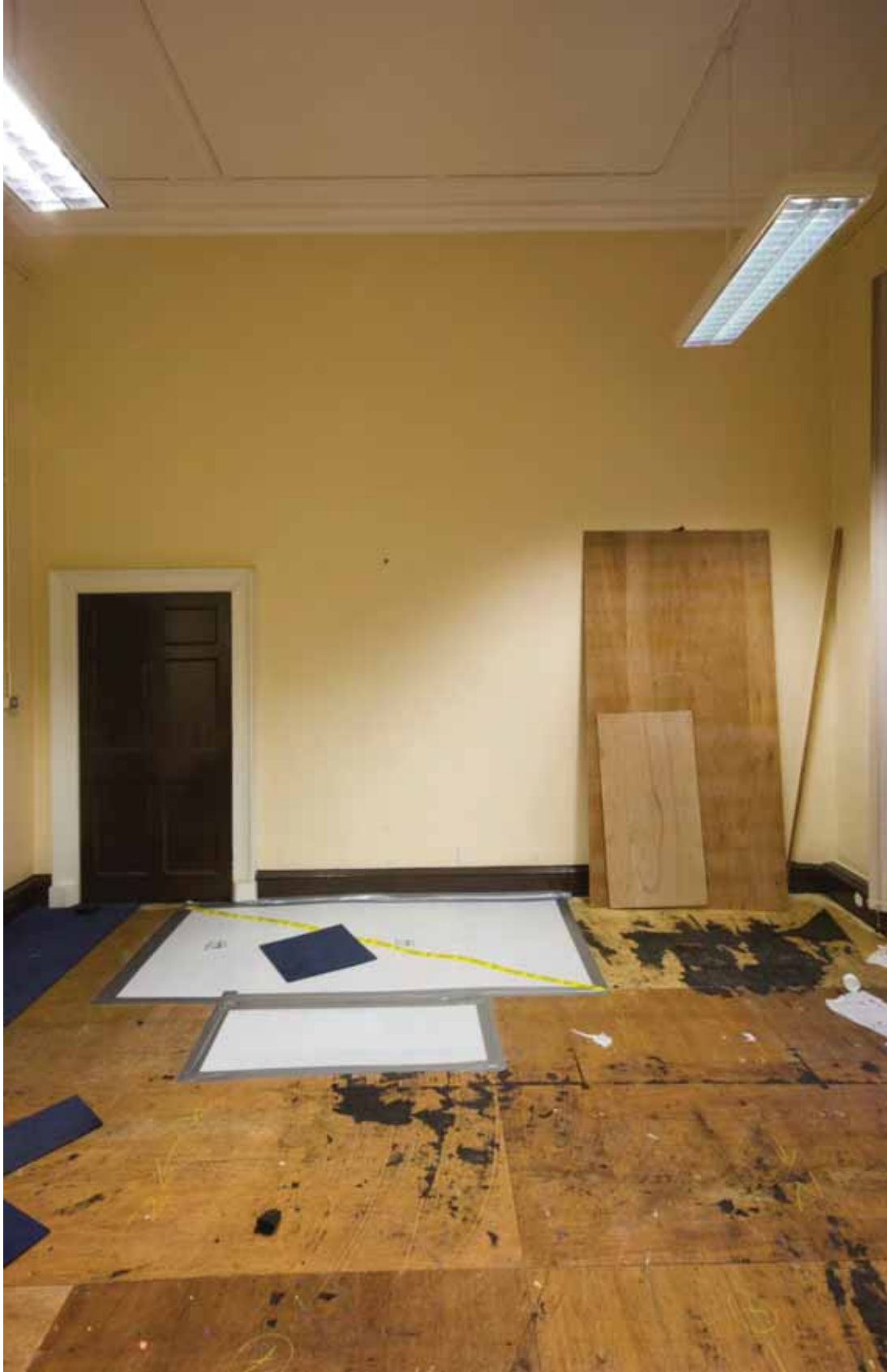
Plate 197: South wall in Room M16, looking south (EAF10 LG100 1091)
