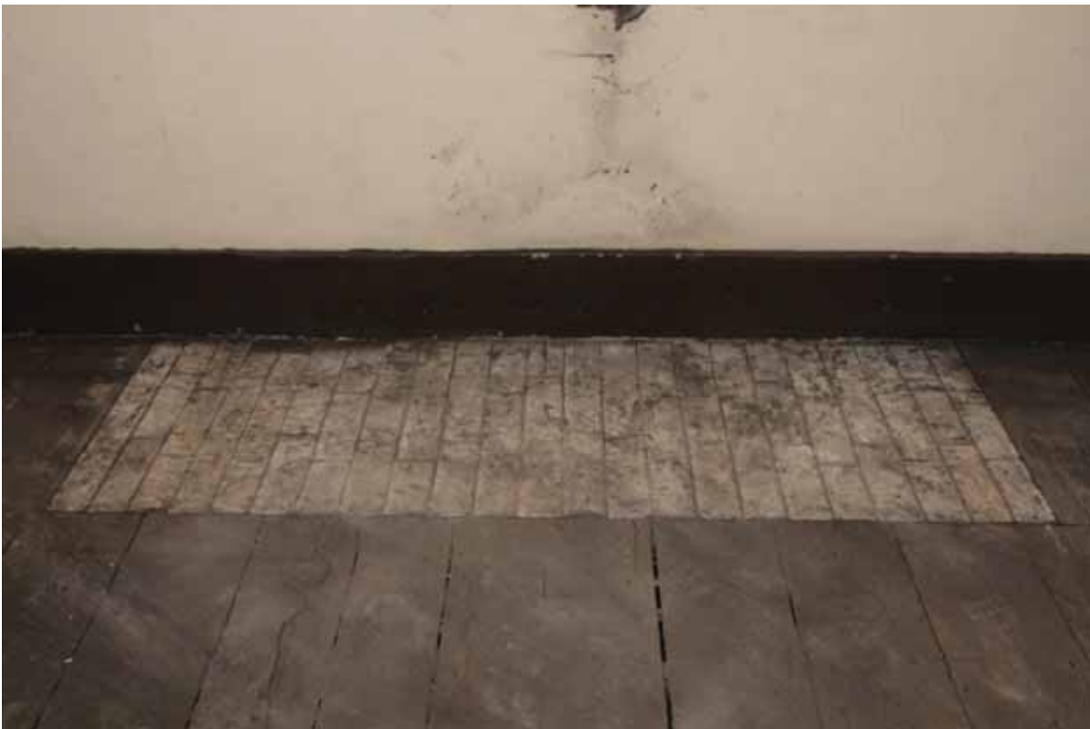
Plate 186: Hearth in front of the infilled fireplace in the north wall of Room M10, looking north (EAF10 307)
