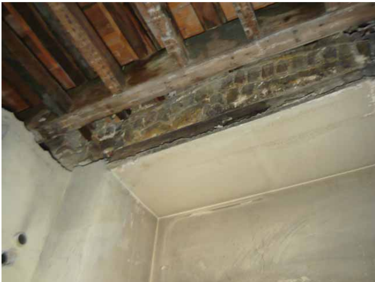
Plate 164: Brick segmental arch visible over the east doorway in Room B54A, looking north-east (EAF10 BHD5 (187))
