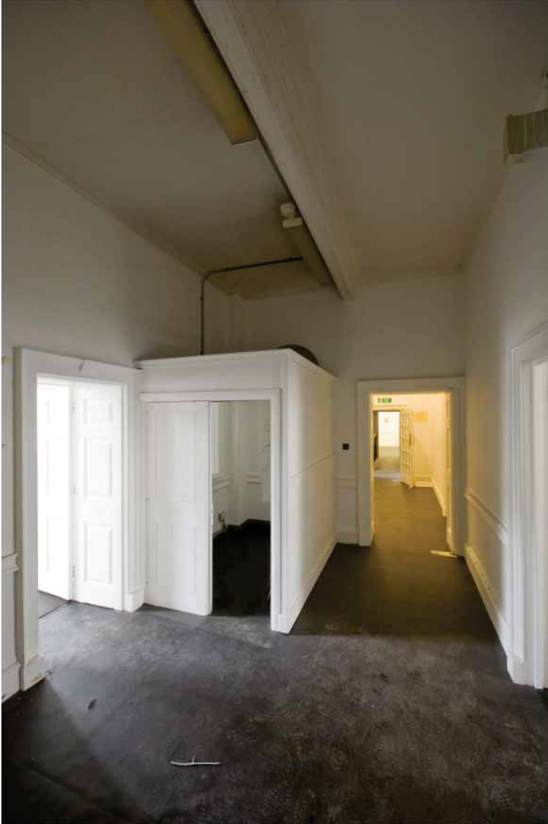
Plate 388a: Corridor 07G looking north-west (DSC_0827 sitecode EAF10 © PCA Ltd 2010_1)
