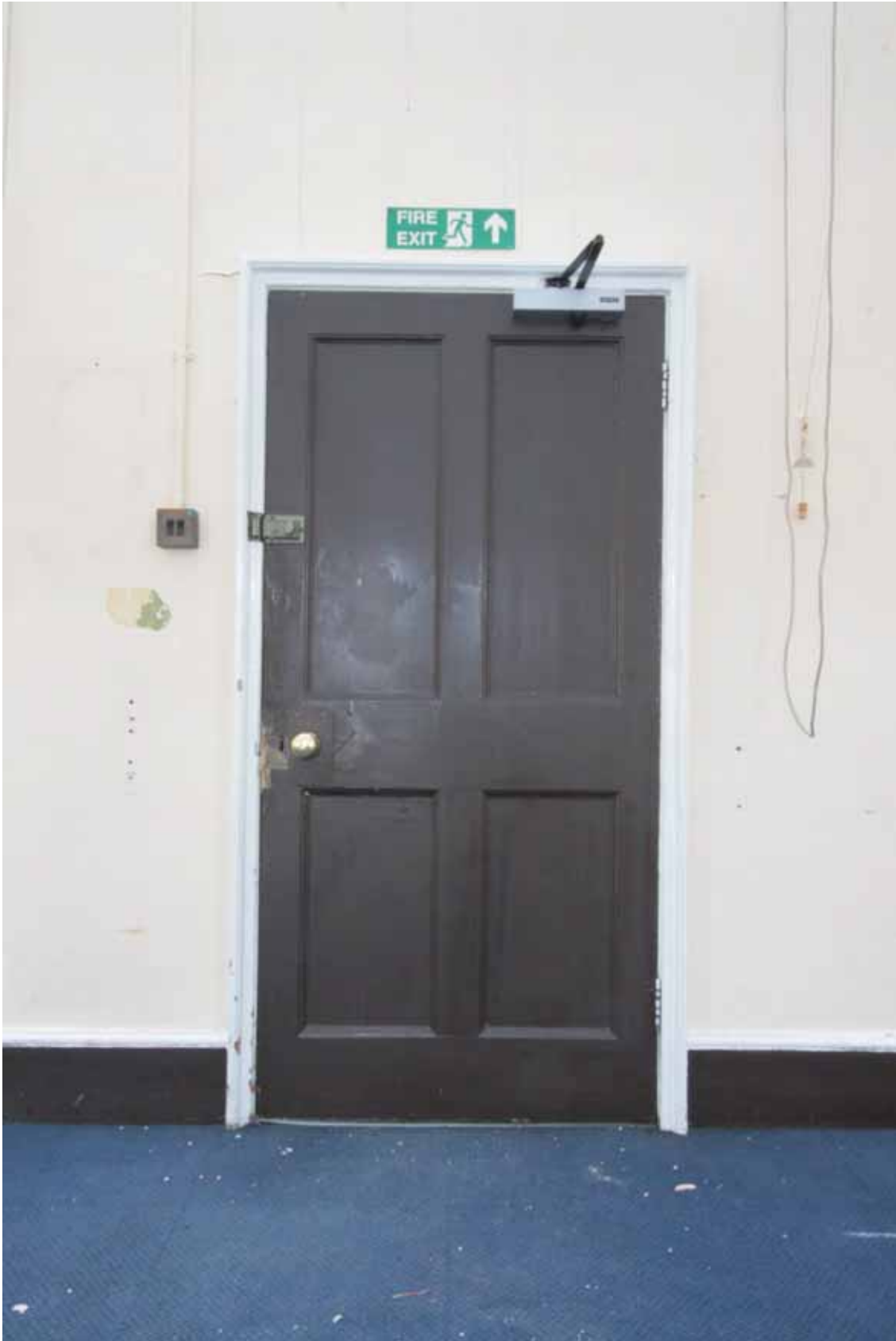
Plate 687: Doorway in the east wall of Room T08, looking east (EAF10 31)
