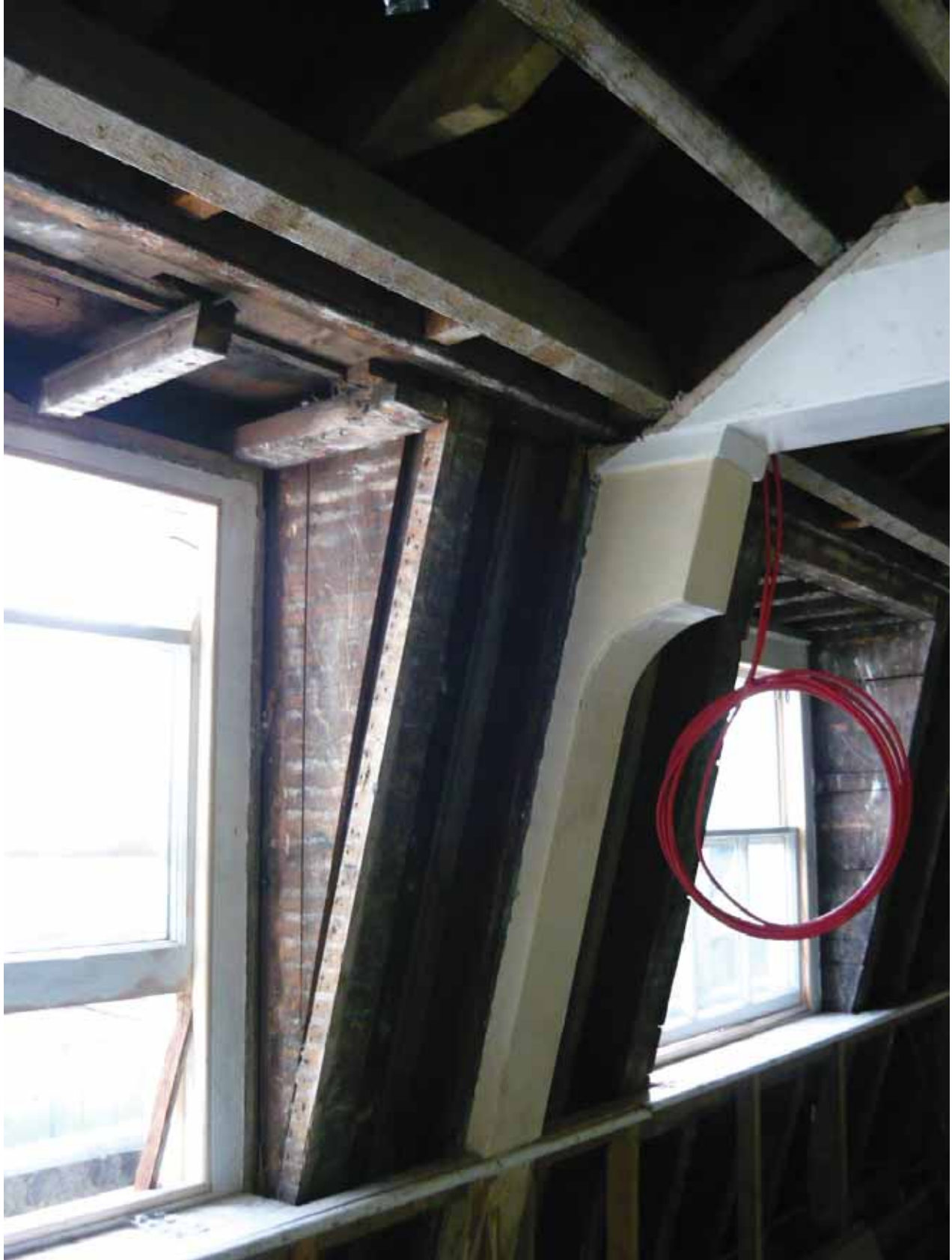
Plate 732: East wall in Room T115, looking south-east (EAF10 BHD10 (44))
