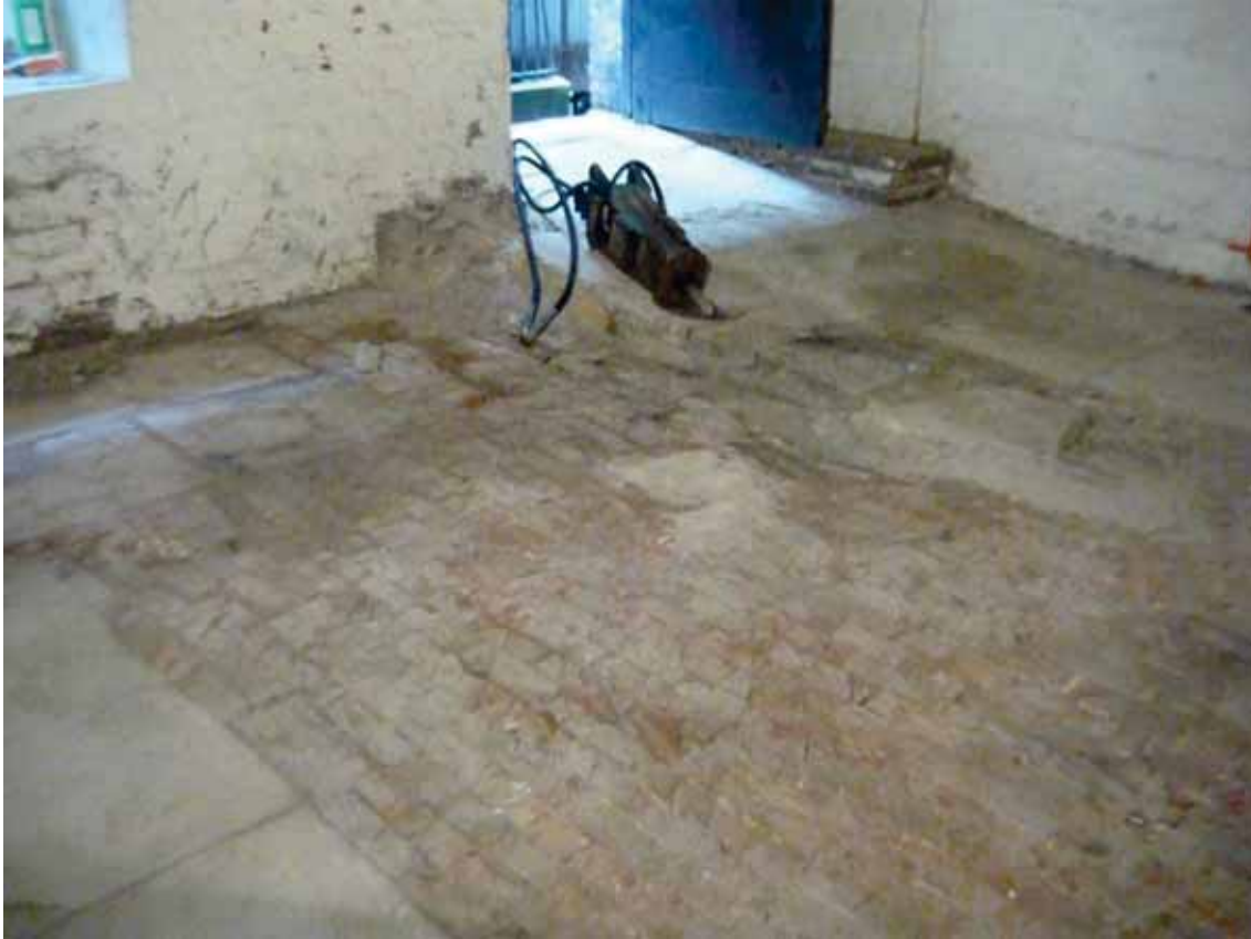
Plate 128: South-east corner of Room B50, looking south-east
