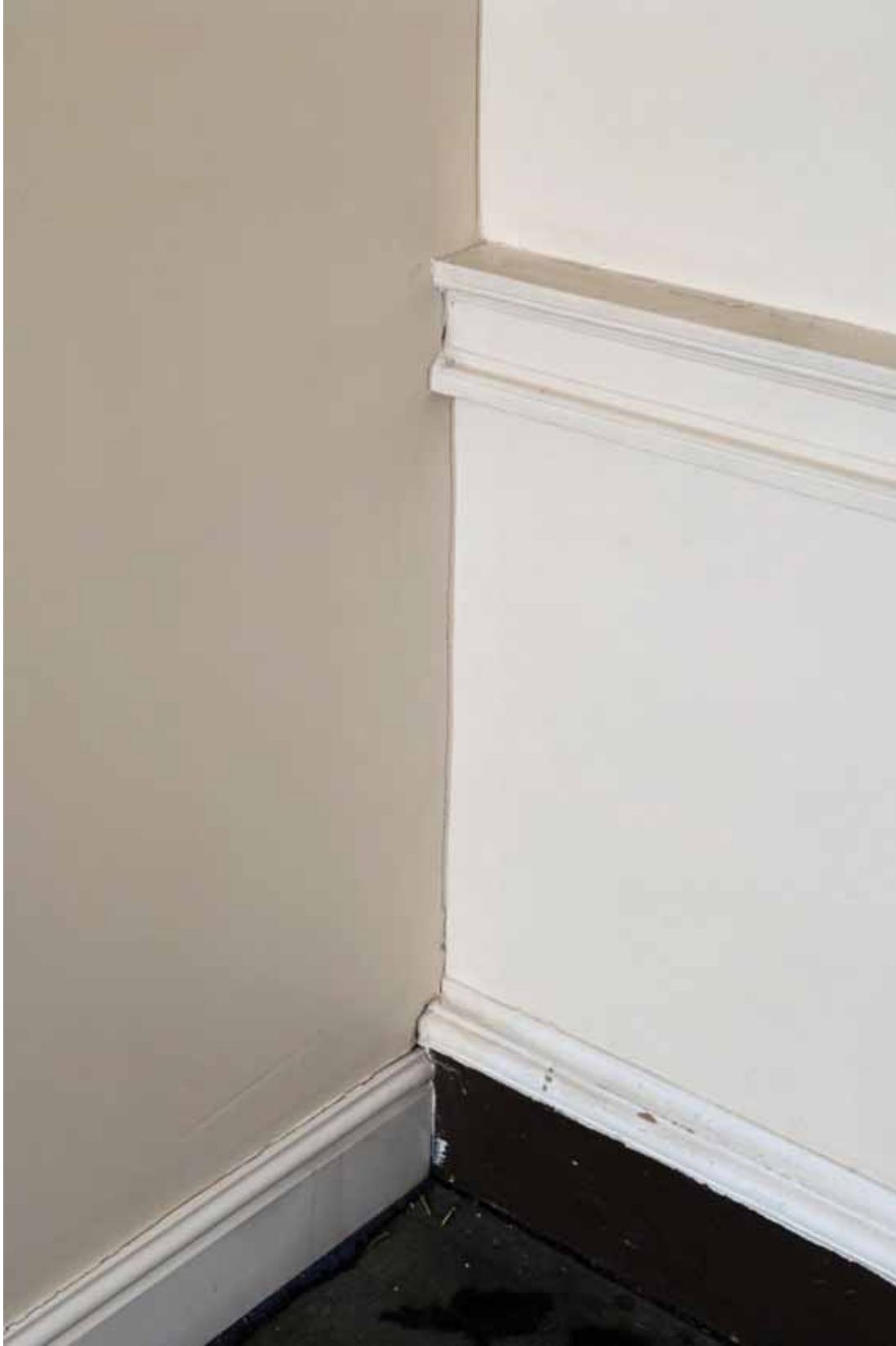
Plate 416: South wall of partition (left) and west wall (right) in Room G18, looking south-west (EAF10 B100 0885)
