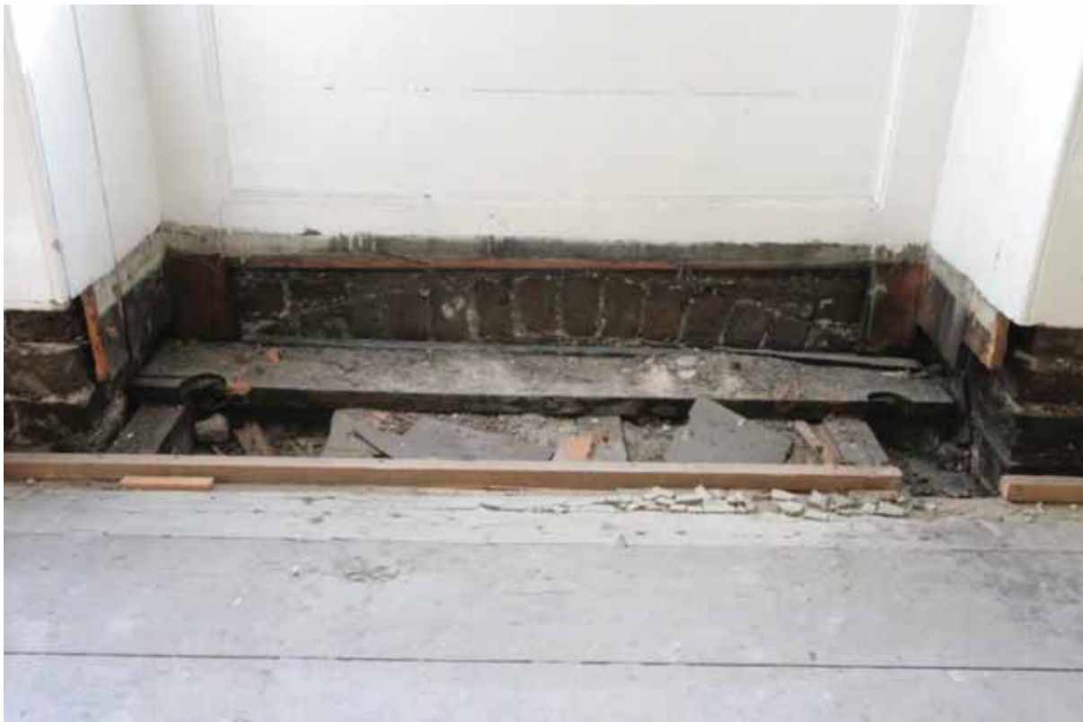
Plate 266: Brick segmental arch revealed following removal of skirting board from below the north window in the east wall, looking east (EAF10 284)
