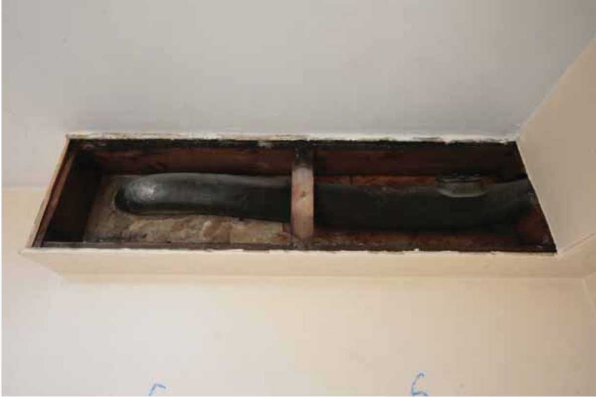
Plate 679: Lead pipe at the south end of Room T03, looking east (EAF10 202)
