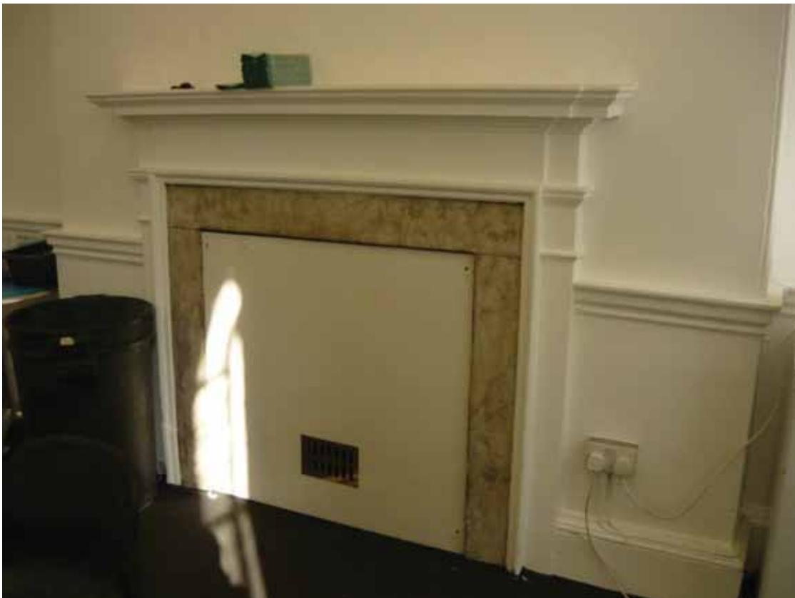
Plate 439: Fireplace (type 6) in the north wall of Room G24, looking north-west (EAF10 BHD1 (43))
