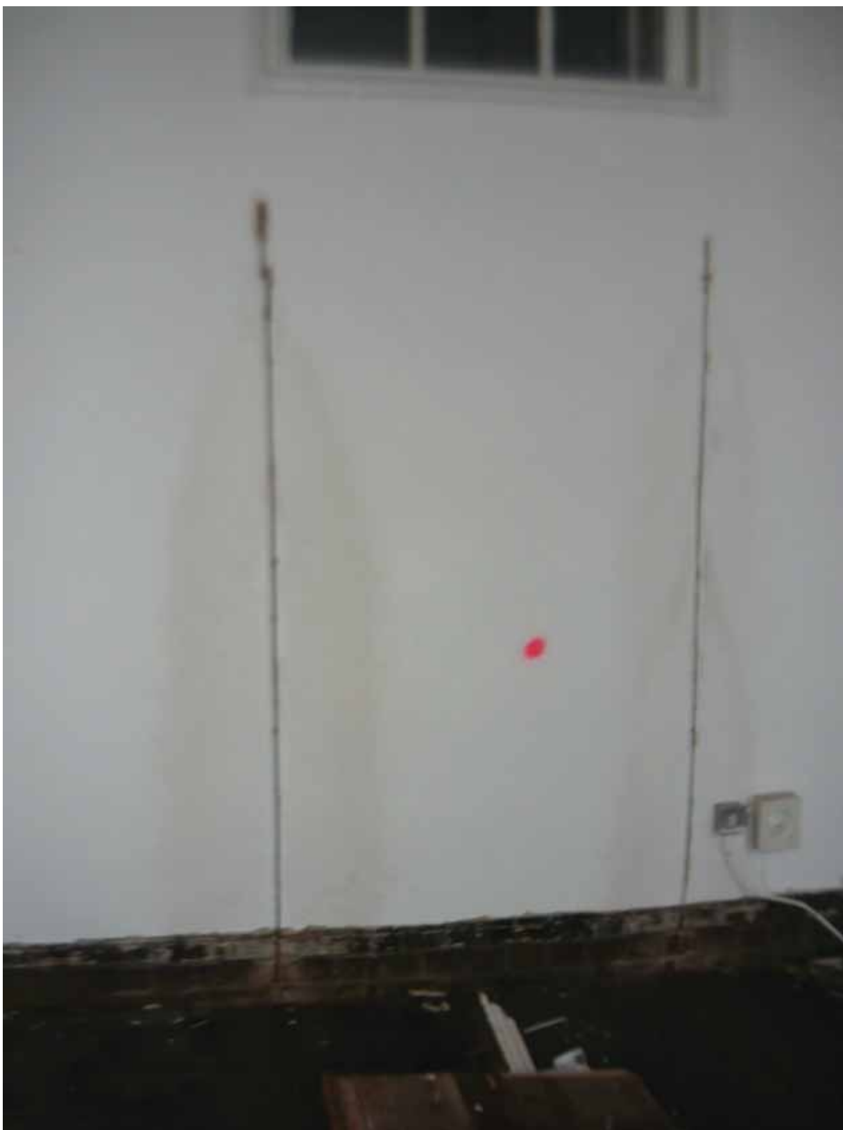
Plate 367: South end of the east wall in Room G08 marked up for a new doorway in 2010, looking east (EAF10 BHD3 (26))
