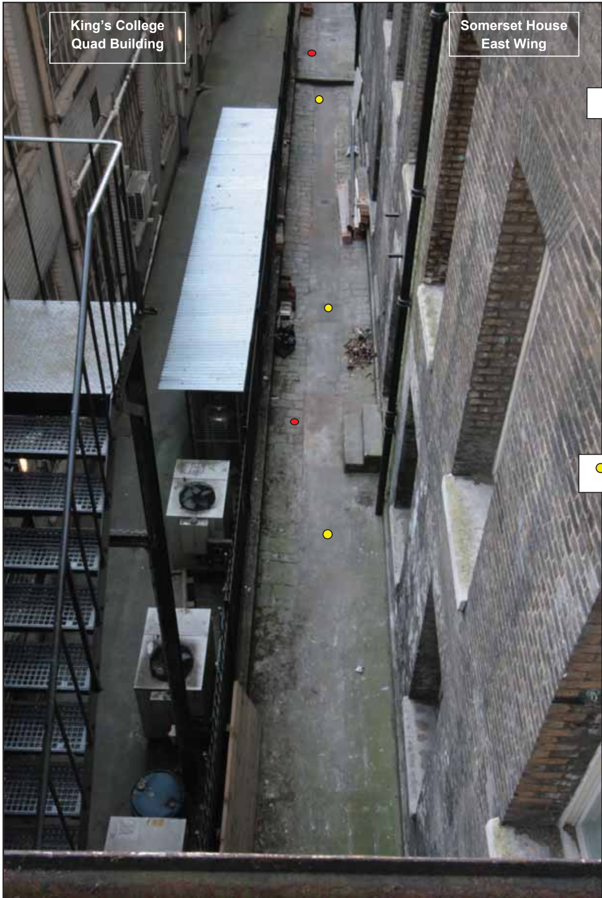
Plate 5: East lightwell with Somerset House East Wing (right) and King's College Quad Building (left), viewed from the north
