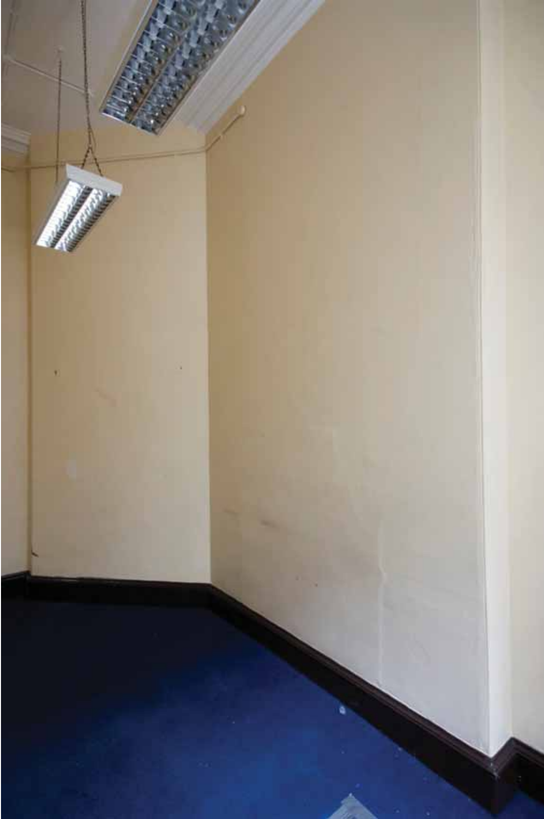
Plate 274: North wall of Room M32, looking north-west (EAF10 LG100 1083)
