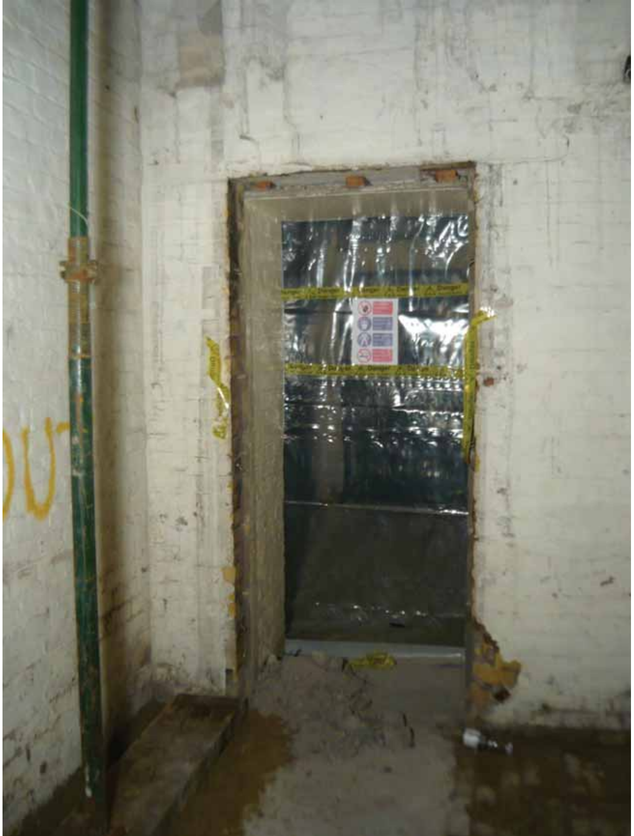
Plate 120: West doorway in Room B49A, looking west (EAF10 BHD5(124))
