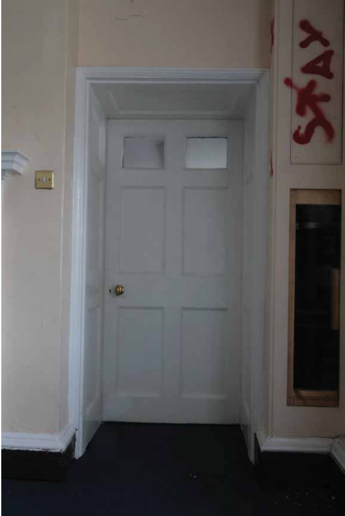
Plate 559: Doorway in the south wall of Room S95, looking south (EAF10 156)
