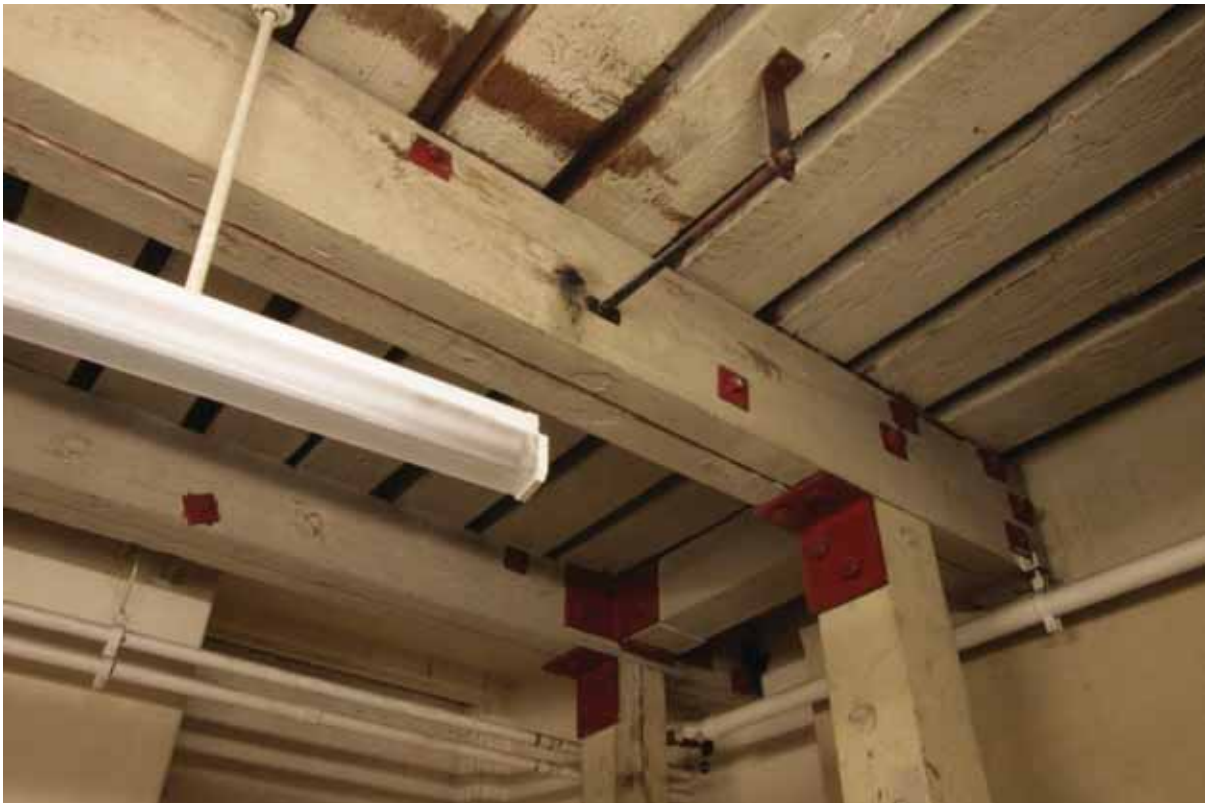
Plate 153: South-east corner of Room B53, looking south-east (EAF10 D100 017)
