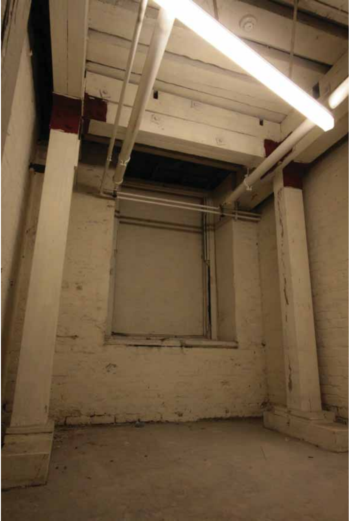
Plate 115: East wall of Room B49A, looking east (EAF10 D100 005)
