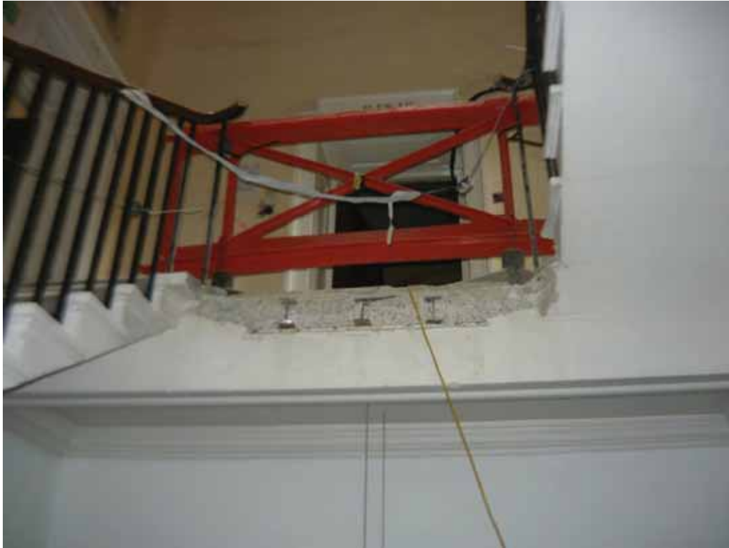
Plate 505: Removed link bridge in Stairs 02F looking south (EAF10 BHD3 (46))
