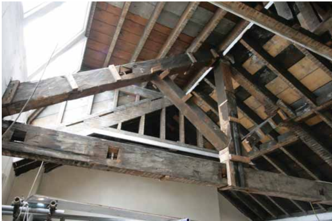
Plate 750: Tiebeam over Room T16, looking north (EAF10 A100 011)
