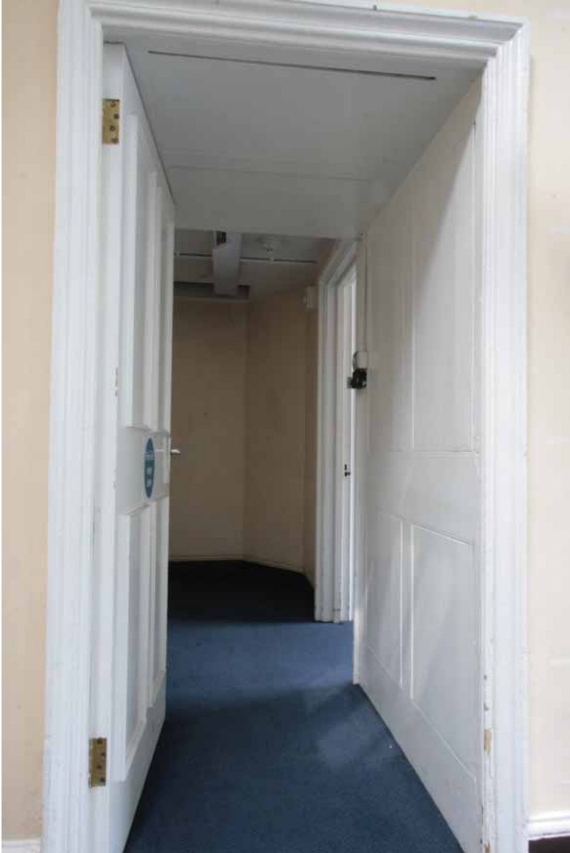
Plate 777: Doorway in the north wall of Room T25, looking north (EAF10 6)
