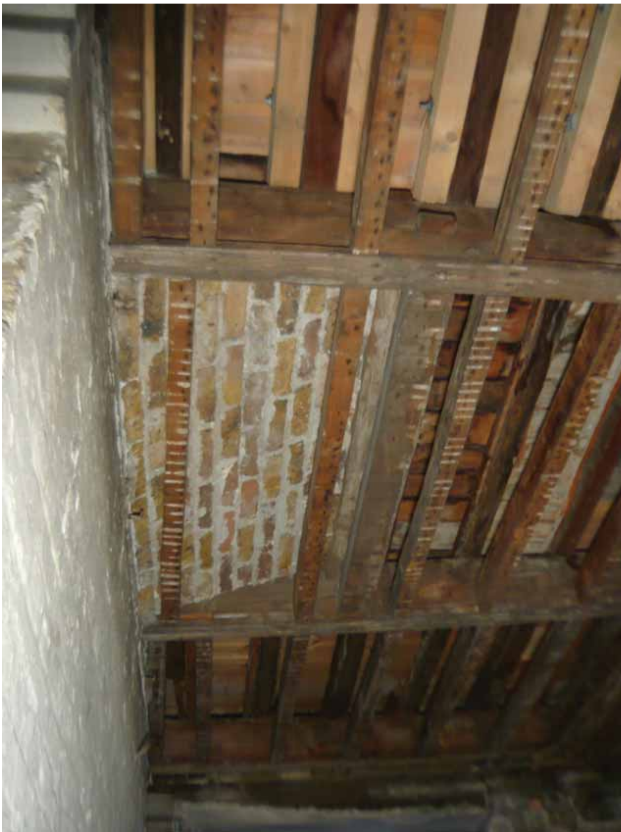
Plate 161: North wall and ceiling of Room B54A, looking east (EAF10 BHD5 (183))
