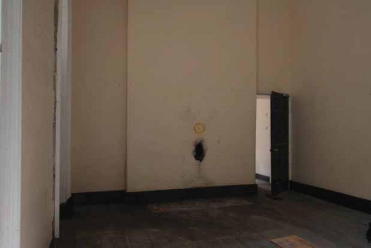
Plate 185: North wall of Room M10, looking north (EAF10 308)
