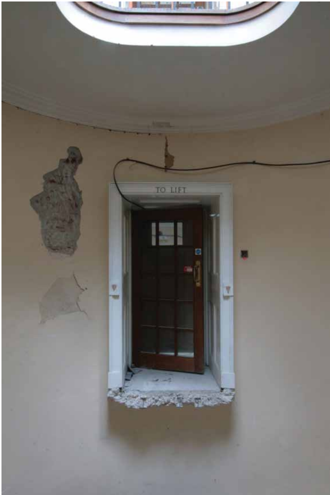
Plate 603: Ceiling in Stairs 02S looking north (EAF10 235)
