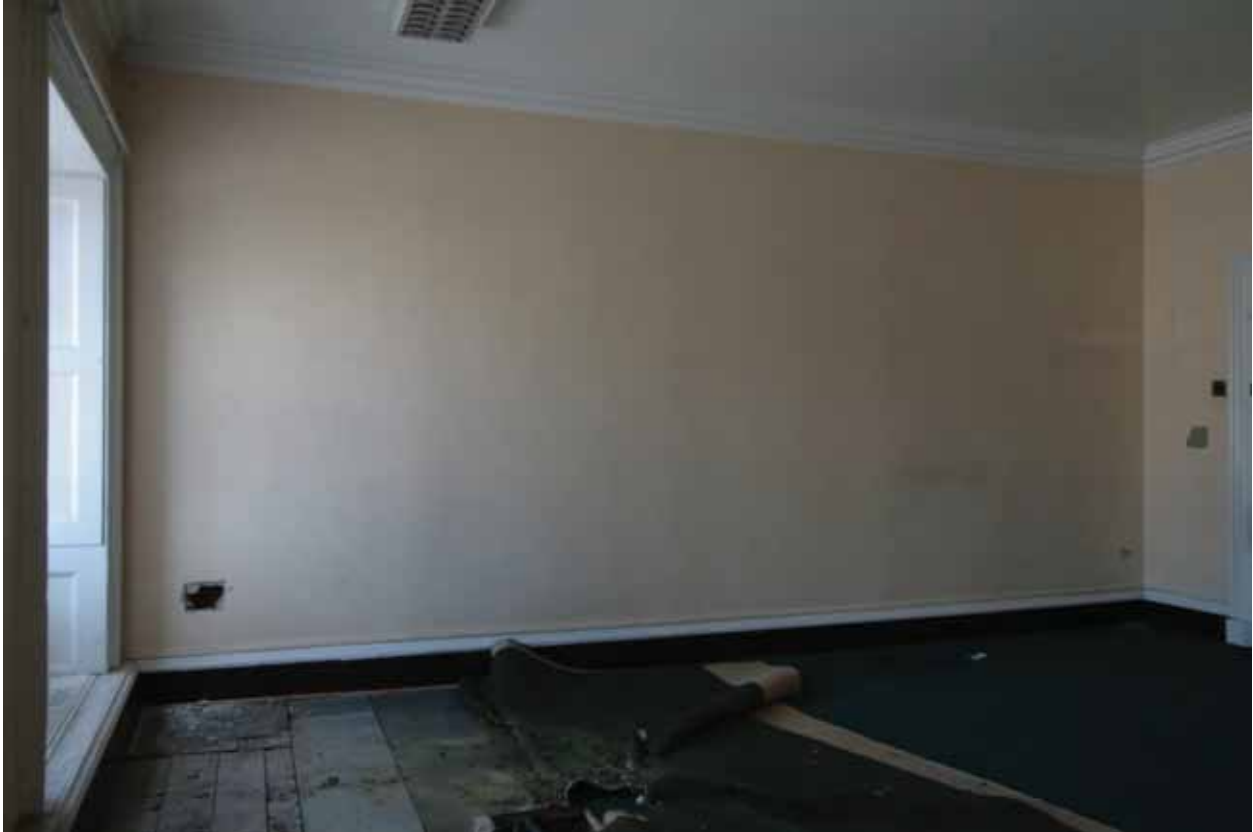
Plate 569: North partition wall in Room S08, looking north (EAF10 0115)
