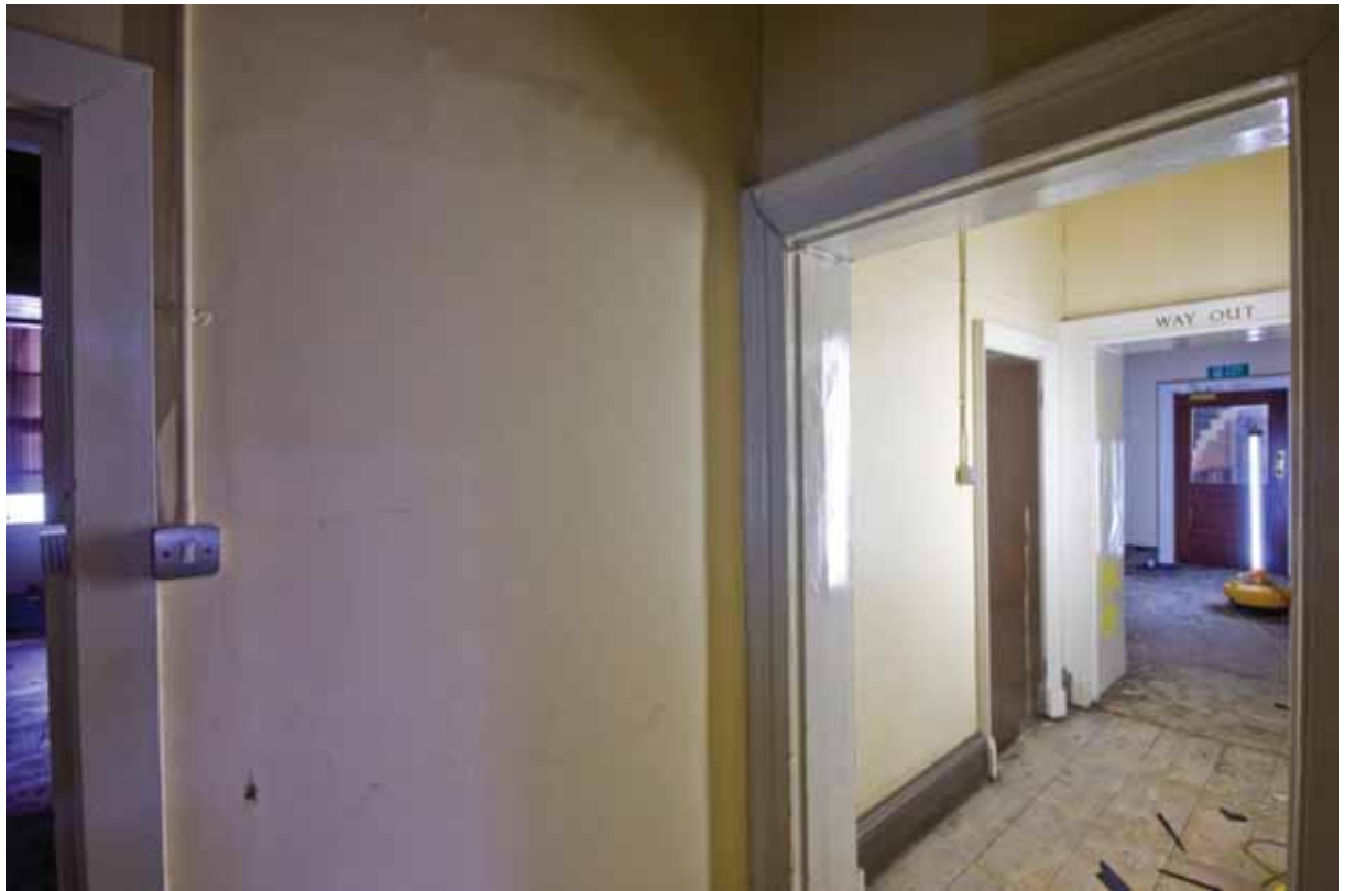
Plate 298: West partition wall in Room M26/M27, looking north-west (EAF10 LG100 1017)
