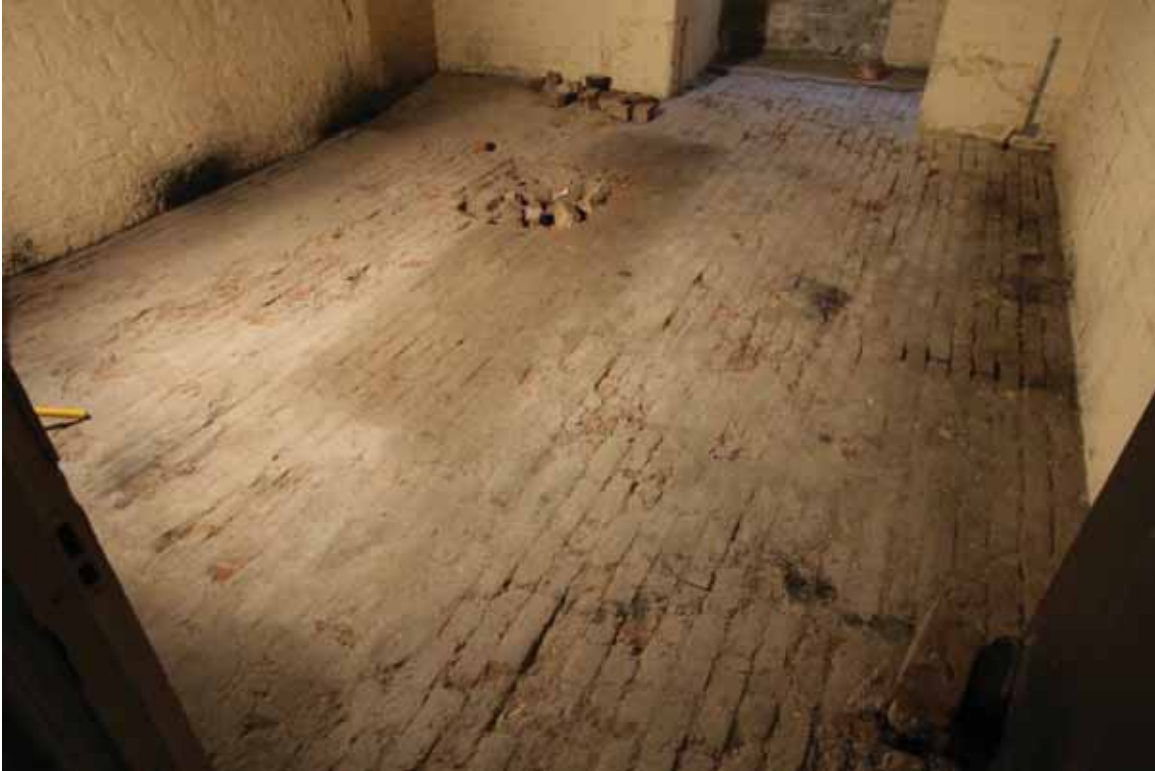
Plate 107c: Exposed brick floor in Room 62, looking south-west (EAF10 IMG_0006 (2))
