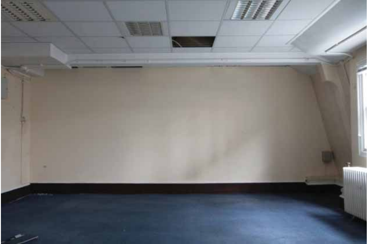
Plate 647: South partition wall in Room T120, looking south (EAF10 53)
