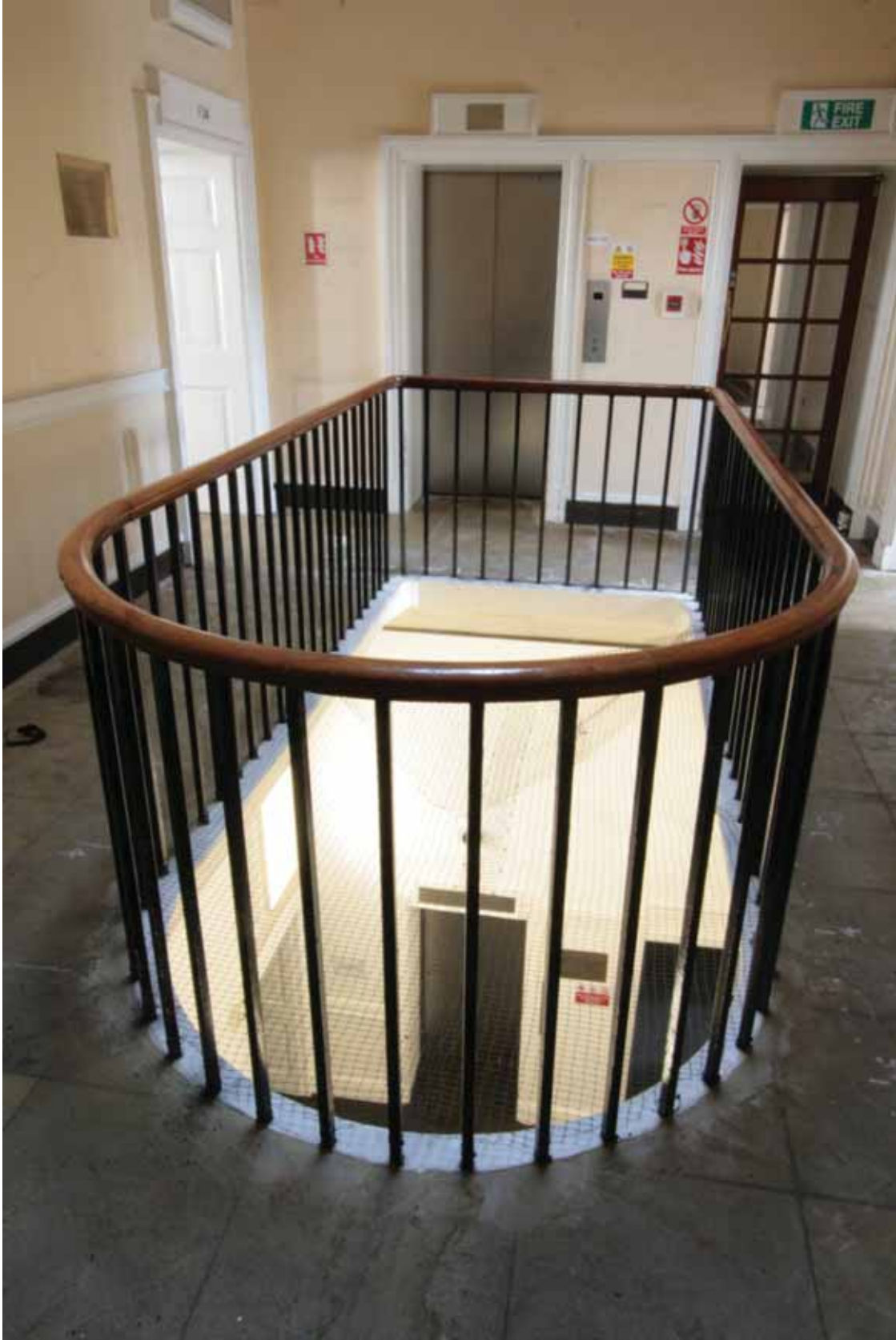
Plate 496: Lightwell in Corridor 03F looking south (EAF10 160)
