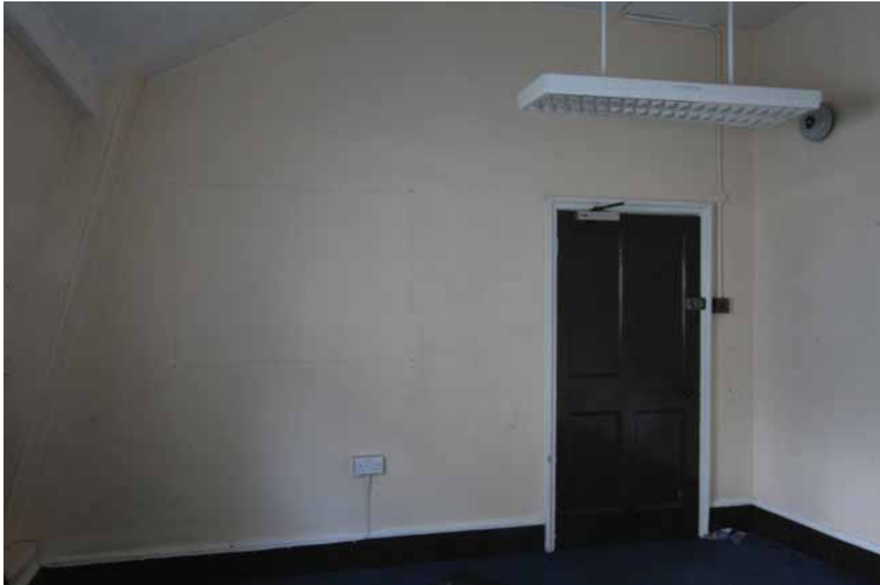
Plate 701: East wall of Room T14, looking east (EAF10 3)
