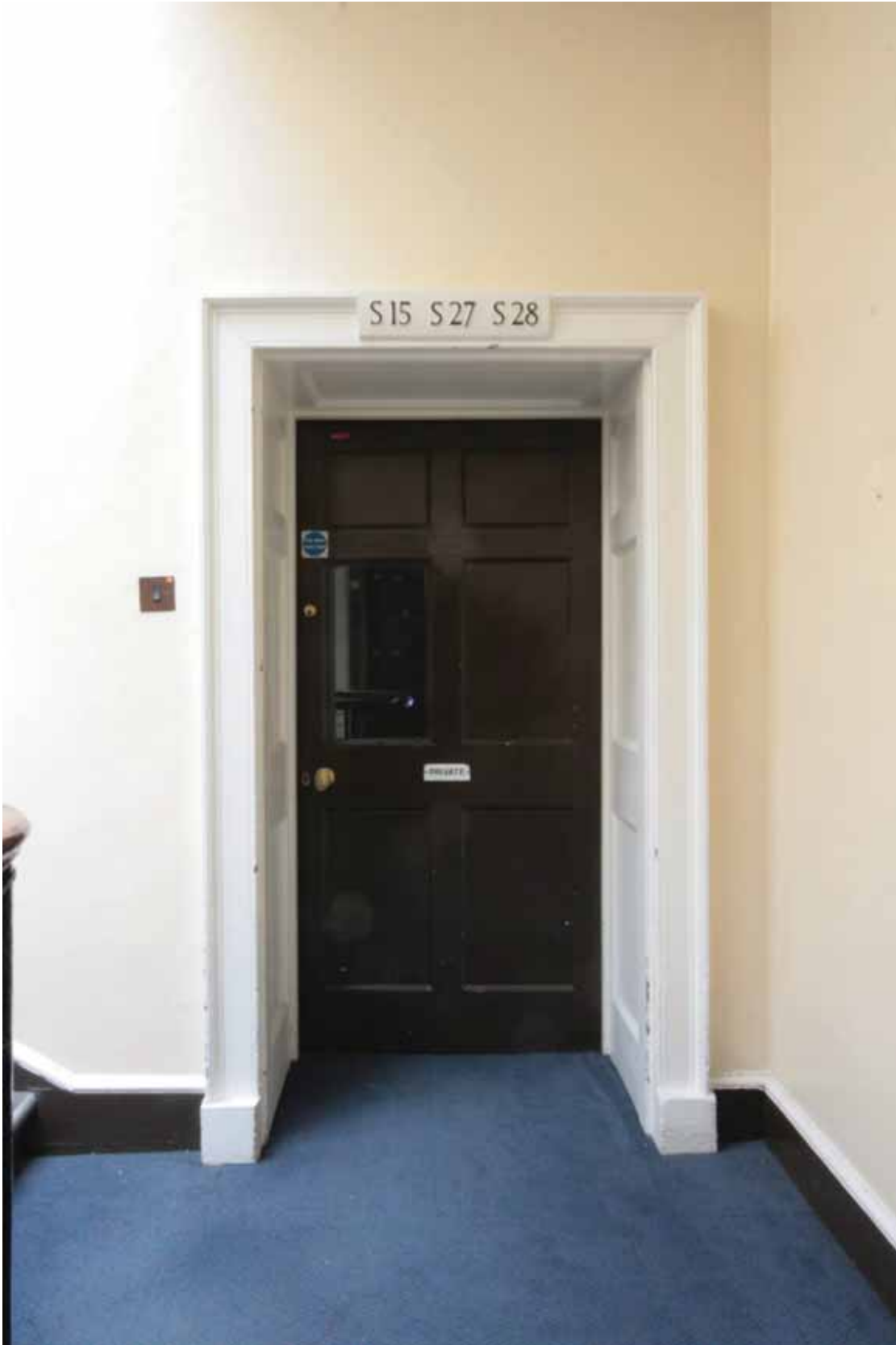
Plate 591: Doorway in the east wall of Stairs 01S, looking east (EAF10 00114)
