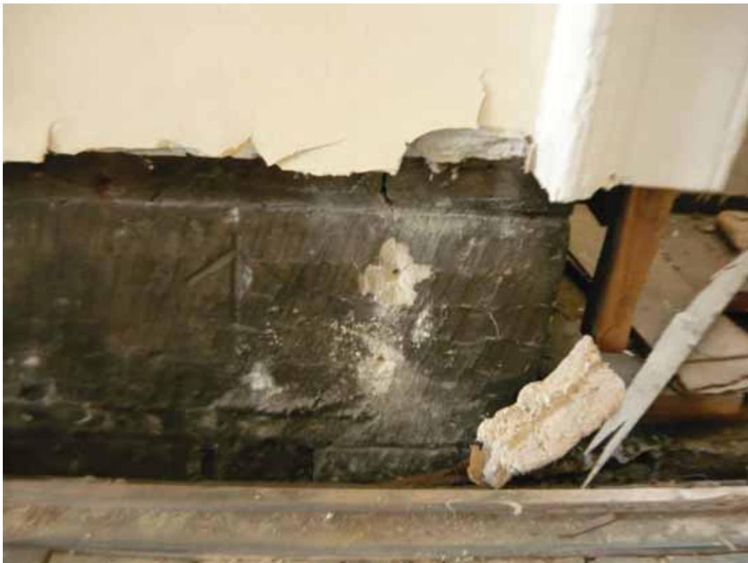
Plate 580: Ashlar block with carved arrow on west side of eastern window in north wall of Room S10, looking north (EAF10 BHD2 (55))
