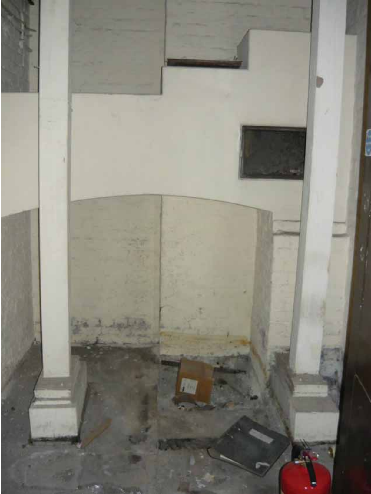
Plate 22: South wall of Room B45, looking south (EAF10 BHD1 (13))
