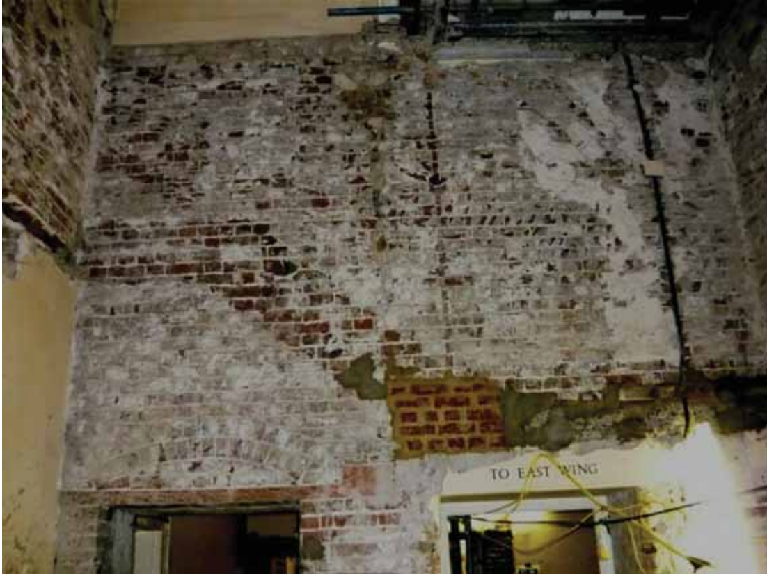
Plate 255: North wall of Corridor 06LG looking north (EAF10 BHD8 (103))
