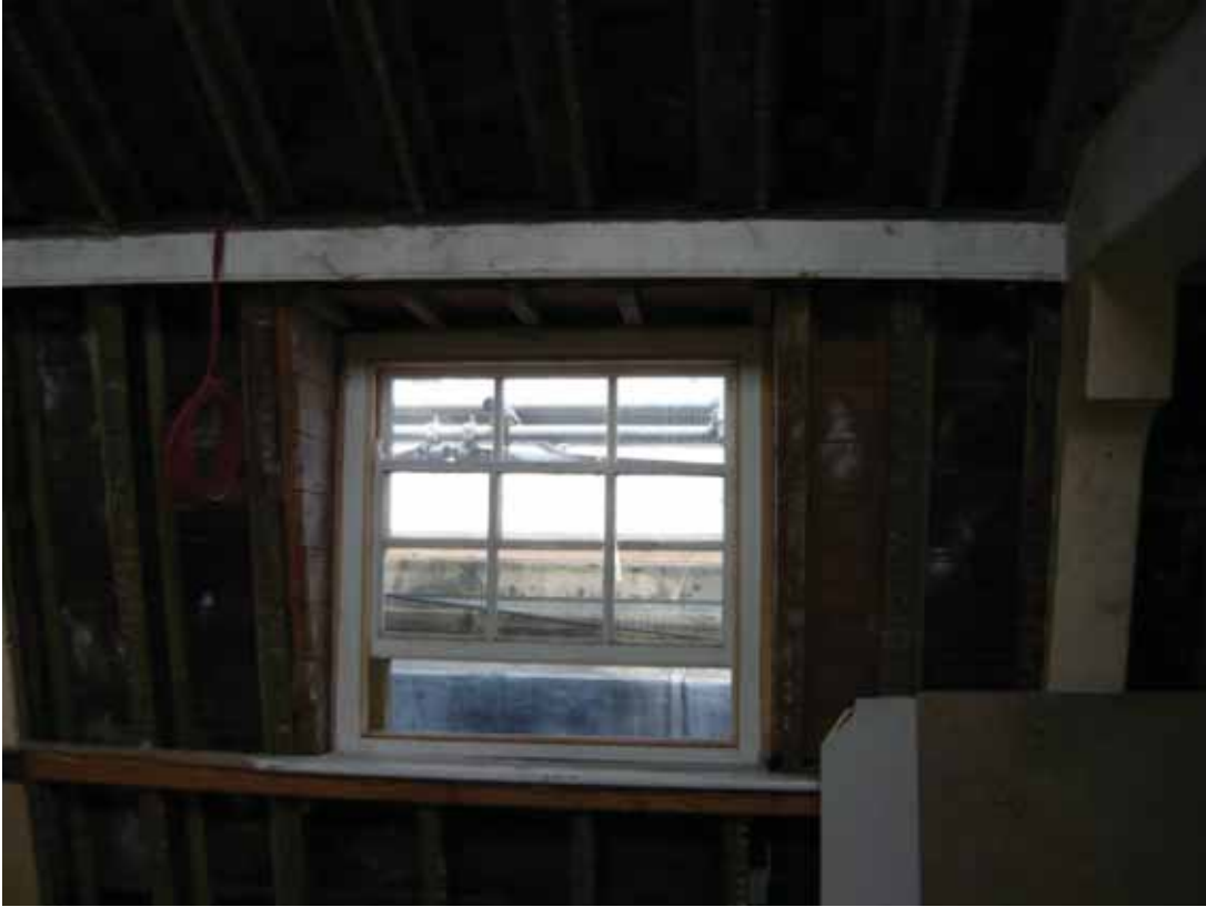
Plate 783: Northern window in the east wall of Room T25, looking east (EAF10 BHD10 (9))
