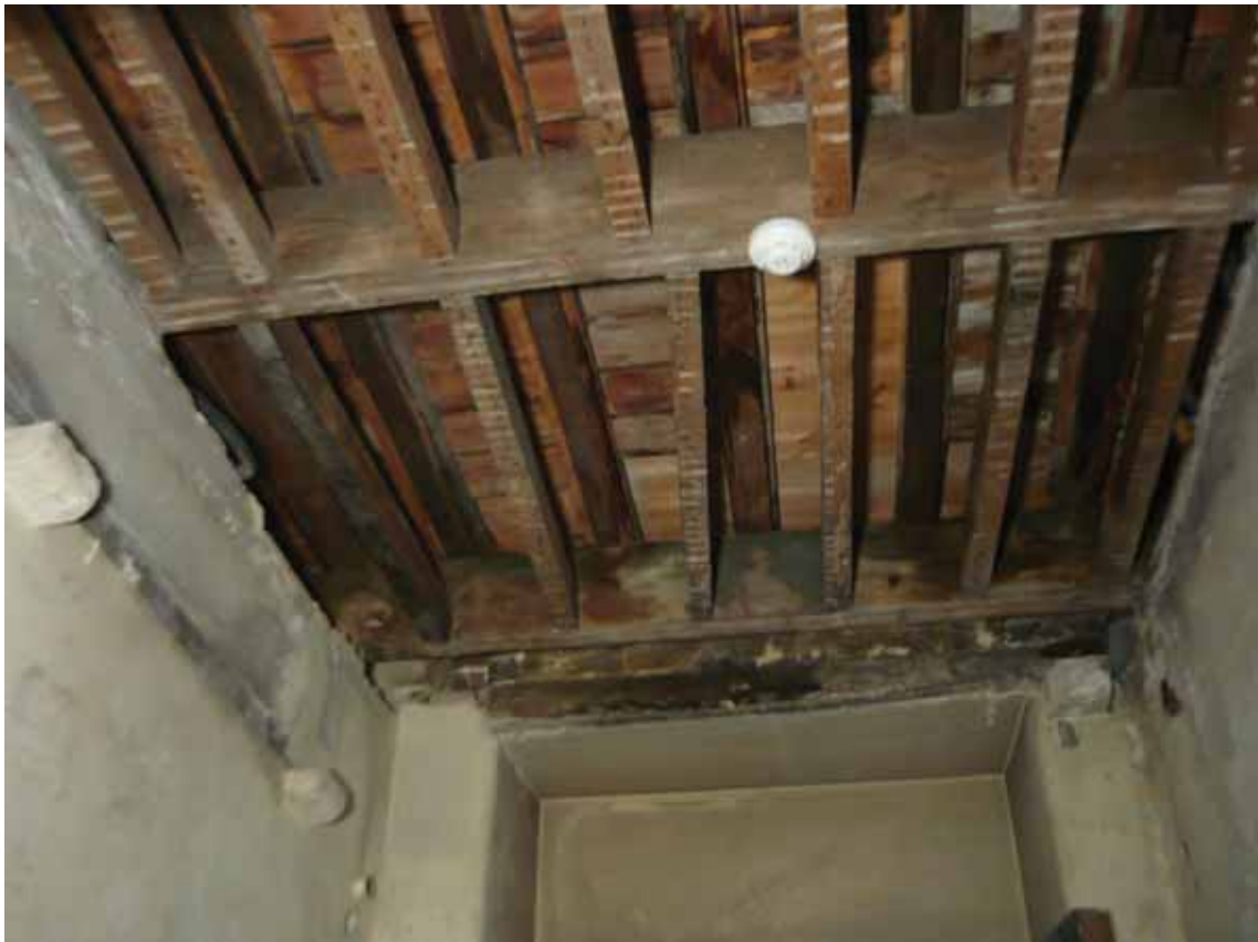
Plate 160: East wall and ceiling of Room B54B, looking east (EAF10 BHD5 (185))
