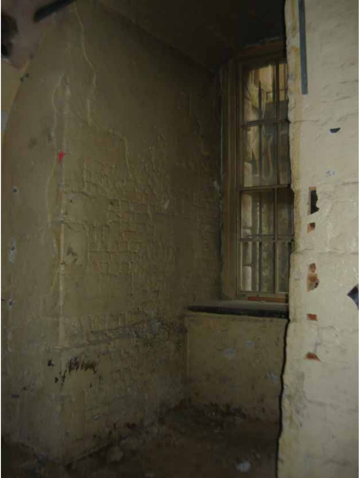
Plate 8: West wall of Room B42, looking south-west (EAF10 BHD5 (207))
