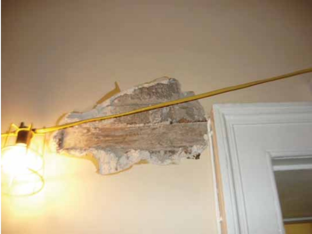
Plate 263: Timber lintel on the south side of the doorway in the west wall of Room M19, looking west (EAF10 BHD2 (106))
