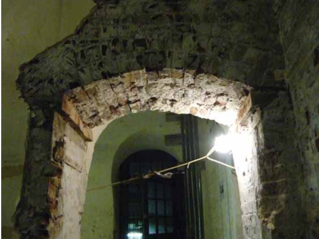
Plate 75: East doorway in Stairs 01, looking east into Room B50 (EAF10 BDH6(67))
