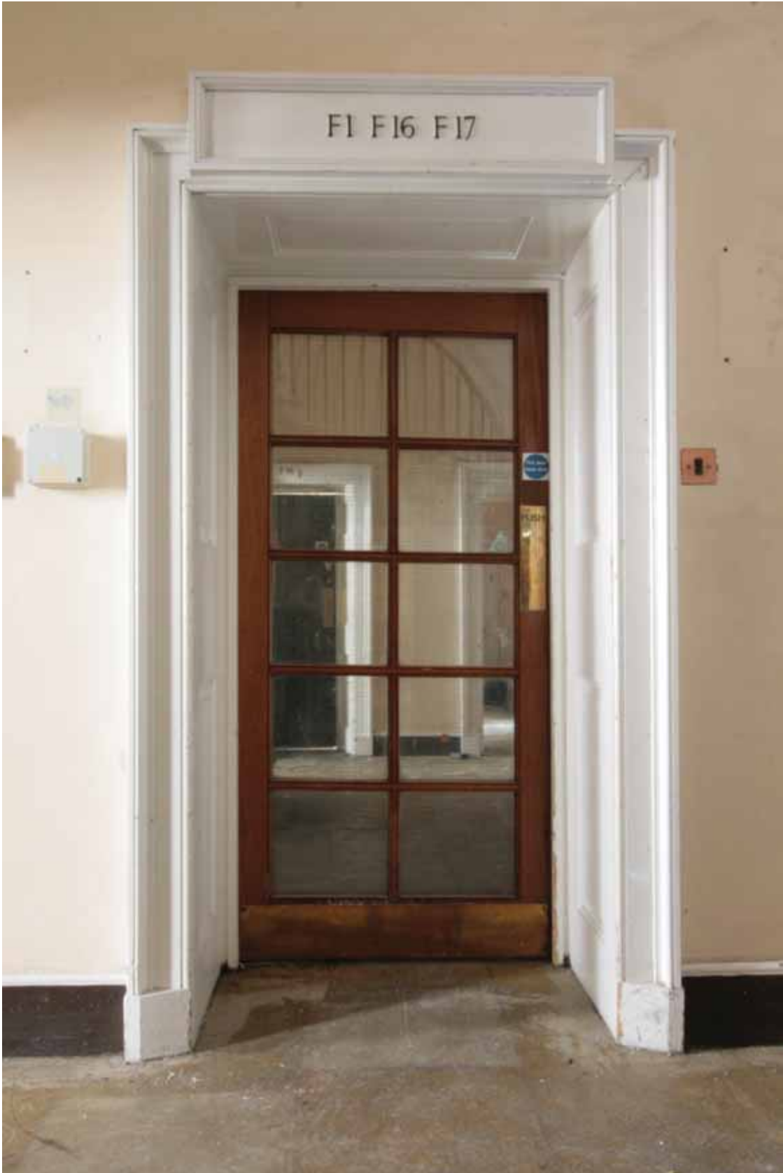
Plate 505: South doorway in Stairs 02F, looking south (EAF10 177)
