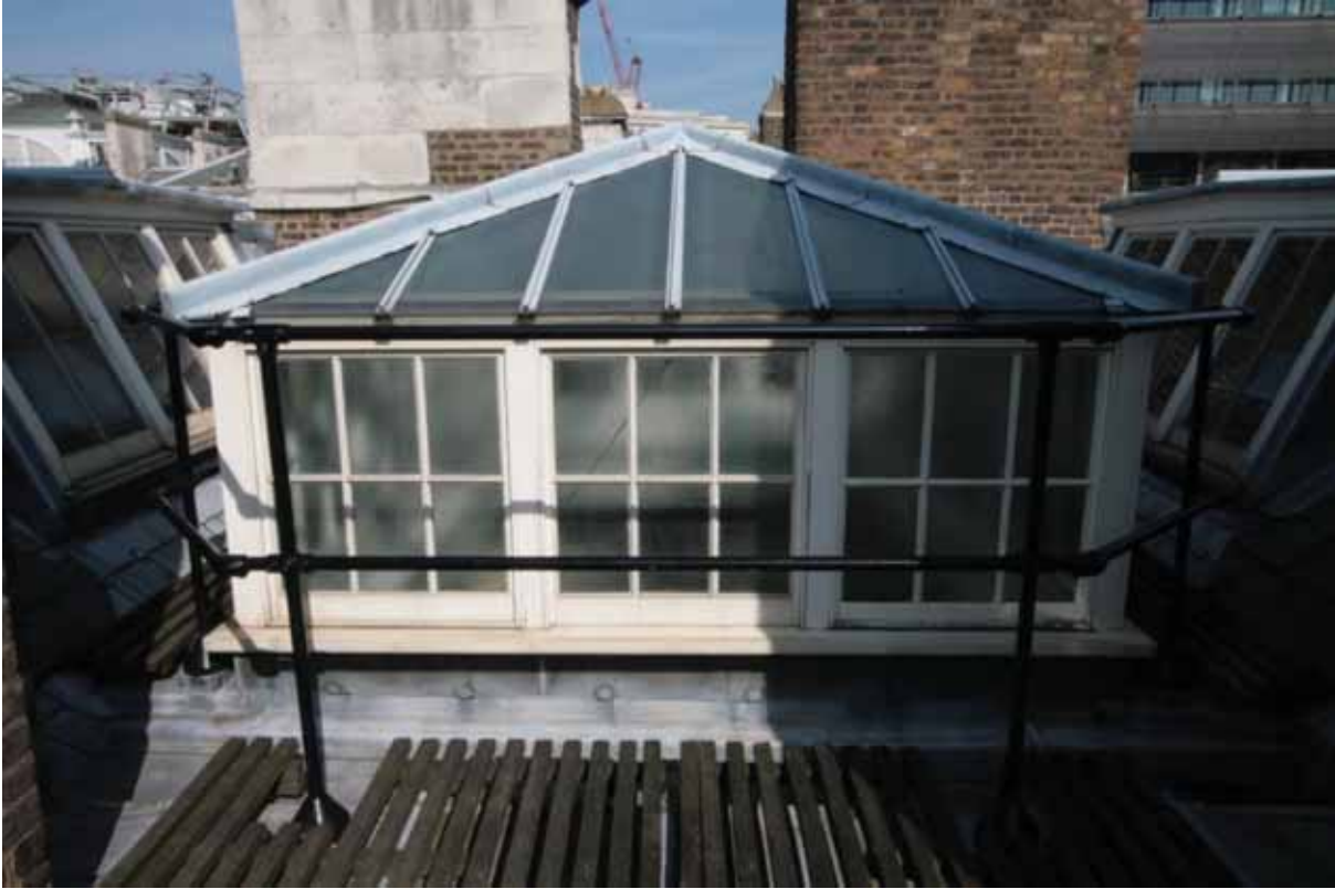
Plate 800: Lantern skylight over the Corridor 02T, looking north (EAF10 22)
