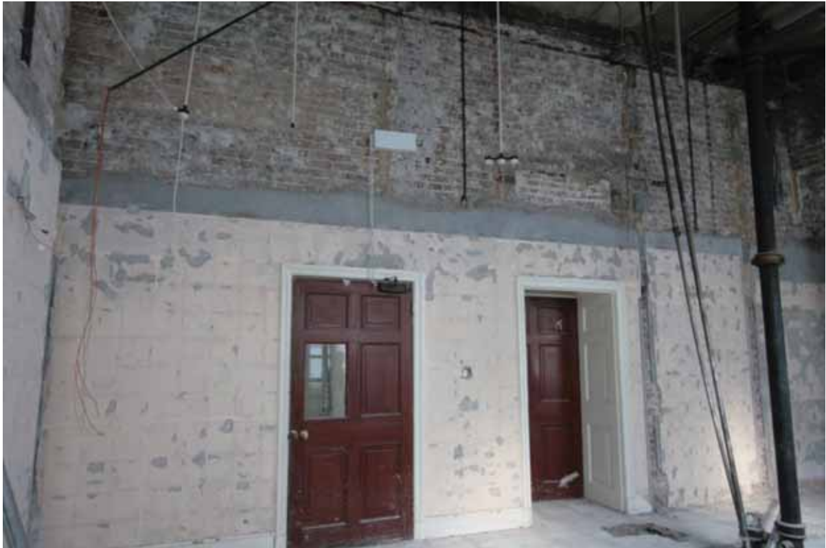
Plate 423: West wall in Room G20, looking west (EAF10 281)
