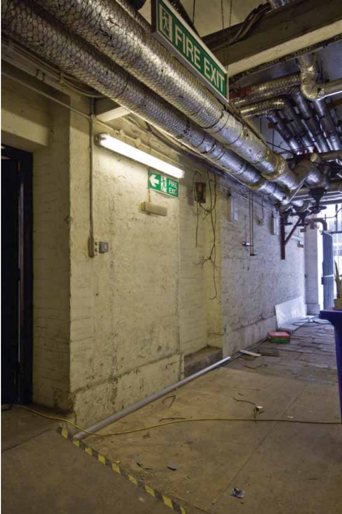
Plate 99: North wall of Corridor 5, looking north-east (DSC_1383_sitecode EAF10_© PCA Ltd 2010)
