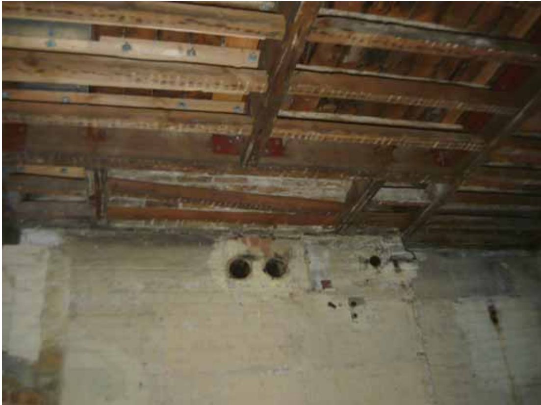
Plate 145: North wall in Room B51, looking north (EAF10 BHD5 (161))
