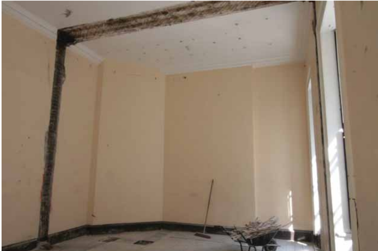
Plate 276: Scar of removed partition wall in Room M21/M32, looking north-west (EAF10 289)
