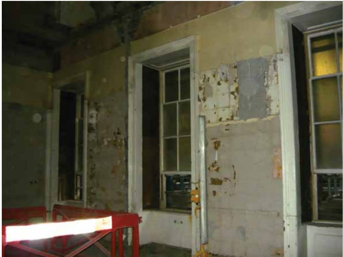
Plate 288: East wall in Room M116, looking east (EAF10 BHD8 (78))
