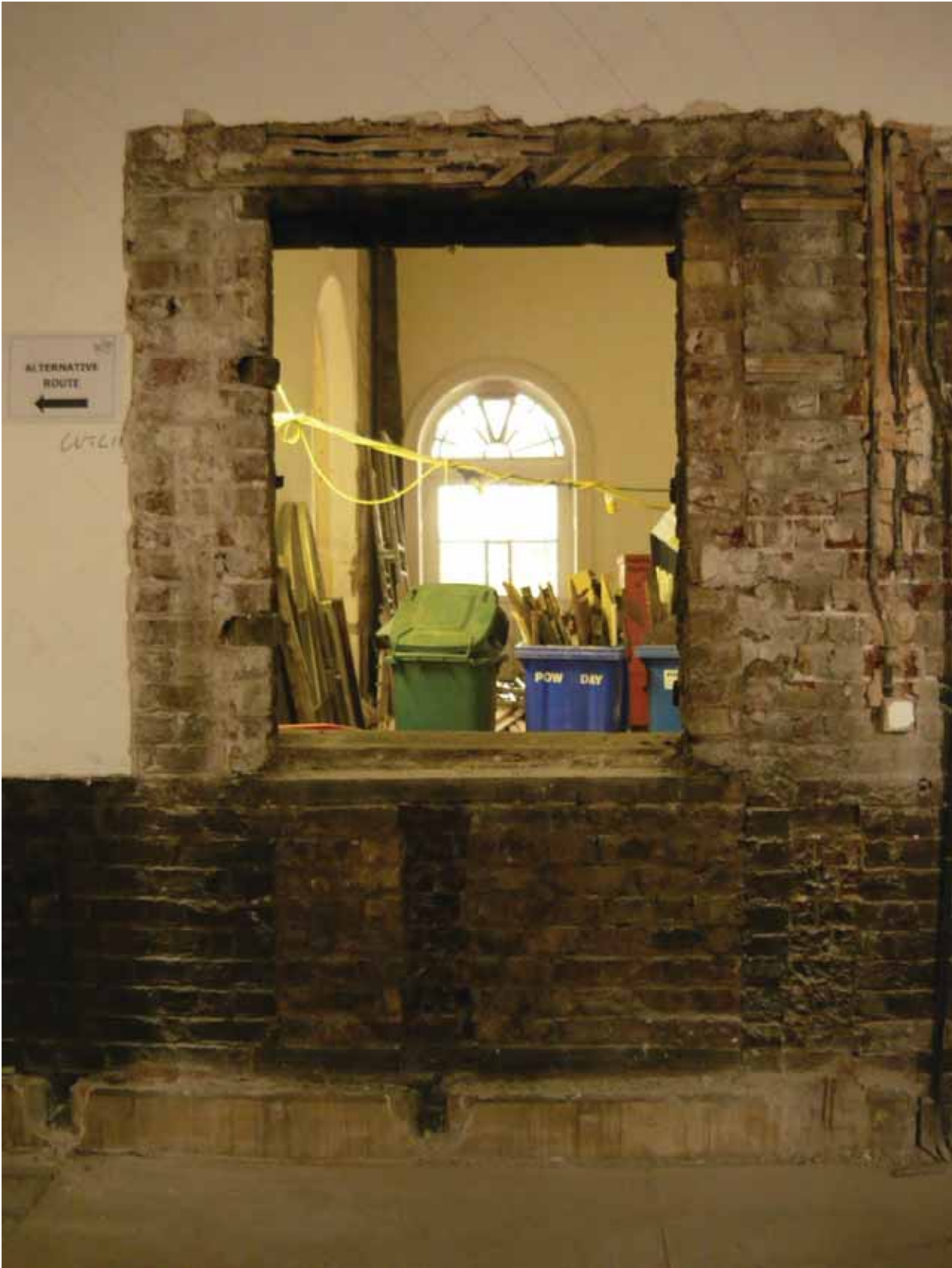
Plate 348: Internal window opening at the north end of the east wall in Room G01, looking east (EAF10 BHD8 (69))
