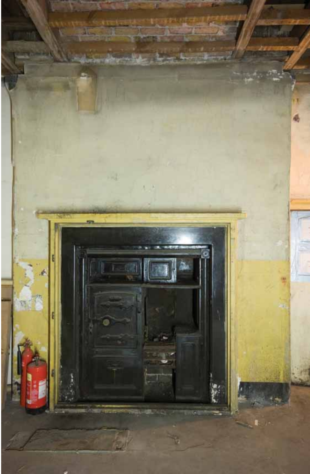
Plate 147: South wall in Room B52, looking west (EAF10 BHD5 (168))
