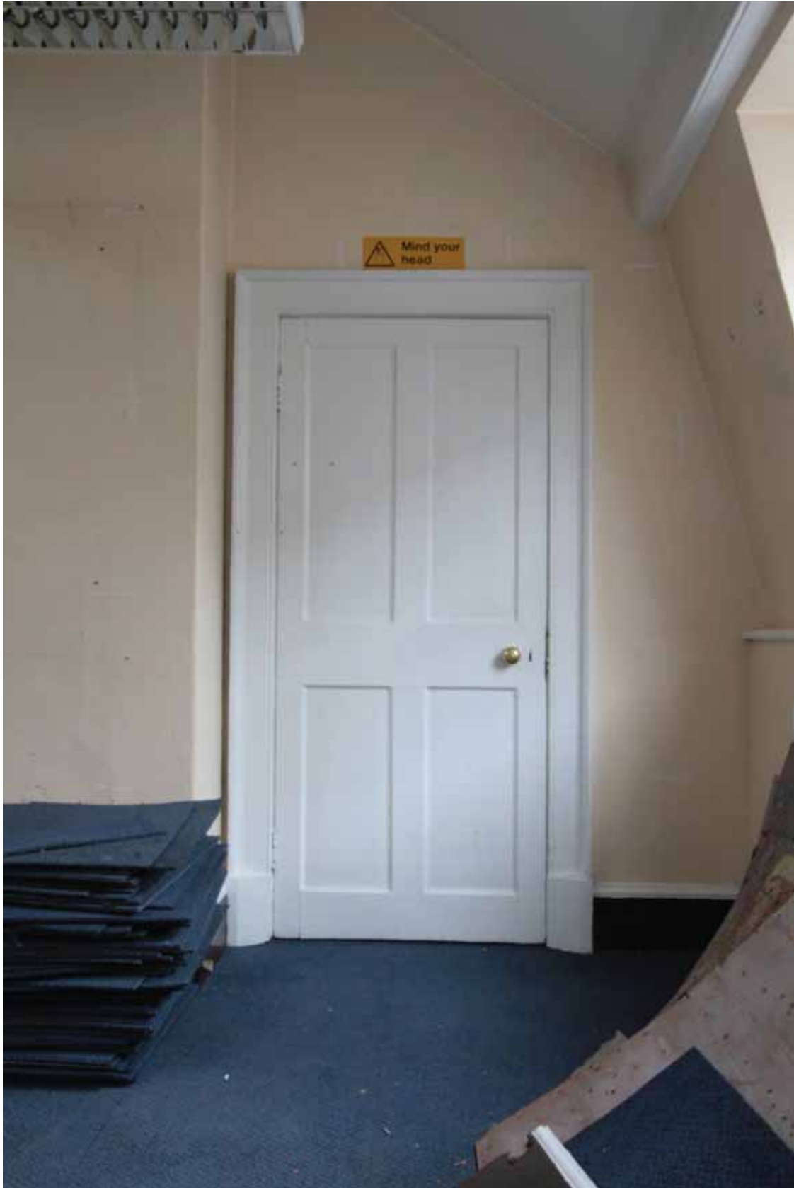
Plate 770: Doorway in the north wall of Room T24, looking north (EAF10 11)
