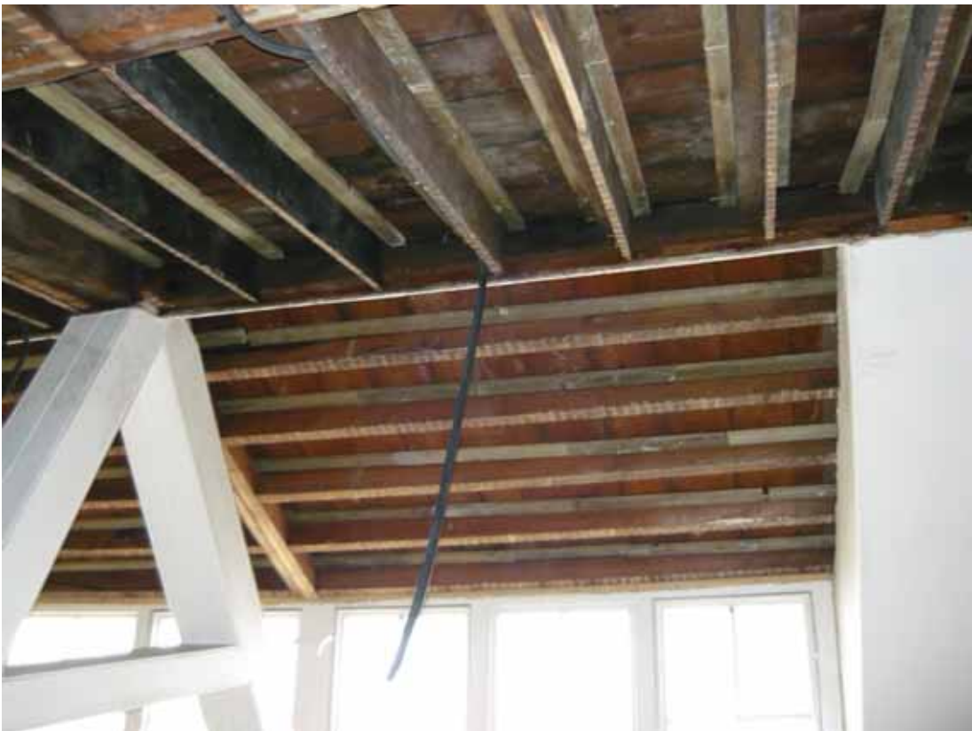
Plate 691: Dormer window above the east wall in Room T08, looking east (EAF10 BHD10 (73))
