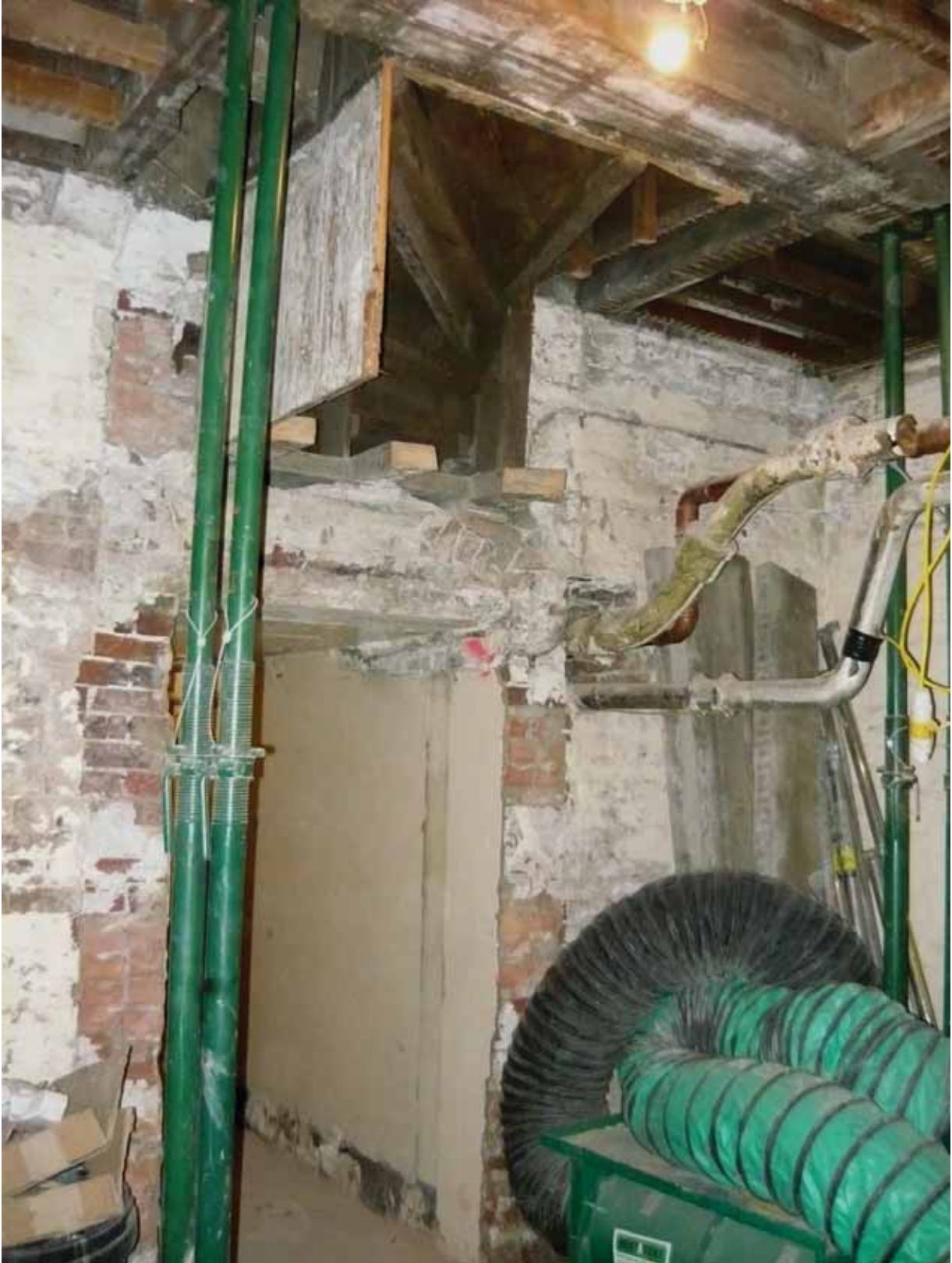
Plate 69: South doorway in Room B63 following removal of its concrete surround, looking south-west (EAF10 BHD6(37))
