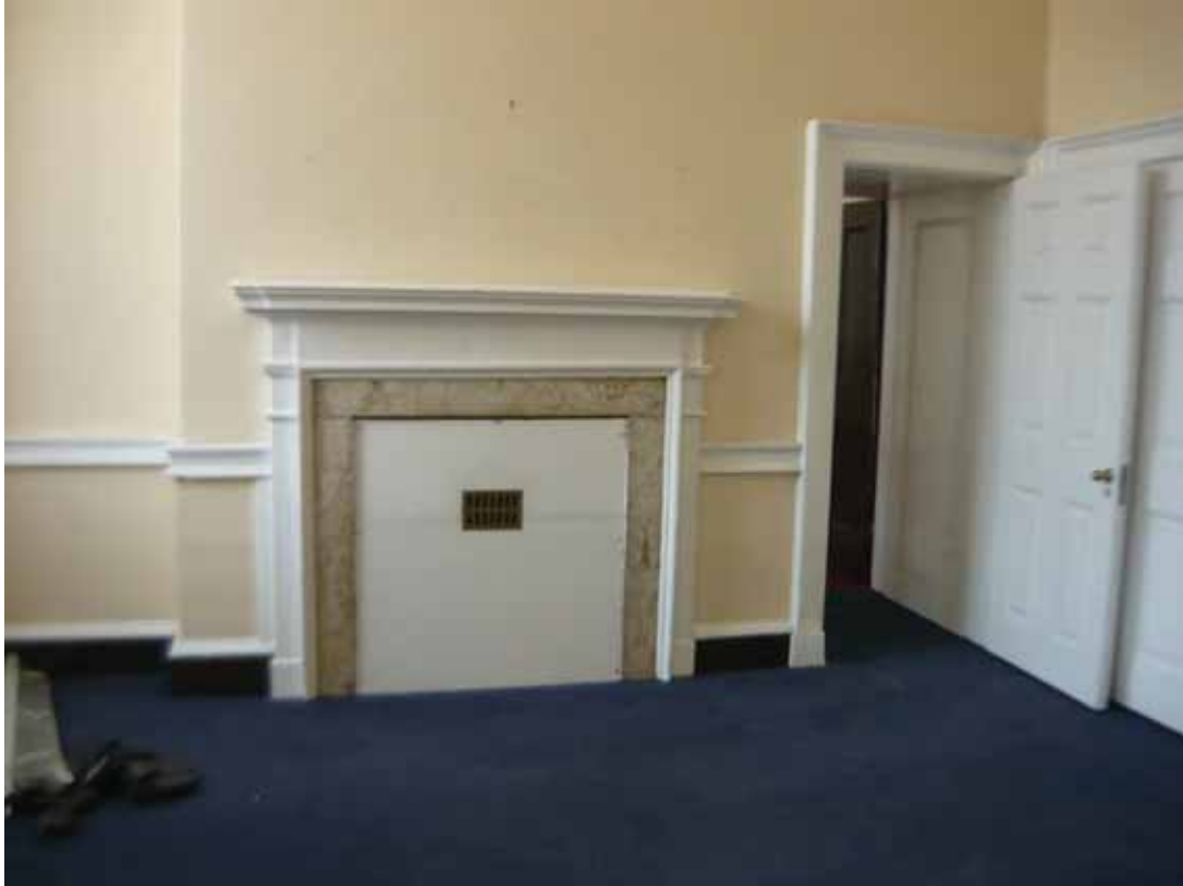
Plate 477: North wall of Room F05, looking north (EAF10 BHD1 (78))
