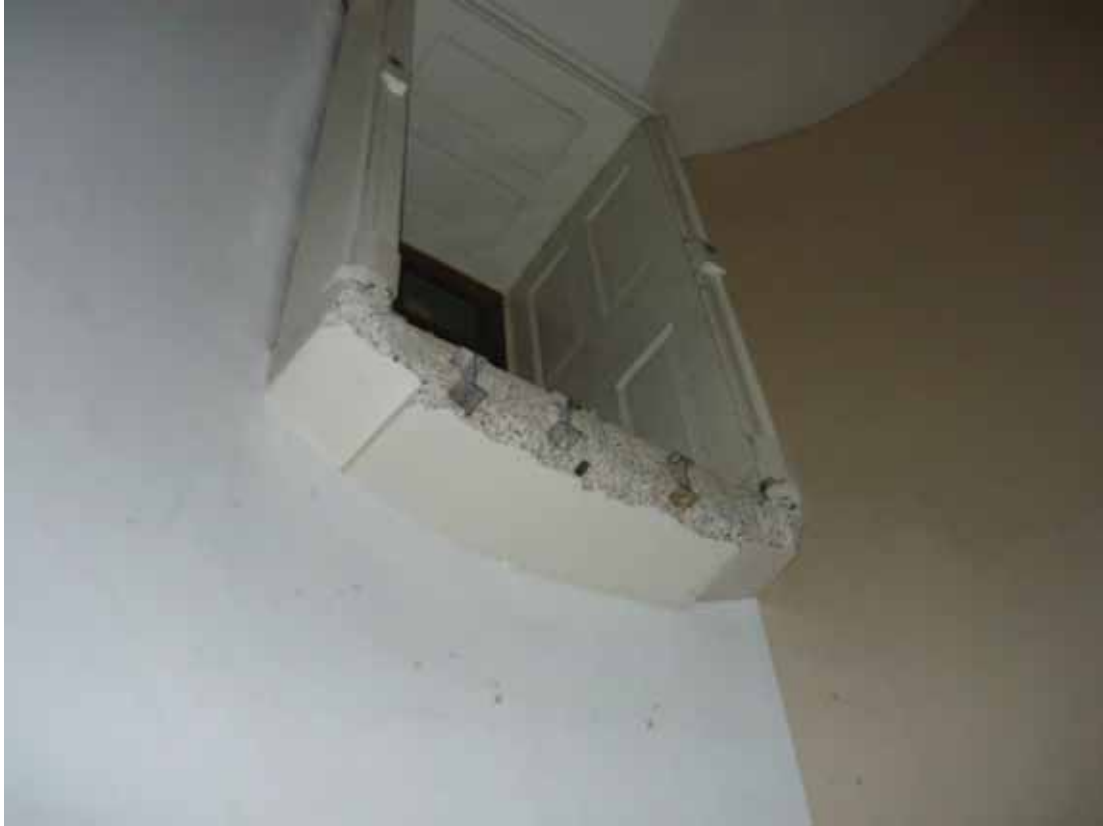
Plate 504: Removed link bridge in Stairs 02F looking north (EAF10 BHD3 (45))
