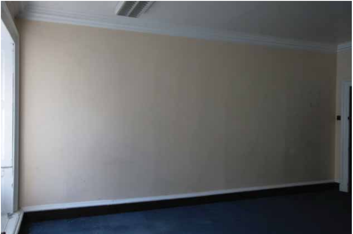
Plate 640: South partition wall in Room S26, looking south (EAF10 0116)
