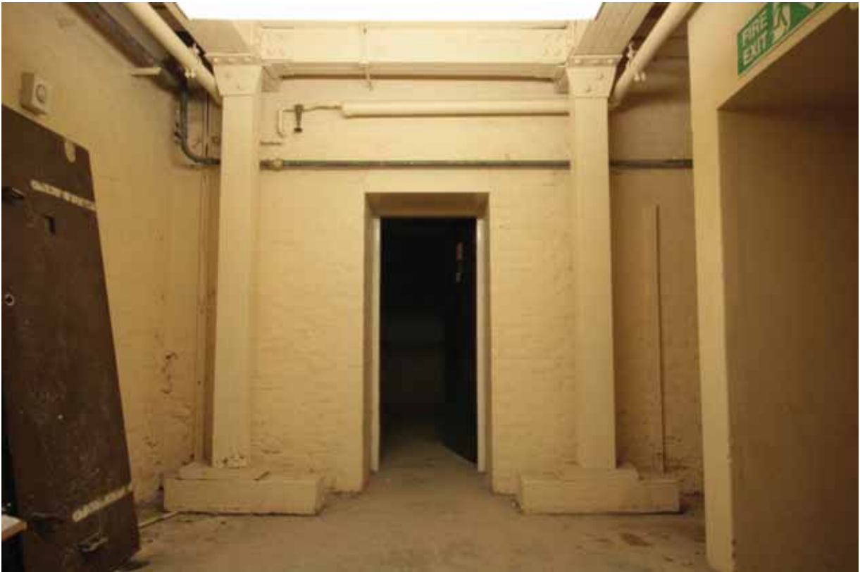
Plate 66: East doorway in Room B63, looking east (EAF10 D100 003)
