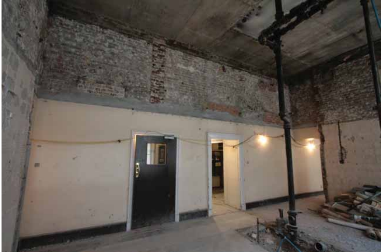
Plate 285: West wall in Room M116, looking west (EAF10 294)
