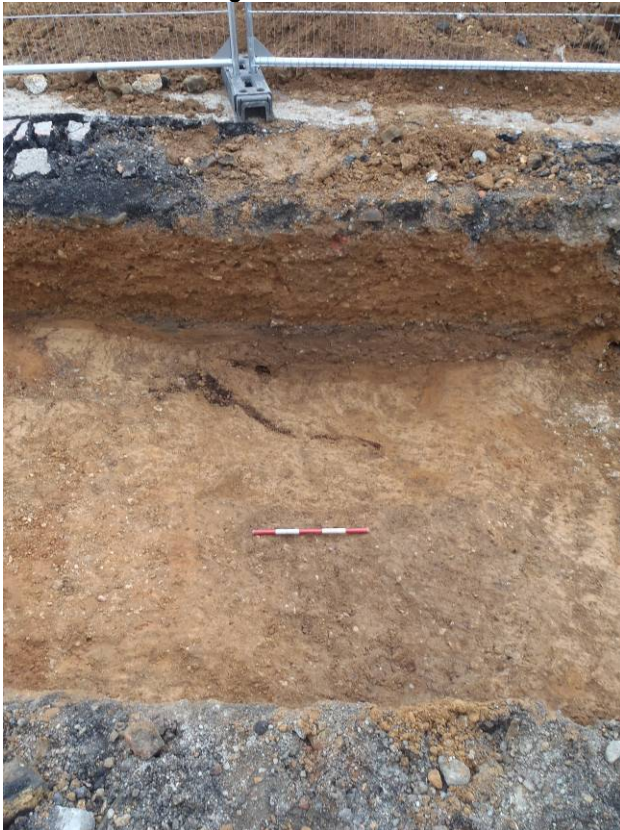
Plate 1: MH 1 facing north
