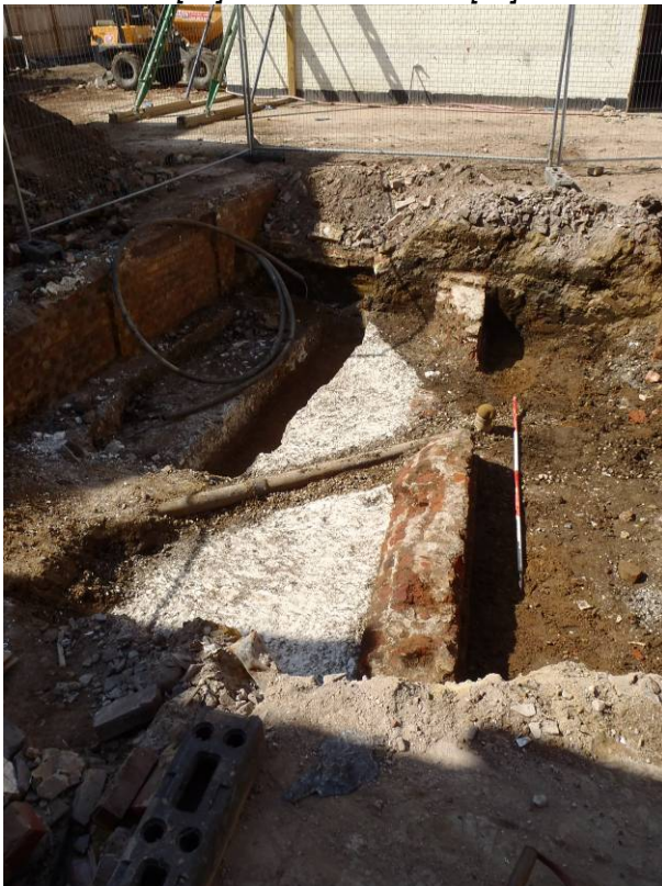
Plate 2: Wall [27] and chalk surface [25] in Trench 3/5, facing northwest
