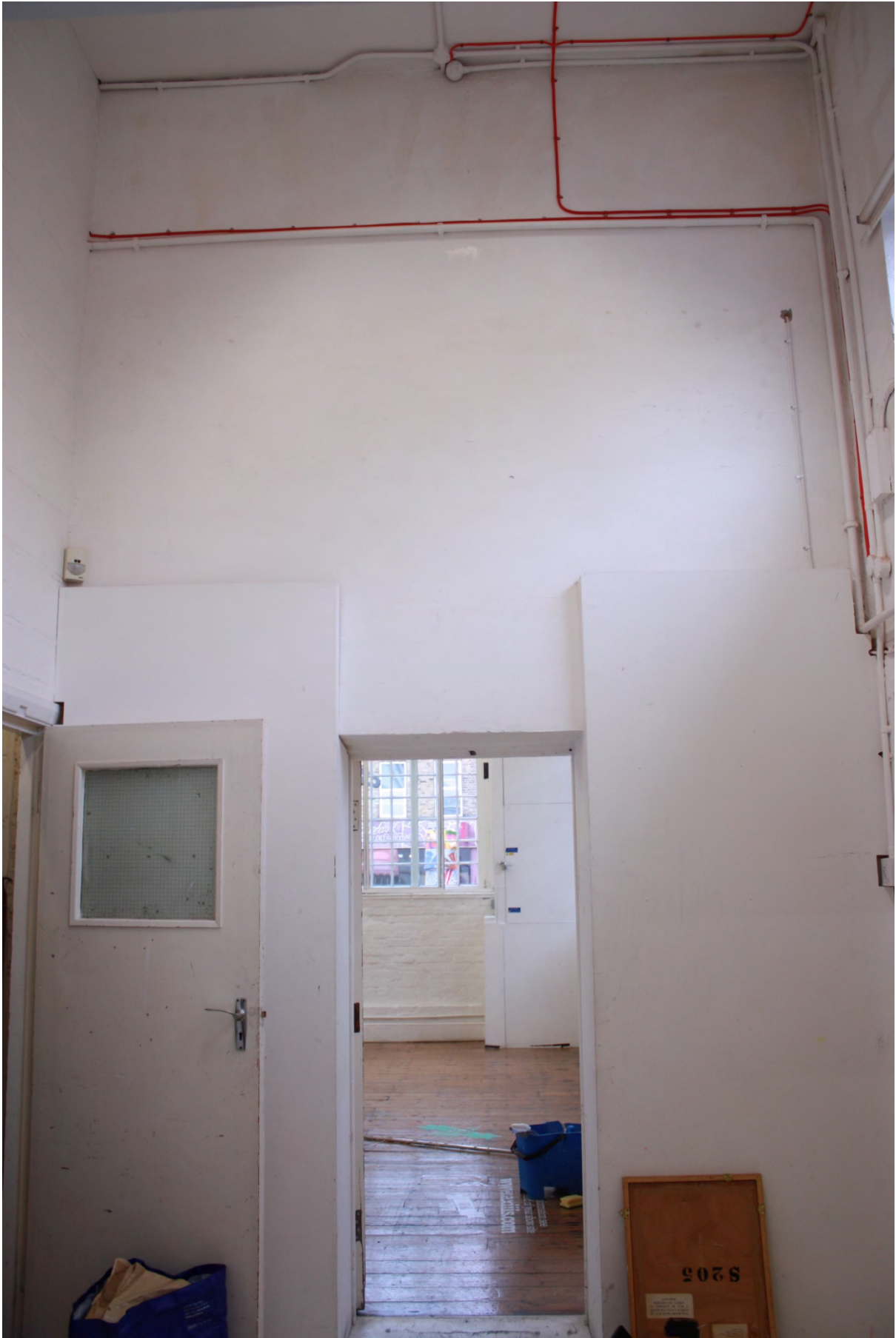
Plate 14d: East wall of Room 4, looking east (D3/6)
