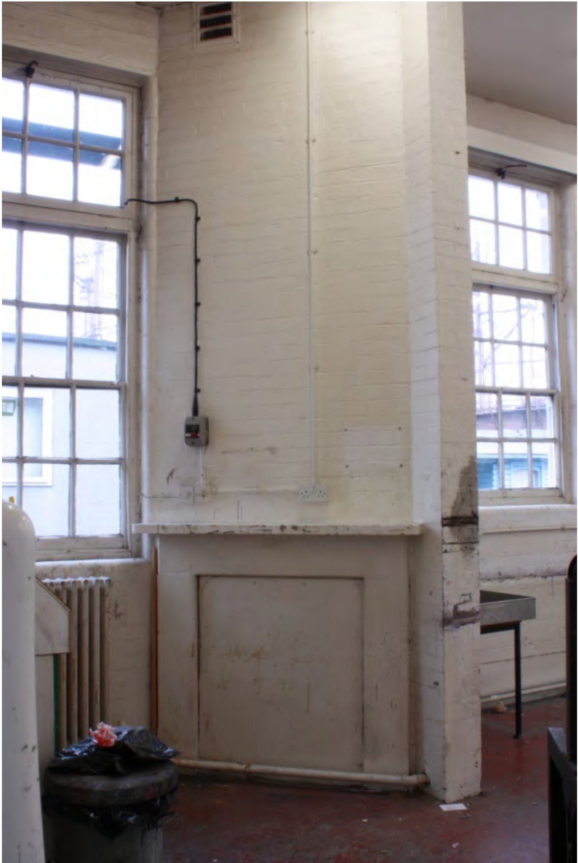
Plate 18: Angled chimney breast and fire surround (the only one with a mantel shelf in-situ ) in the west wall Room 10b in Block 200, looking north-west (D3/29)
