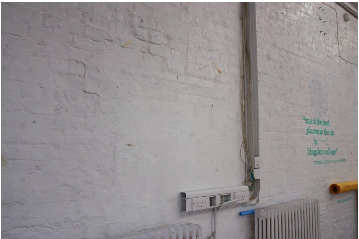
Plate 12c: Blocked doorway in the west wall of Room 1 in the Penny Gallery, looking north-west (D3/3)
