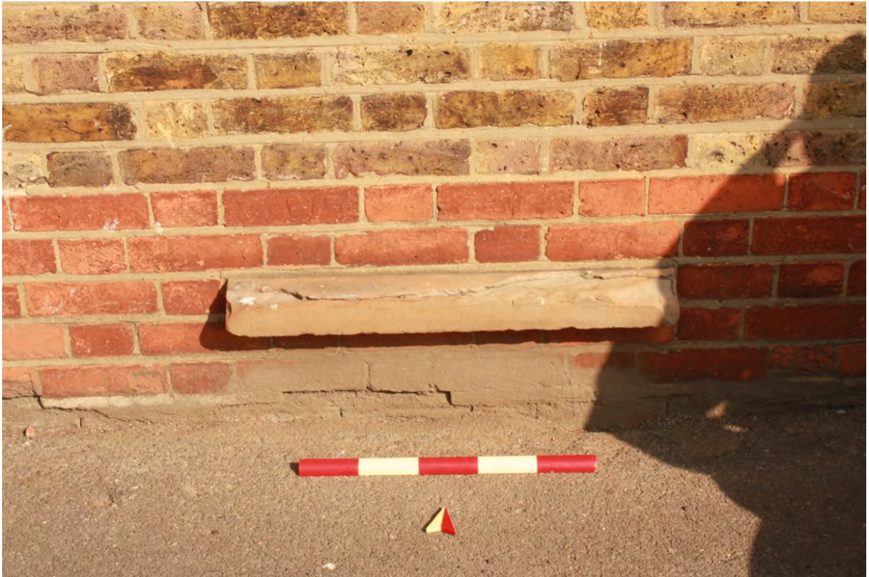
Plate 7: Stone sill boot scraper on the south elevation of Block 200, looking north. Scale 0.5m (D1/35)
