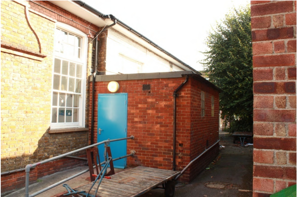
Plate 4e: Toilet extension to the side (south) elevation of the Penny Gallery, looking north-east (D1/29)
