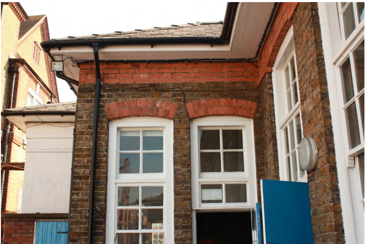
Plate 4f: West external wall of Room 2, looking east (D2/6)
