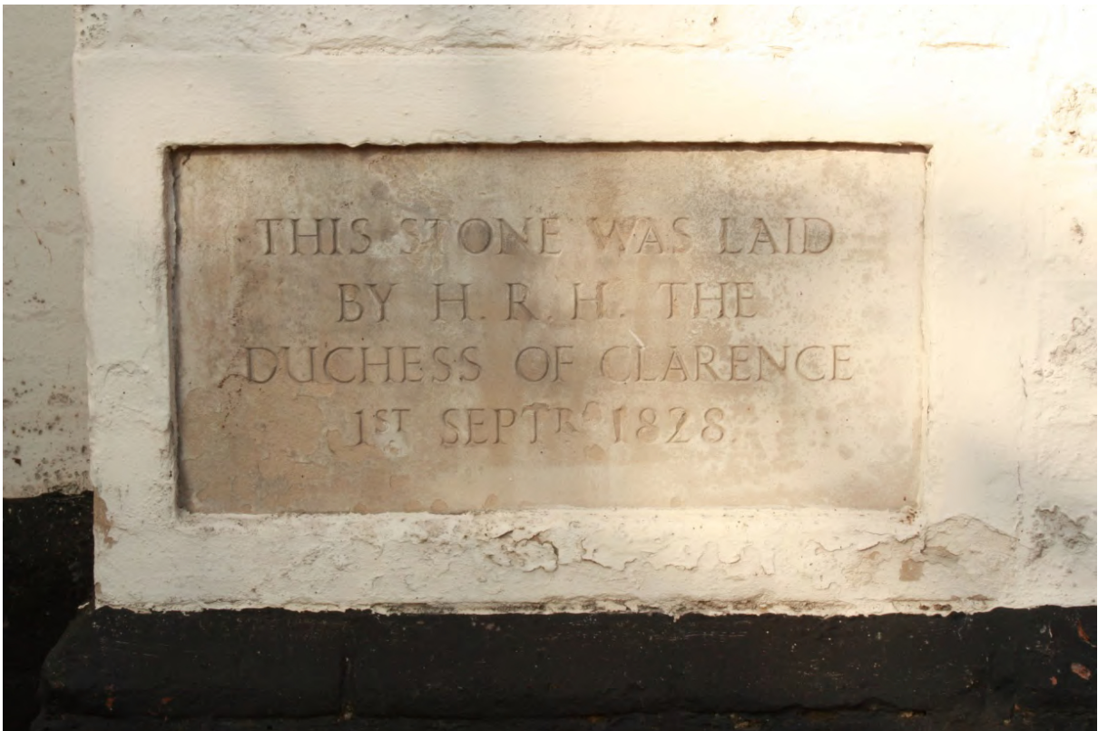
Plate 4a: Foundation stone in the front (east) elevation of the Penny Gallery, looking west (D1/13)
