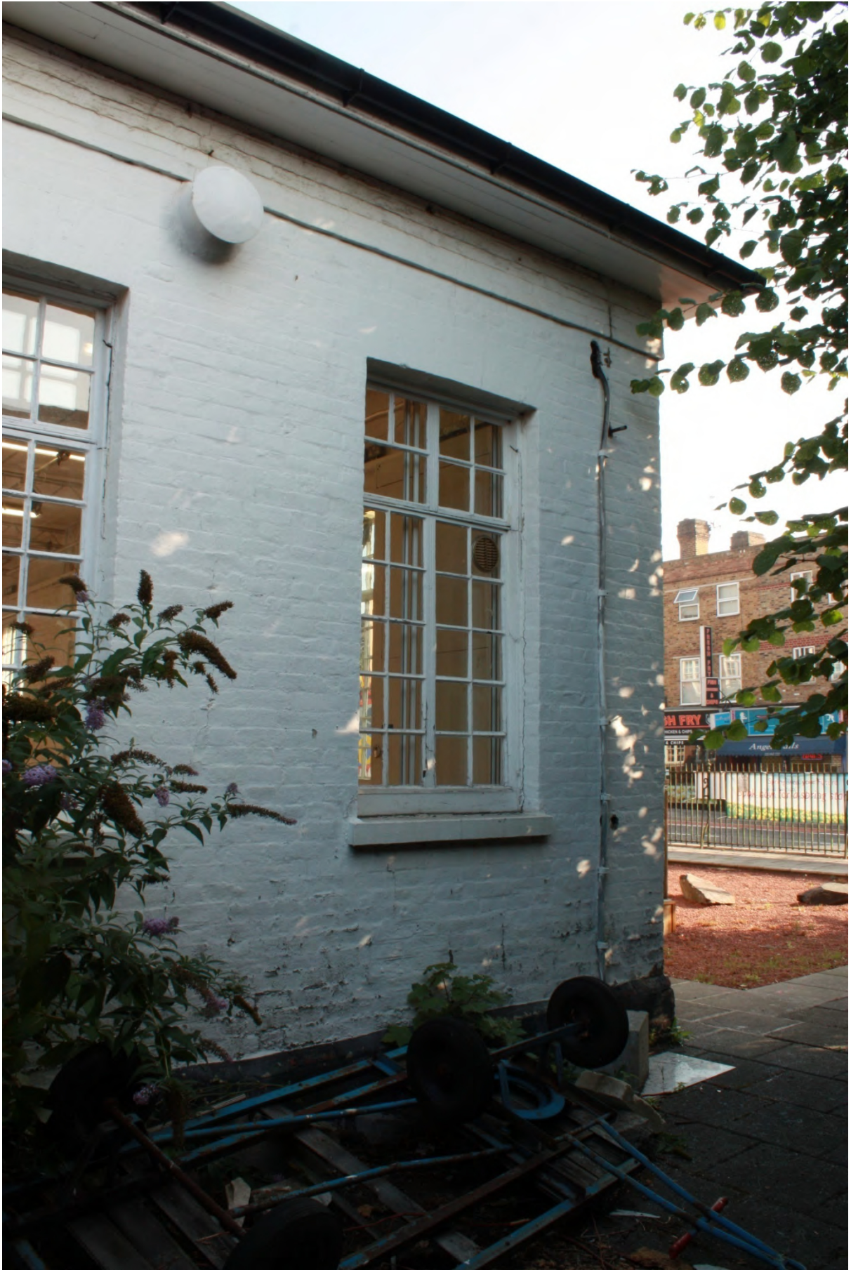
Plate 4d: Side (south) elevation of the Penny Gallery, looking north-east (D1/18)
