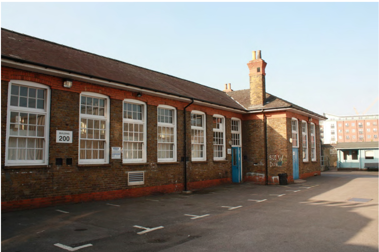
Plate 5: North elevation of Block 200, built in 1907, looking south-west (D1/3)
