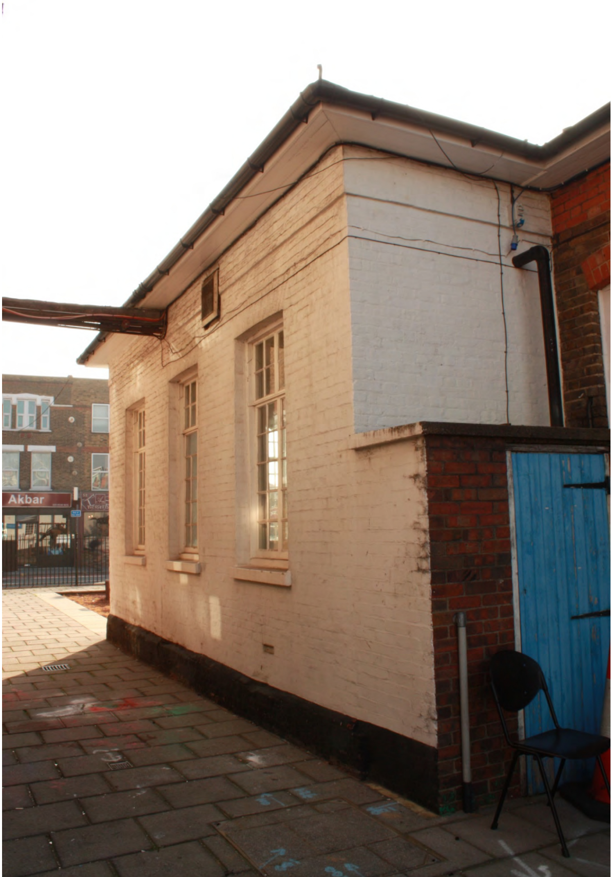
Plate 4c: Side (north) elevation of the Penny Gallery, looking east (D1/19)
