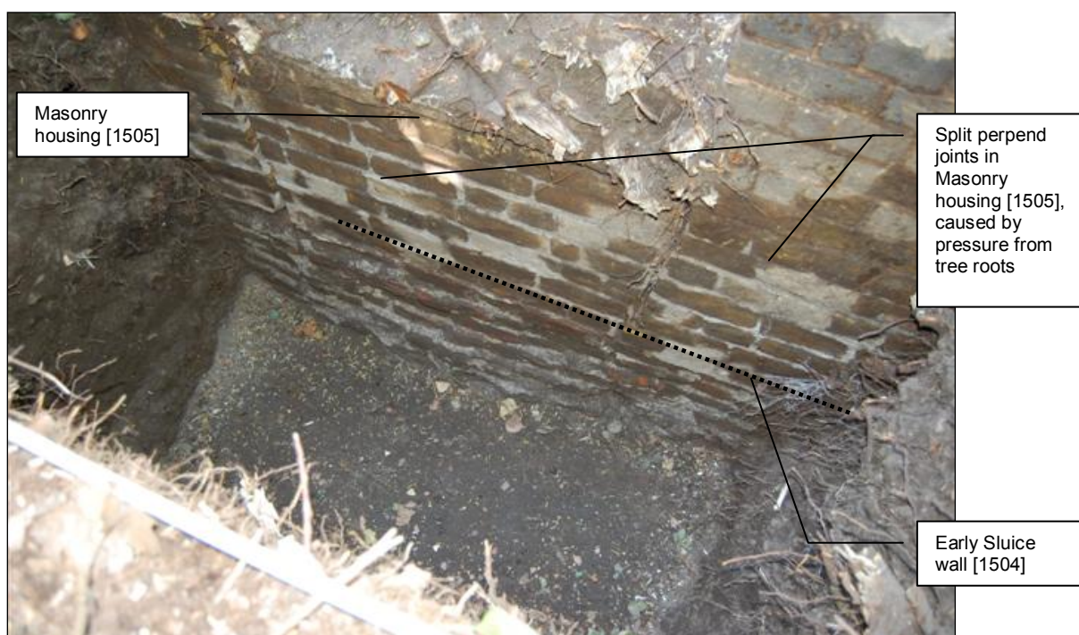
Figure 19: S elevation of moat sluice
