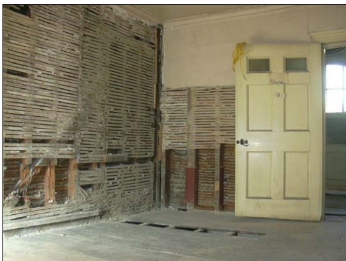
Figure 14: Stripped-off plaster revealing typical studwork and lath wall construction (Room 231 ↑NW)
