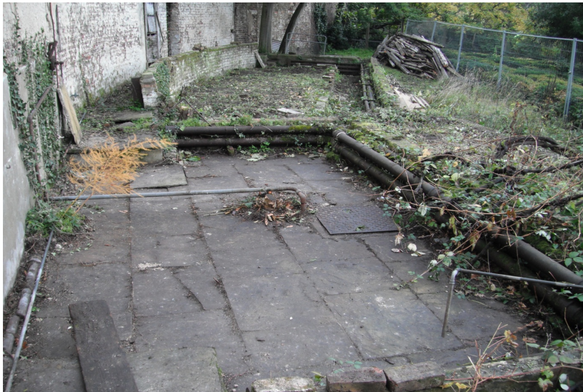
Figure 25: Vinery, facing southeast
