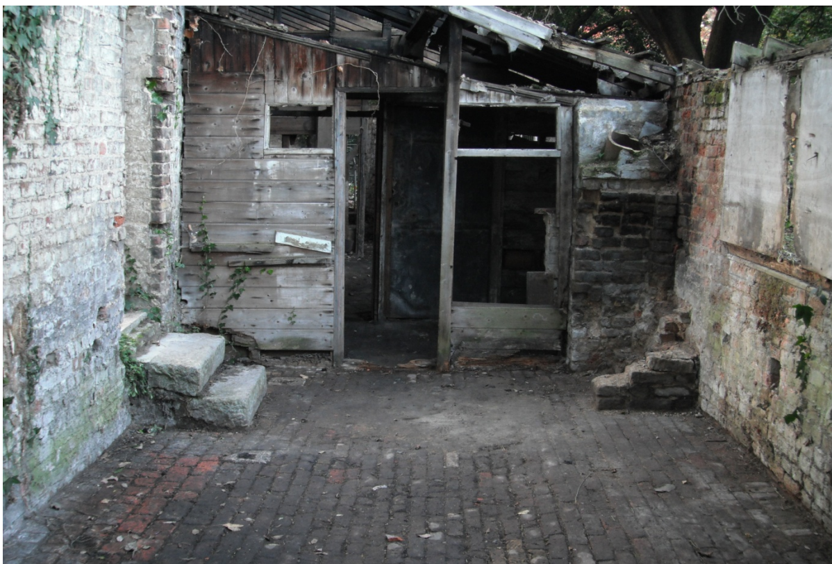
Figure 24: Interior of Bothy, facing northwest
