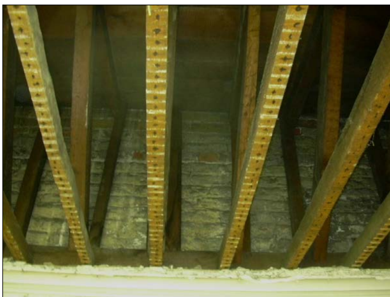
Figure 15: Brickwork with later build above rooms 230 & 231 (Room 227 ↑S)
