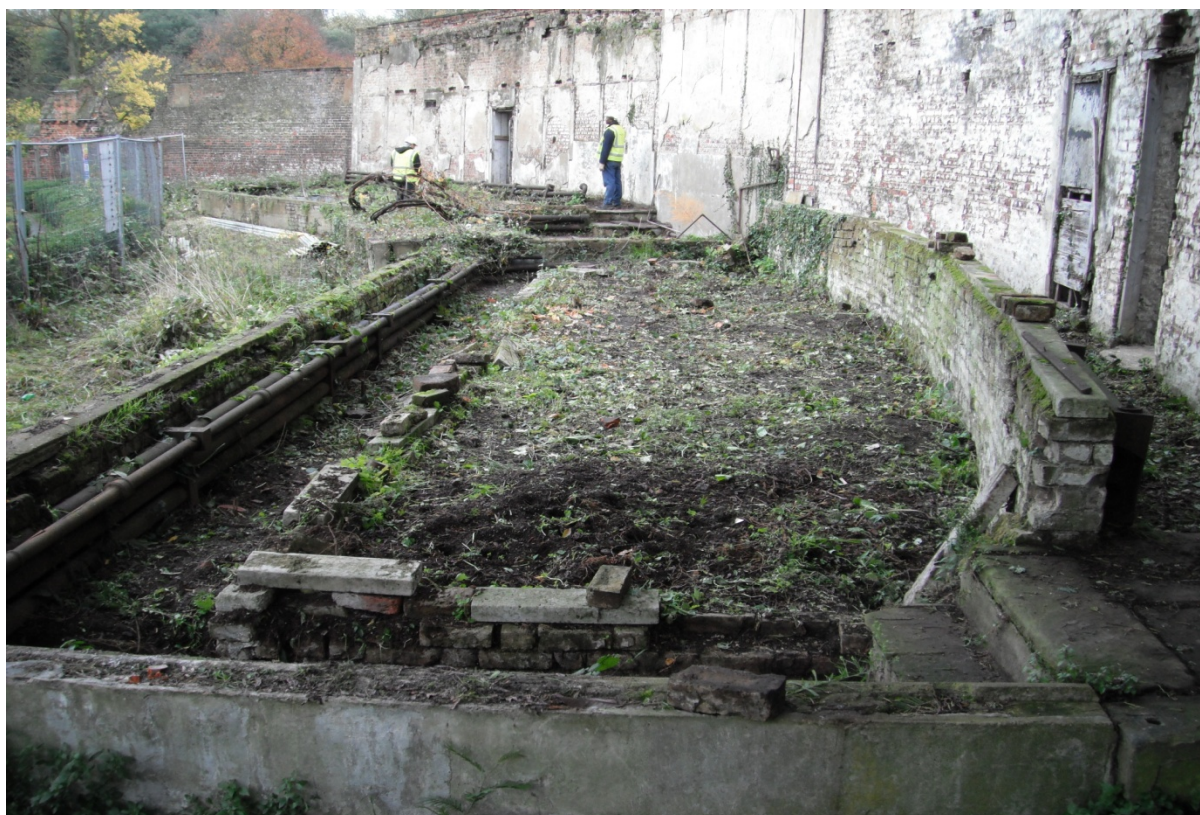
Figure 26: Vinery, facing west courses, which sprang from a stepped out brick plinth/foundation. Their presence in this area and a
