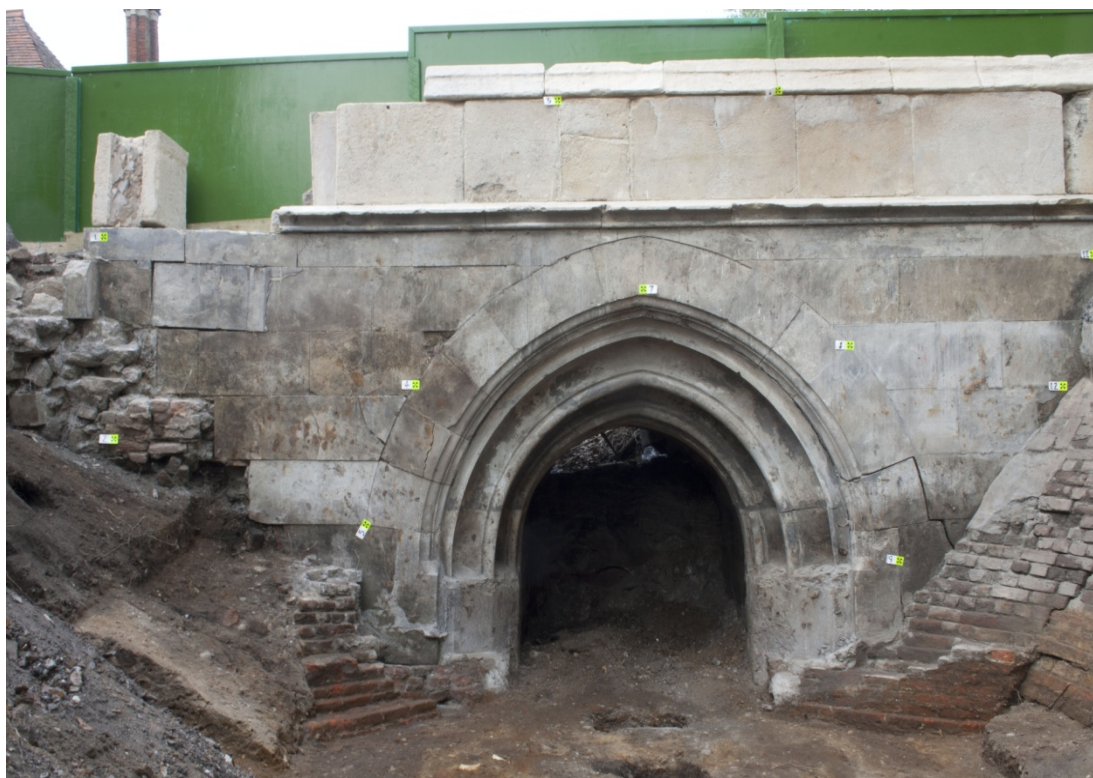
Figure 22: Moat Bridge, southwest facing
