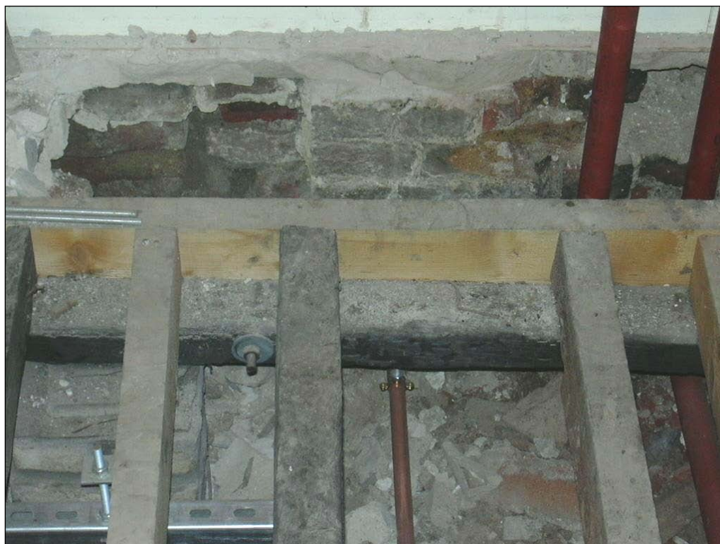
Figure 4: Possible Tudor Brickwork below later floor joists (Room 44 ↑E)
