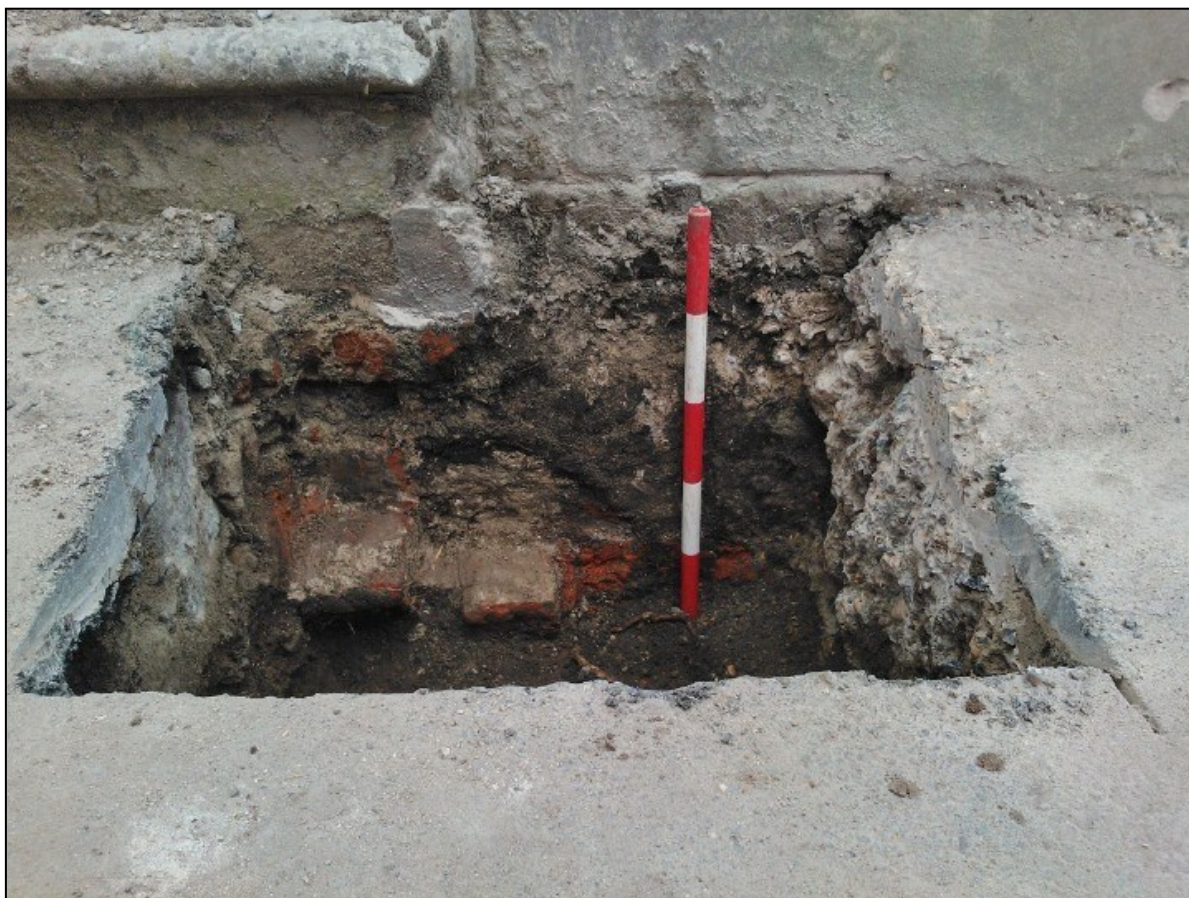
Plate 10: Northeast shot of 18th-century brickwork beneath the 19th-century gate pier in Trench 280
