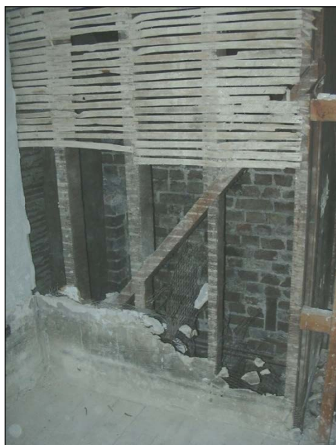
Figure 16: Construction details, (a) Room 239 – stud wall; (b) Room 240 – ceiling laths
