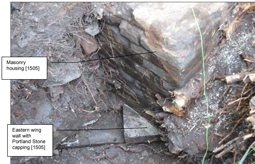
Figure 20: N elevation of moat sluice and eastern wing wall
