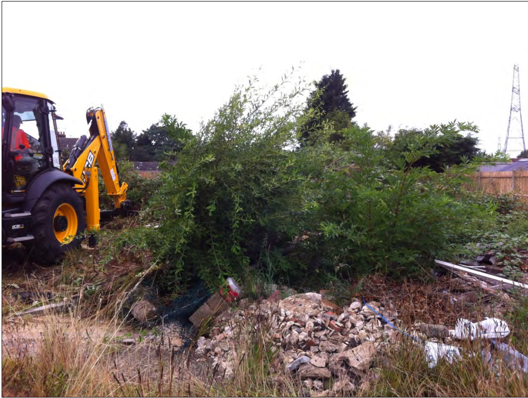
Plate 1: The site, view south-west
