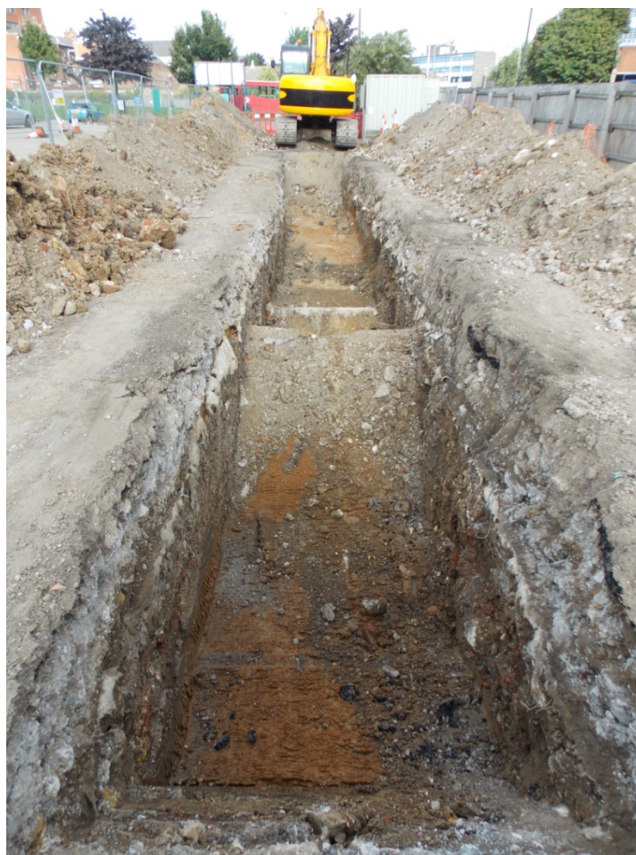
Plate 4: Trench 3, looking northeast
