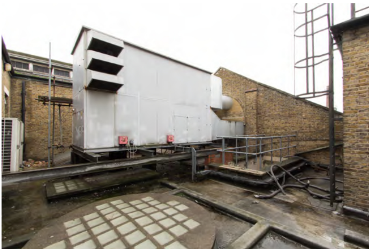
Plate 56 Air extractor/conditioner unit mounted on flat roof south of the Minor Pool, looking north-west
