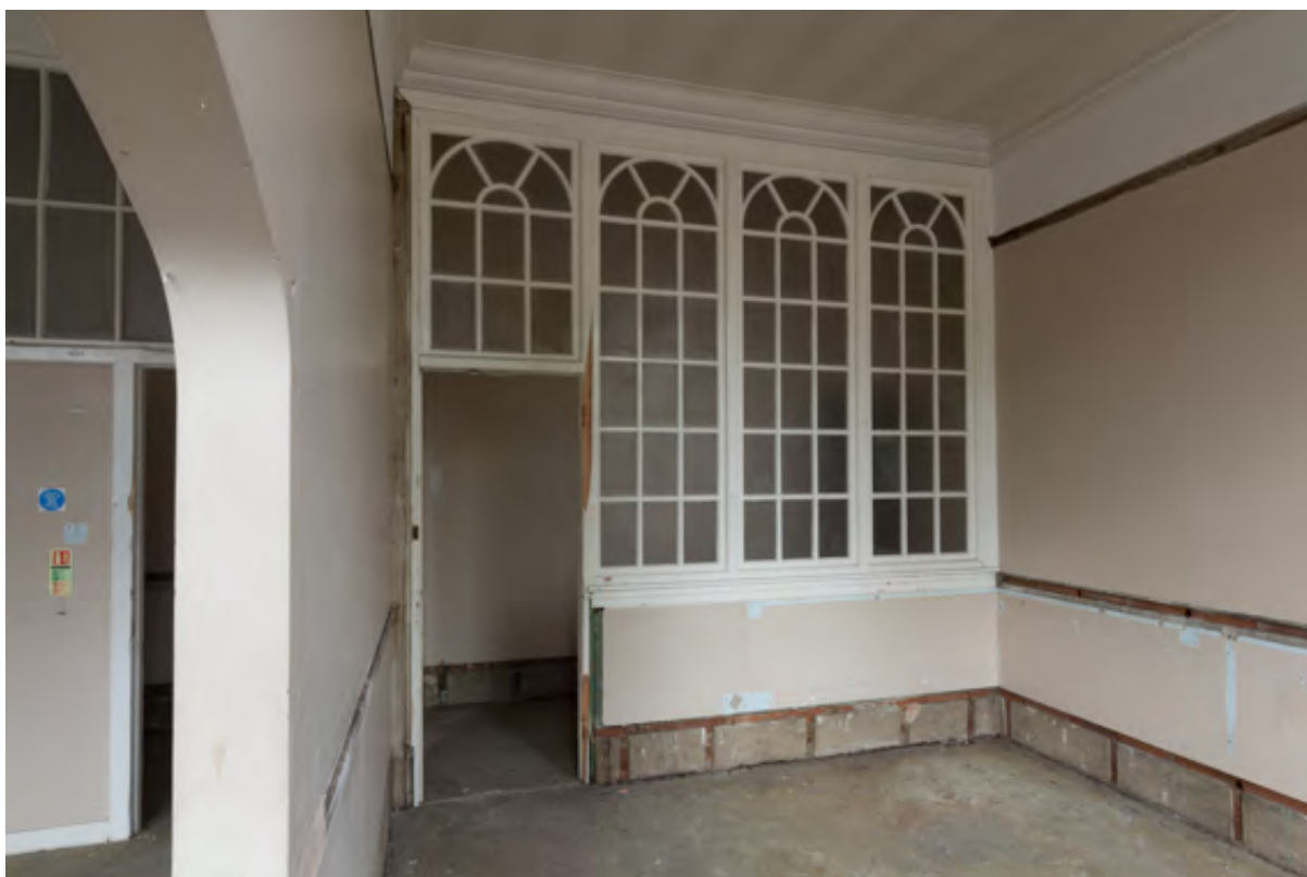
Plate 27 Original part glazed partition wall in Office Room (9), looking north-east
