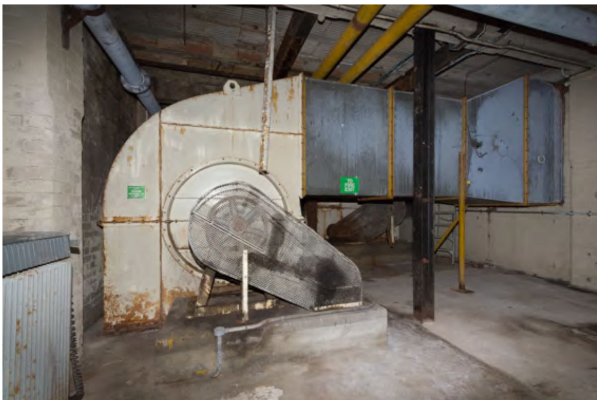
Plate 55 Air extractor unit in the Boiler House (northern Bays), looking west
