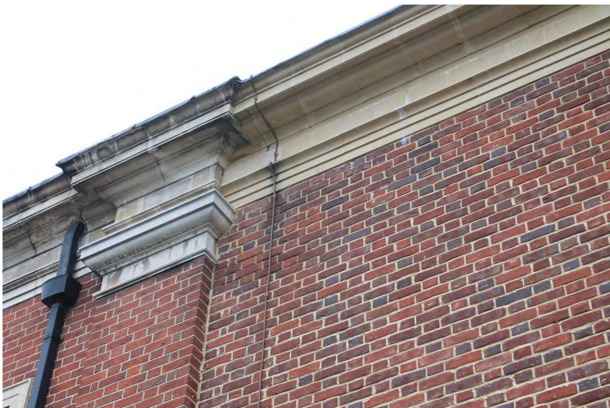
Plate 11 Rebuilt upper wall of hall and mismatching cornice in Atherton Road side (east) elevation, looking west
