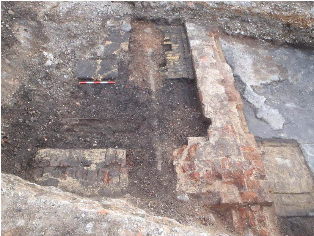
Plate 4: Wall [1] showing internal floor [2], machine/engine base [3] and external surface [5] looking east
