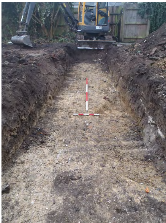
Plate 2: South facing view of Trench 2
