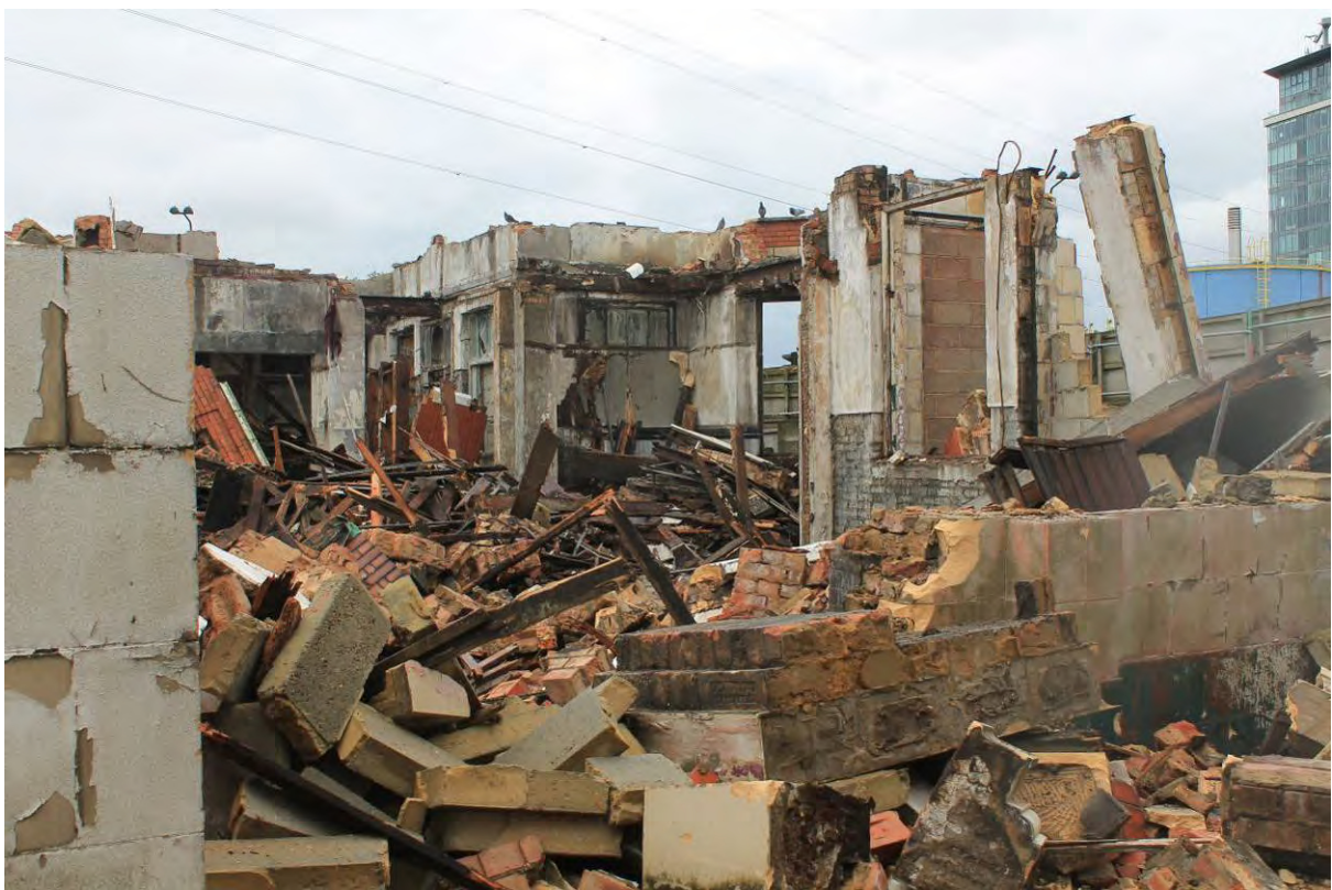
Plate 52 General view during demolition the Tidal Basin Tavern, looking north-east
