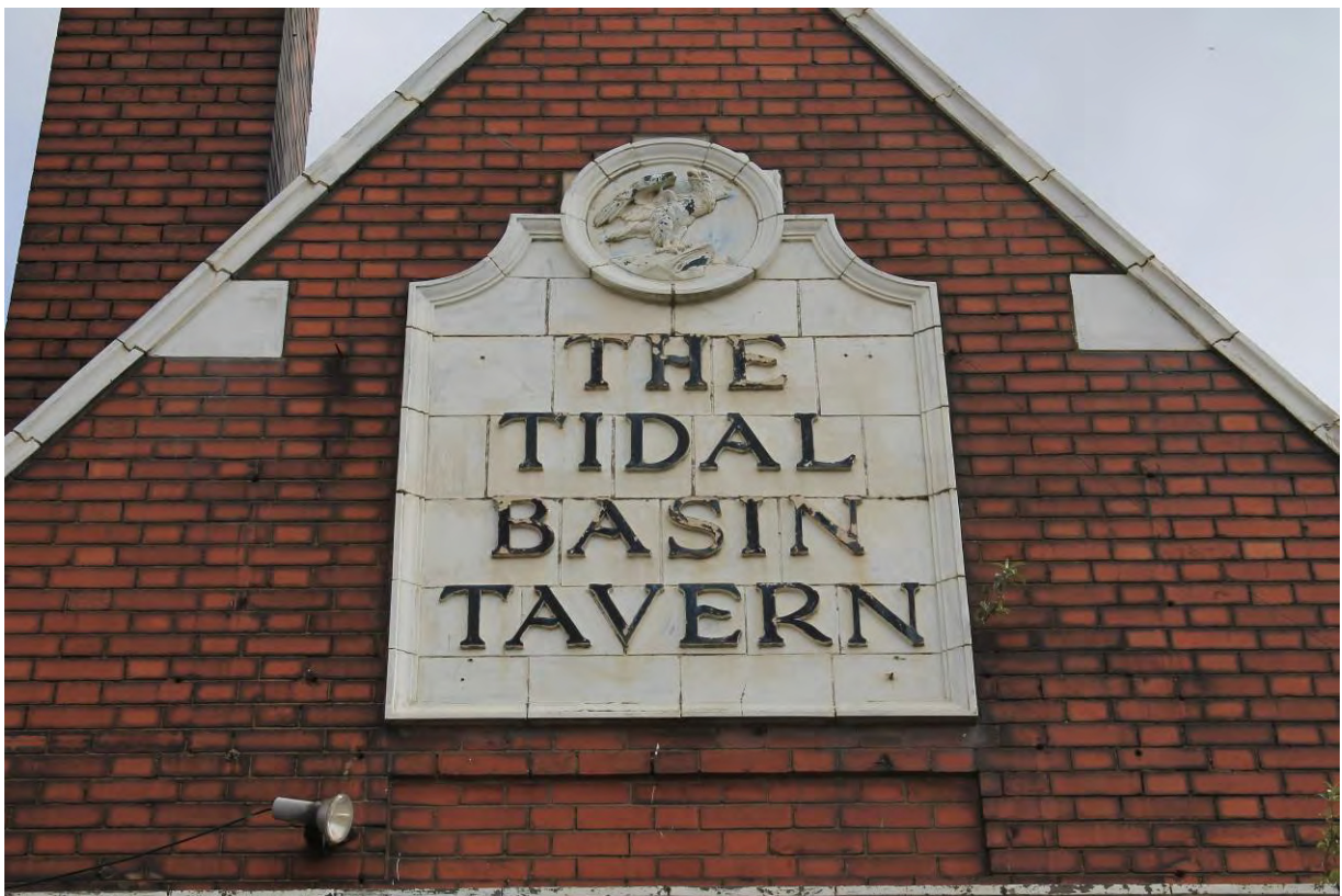
Plate 8 Terracotta name plaque with Truman's eagle inset on the north elevation of Tidal Basin Tavern, looking south
