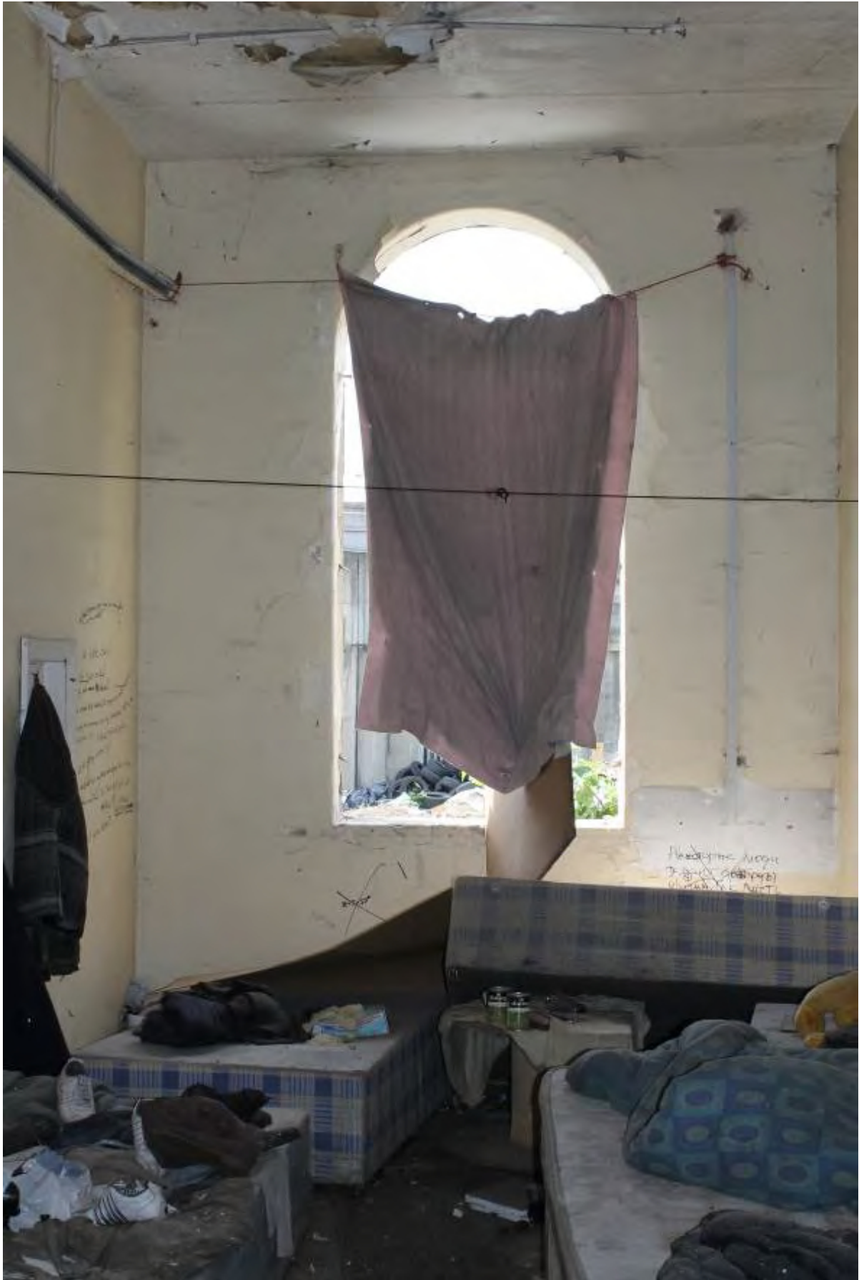
Plate 29 GF4 in Tidal Basin Road Post and Sorting Office, looking south
