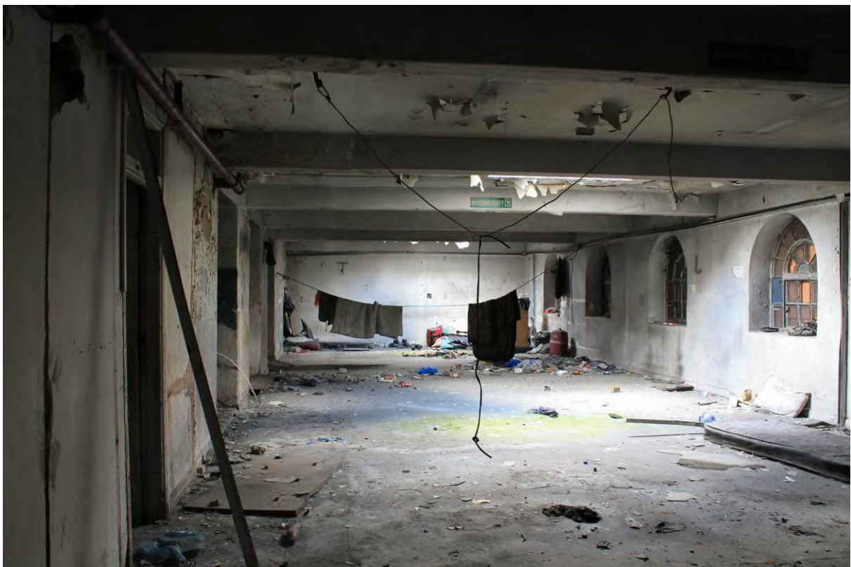
Plate 31 FF1 in Tidal Basin Road Post and Sorting Office, looking west
