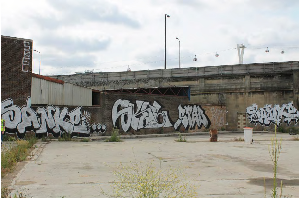
Plate 19 Western boundary wall of Tidal Basin Road Post and Sorting Office, looking south-east
