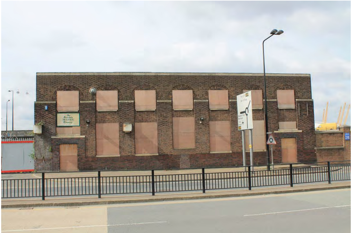
Plate 13 Front (north) elevation of Tidal Basin Road Post and Sorting Office, looking south
