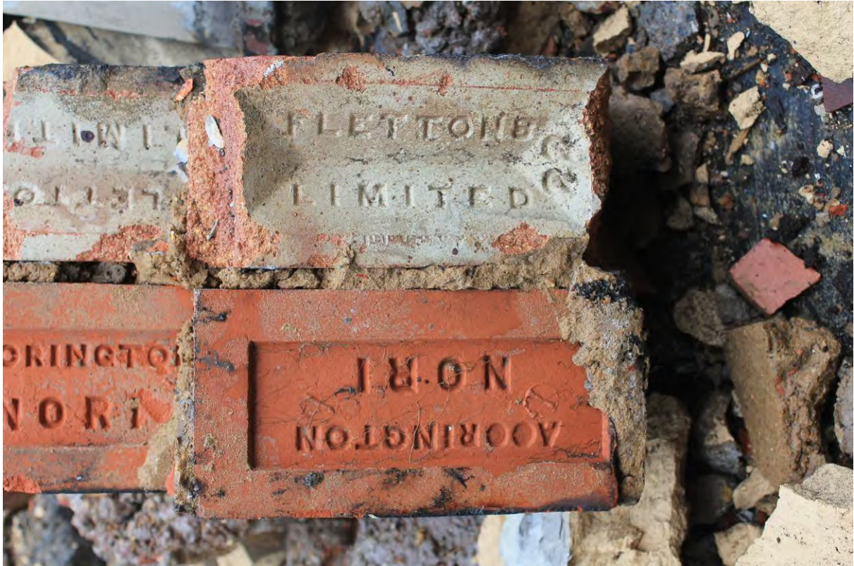
Plate 45 Typical wall section of the Tidal Basin Tavern with NORI facing brick and Fletton brick inner skin
