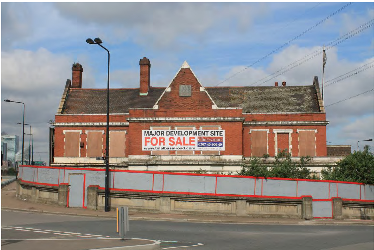
Plate 2 Tidal Basin Tavern east elevation, looking west
