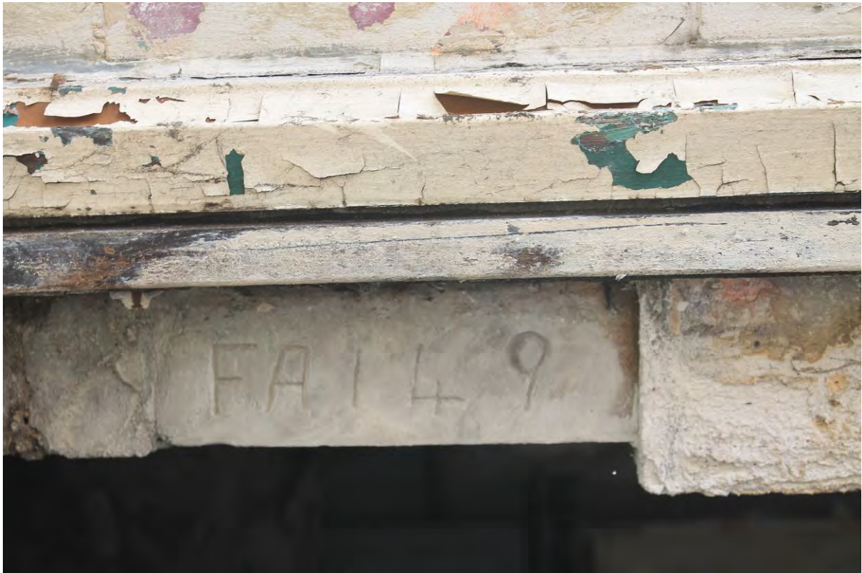
Plate 47 Terracotta block with batch ID mark within window jamb of principal (eastern) elevation of Tidal Basin Tavern, looking west
