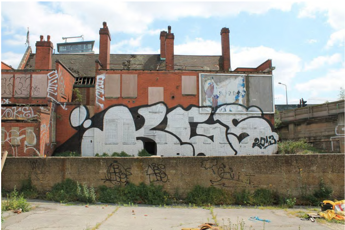
Plate 10 Rear (west) elevations of Tidal Basin Tavern, looking east
