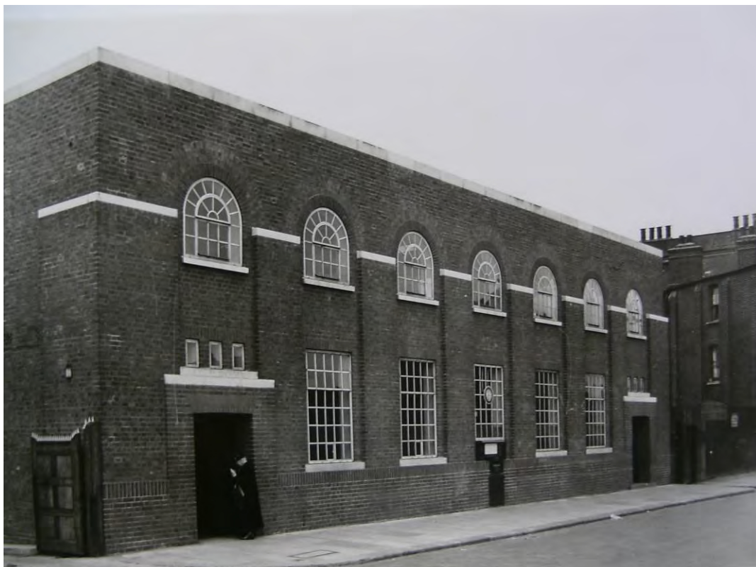
Plate 54 Photograph taken in 1934 of the recently opened Tidal Basin Road Post and Sorting Office showing its front (north) elevation, looking south-west (©British Postal Museum and Archive)
