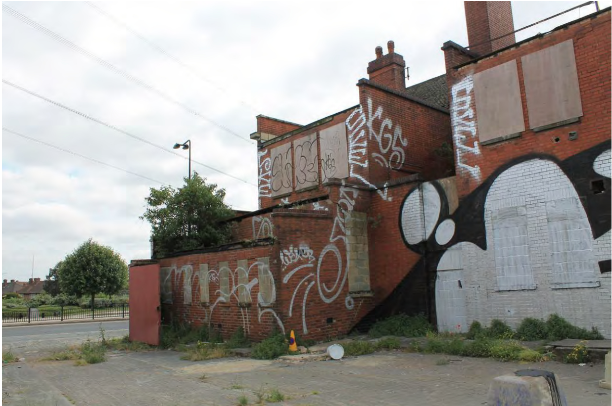
Plate 11 Rear (west) elevations and toilet block of Tidal Basin Tavern, looking north-east
