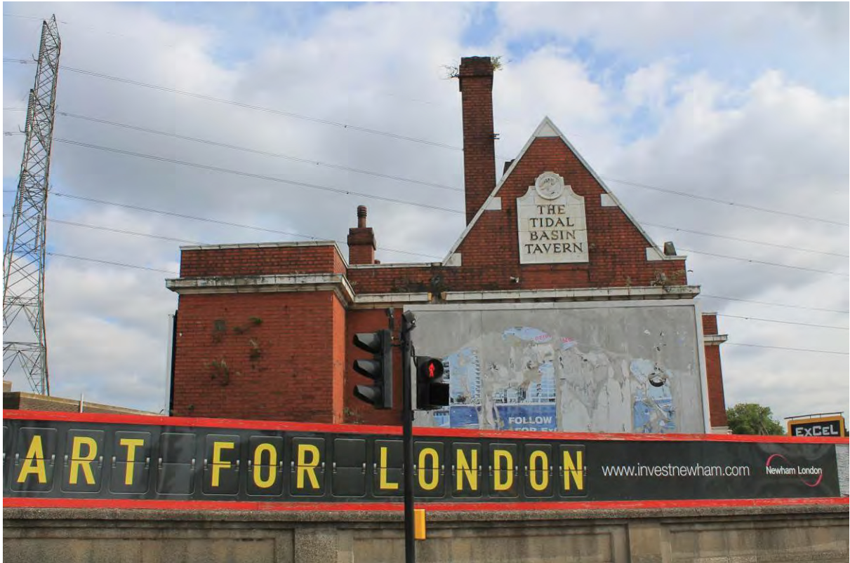
Plate 9 Tidal Basin Tavern south elevation, looking north
