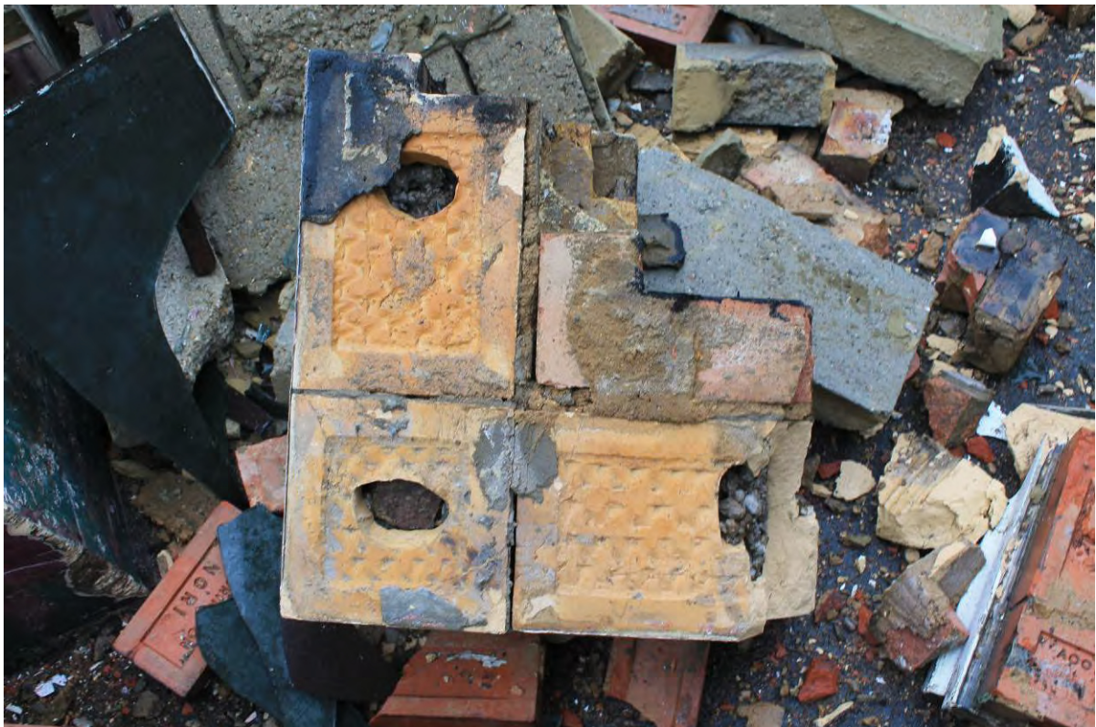
Plate 46 Hollow concrete filled terracotta facing blocks with internal Fletton brickwork from the Tidal Basin Tavern
