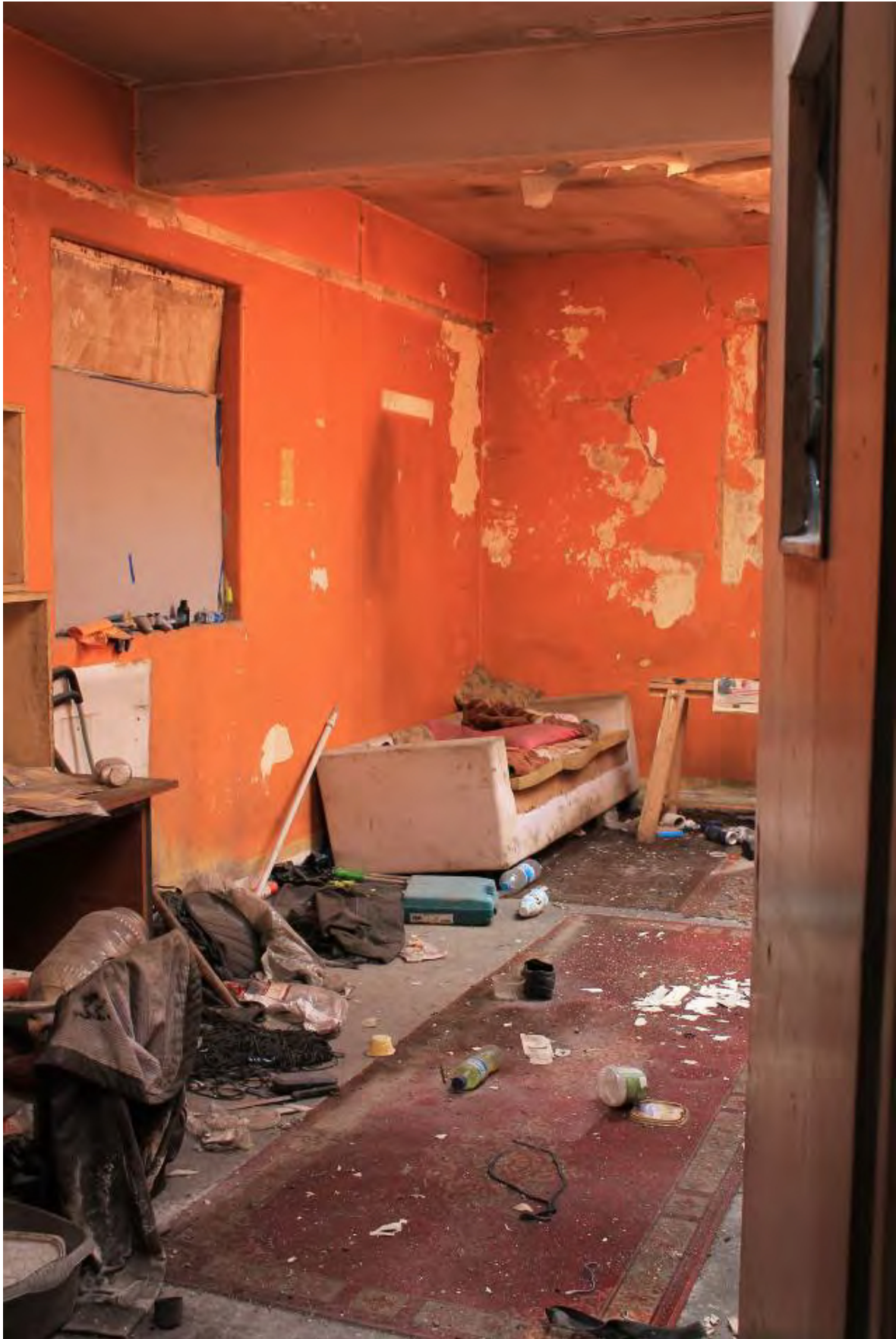
Plate 33 FF2 in Tidal Basin Road Post and Sorting Office, looking south
