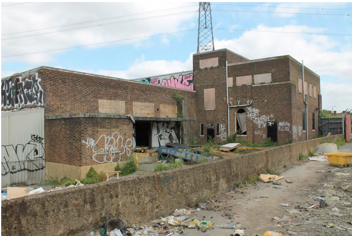
Plate 14 Side (east) elevation of Tidal Basin Road Post and Sorting Office, looking north-west
