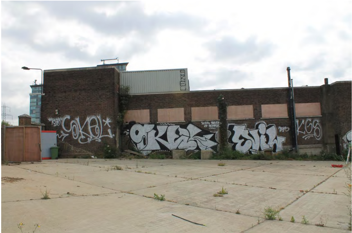
Plate 17 Western (side) elevations of Tidal Basin Road Post and Sorting Office, looking east
