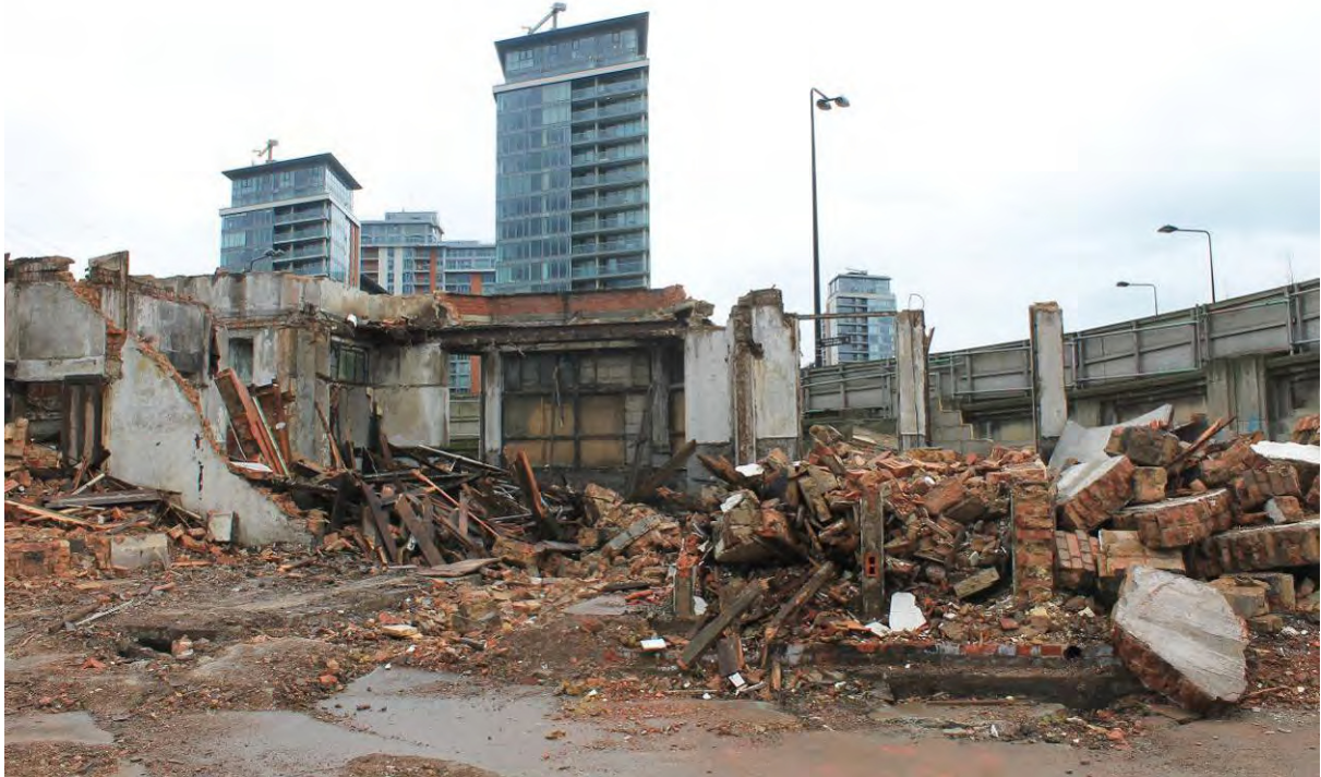
Plate 51 General view during demolition of the Tidal Basin Tavern looking east
