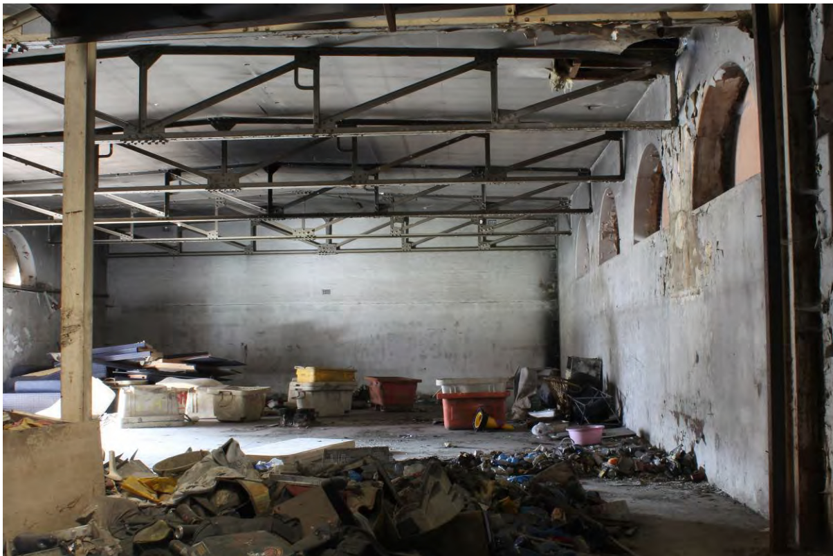
Plate 24 GF7 in Tidal Basin Road Post and Sorting Office, looking south
