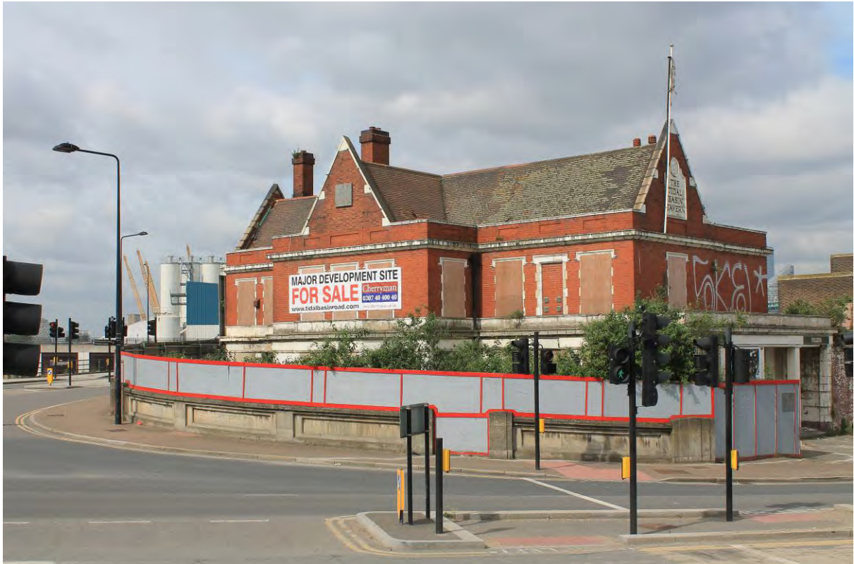
Plate 1 Tidal Basin Tavern east and north elevation, looking south-west
