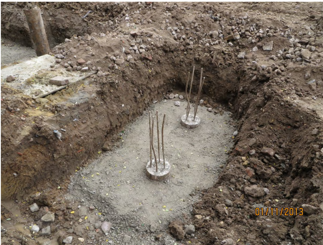
Plate 8: Trench 5, looking north-east (QUE13 D2 (8))
