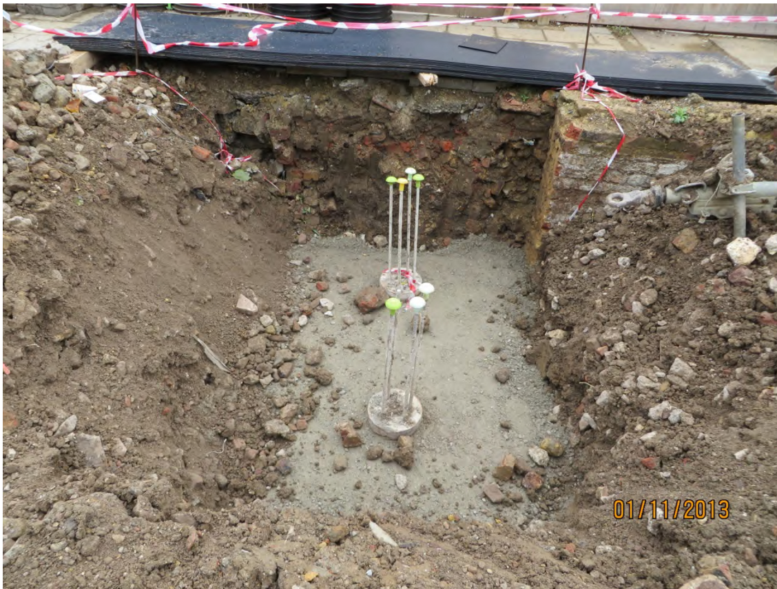
Plate 12: Trench 8, looking east (QUE13 D2 (19))
