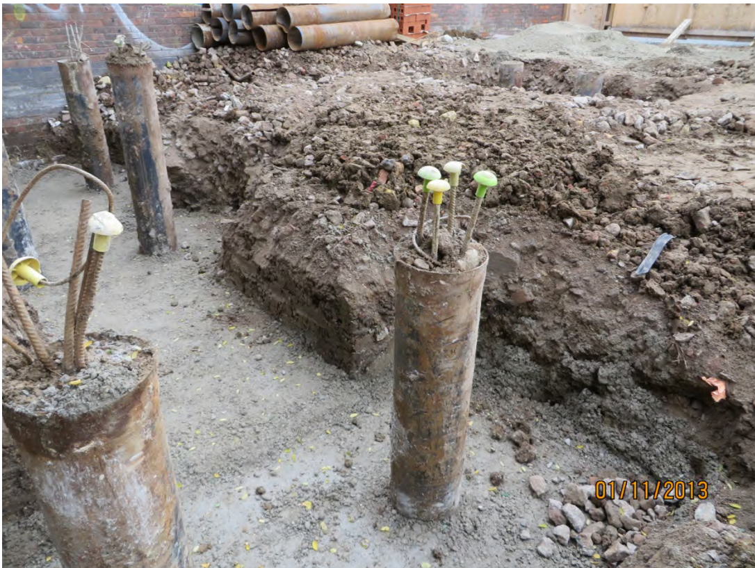
Plate 10: Trench 6, looking north-east (QUE13 D2 (15))
