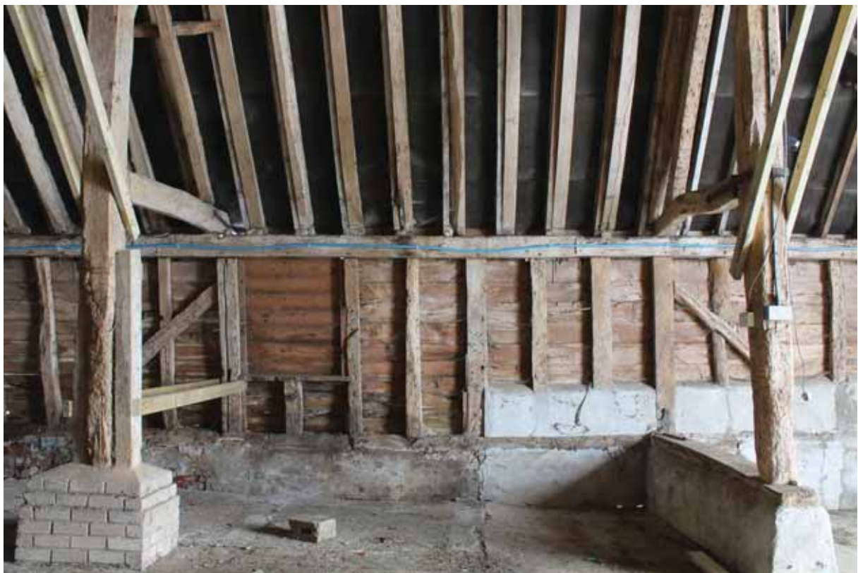
Plate 19 Northern aisle Bay 2, looking north
