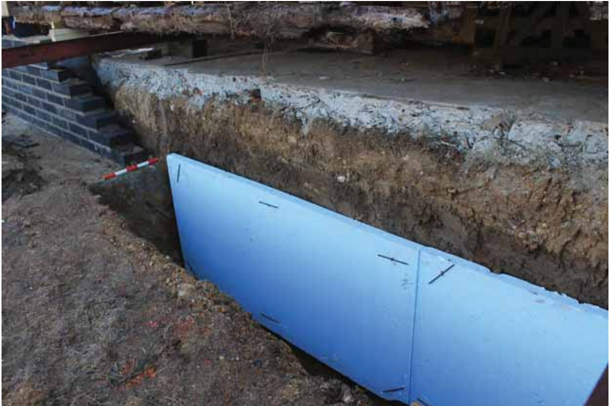
Plate 32 Trench C showing continuation of soil (102)
