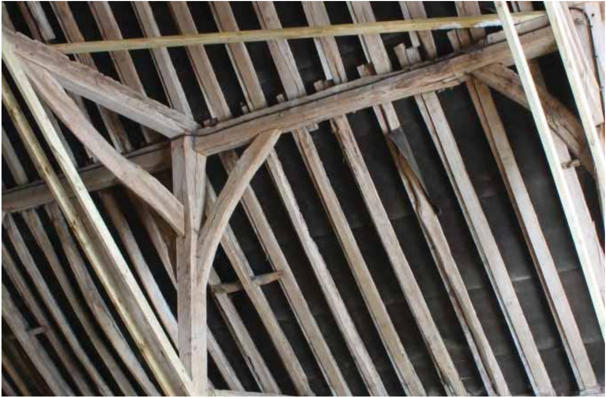
Plate 15 Jowled post of northern arcade, looking north-west
