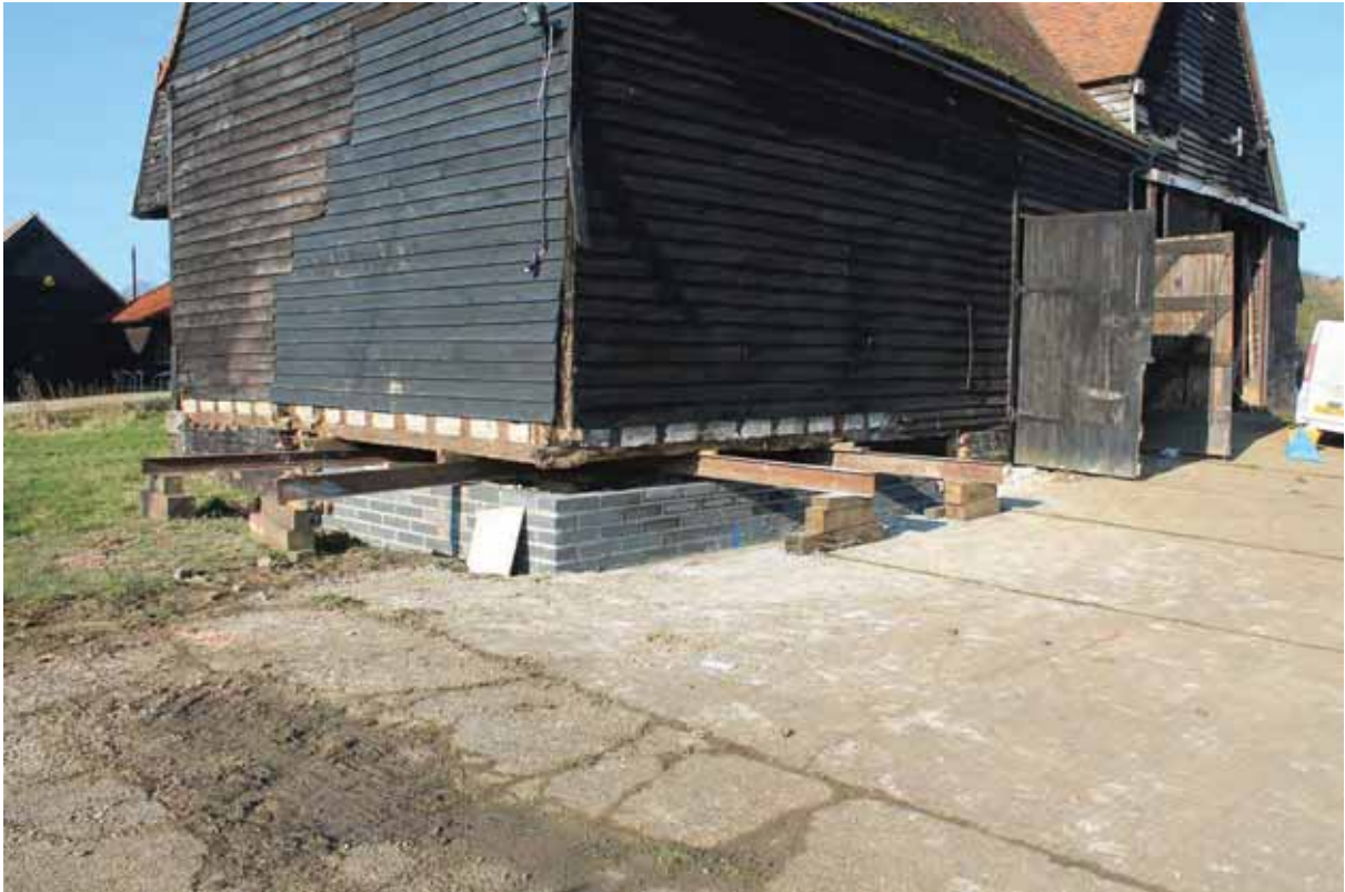
Plate 34 Underpinning south-eastern extension, looking north-west
