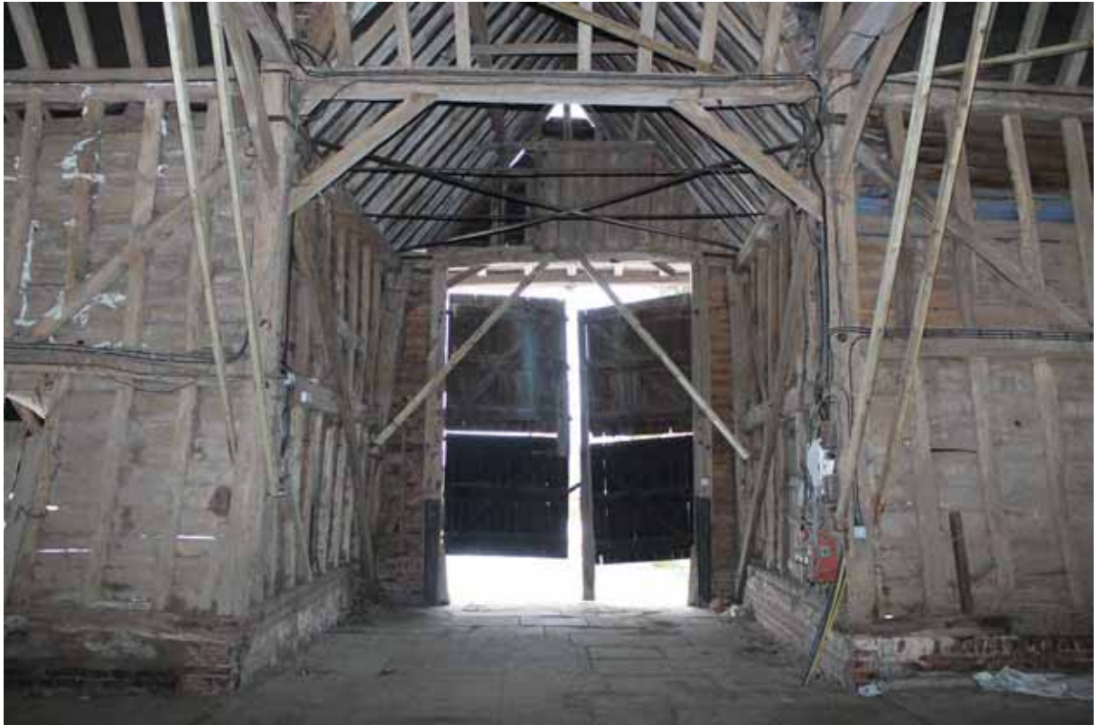
Plate 22 Midstrey (Bay 5), looking south
