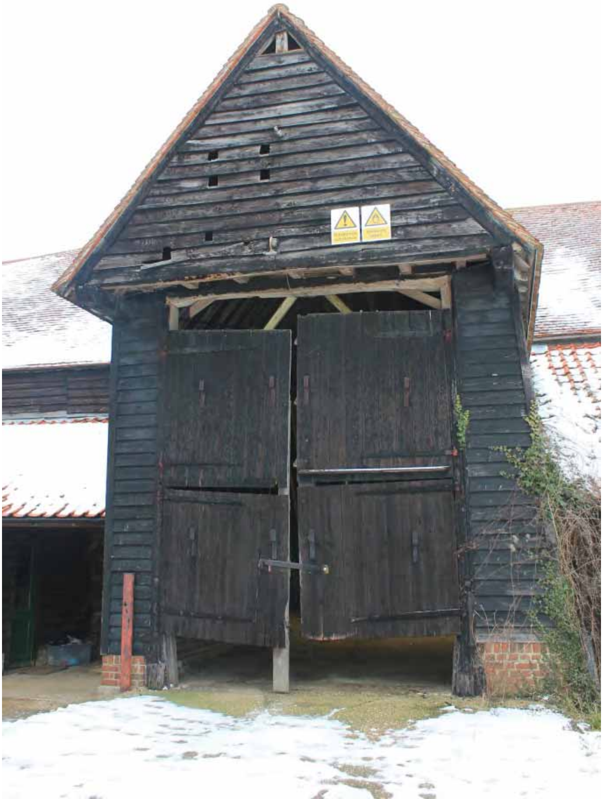
Plate 7 Midstrey with over-sailing gable dove-cote, looking north
