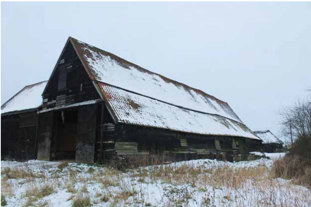
Plate 10 Northern Elevation, looking south-west
