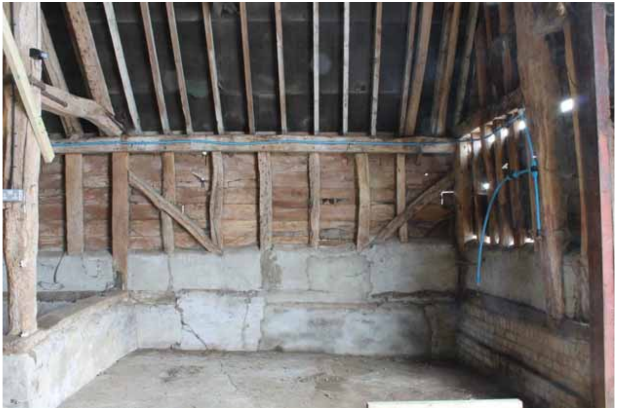
Plate 18 North aisle Bay 1, looking north
