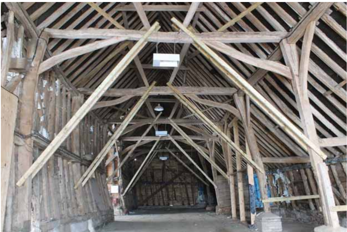
Plate 12 Interior of aisled barn, looking west
