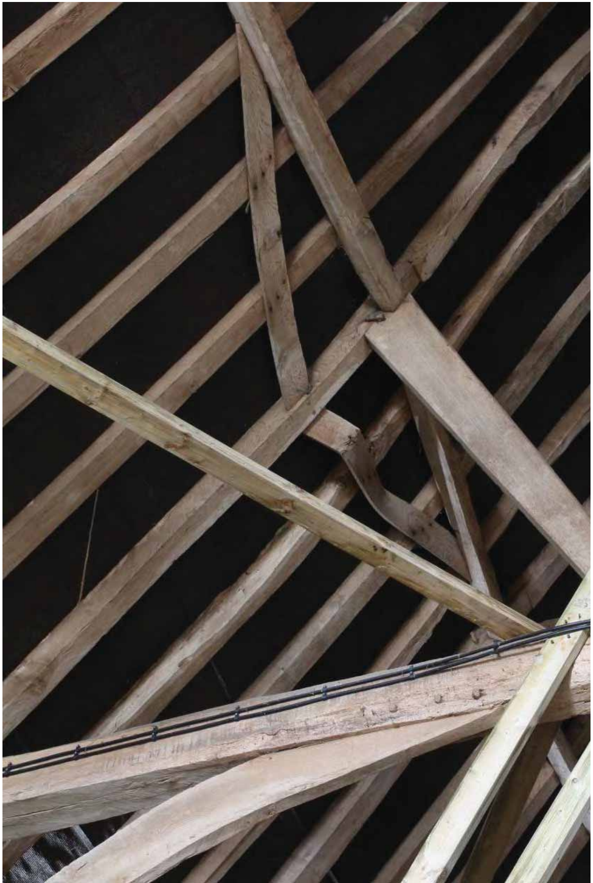
Plate 17 Wind brace over Bays 6 and 7, looking south-west
