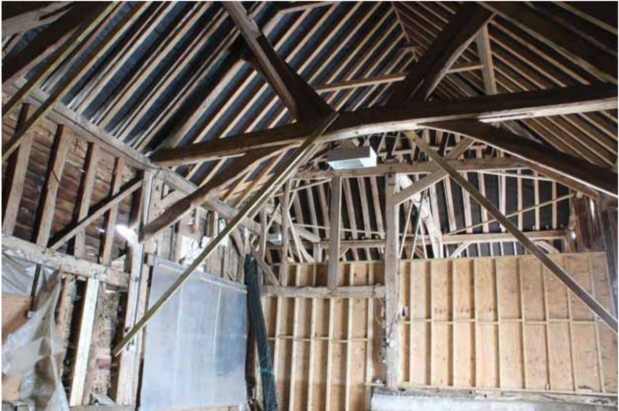
Plate 26 South-eastern extension, showing deep arch braces, looking north-west
