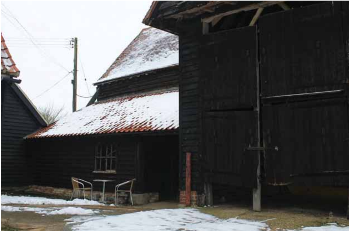
Plate 9 Lean-to Building, looking north-west
