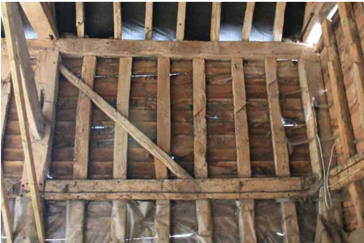
Plate 25 Eastern wall frame of south-eastern extension (Bay E1), looking east
