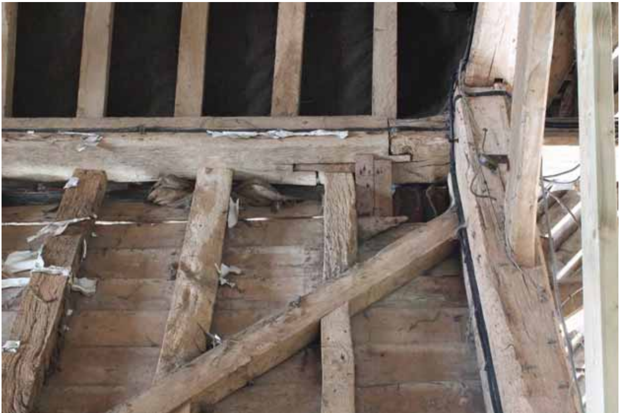
Plate 16 Face halved and counter bladed scarf joint in south wall plate, looking south
