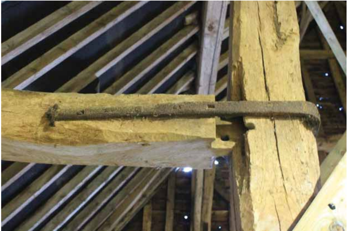
Plate 20 Historic repair using wrought iron strap (Bay 1/2), looking east
