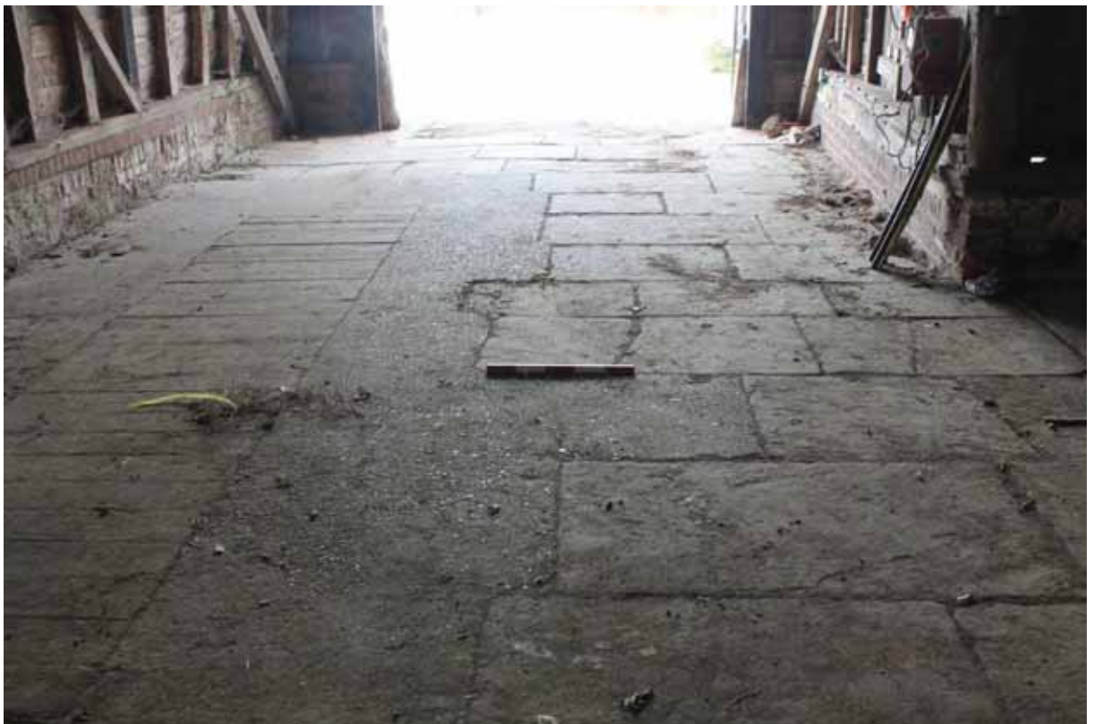
Plate 23 Remains of the stone flag threshing floor in the midstrey, looking south
