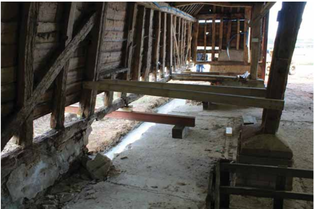
Plate 33 Underpinning works along northern aisle, looking east
