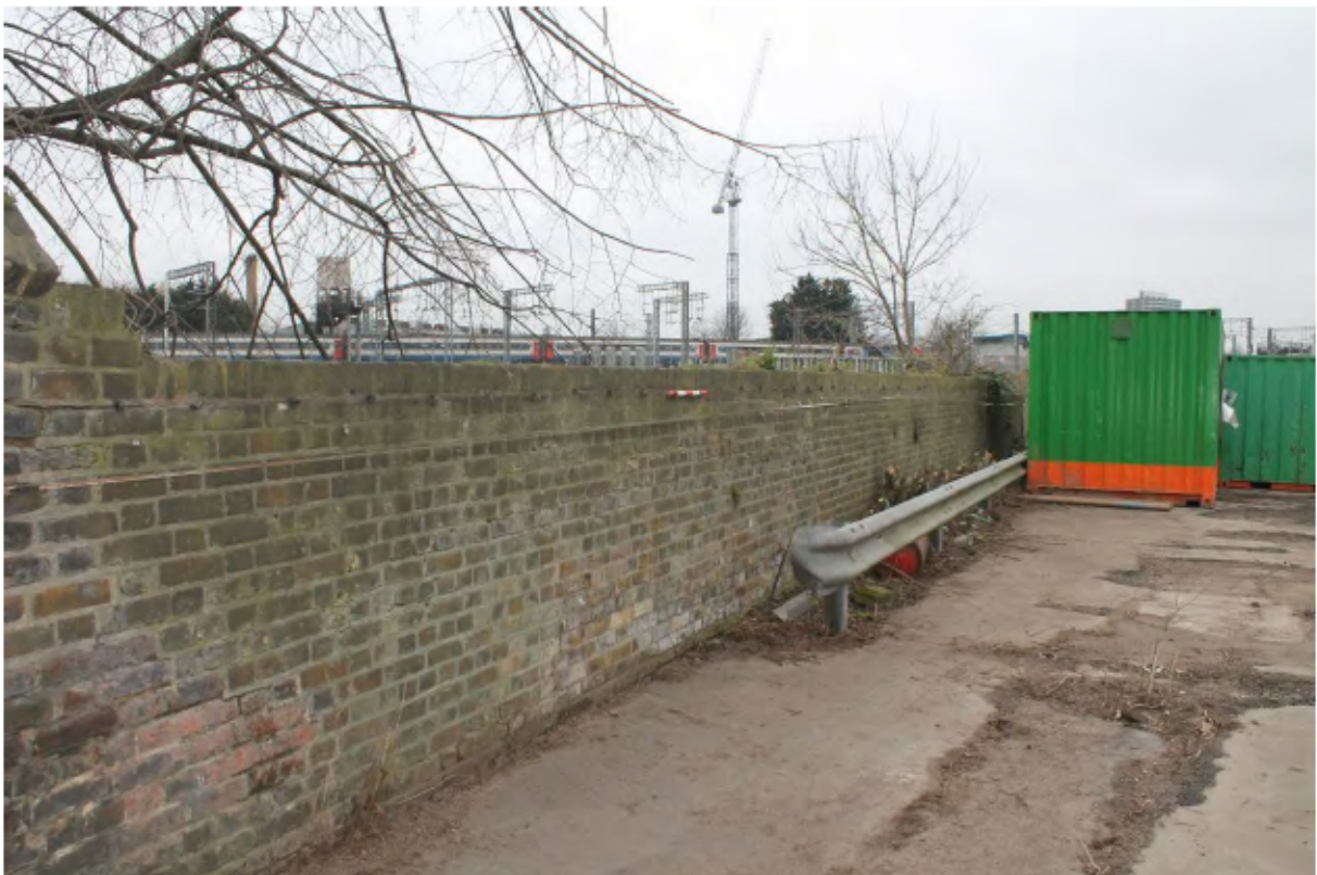
Plate 8: North-east (land) side of the north canal wall showing rebuilt yellow stock brick wall, looking north-west from Point M towards Point N
