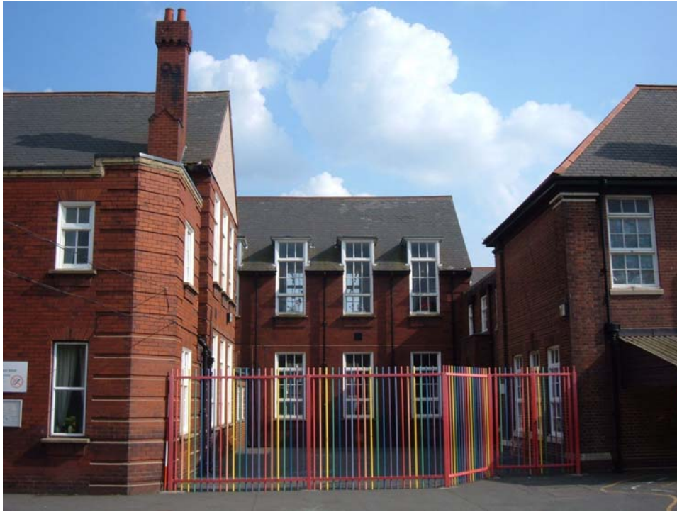
Plate 9. Main building, hall block, north elevation (west end), from the north-west (2m scale).
