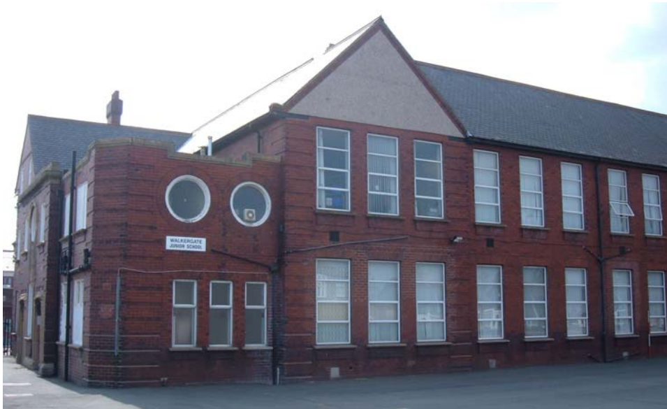
Plate 3. Main building, east elevation (south end), from the east (2m scale).
