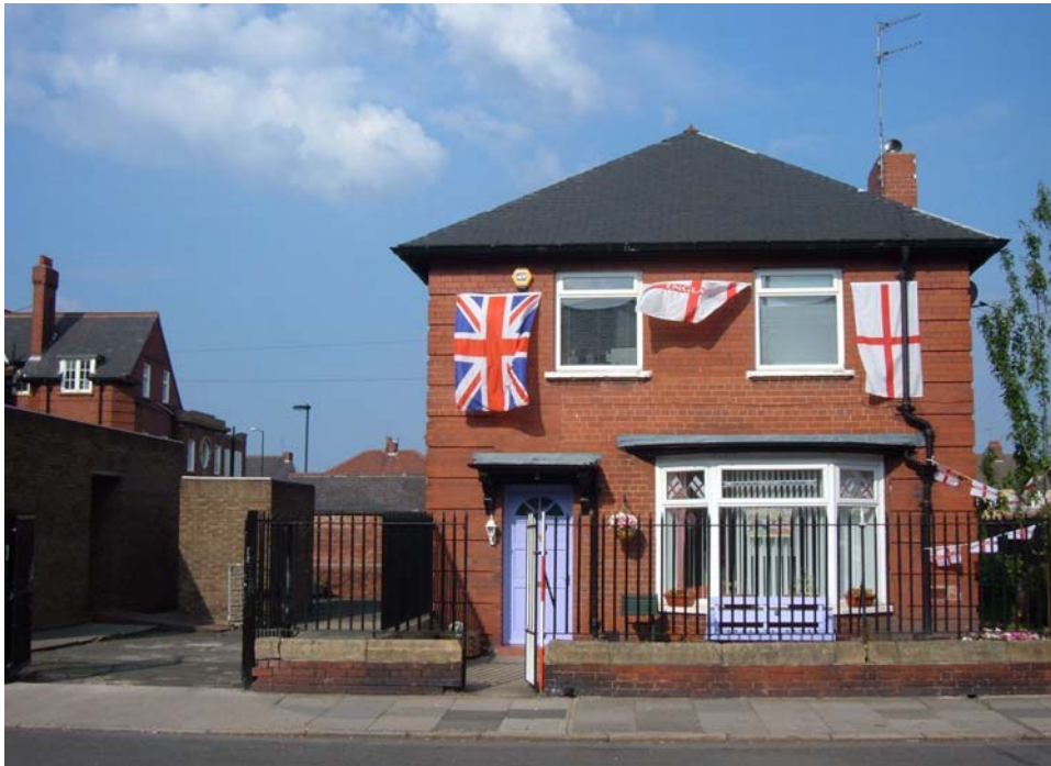
Plate 40. Caretaker's house, west elevation, from the south-west (2m scale).
