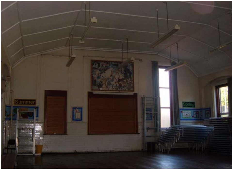
Plate 63. Former infants' block, hall interior, from the north-east.
