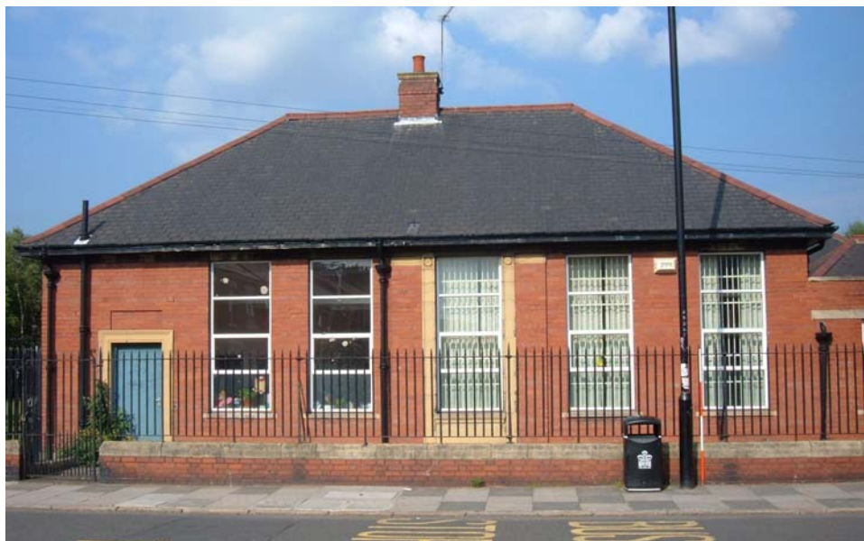
Plate 32. Former infants' block, west wing, west elevation, from the south-west (2m scale).
