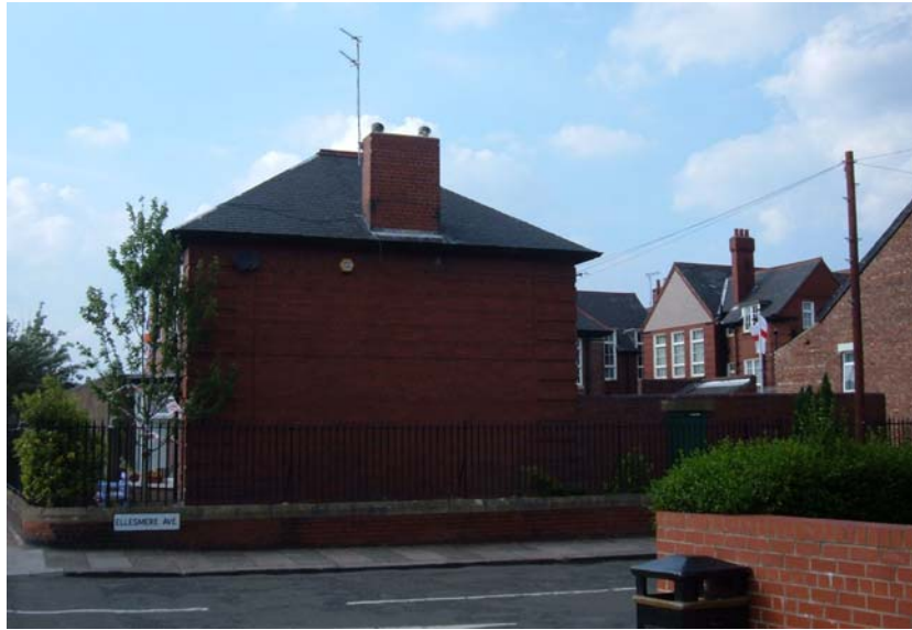
Plate 41. Caretaker's house, south elevation, from the south.
