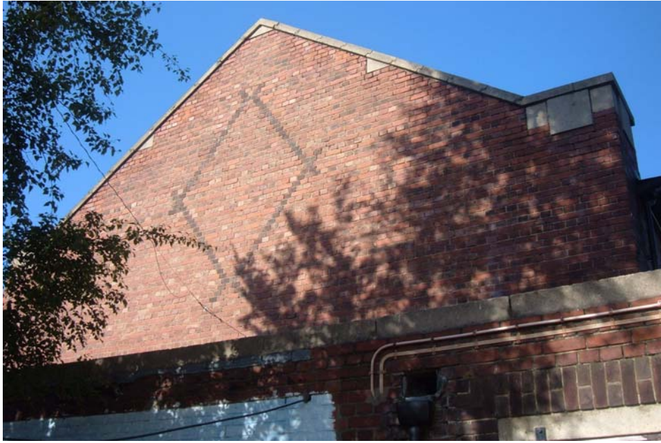
Plate 15. Gym block, west elevation, upper part, from the south-west.
