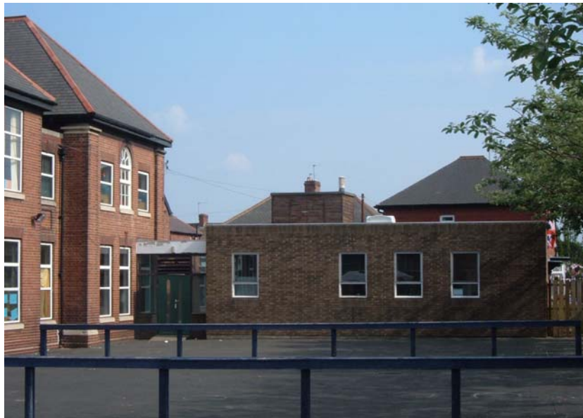
Plate 42. Kitchen block, north elevation, from the north-west.
