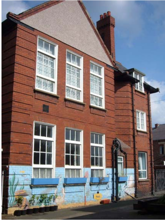
Plate 5. Main building, south wing, west elevation, from the north-west (2m scale).
