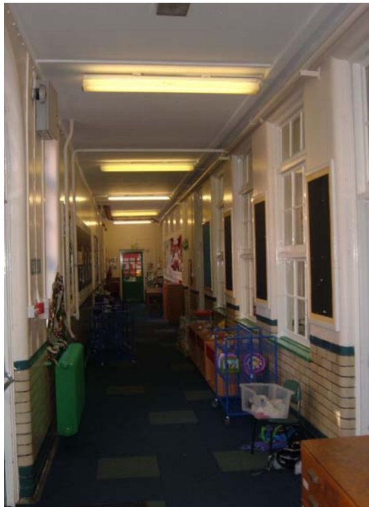
Plate 54. Former secondary modern block, ground floor, main corridor, from the north-west.
