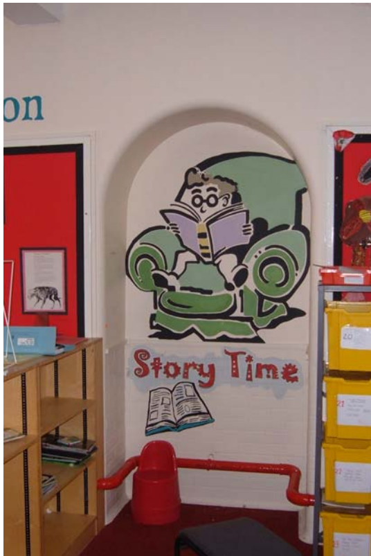
Plate 59. Former secondary modern block, ground floor, south wing, detail of former furnace in south wall of classroom, from the north-west.
