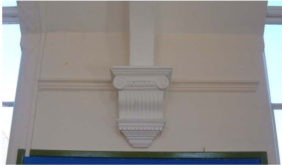
Plate 53. Main building, first floor, detail of impost in upper hall, from the south-east.
