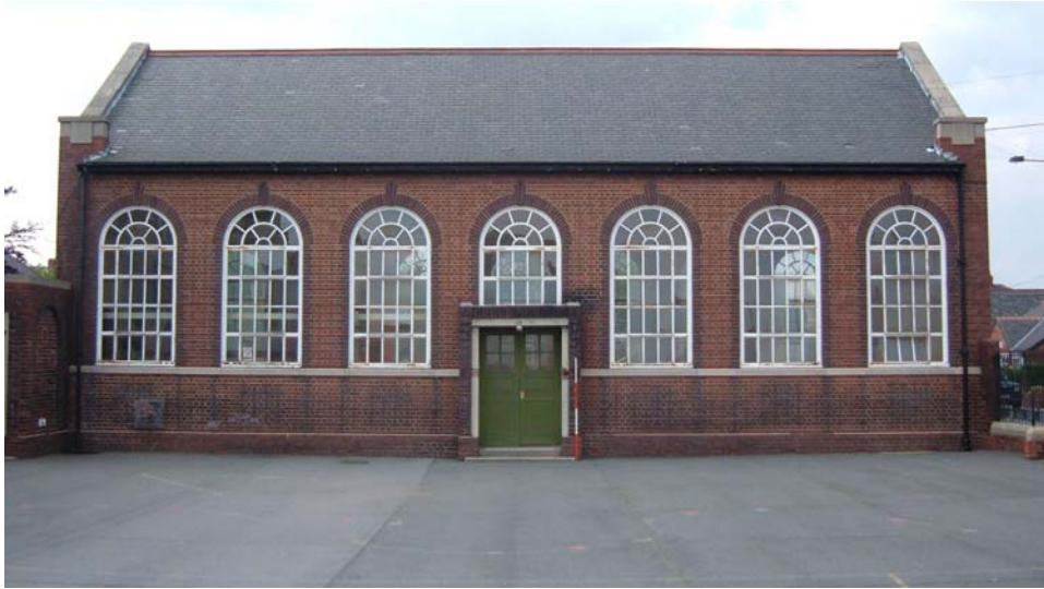
Plate 13. Gym block, south elevation, from the south-east (2m scale).
