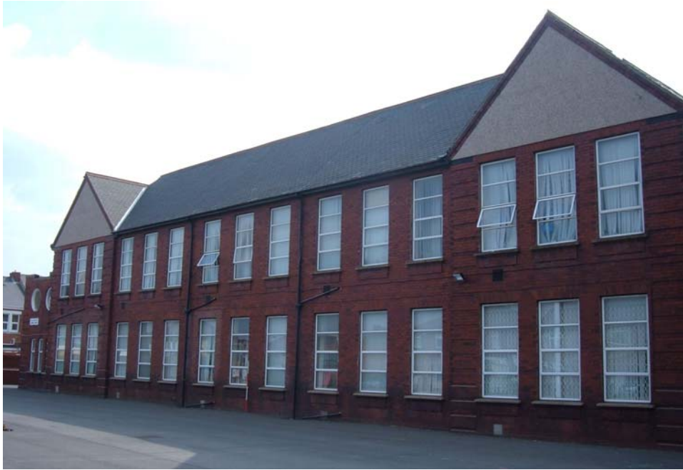
Plate 1. Main building, east elevation, from the north-east ( 2m scale ).
