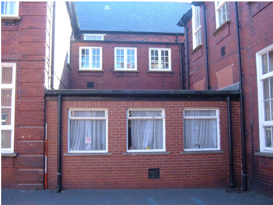
Plate 10. Main building, central range (north), west elevation and hall block, north elevation (east end), from the north-west (2m scale).
