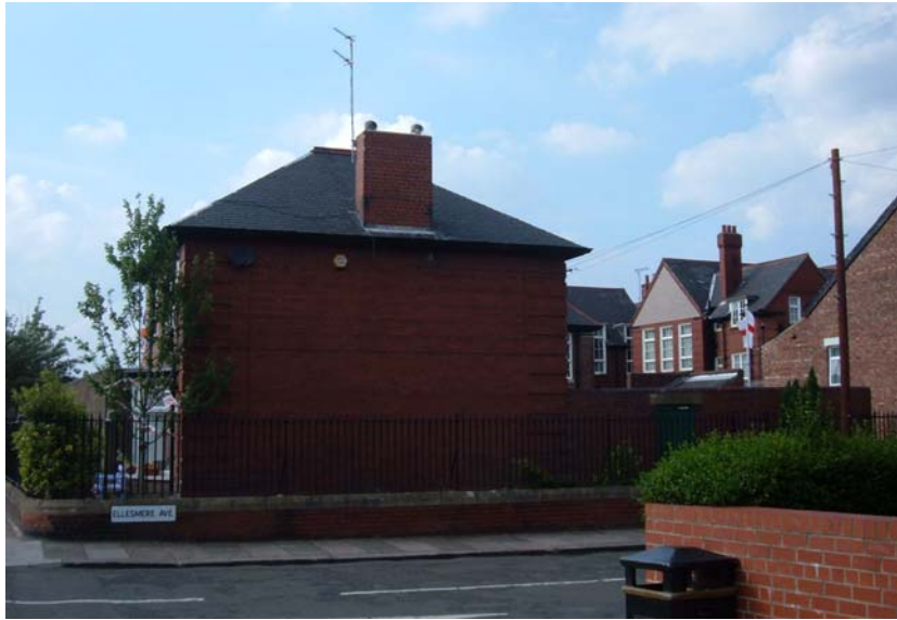
Plate 41. Caretaker's house, south elevation, from the south.
