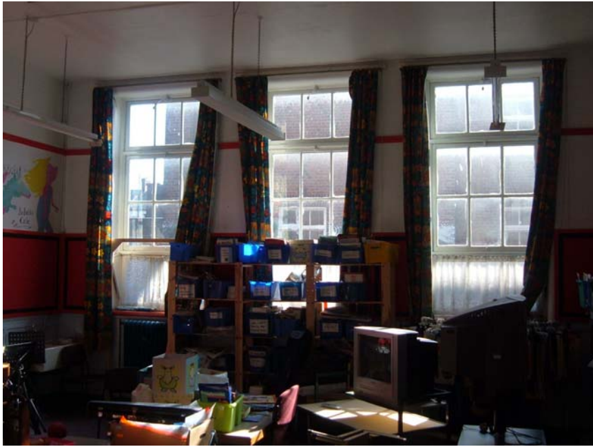
Plate 45. Main building, ground floor, south wing, western classroom, from the north-east.
