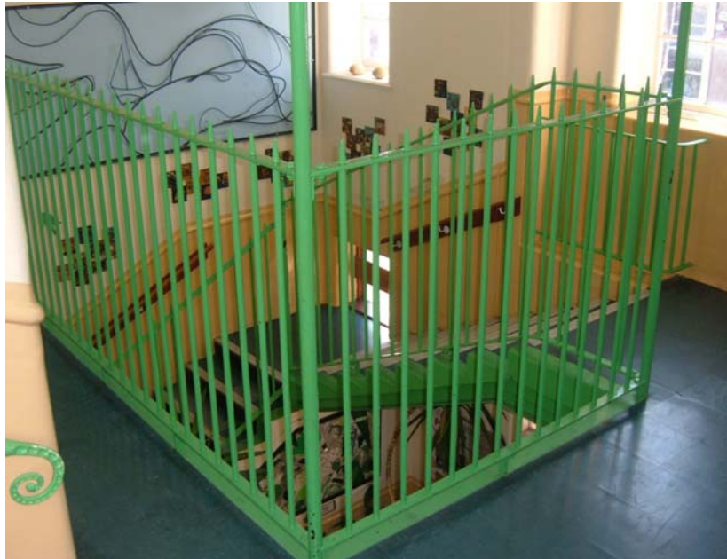
Plate 47. Main building, first floor (north end), detail of staircase, from the south-east.
