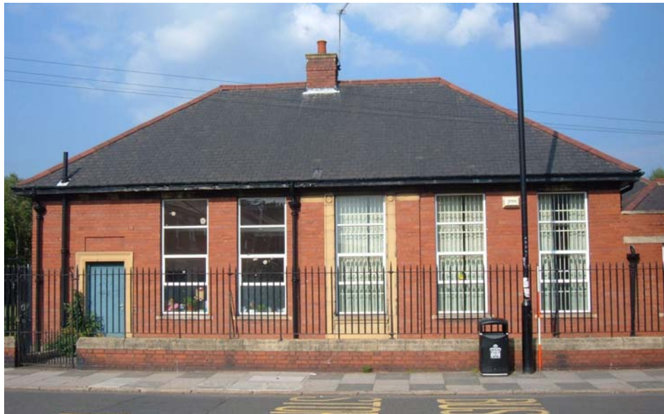
Plate 32. Former infants' block, west wing, west elevation, from the south-west (2m scale).
