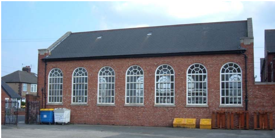
Plate 16. Gym block, north elevation, from the north-west.
