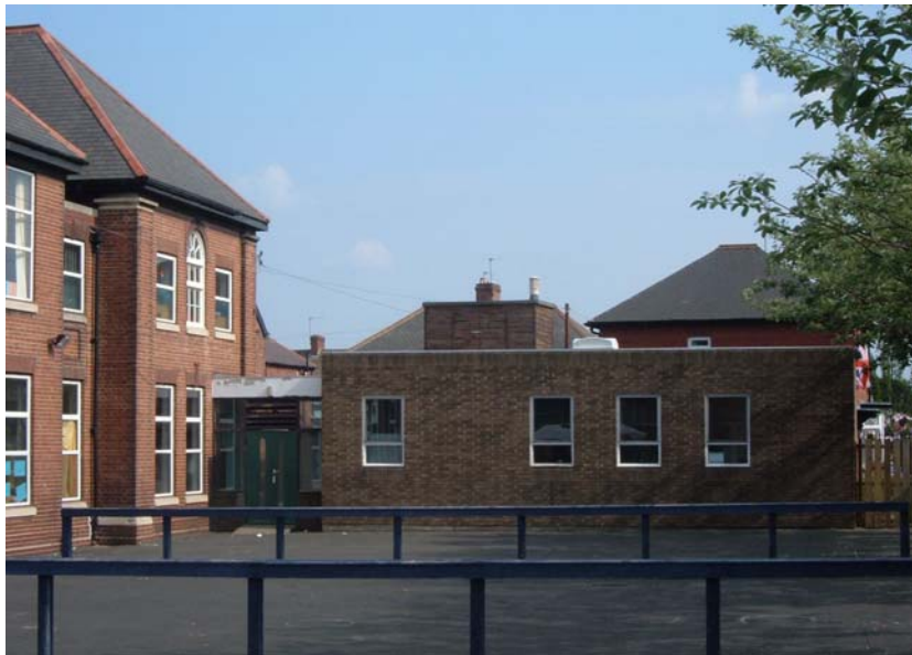
Plate 42. Kitchen block, north elevation, from the north-west.
