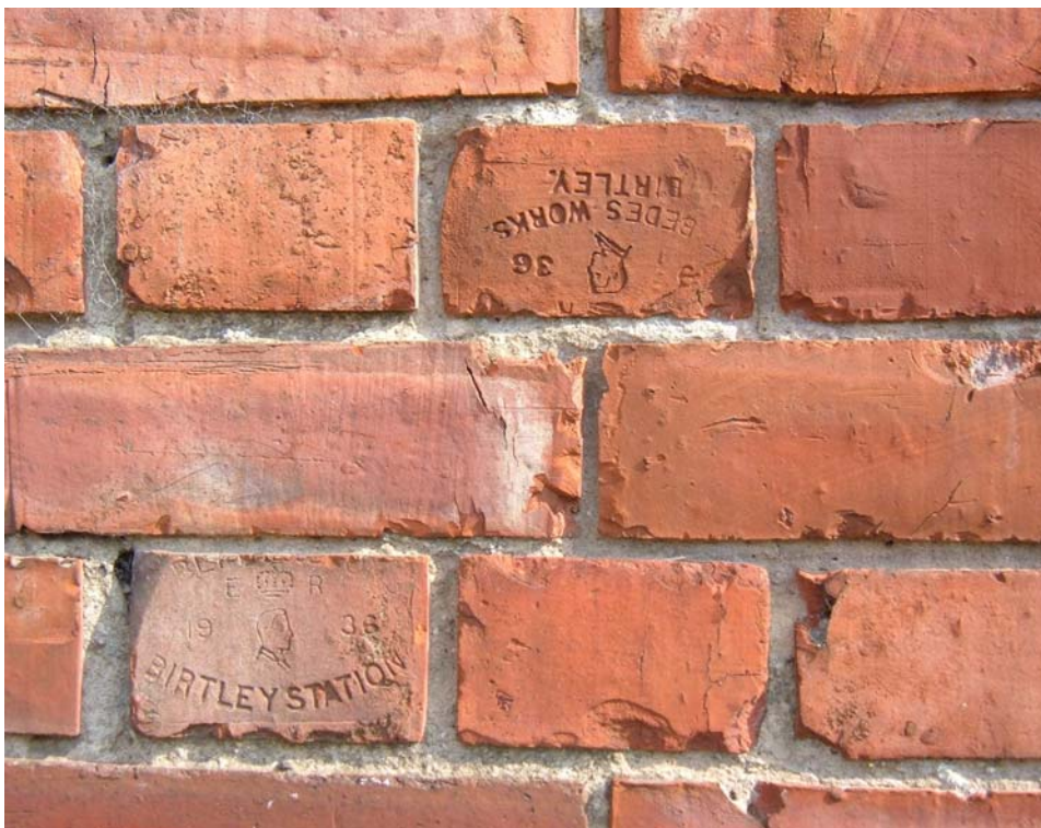
Plate 18. Gym block, north elevation (west end), detail of brick stamps, from the north.
