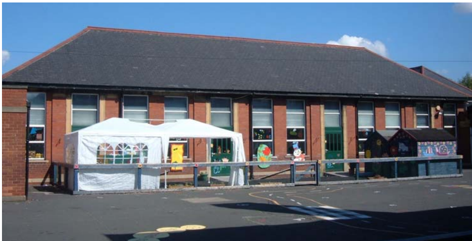
Plate 28. Former infants' block, central range, south elevation, from the south.
