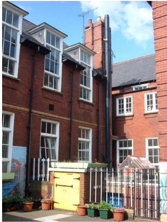
Plate 7. Main building, central range (south), west elevation and hall block, south elevation (east end), from the south-west (2m scale).
