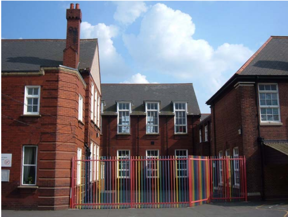
Plate 9. Main building, hall block, north elevation (west end), from the north-west (2m scale).
