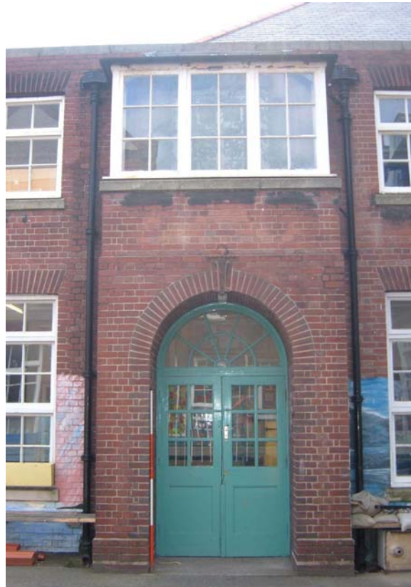
Plate 25. Former secondary modern block, central range, south entrance in west elevation, from the north-east (2m scale).
