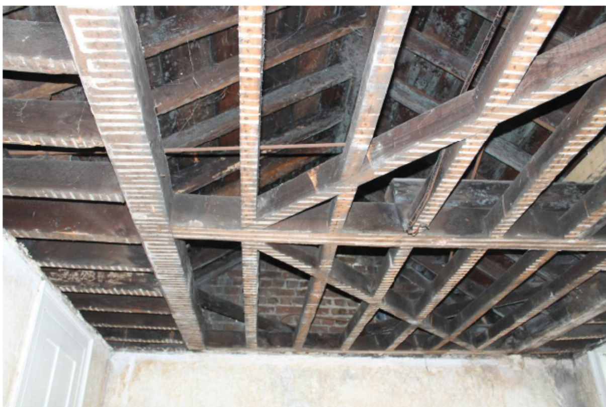
Plate 57 Fully-framed second floor ceiling joists and roof structure, looking north
