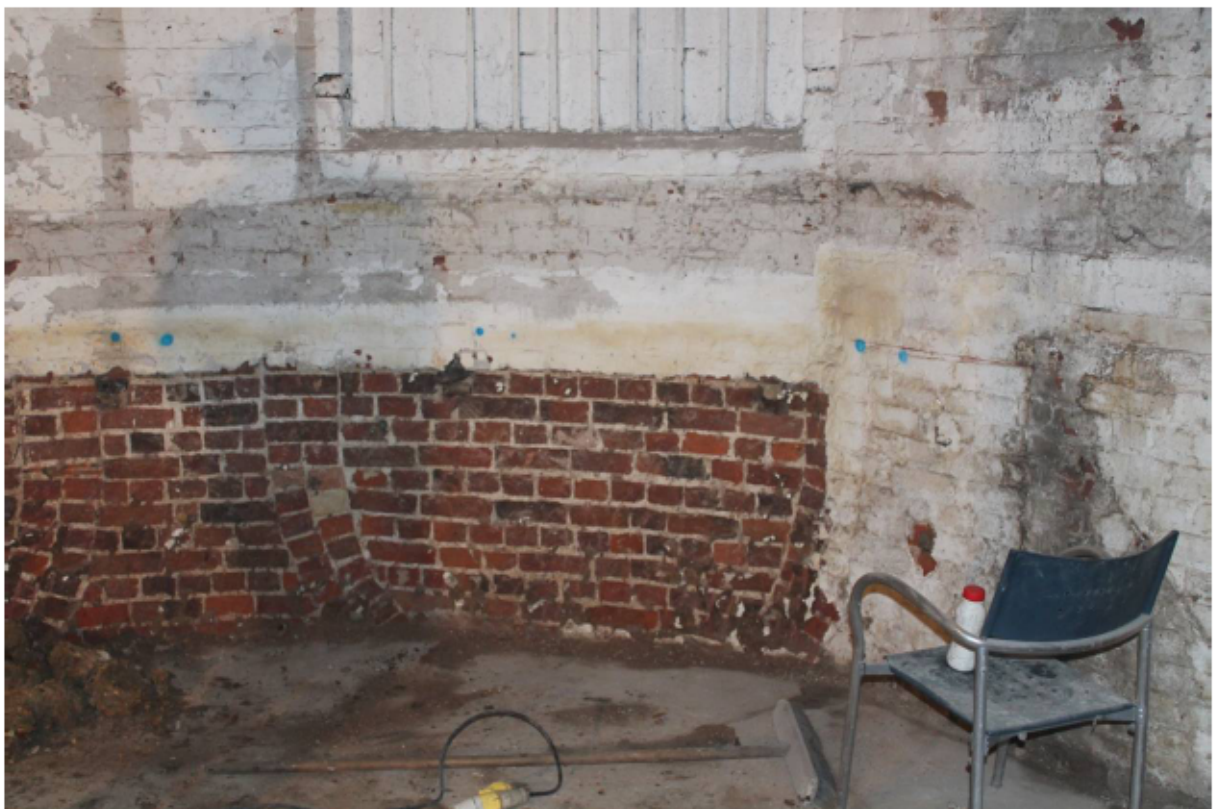
Plate 55 Reverse arch of below window in Basement (B17), looking south-east
