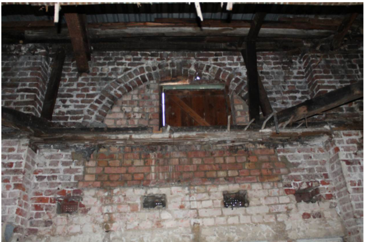
Plate 53 Blocked arched opening in the east wall of the Billiard Room (G23), looking east
