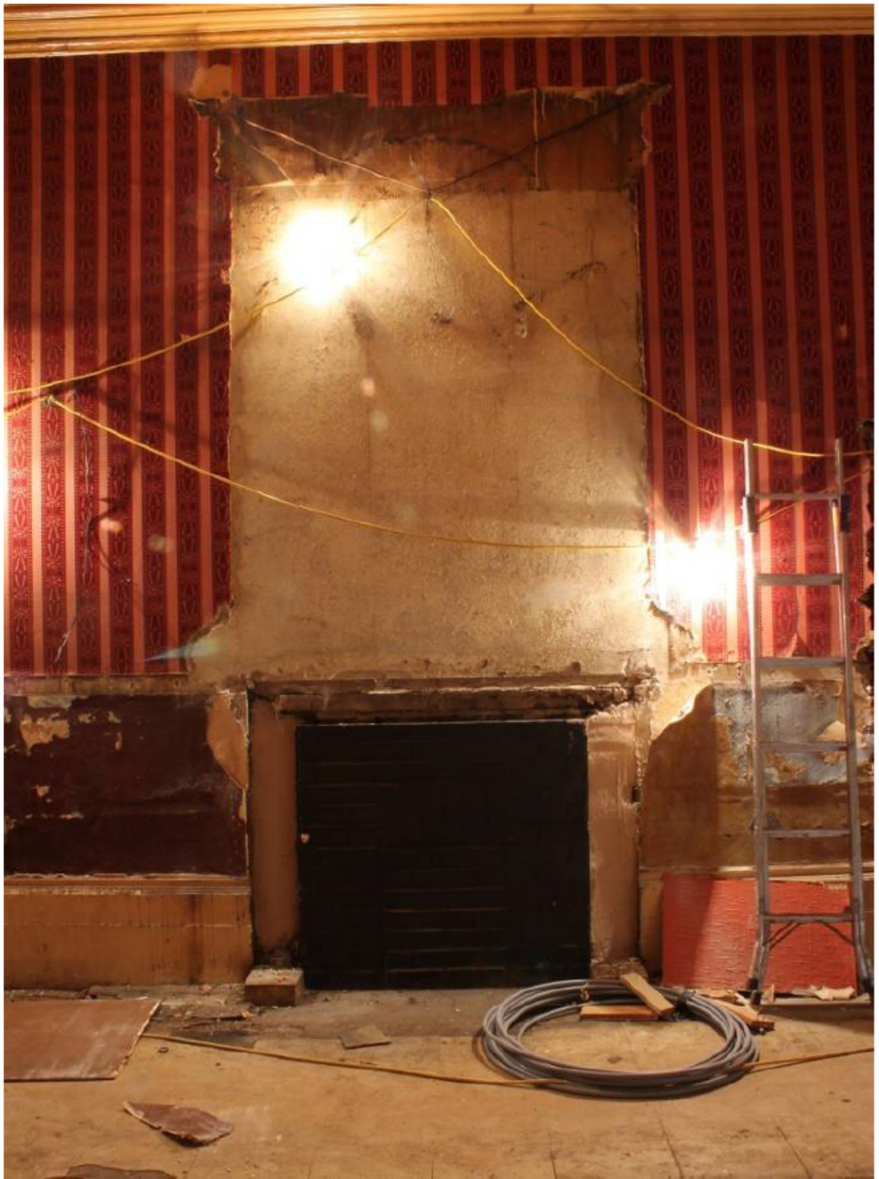
Plate 16 Scar of fireplace and overmantle in Withdrawing Room (G4), looking south
