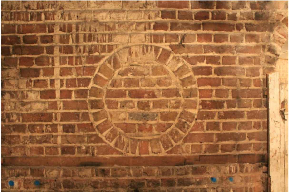
Plate 54 One of two blocked circular windows in (B17), looking west
