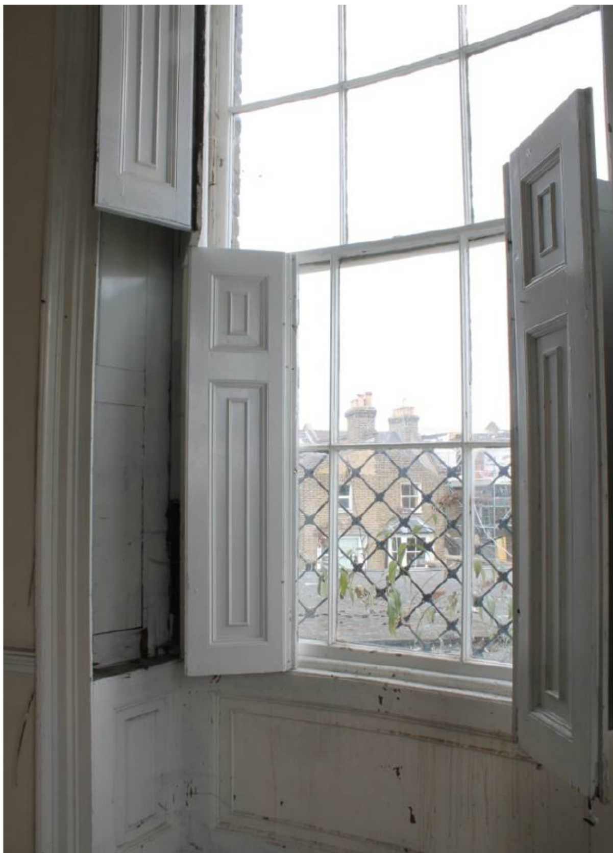
Plate 22 Sash window shutters in (F6), looking north-east
