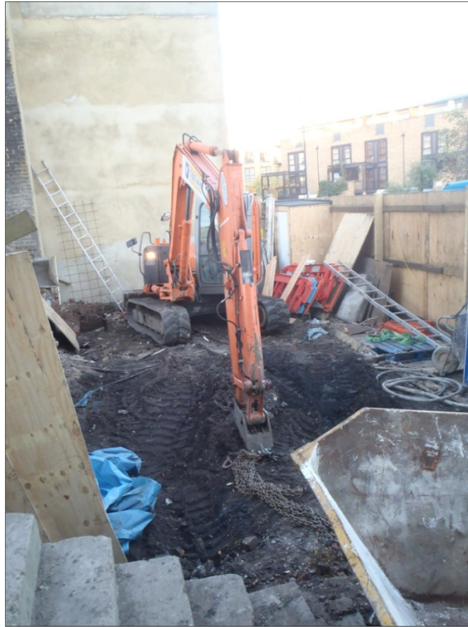
Plate 1: Northern Area Before Excavation, Looking West
