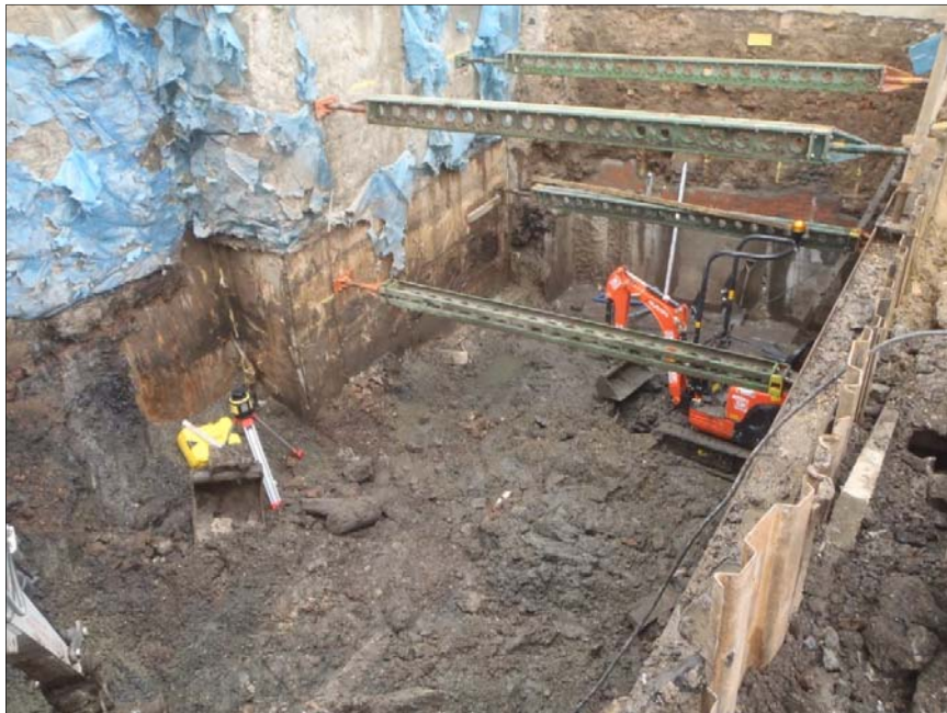
Plate 2: Northern Area Excavated to Full Depth, Looking South-West
