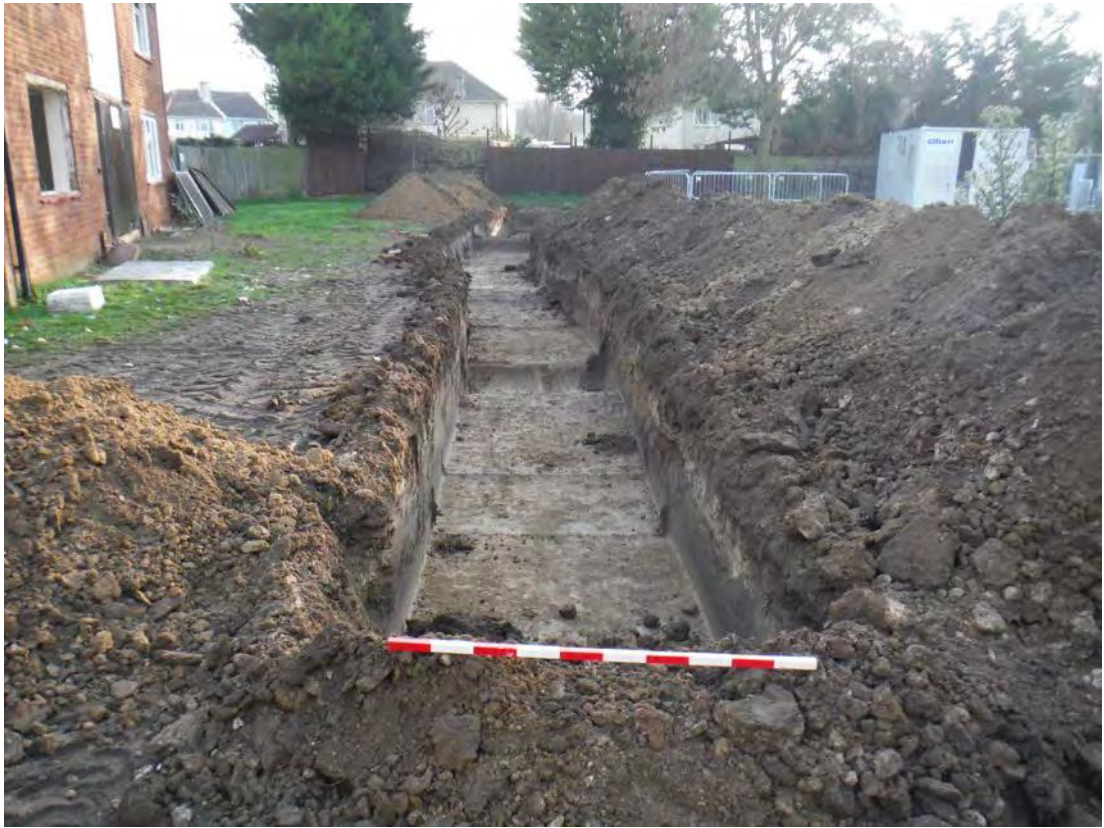
Plate: 1. Shot of Trench 1, taken from north.
