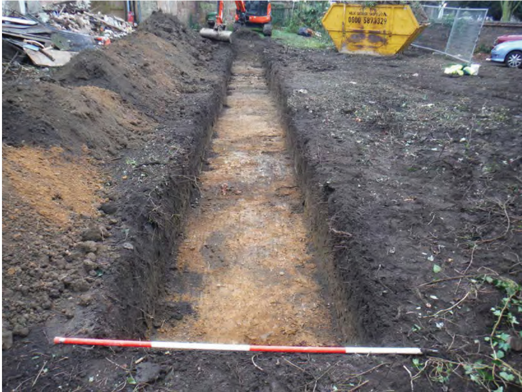
Plate 1. Shot of Trench, taken from the north.
