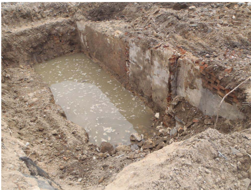
Plate 2: Basement Exposed during watching Brief, Looking South-West
