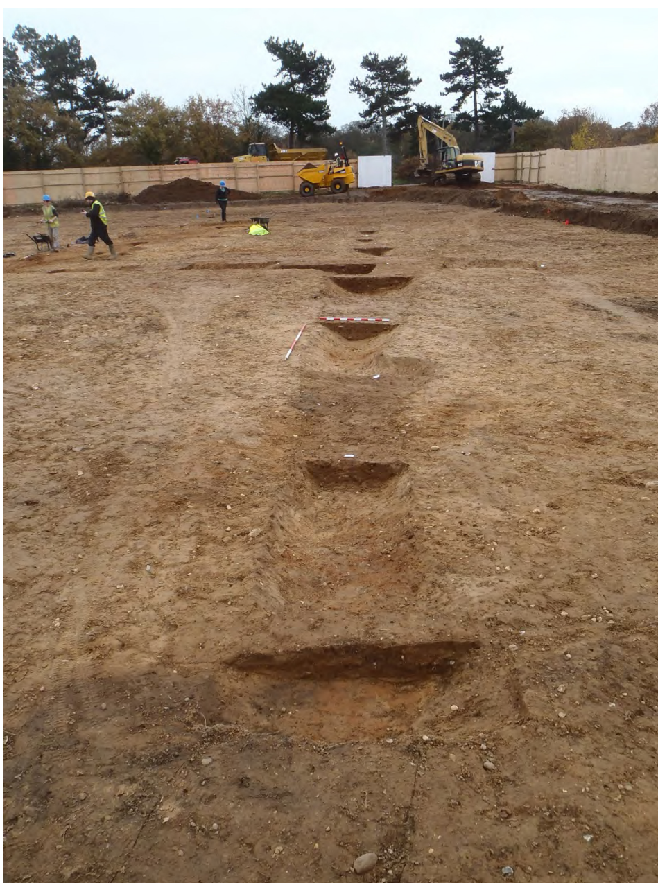
Plate 10: DITCH 8, south end, view south
