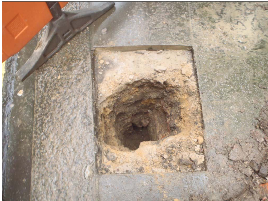
Plate 6: Wall footing [22] exposed in north of BH2, Looking west
