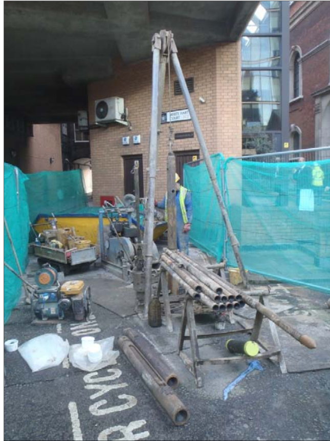
Plate 3: Coring BH1, Looking east
