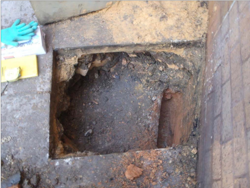
Plate 1: Surface of concrete [4] in TP1, Looking north
