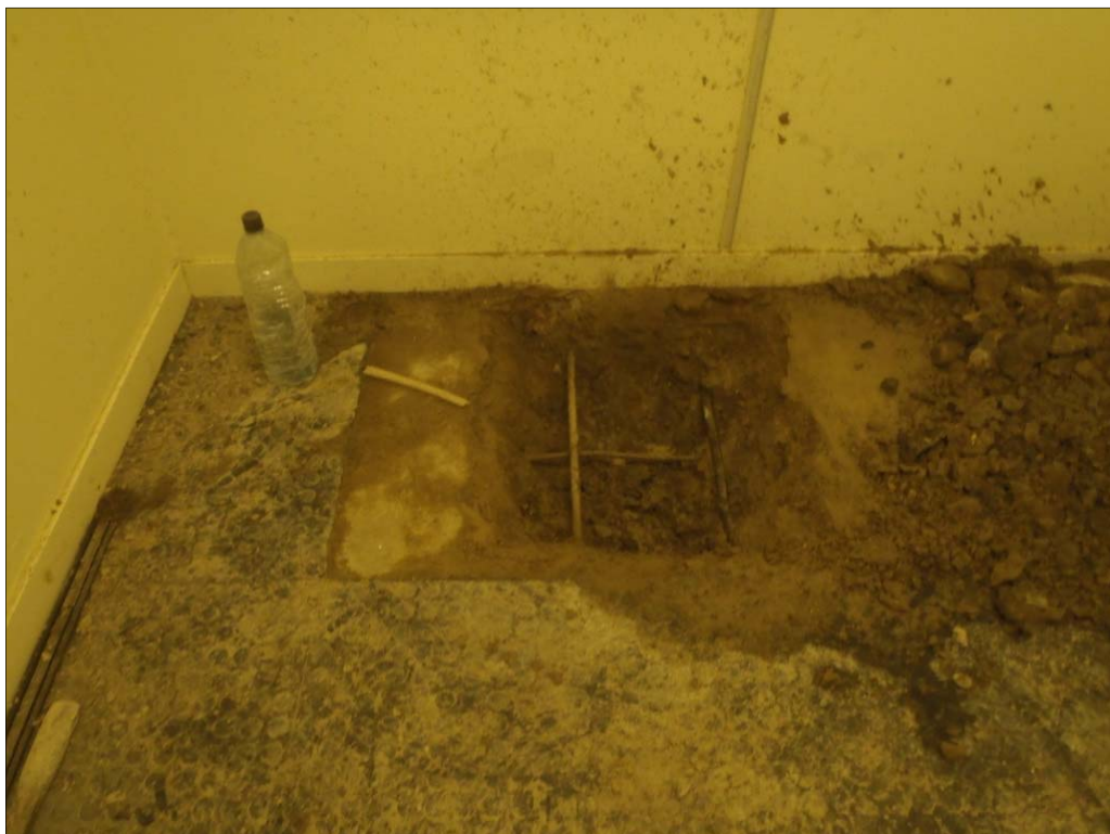
Plate 2: Rebars in basement slab [7], TP3, Looking North
