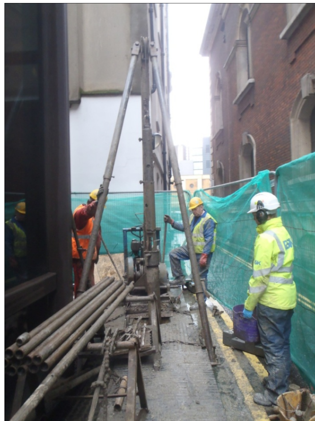
Plate 4: Coring BH2, Looking east
