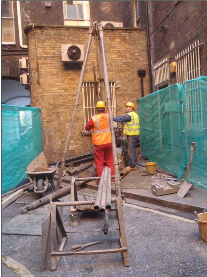
Plate 5: Coring BH3, Looking east
