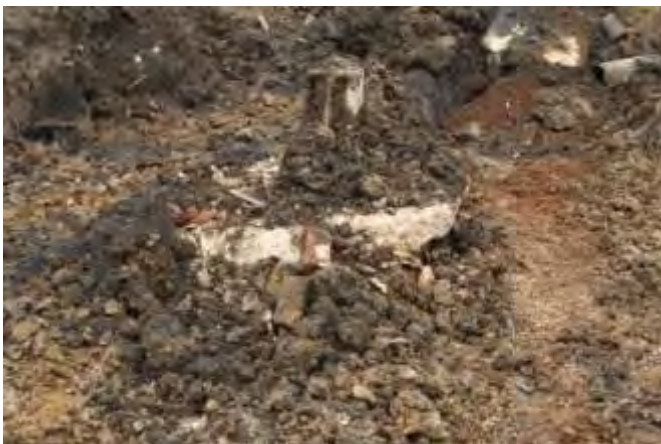
Plate 2 Concrete turntable base, central section.
