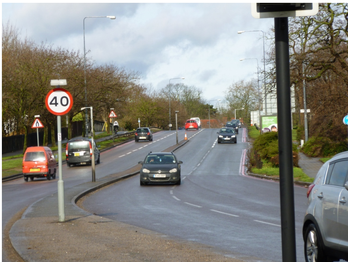
Plate 1: Rise in the embankment carrying Gunnersbury Avenue (A406) towards the bridge over the railway bridge, looking north from the Chiswick Roundabout
