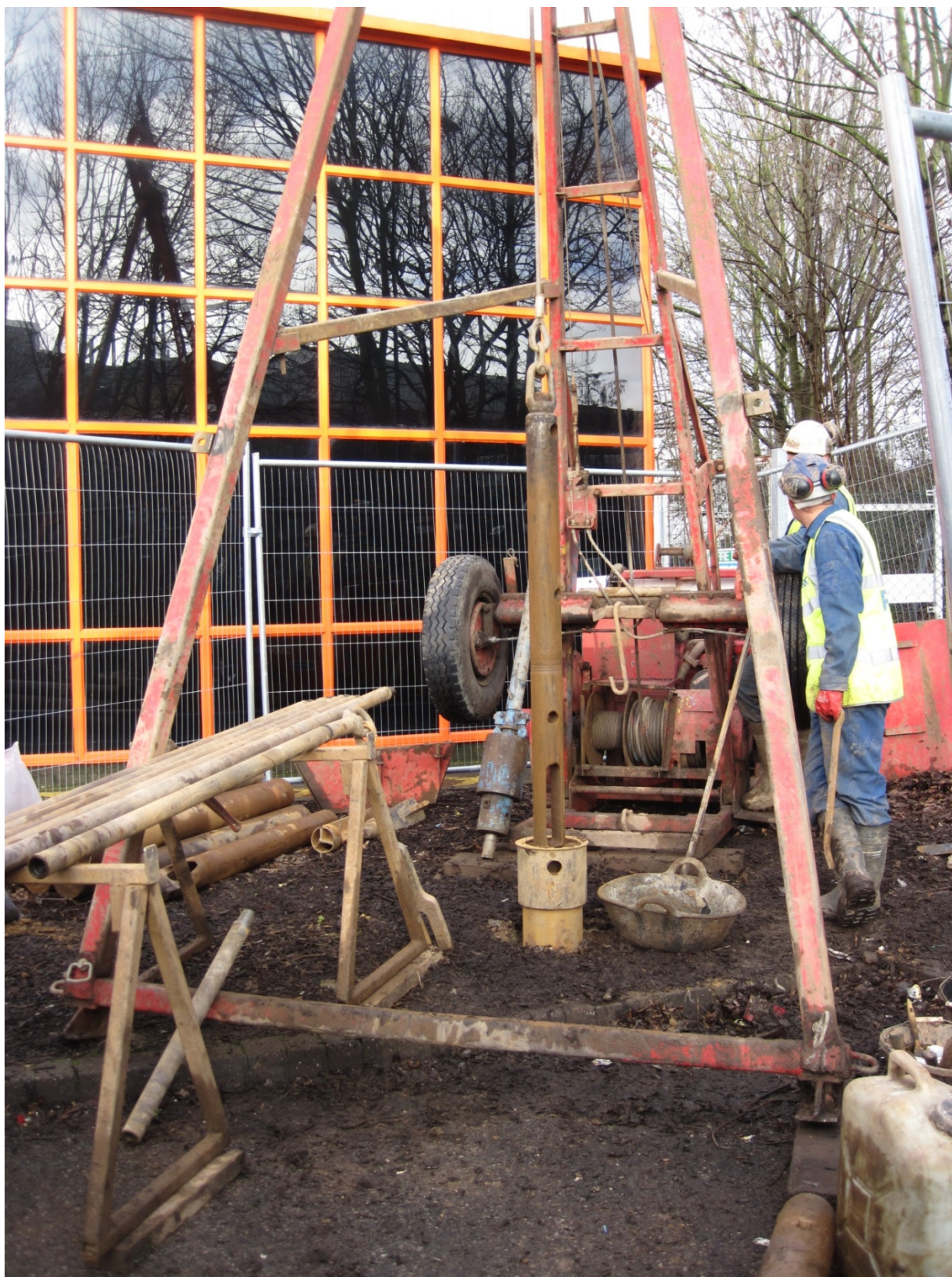
Plate 6. Percussion borehole BH102, looking north-east
