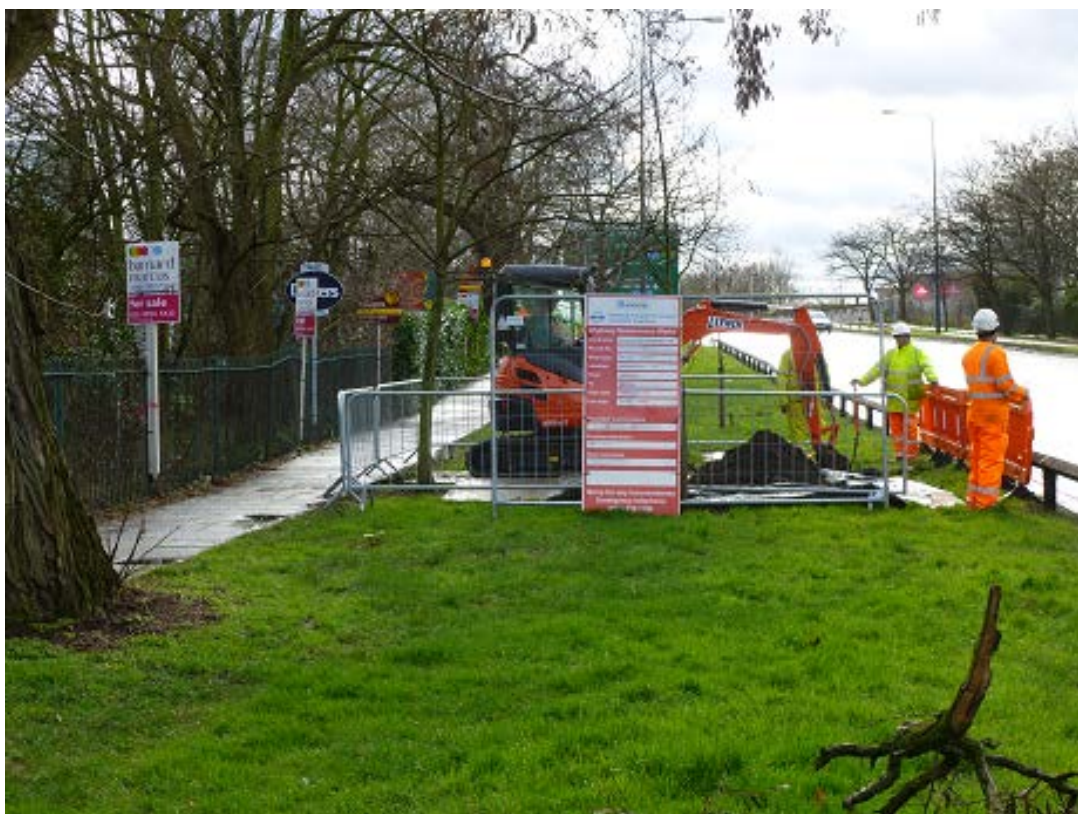
Plate 9: Trench ST07, looking south
