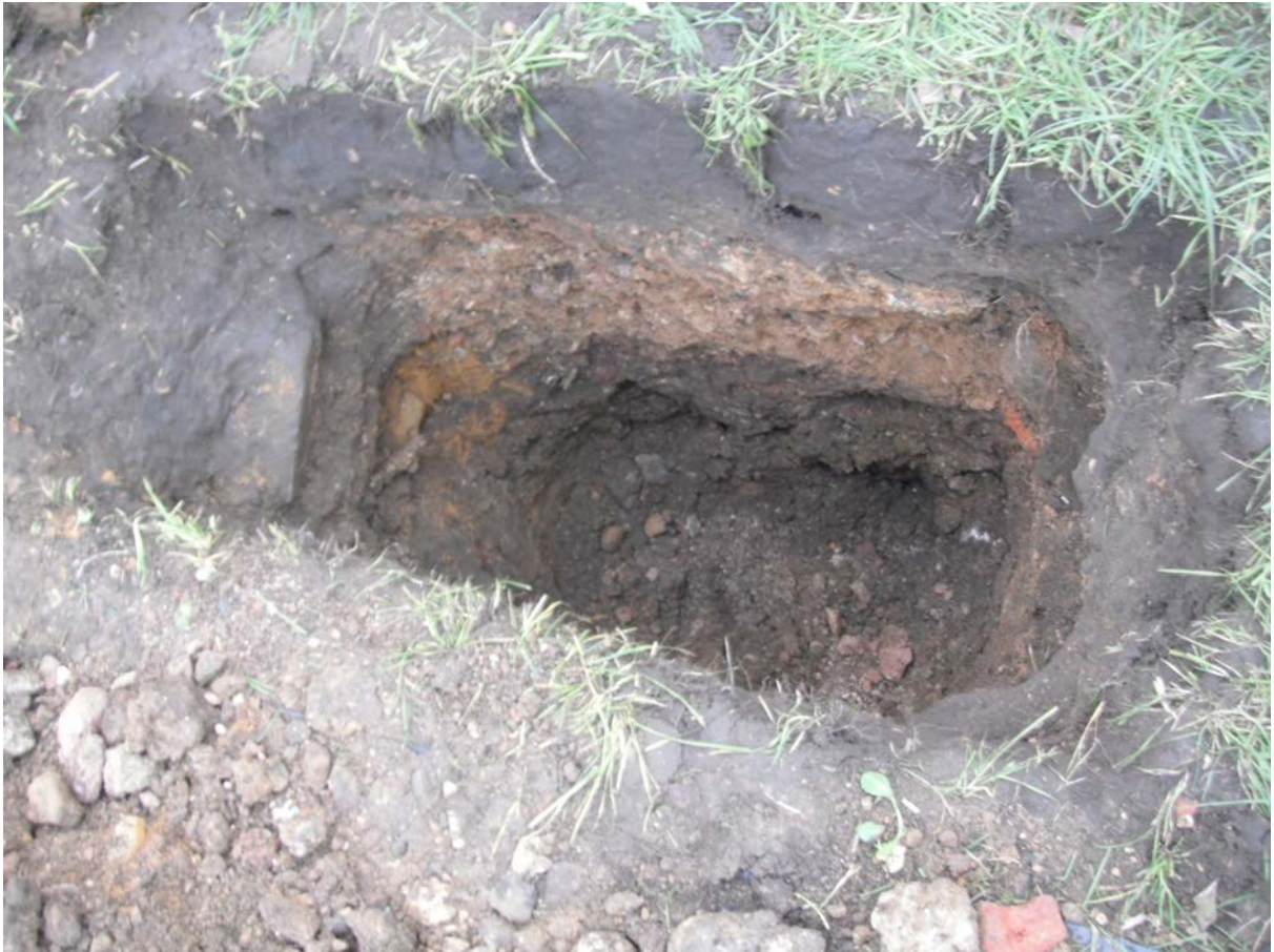
Plate 5. Window sample WS02 during excavation
