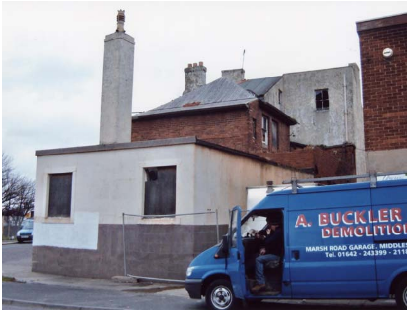
Plate 9. The Rose & Crown, south and east elevations, from the south-east.
