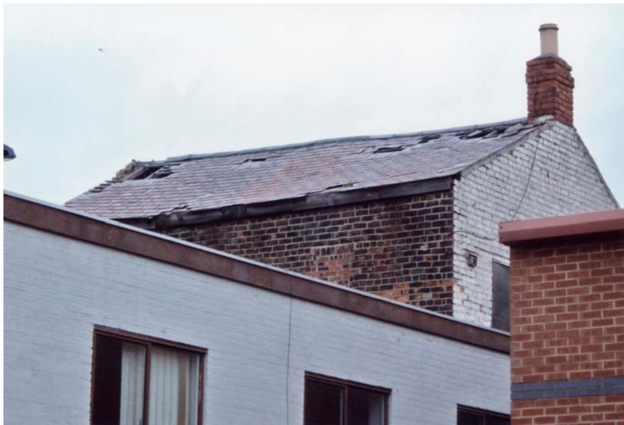
Plate 12. 6 Walker Road, south elevation, from the south-east.
