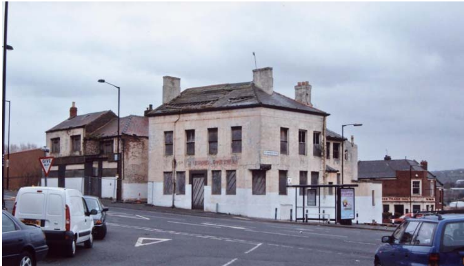
Plate 2. The Rose & Crown and 4 & 6 Walker Road, from the north-west.
