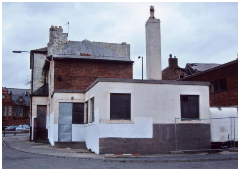
Plate 8. The Rose & Crown and 4 Walker Road, south elevations, from the south ( 2m scale ).
