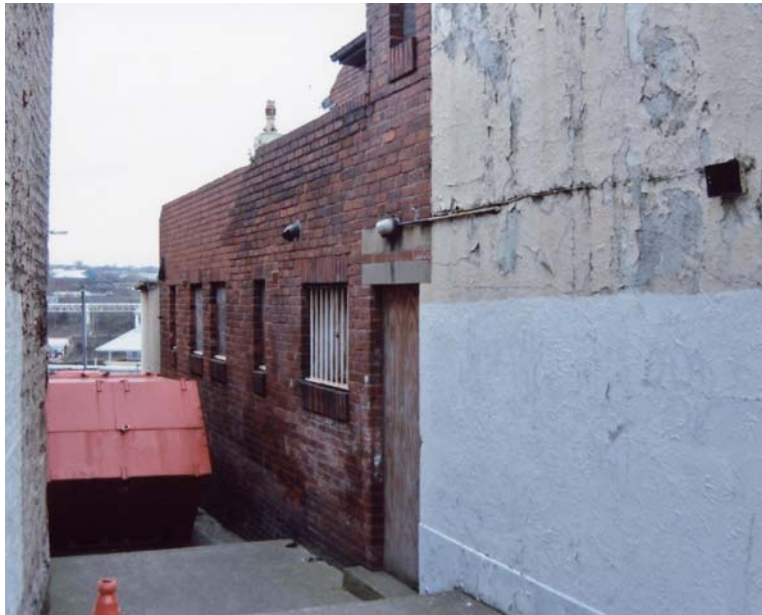
Plate 13. The Rose & Crown, east elevations, lower section, from the north-east.
