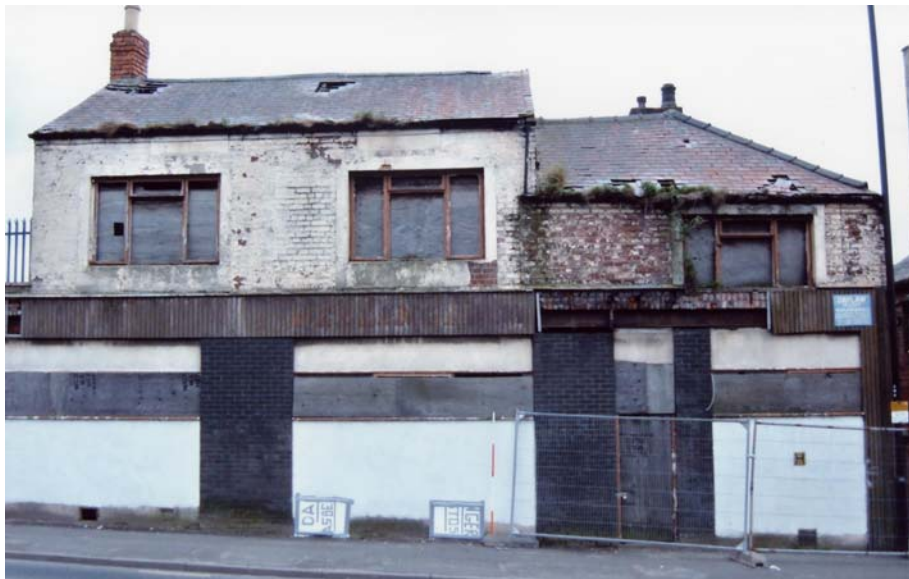
Plate 11. 4 & 6 Walker Road, north elevation, from the north (2m scale).
