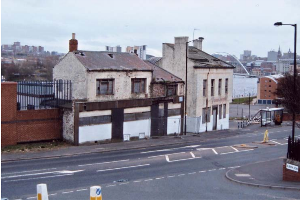
Plate 1. The Rose & Crown and 4 & 6 Walker Road, from the north-east.
