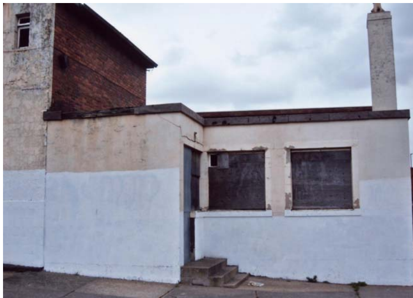
Plate 6. The Rose & Crown, rear buildings, west elevation, from the west.
