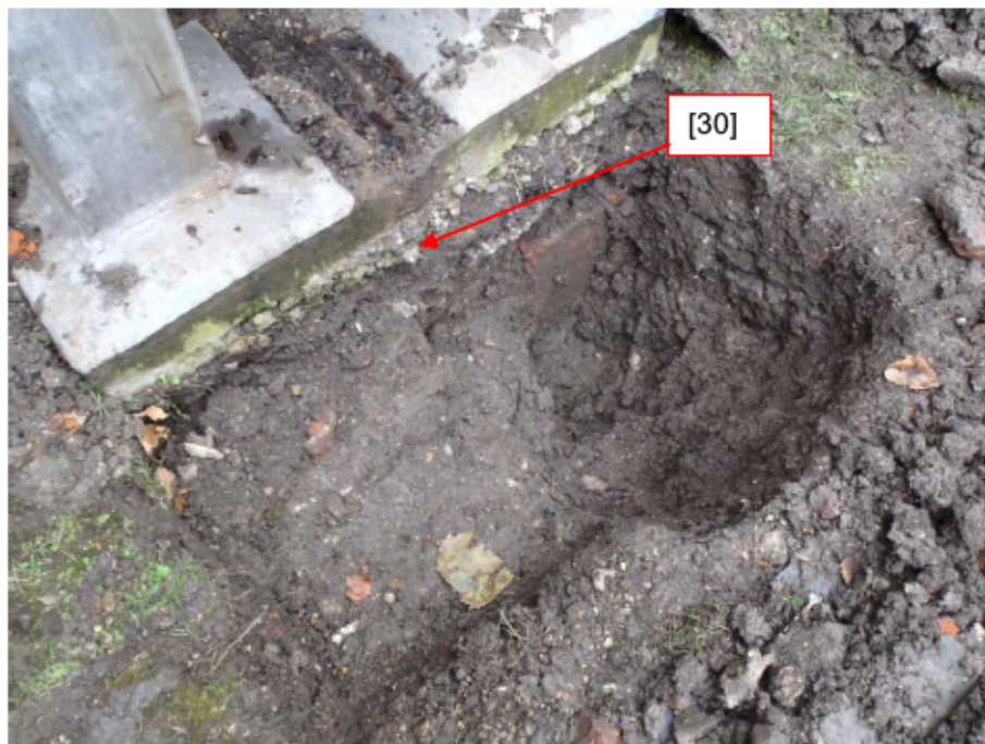
Plate 3: View north-west within Test Pit 6 showing brick footing [30] beneath footing of the extant 1915 bridge.
