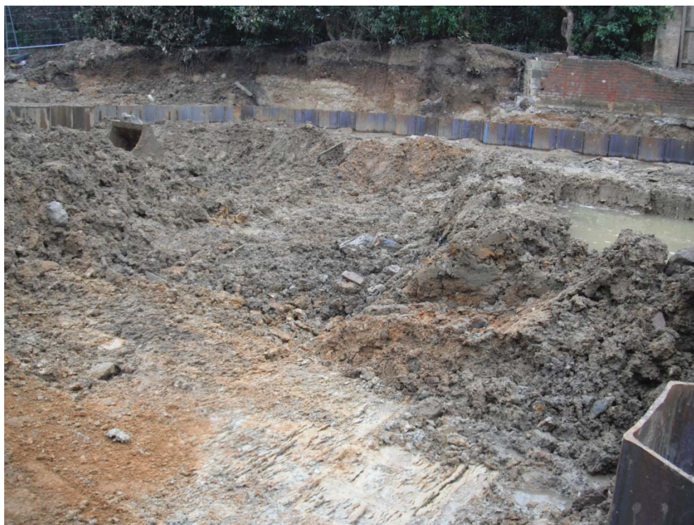
Plate 4: Site conditions, looking S
