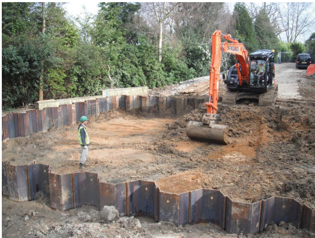
Plate 2: Excavation in progress, deposits reduced with grading bucket, looking E
