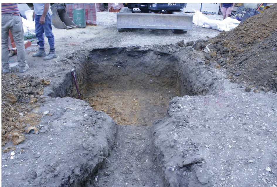
Plate 16: Excavation of the soakaway pit, view east
