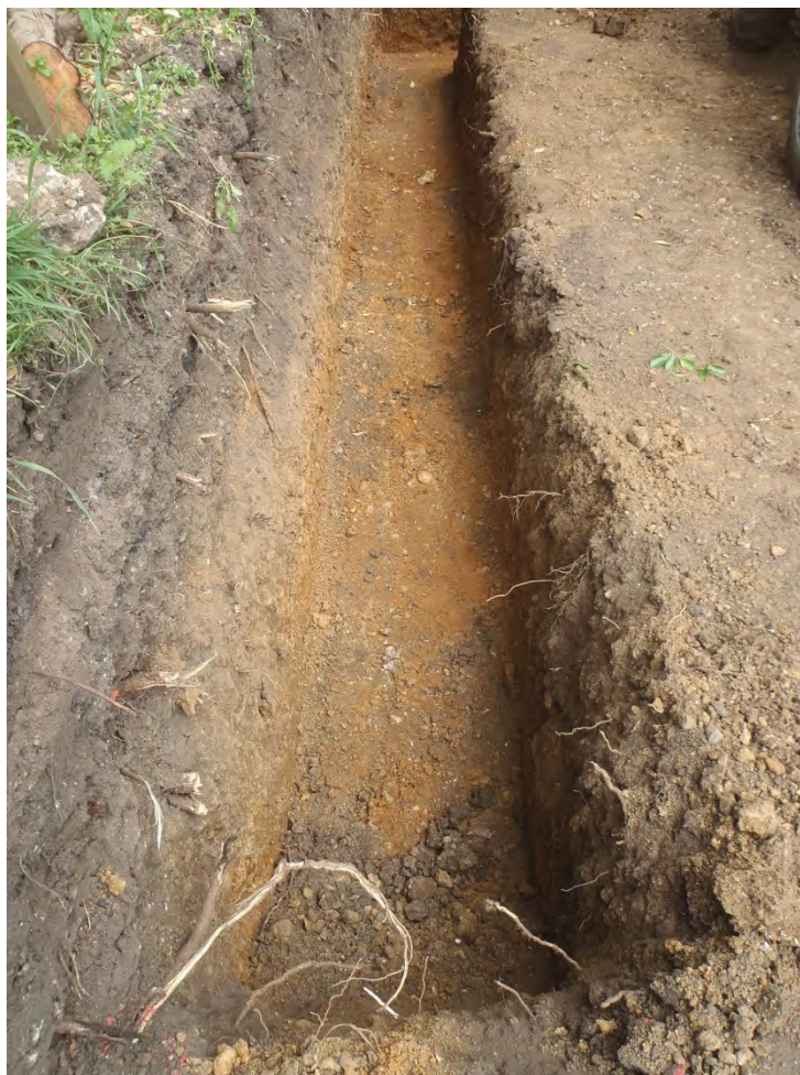
Plate 15: The footings for the garage, view north
