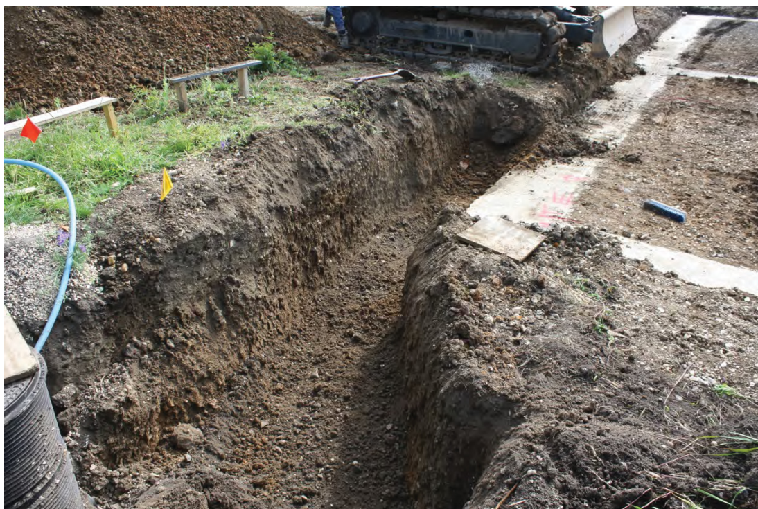
Plate 17: Service trench, view north-east
