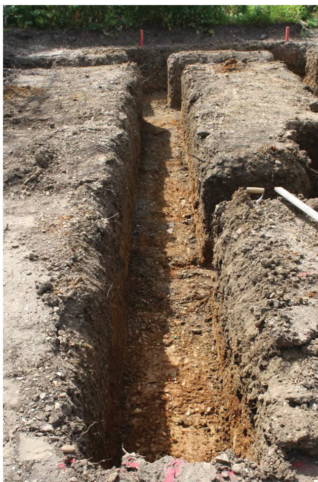
Plate 14: The footings for 21A, view west
