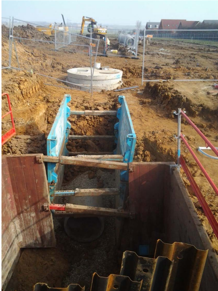
Plate 5: Pipe trenching in area of section 8 (see Figure 2)
