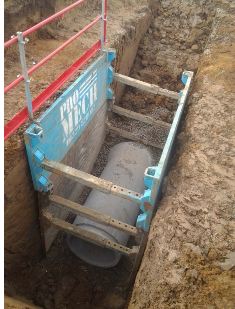
Plate 6: Pipe trenching in area of section 10 (see Figure 2)
