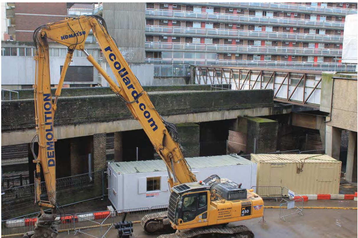
Plate 4: Length of the viaduct rebuilt in the 1920s with concrete beam and 1980s link bridge to multi-storey car park, looking south-south-west
