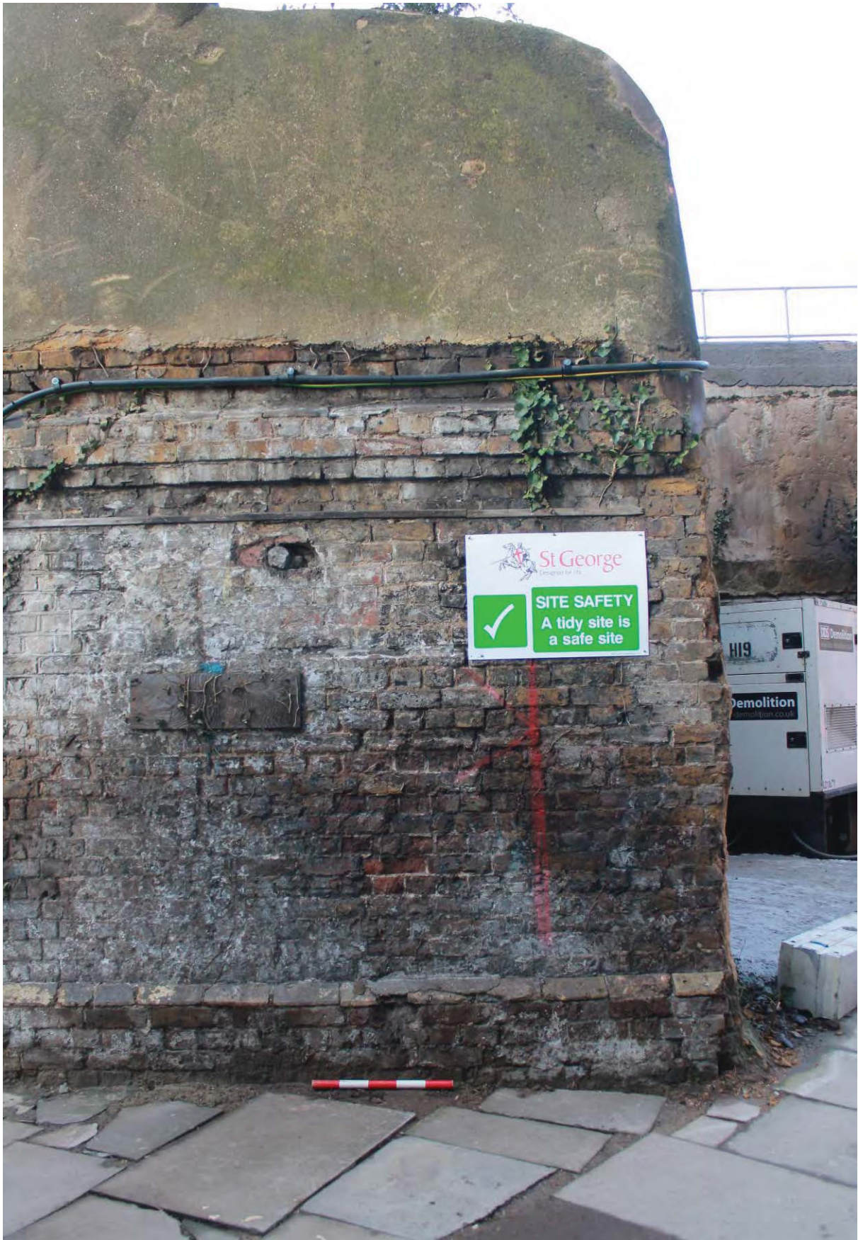
Plate 7: North-east facing end elevation of the viaduct, looking south-west
