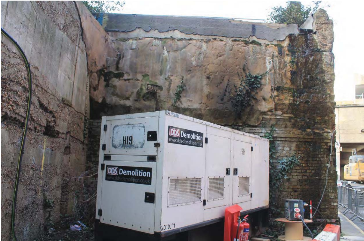
Plate 10: Cut back, part rendered eastern facing elevation, looking west-south-west
