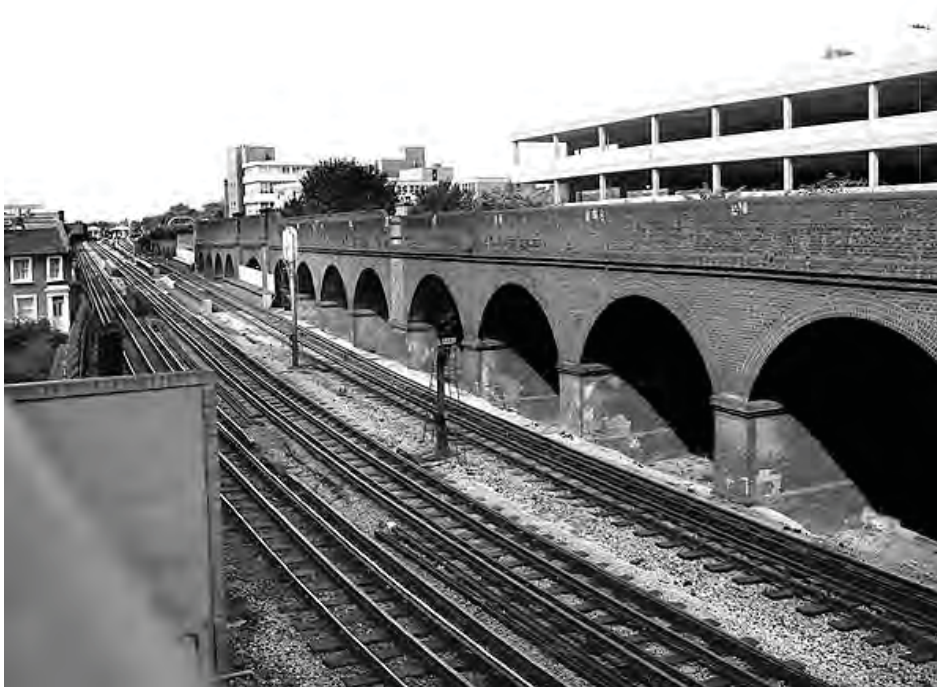
Plate B: Photograph taken in 1980 showing the 1869 viaduct, looking west with the Kings Mall Car Park behind (north)
