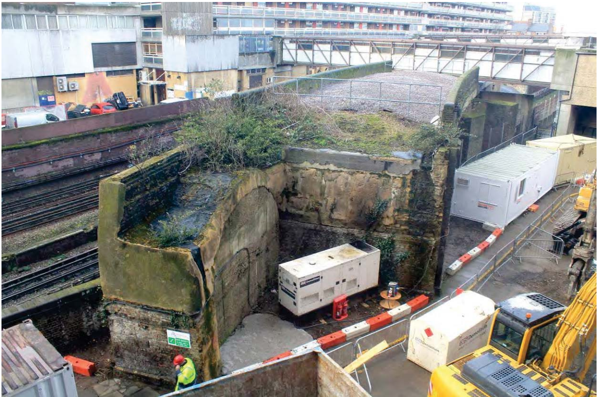
Plate 2: Remains of the viaduct within the site, looking south-west
