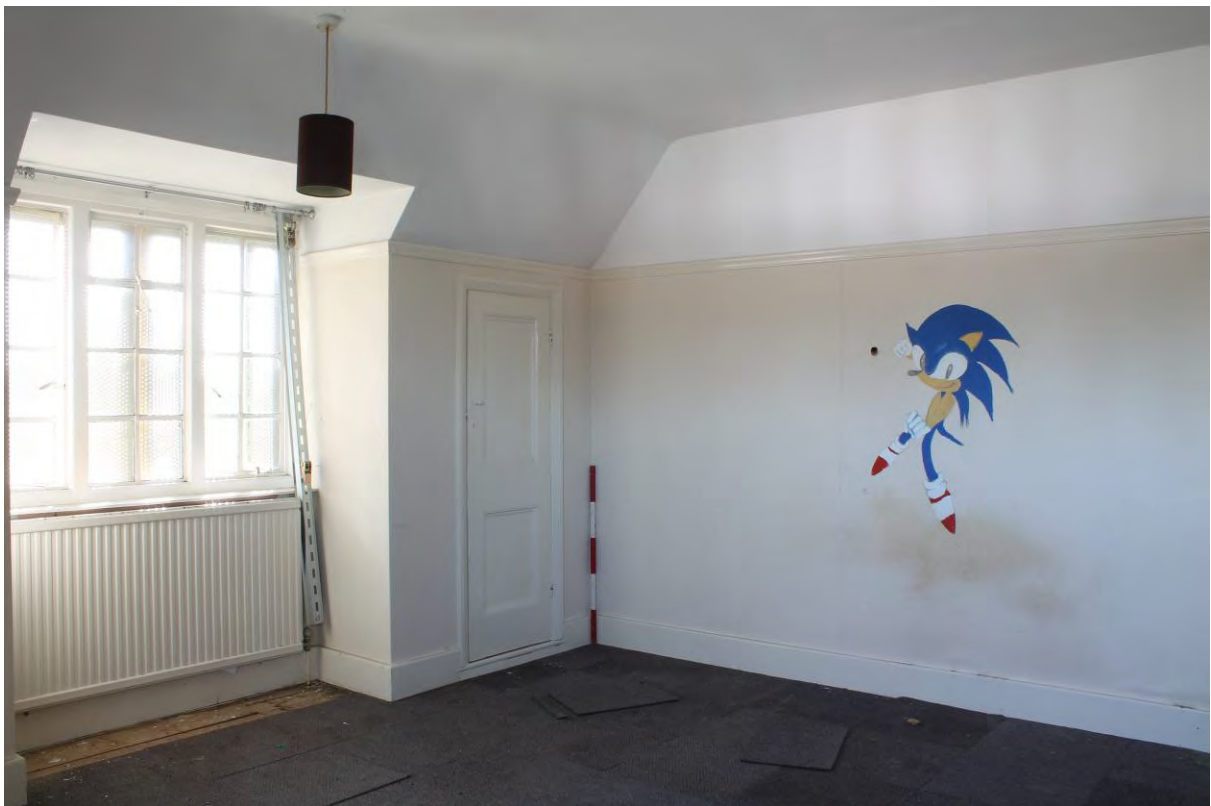
Plate 22 Bedroom FF2 showing under eaves cupboard, looking South-west
