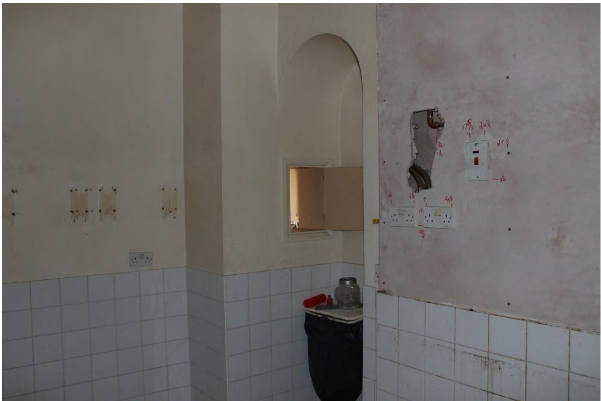
Plate 18 Kitchen, showing food hatch to Public Bar
