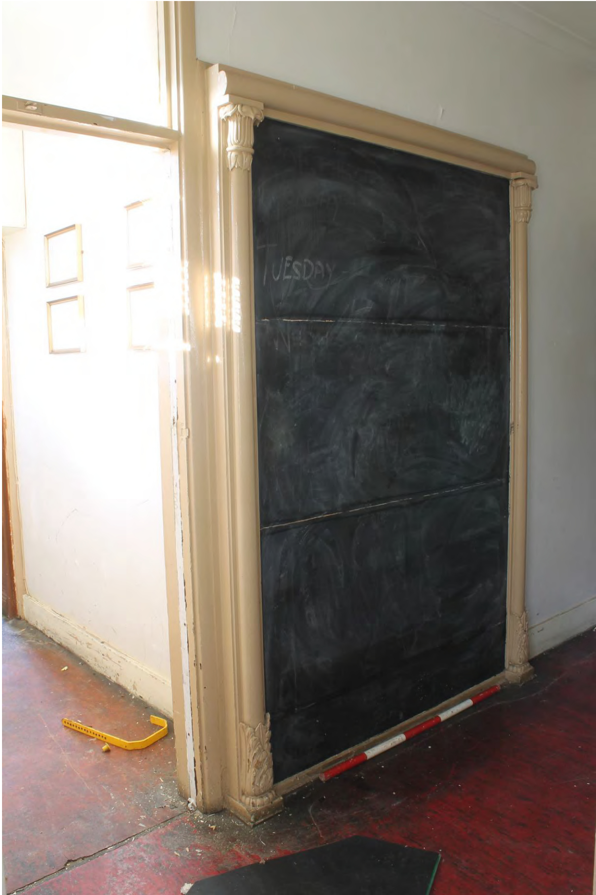
Plate 16 Ornate Blackboard to former Tea Room (now within rear corridor to WCs)
