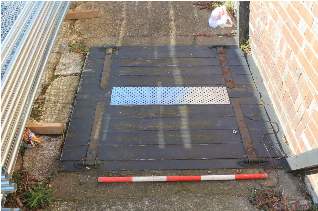
Plate 4 Barrel Drop to Cellar along Southern Elevation
