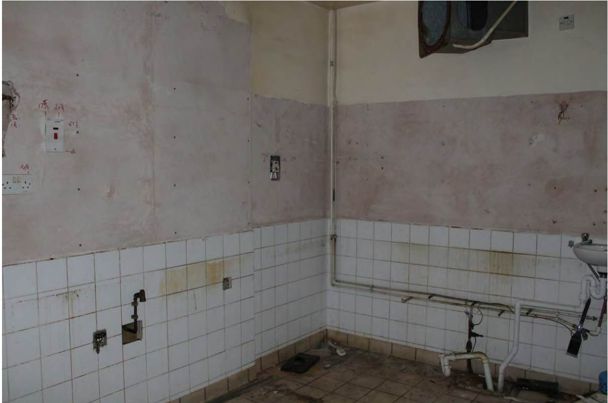
Plate 17 Kitchen looking East
