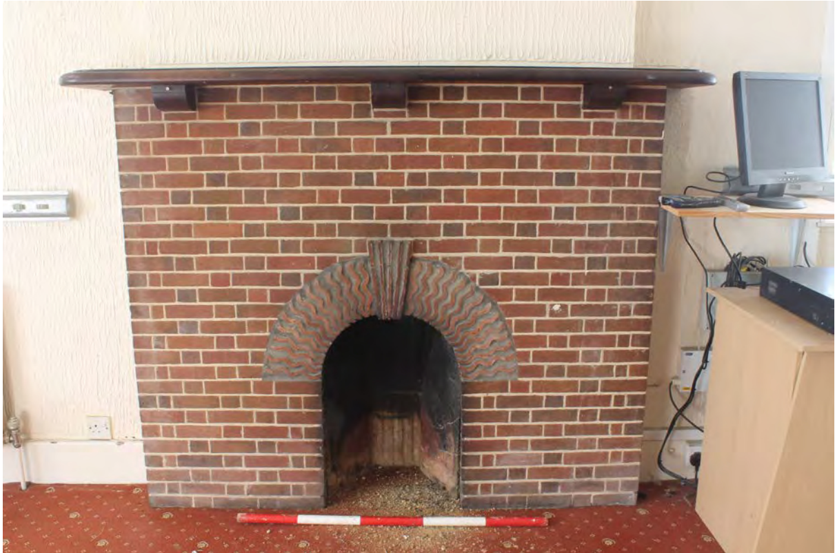
Plate 21 Detail of Fireplace in FF1
