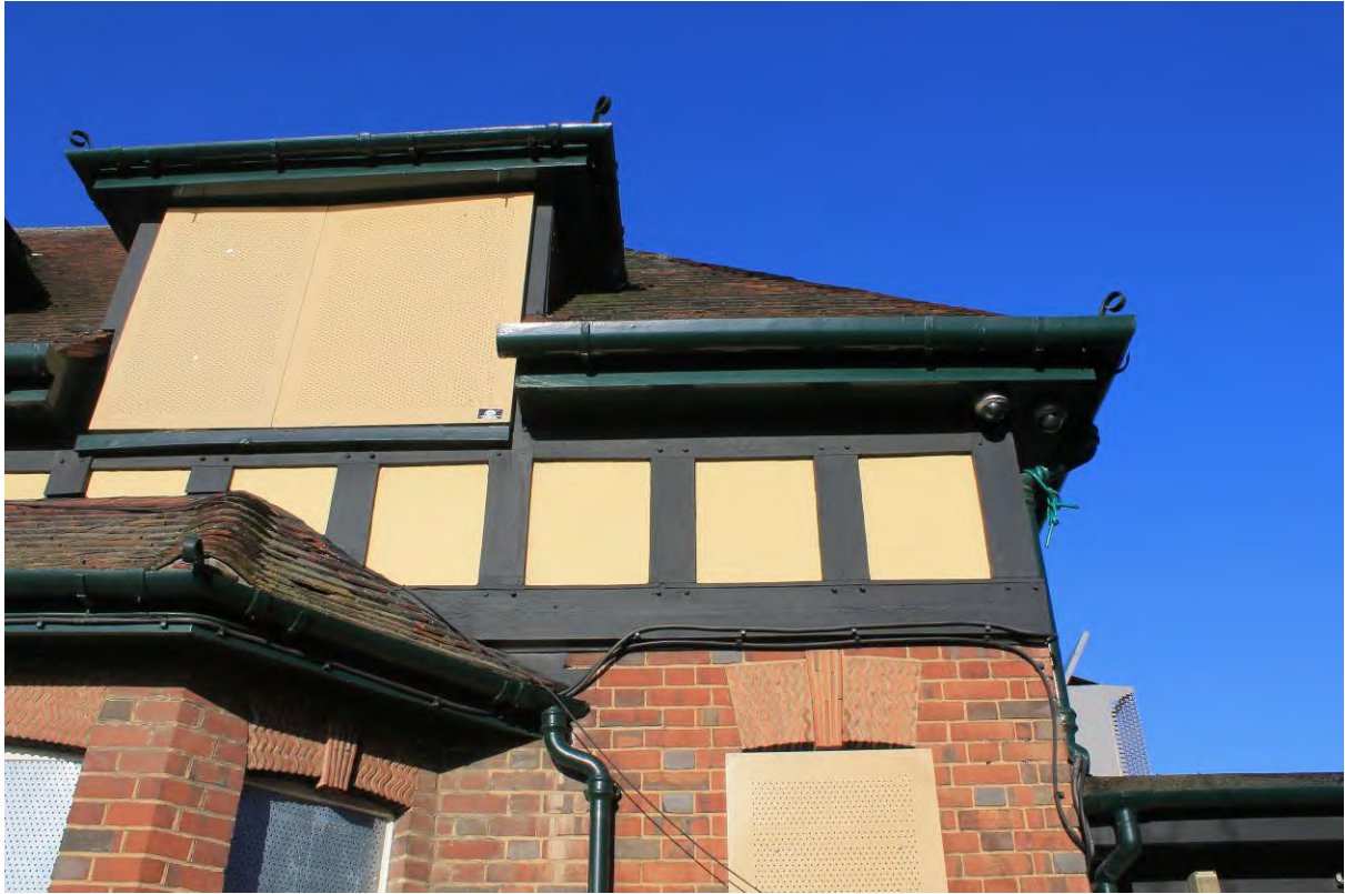
Plate 3 Architectural Detail to South Elevation
