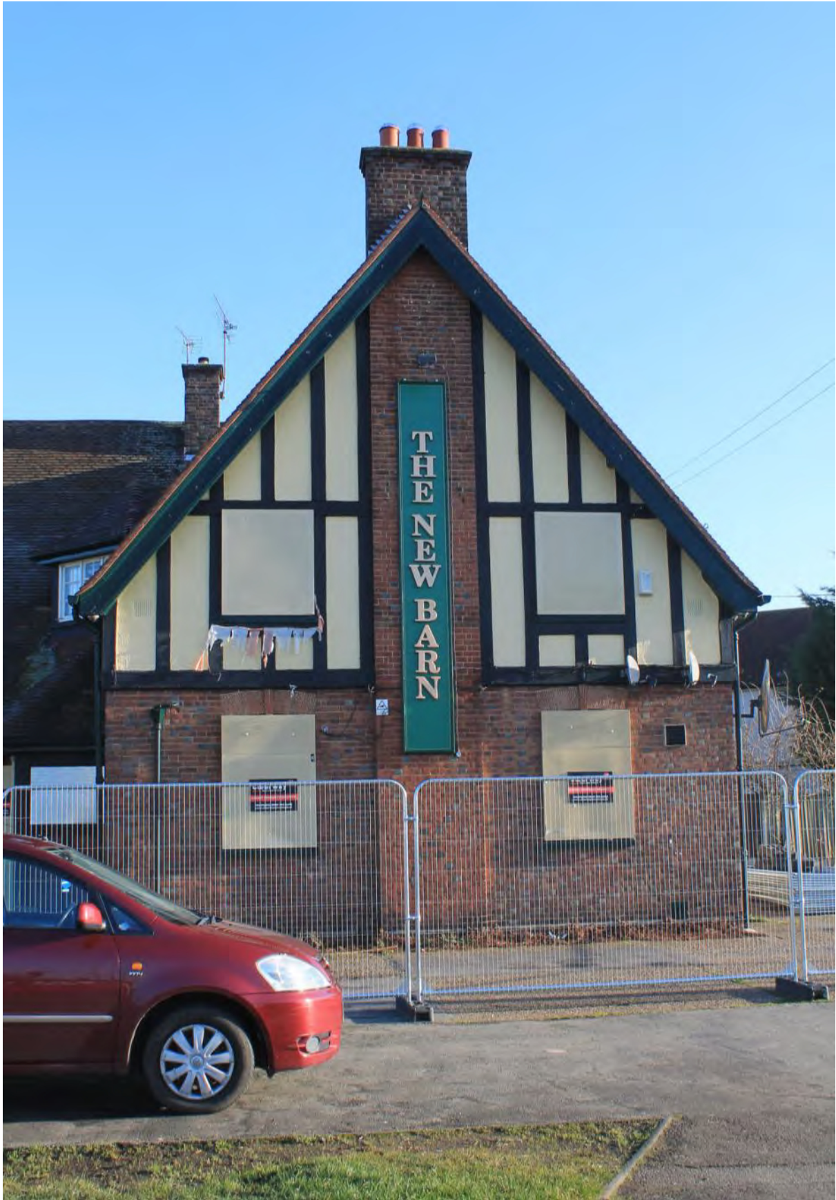
Plate 5 The New Barn, Western Gable Elevation
