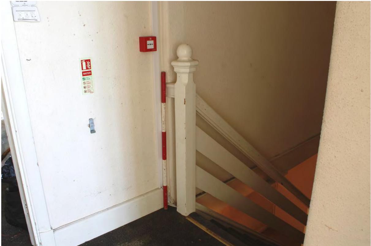
Plate 19 First Floor Landing Stair Newel Post
