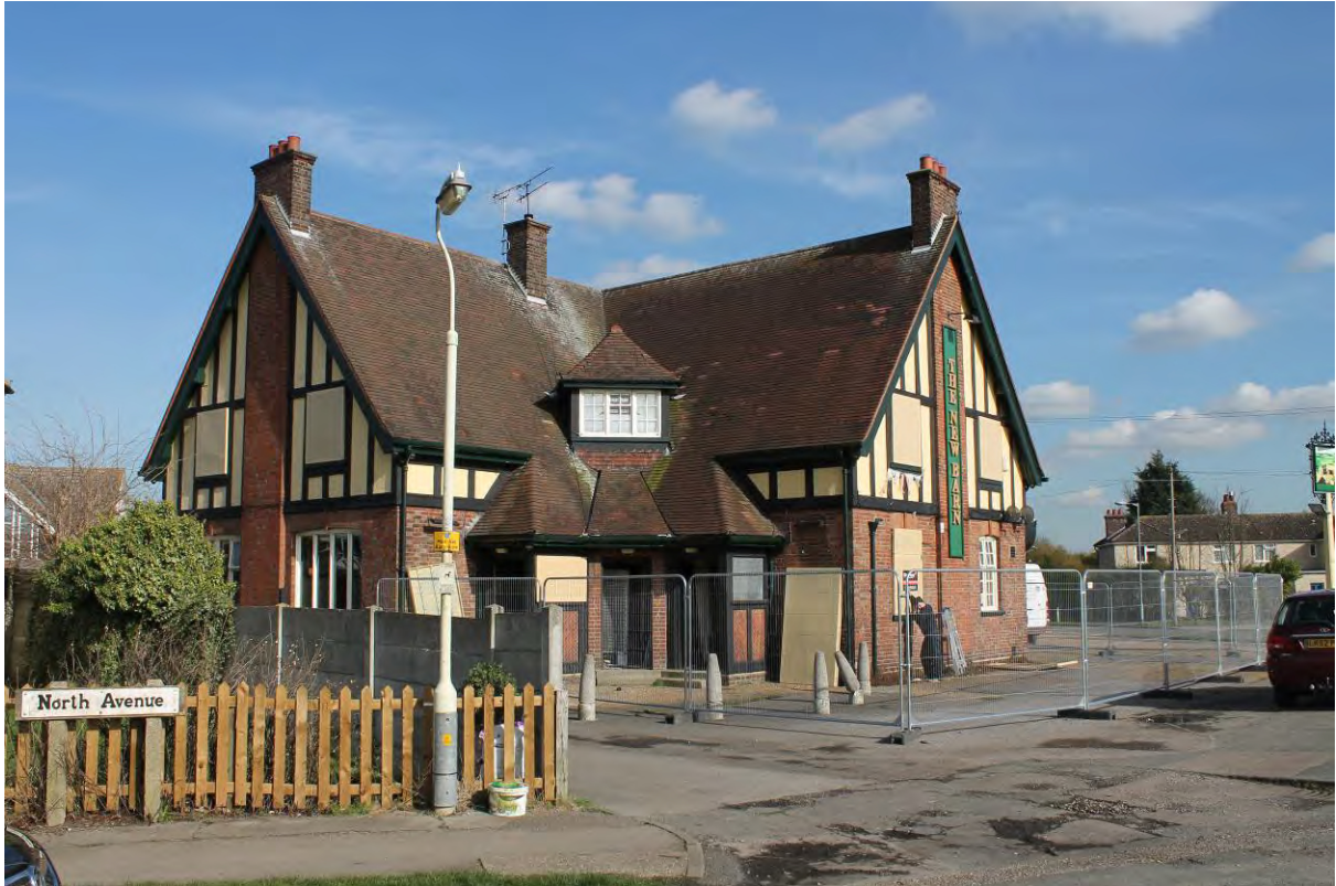
Plate 6 The New Barn North and Western Elevations, looking South-east
