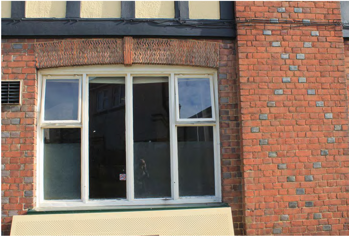
Plate 8 Detail of Window to Public Bar and Diaperwork, North Elevation
