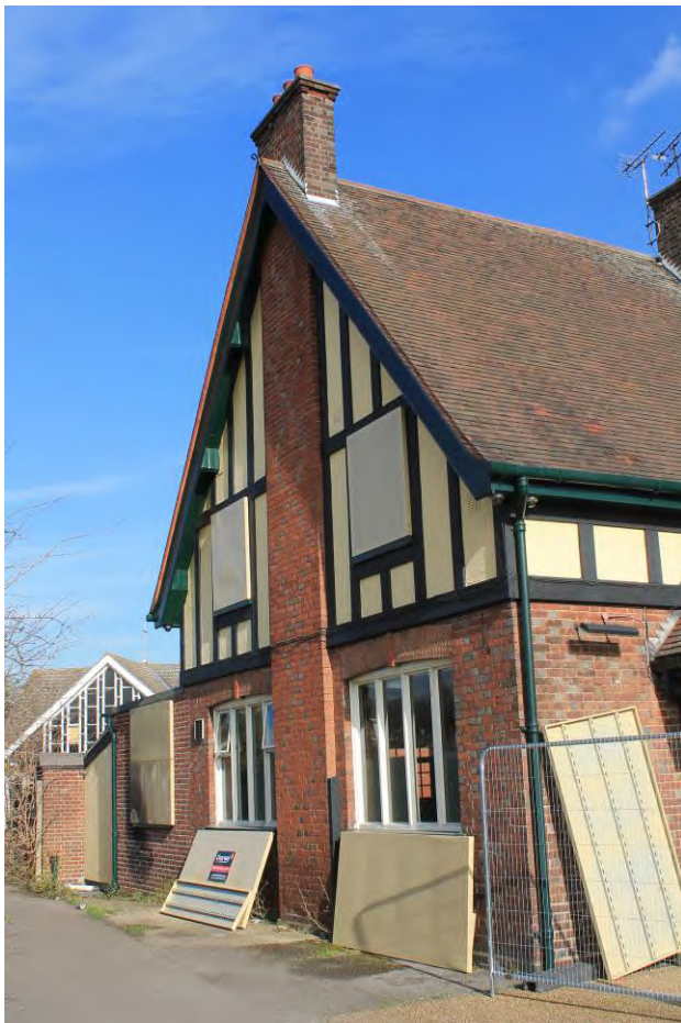
Plate 7 Northern Elevation, looking South-east
