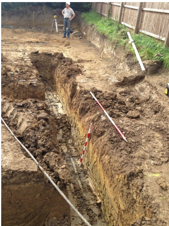
Plate 3: General view of excavated foundations, (south west facing 1x 2m scales)
