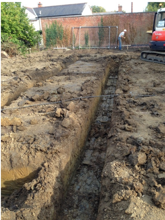
Plate 4: General view of excavated foundations (east facing)
