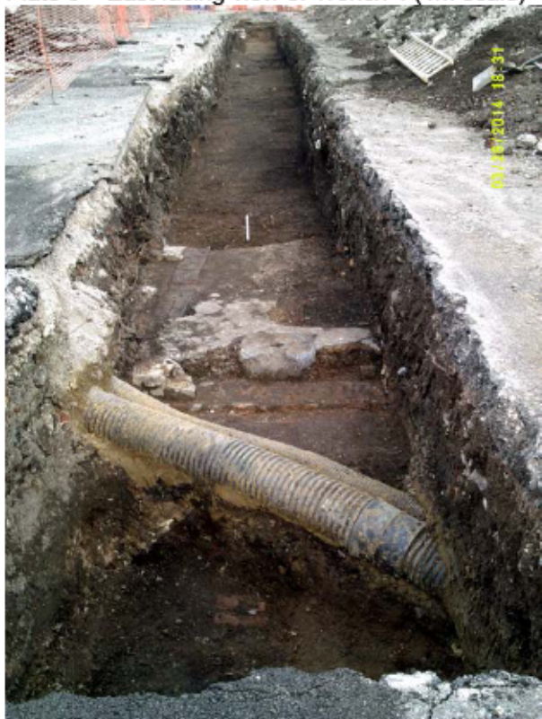
Plate 6 – East facing view of Trench 4 (1m scale)
