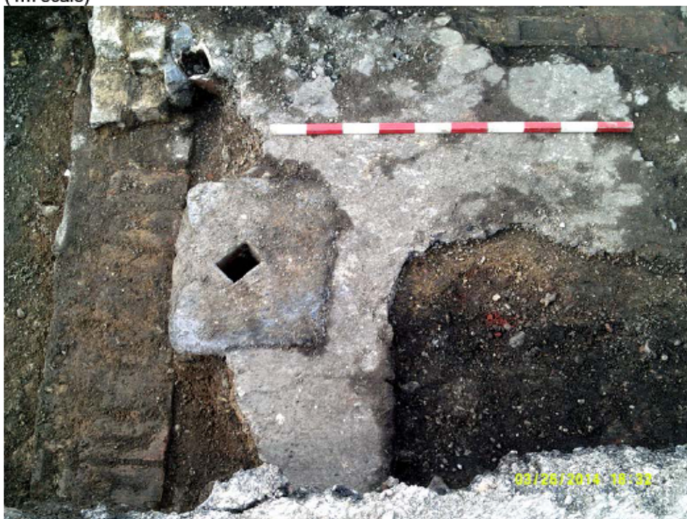
Plate 7 – North facing view of concrete slab [29] and associated walls [28] and [30] in Trench 4 (1m scale)
