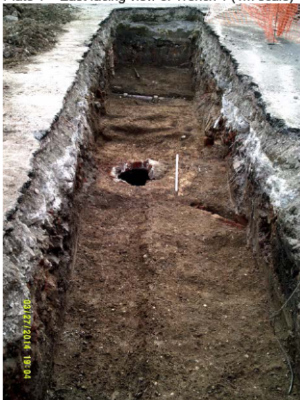
Plate 1 – East facing view of Trench 1 (1m scale)
