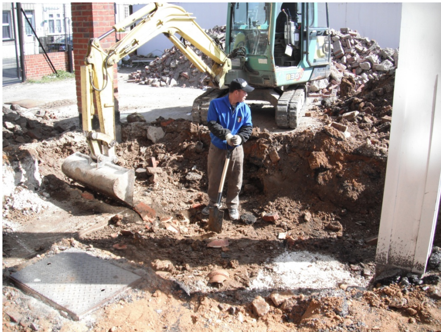
Plate 2. View of site looking north as ground reduction commences.
