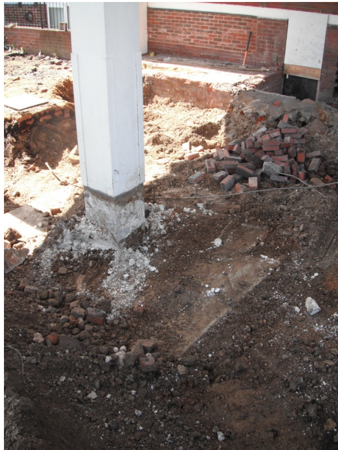
Plate 4. Excavation to -800mm below ground level. Shows extant foundations
