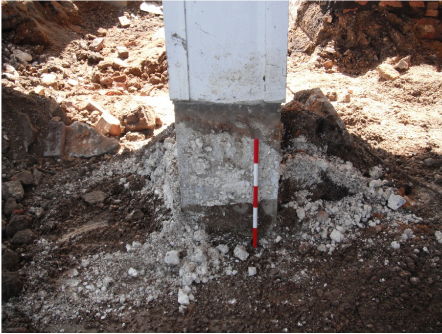
Plate 5. Looking South at existing foundations. 0.5m scale
