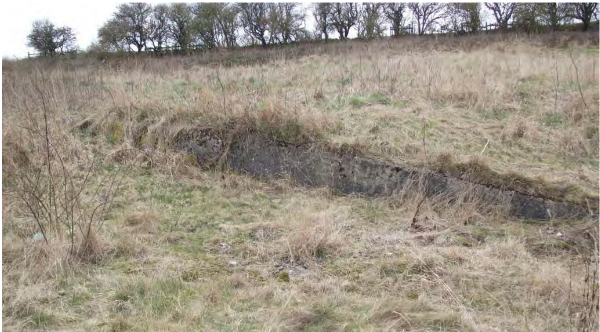
Plate 12. Structural remains (concrete retaining wall) in southern part of site, looking WSW
