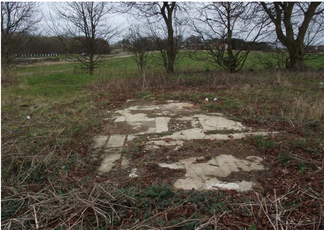
Plate 10. Structural remains (floor of former hospital building) at northern end of site, looking ENE
