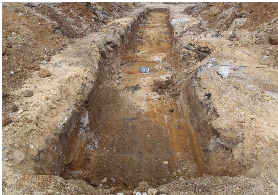
Plate 4: Trench 7, looking northwest. Ditch [15] can clearly be seen cutting from beneath the upper made ground deposits.
