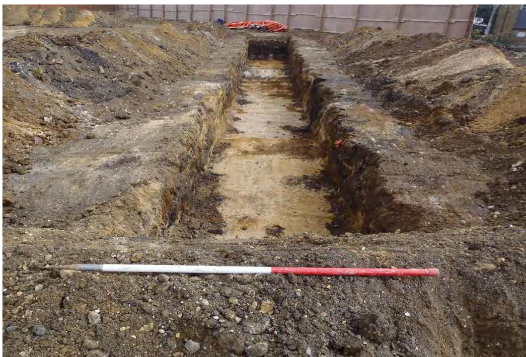
Plate 2: Trench 2 looking east showing truncated natural substrate.
