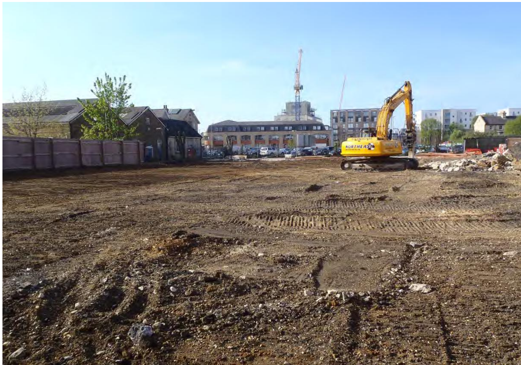
Plate 1: The site before excavation.
