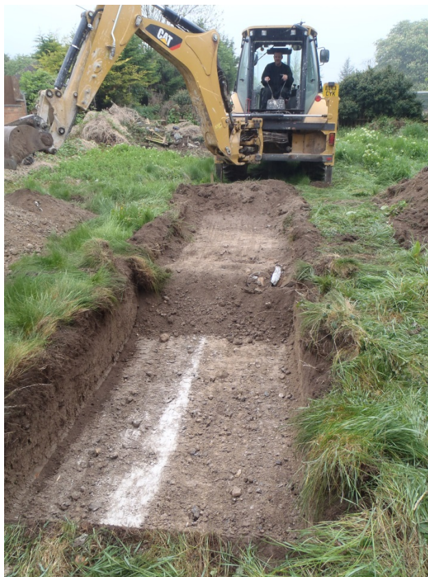
Plate 2: Machine excavation of Trench 1
