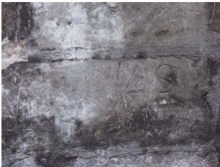
Plate 7: Inverted inscription 'S7' on wall refacing [32]
