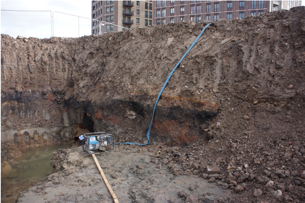
Plate 4: North-east corner of the observed trench in Plot S4, looking north-east
