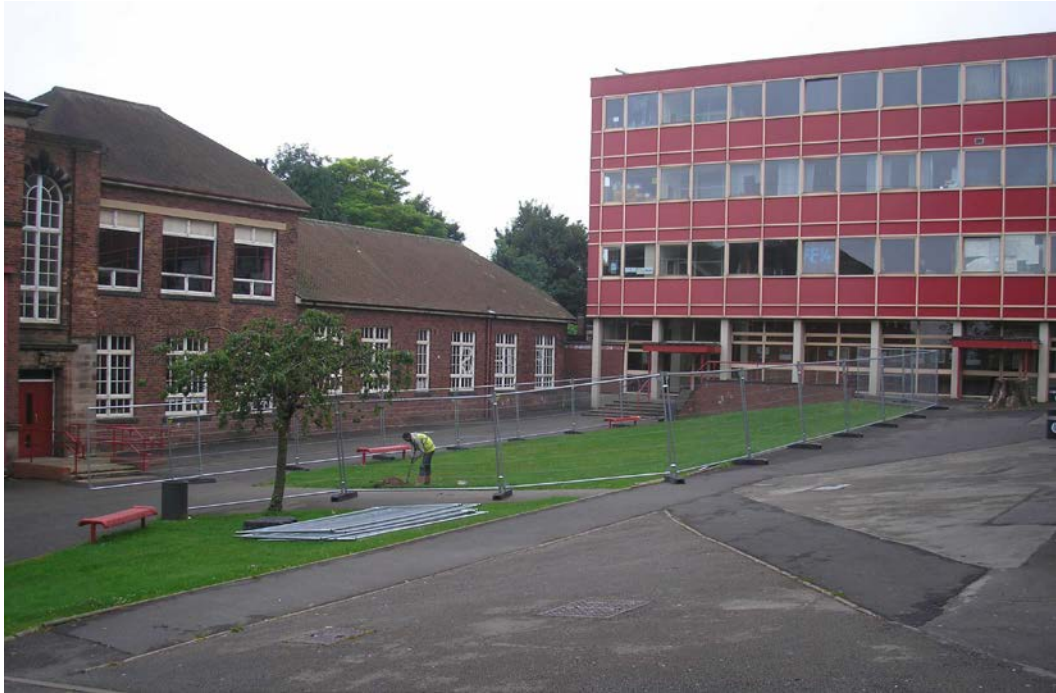
Plate 1: Area 1, Pre-excavation view, looking south-west
