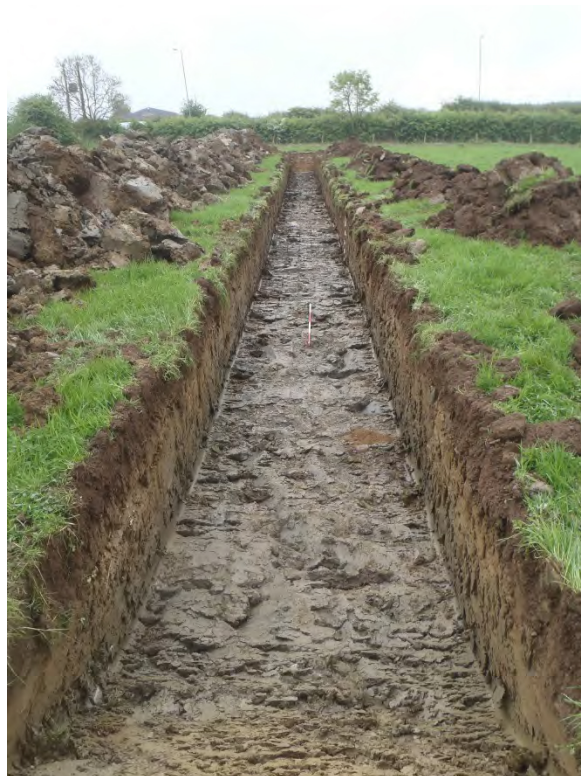
Plate 16: South facing view of Trench 12
