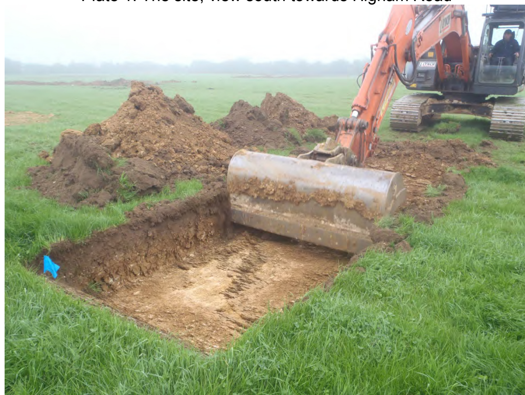
Plate 2: Machine excavation, 22 tonne excavator
