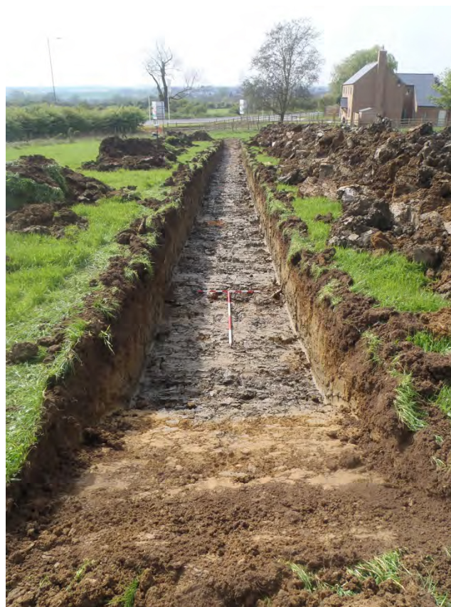
Plate 17: West facing view of Trench 13
