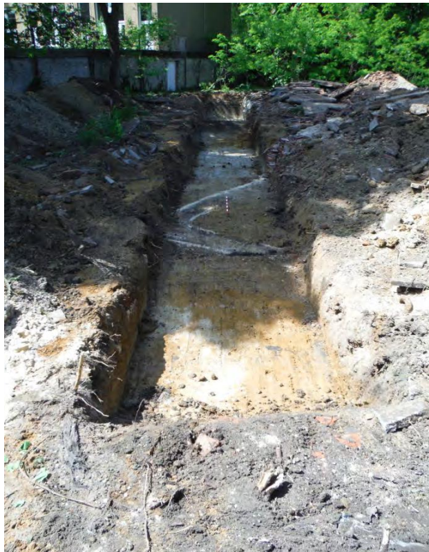
Plate 3: Trench 1, looking southwest
