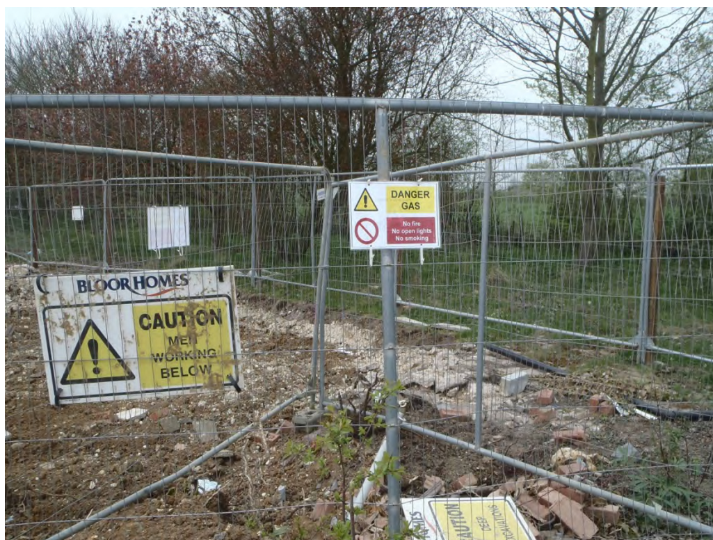
Plate 3: Gas pipes limiting excavation, view north-west
