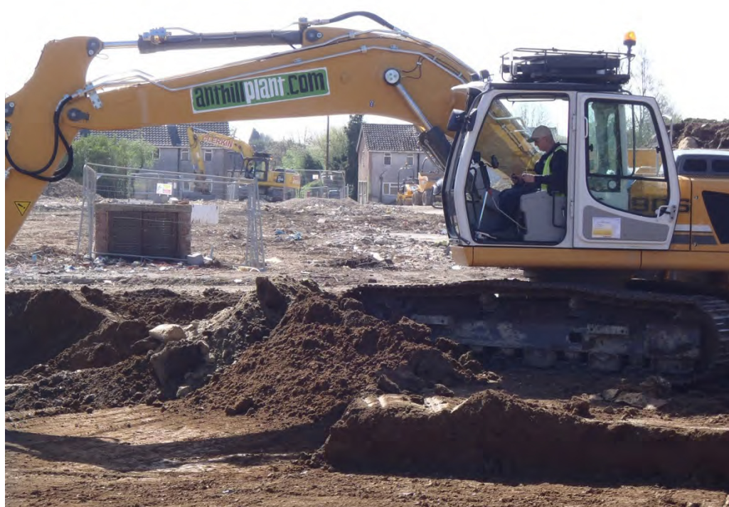
Plate 4: Subsoil removal, view south
