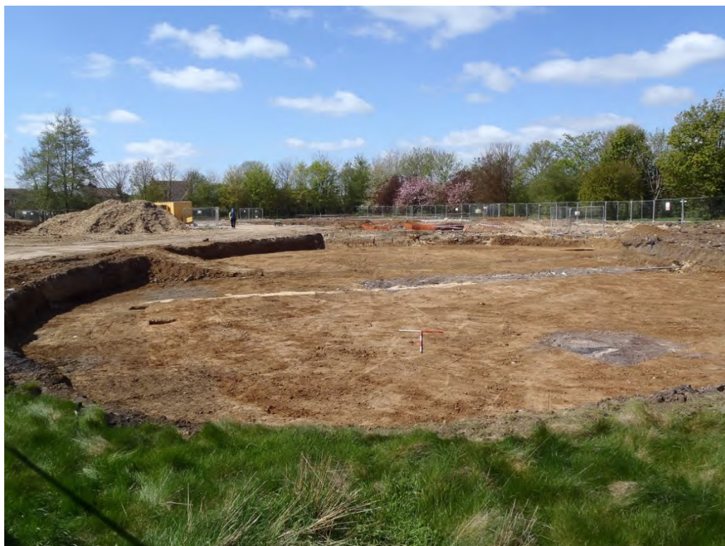
Plate 5: Excavation area, view west from south-east corner
