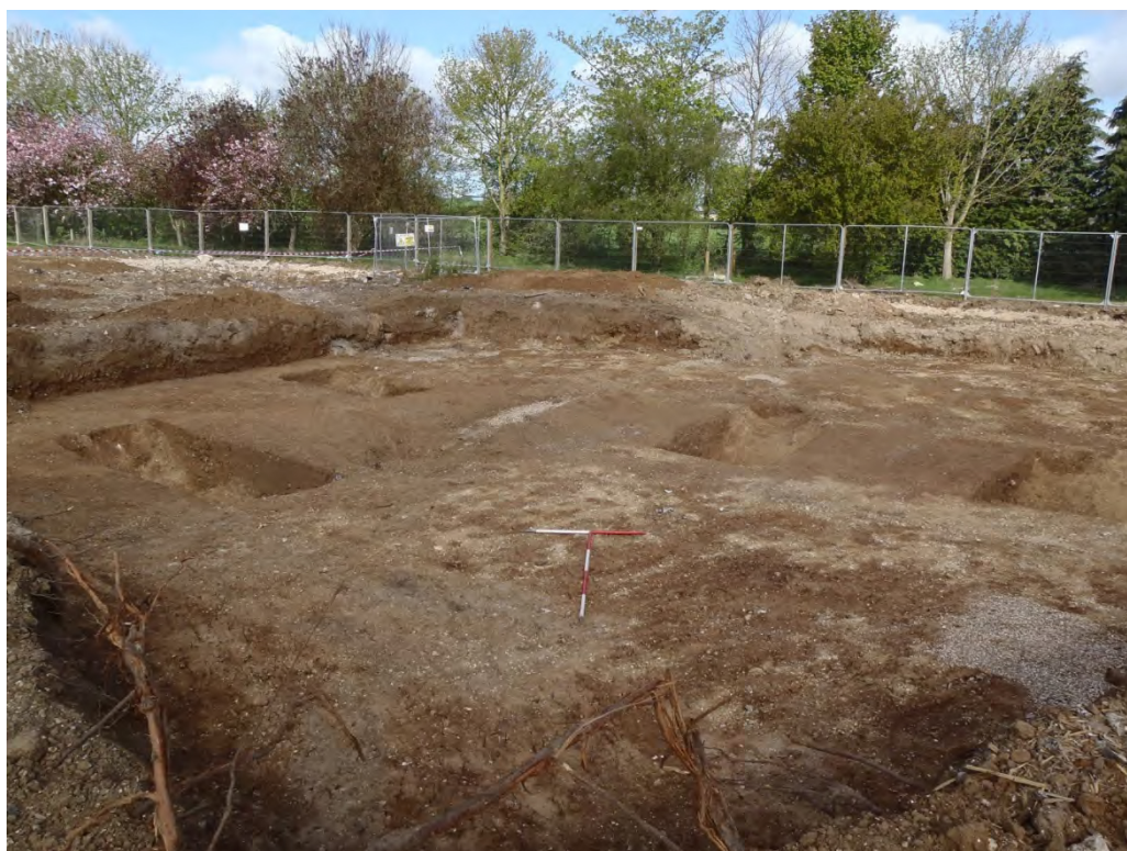
Plate 10: Site post-excavation (central area), view north-west
