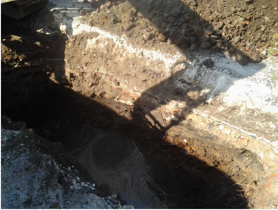
Plate 3: Section 2 in Trench 2
