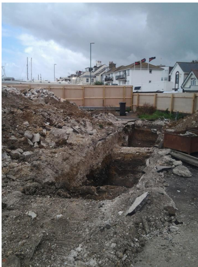
Plate 1: Trench 1 under excavation, looking north-west
