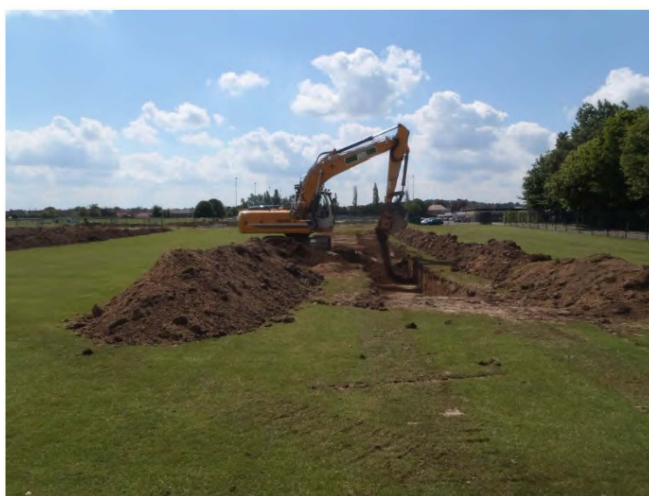
Plate 23: Trench backfilling
