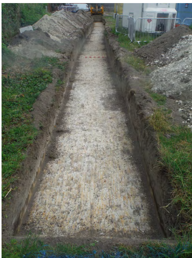
Plate 4: Trench 1, view south-east
