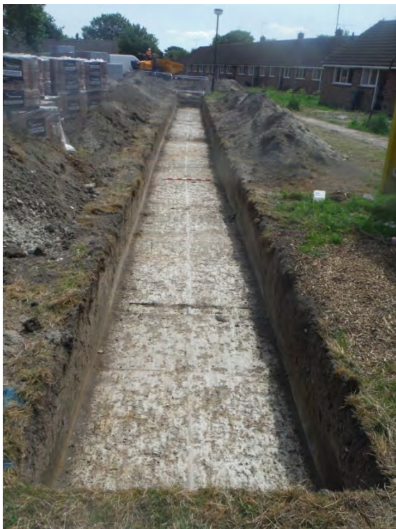
Plate 5: Trench 2, view south-east
