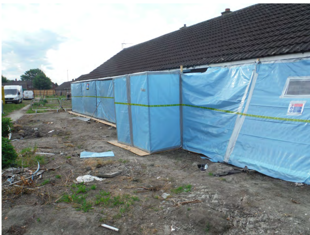
Plate 2: Existing structures on site, view south-east
