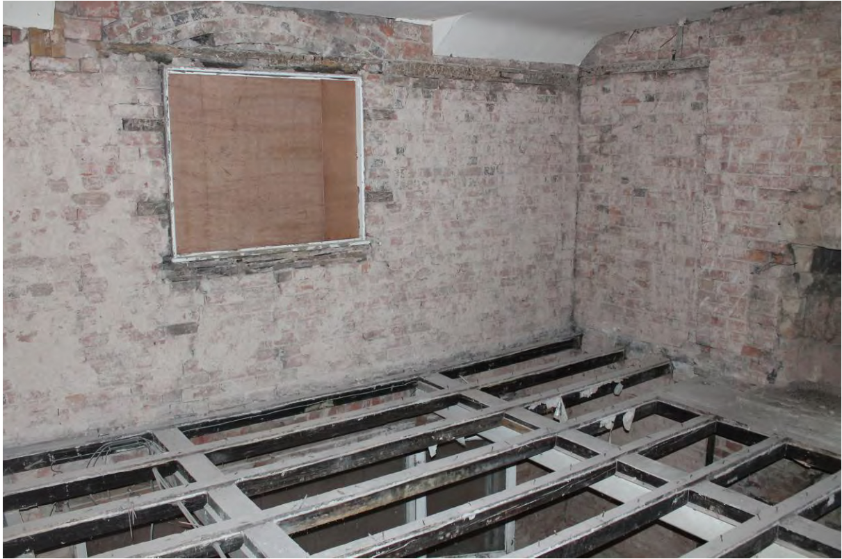
Plate 23 First floor room F1 looking north-east
