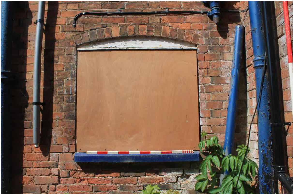
Plate 9 Eastern elevation ground floor window (original opening)
