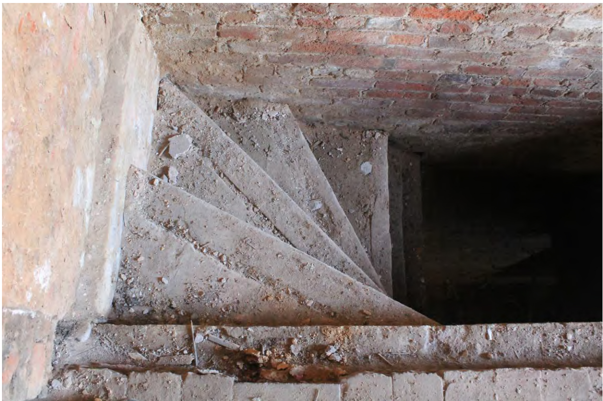
Plate 14 Stone steps to basement (G3)
