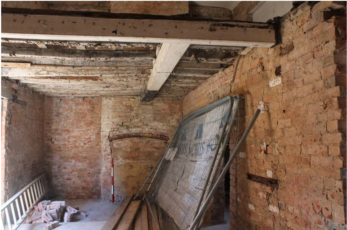
Plate 17 Room G2 looking south
