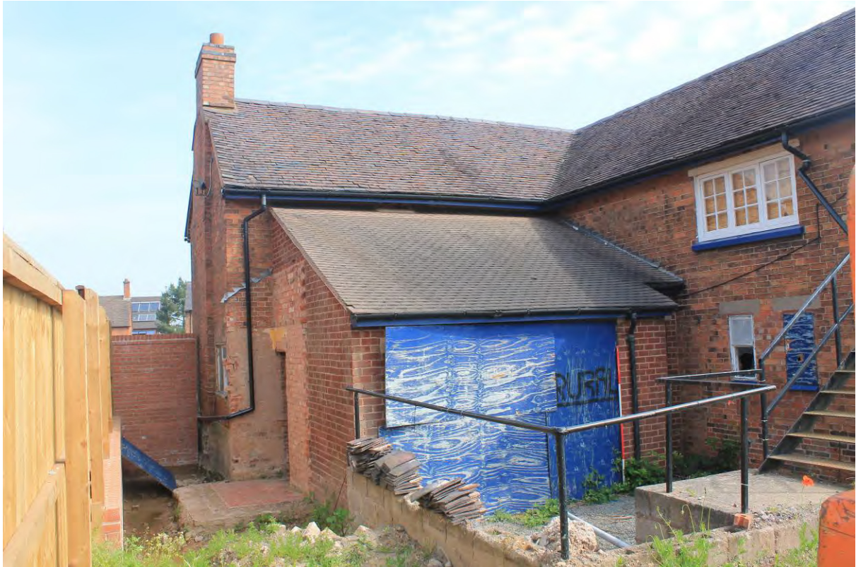
Plate 5 Western elevations and modern lean-to extension
