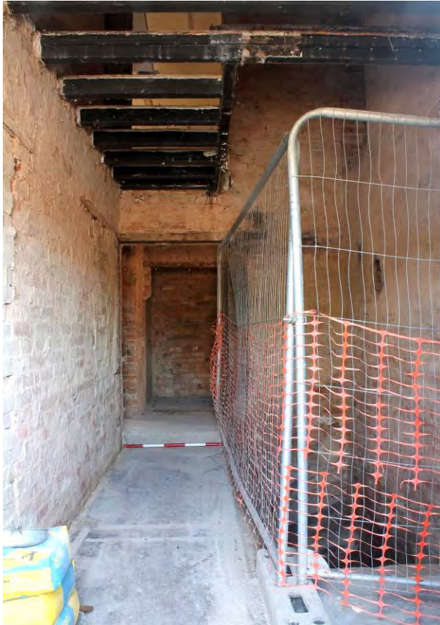
Plate 13 Entrance bay G3 looking south (entrance to basement to right)
