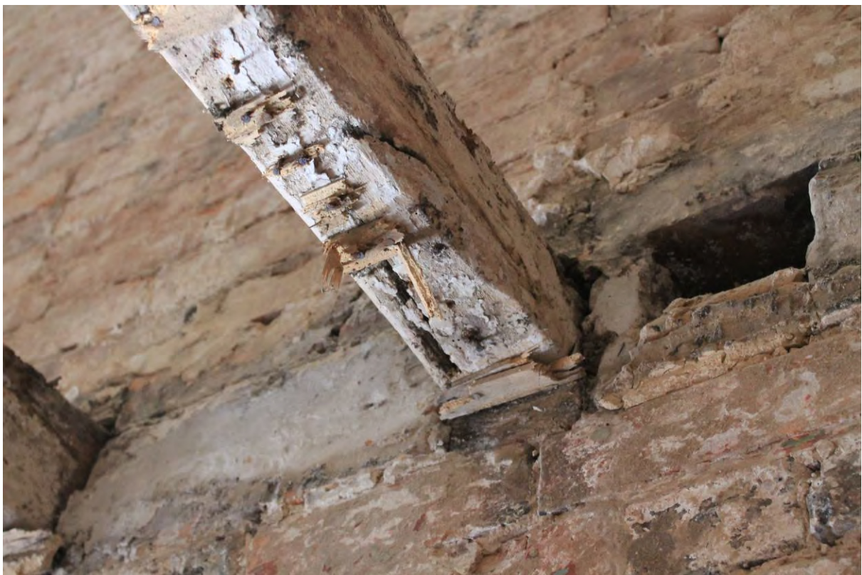
Plate 20 Chamfer and stop to common joist (G2)
