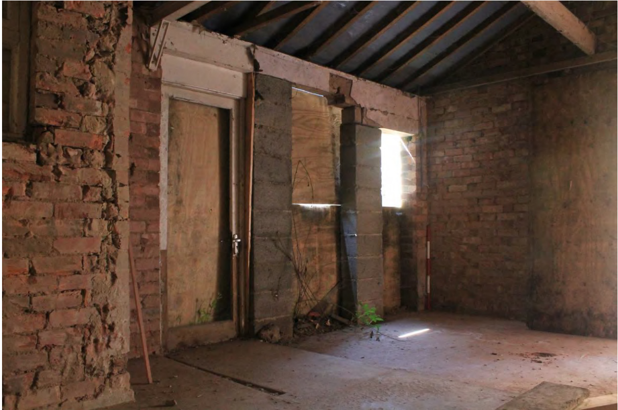
Plate 21 Modern lean-to addition (G5) looking south-west
