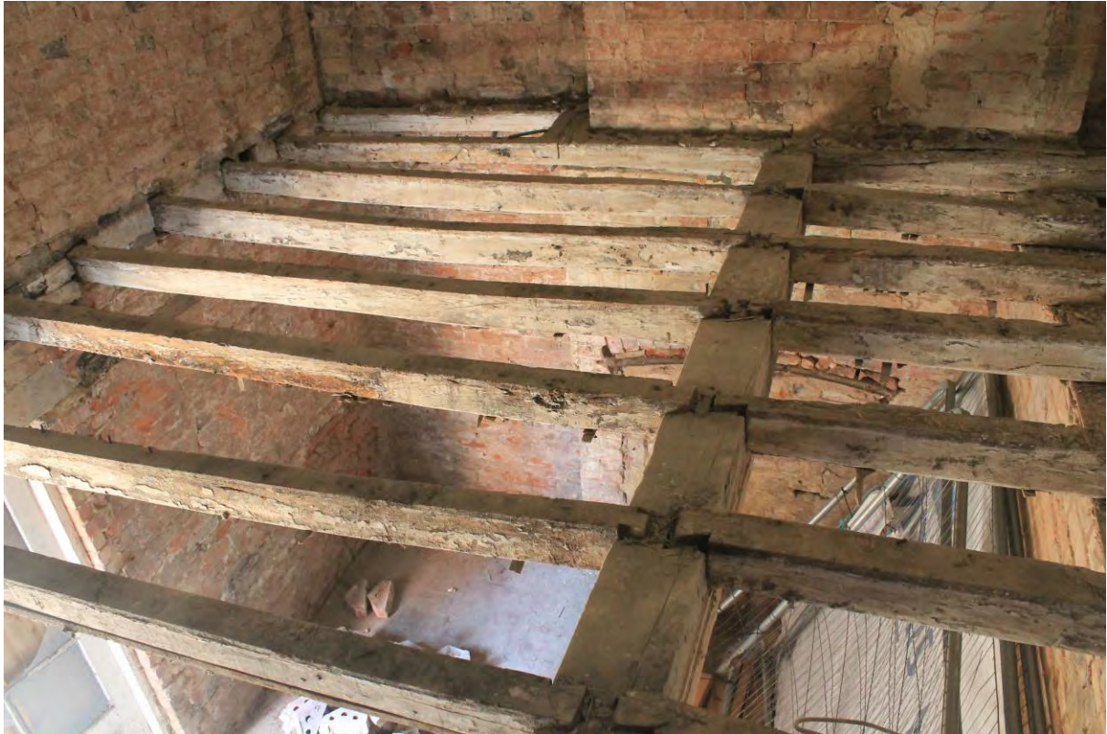
Plate 19 First floor structure over G2
