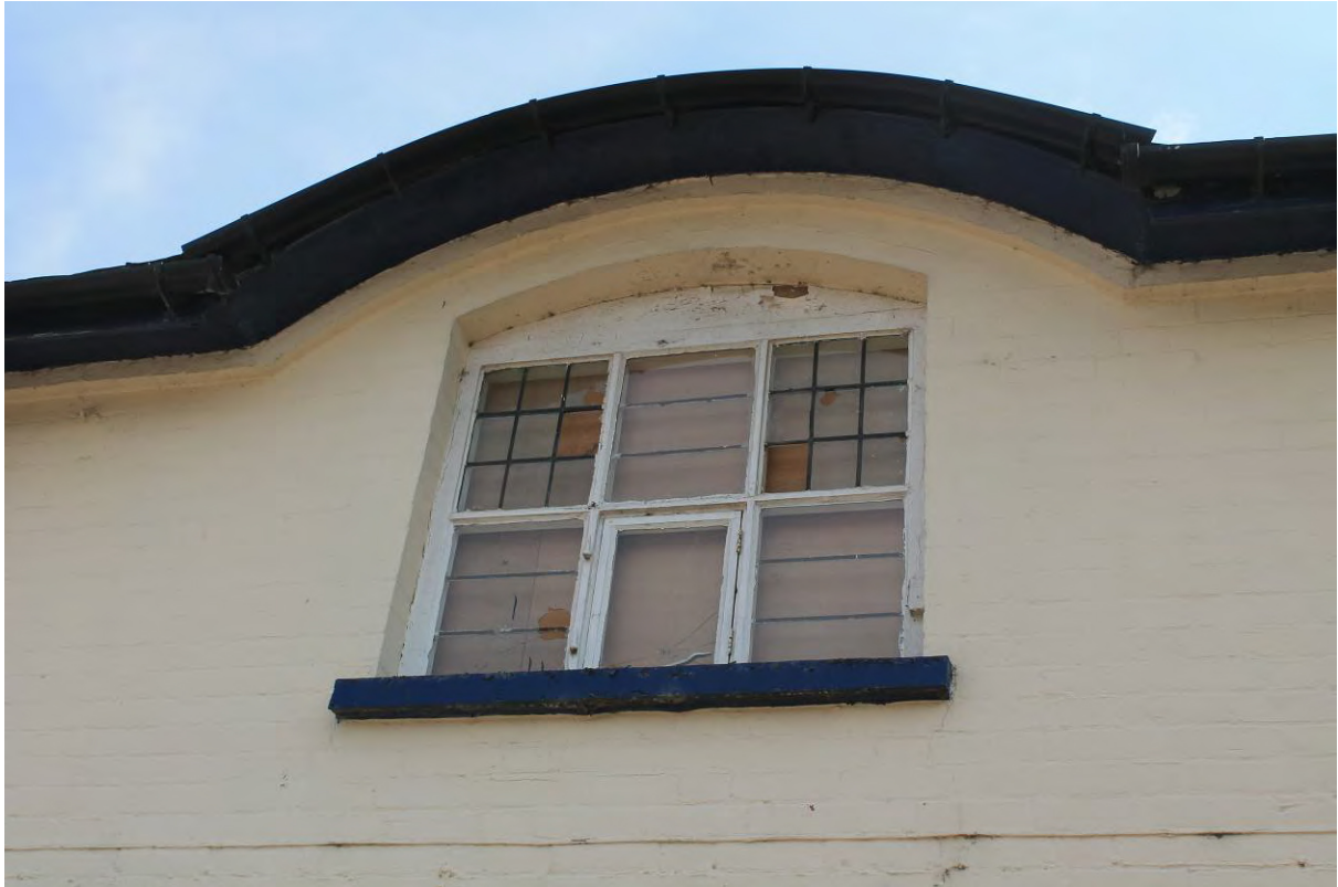
Plate 11 Eyebrow dormer style first floor window
