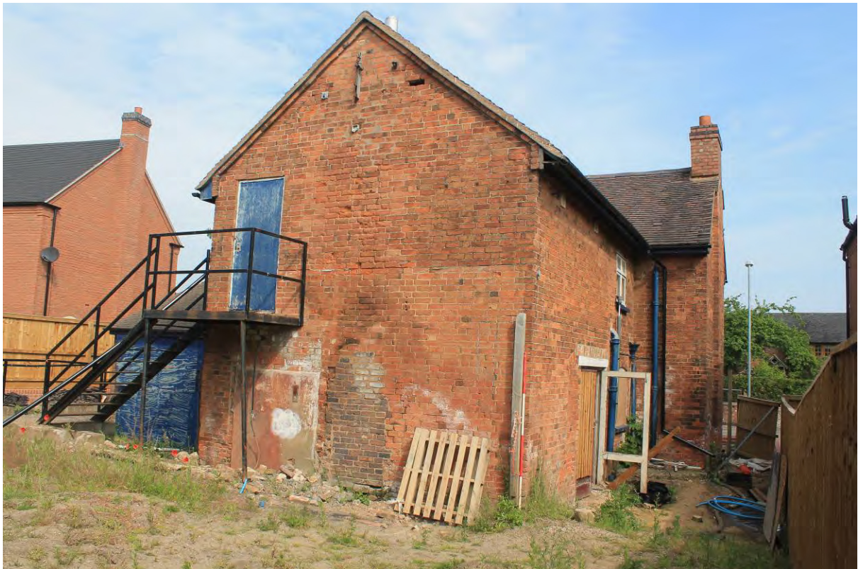
Plate 8 Eastern elevation and southern gable elevation
