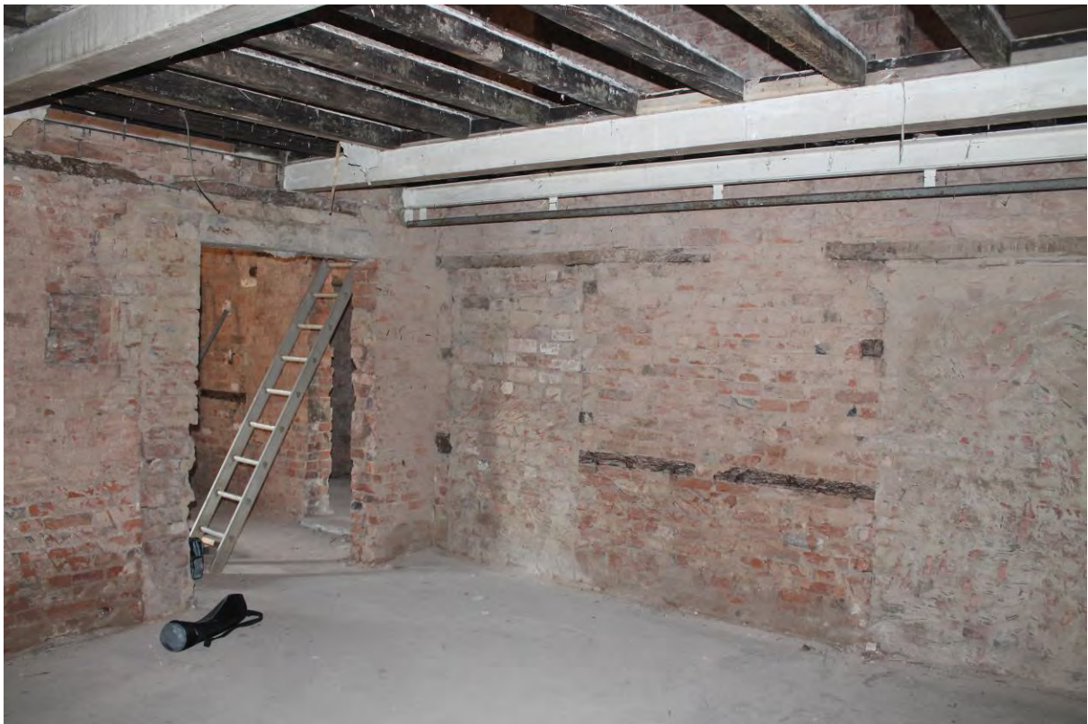
Plate 12 Room G1 looking south-west and showing blocked door openings
