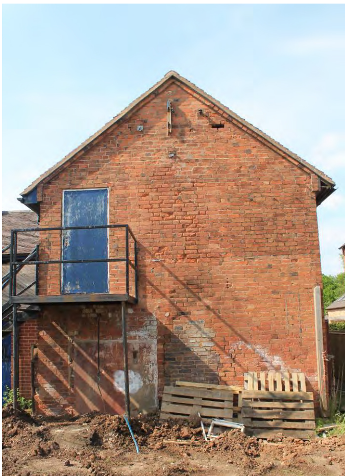
Plate 10 South gable elevation
