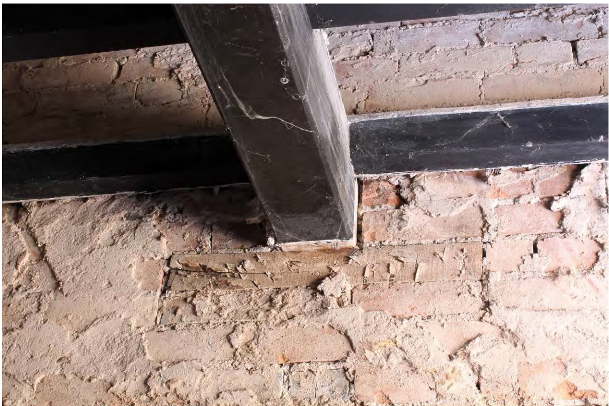
Plate 16 First floor binding joist and timber bearer (G6)
