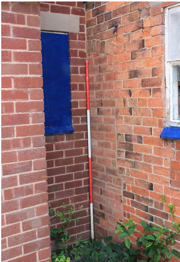
Plate 6 Partially built-over blocked door opening in western wall of rear projection
