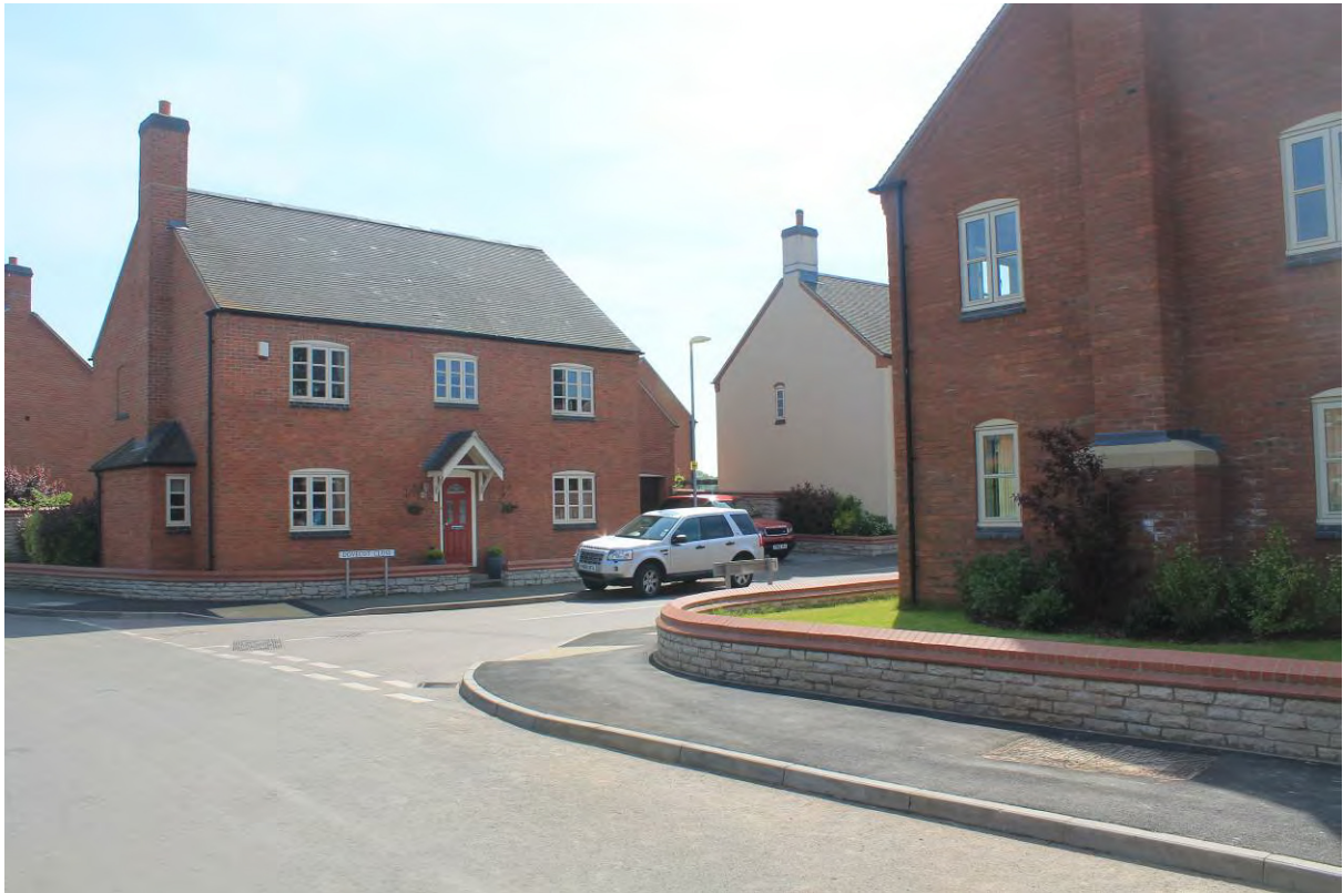
Plate 1 Modern development at Dovecote Close, east of site
