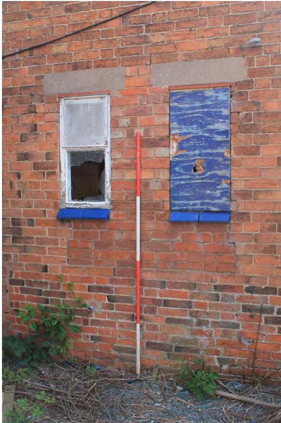
Plate 7 Blocked window and later inserted toilet windows, west wall, rear projection
